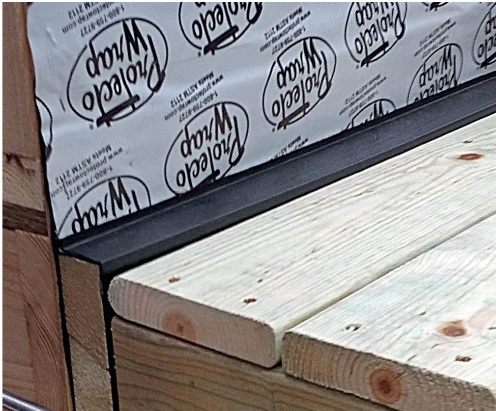
A cutaway view of ledger flashing.
