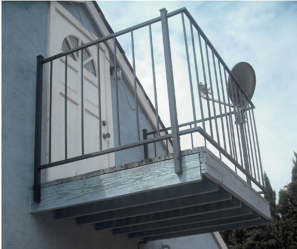
A cantilevered balcony.
