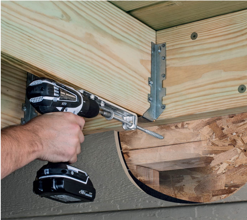
Simpson Strong-Tie DTT1 installed. Photo courtesy Simpson Strong-Tie.
