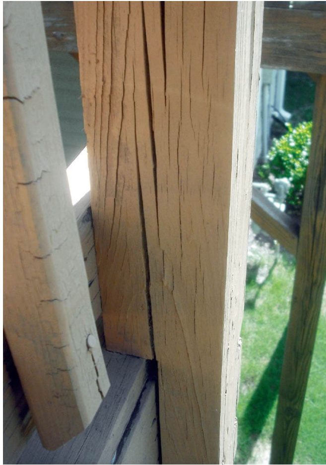
Notched deck guard posts can split at the notch and fail.
