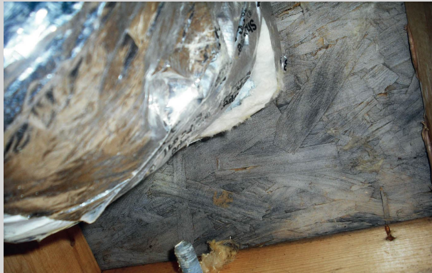
Water stains under an improperly flashed door.
