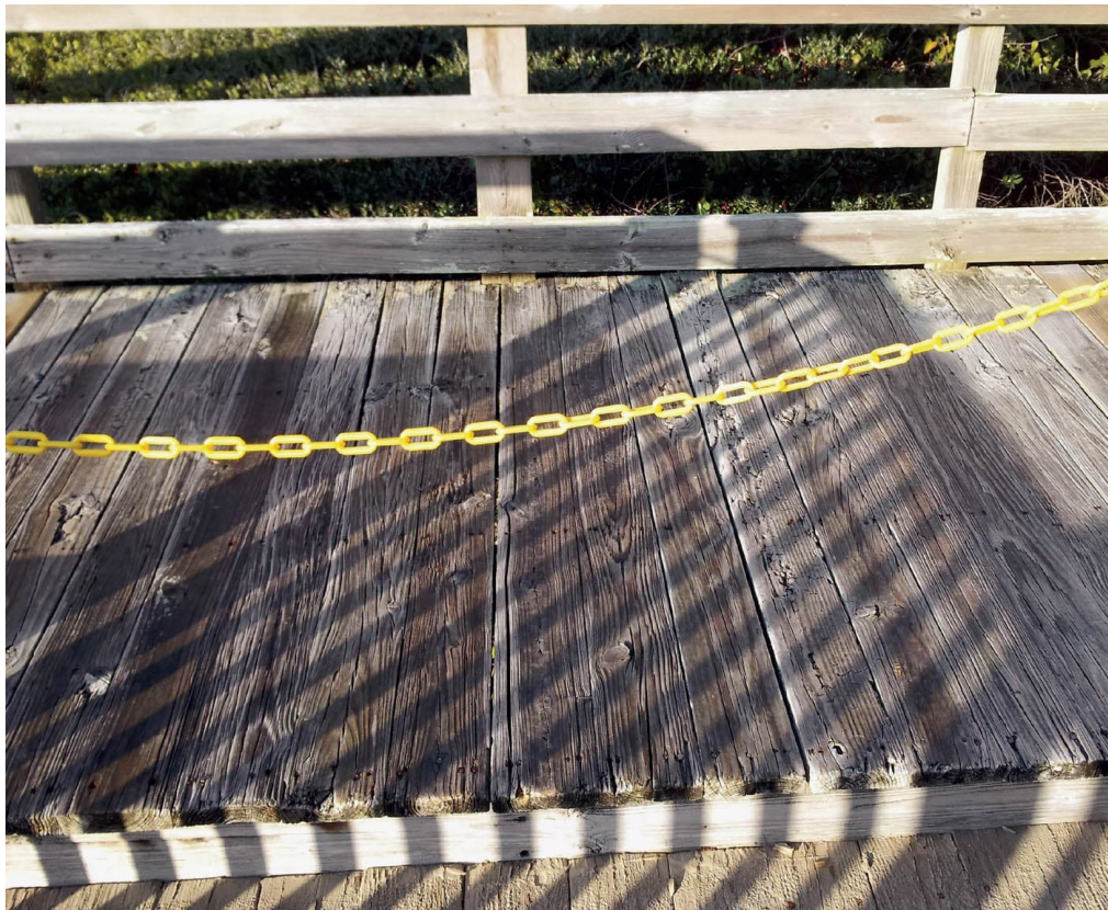
Severely deteriorated decking.
