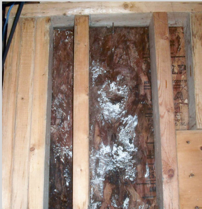
Water damage under improperly flashed deck ledger.
