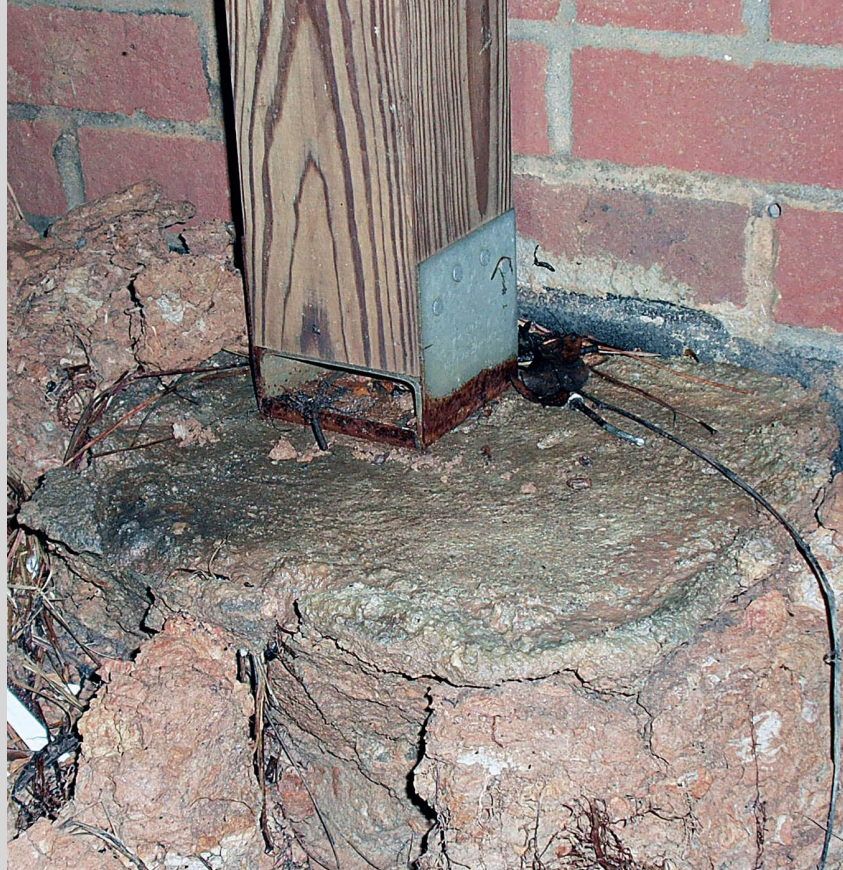
Deck post is off center on footing. Post base is rusted. Footing is too small.
