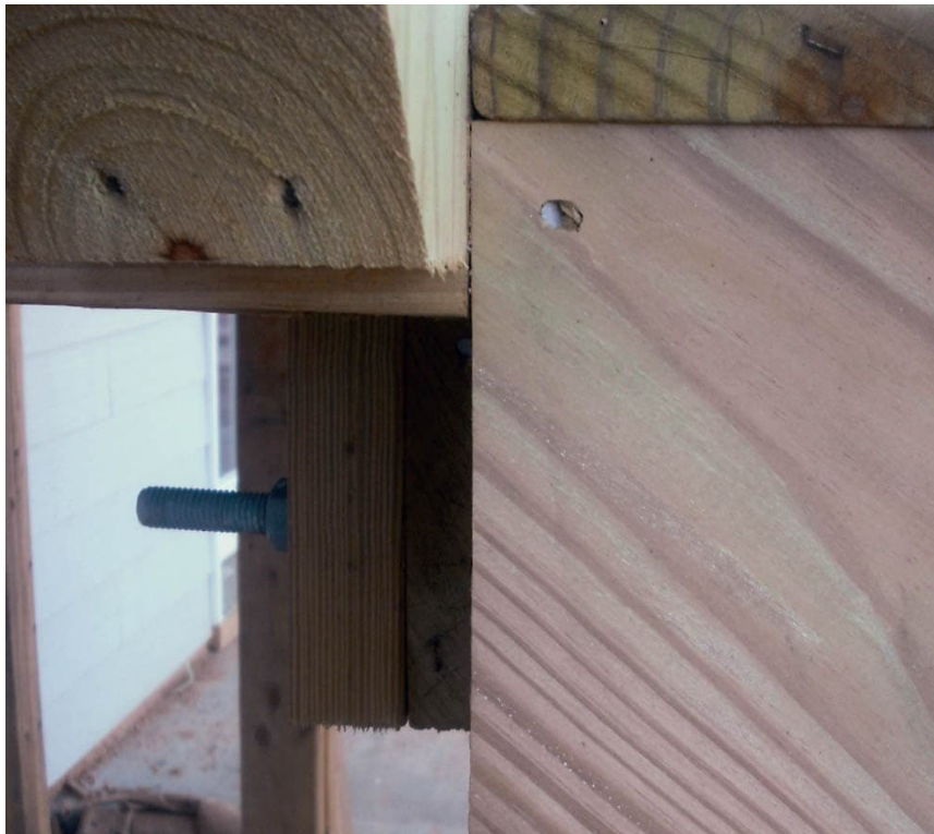
Stringer plumb cut is not in full contact with deck rim joist.
