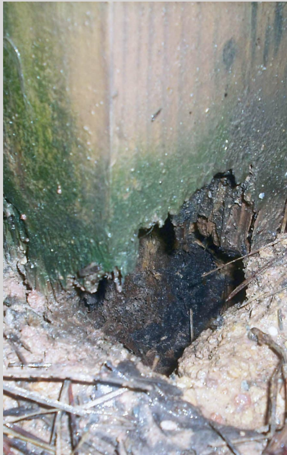
Deteriorated deck post.
