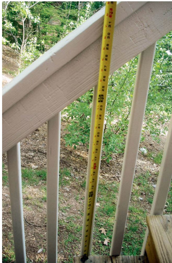
A deck stair guard should be at least 34" above the tread leading edge.
