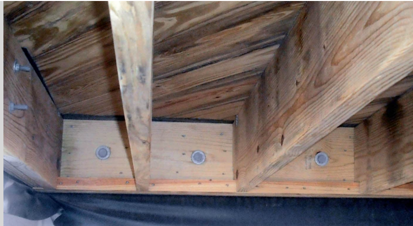
Deck ledger attachment bolts are not staggered as they should be.
