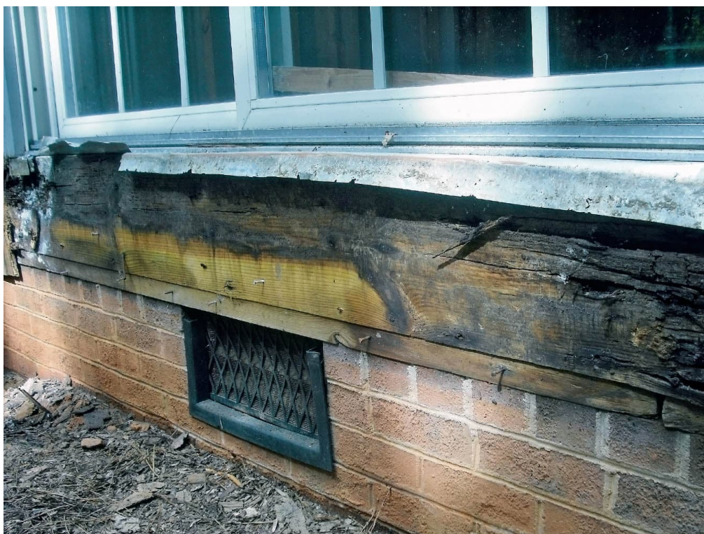
House rim joist is rotted due to improper flashing.
