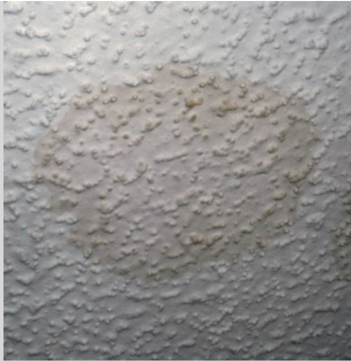
Water stains on a ceiling below an improperly flashed deck ledger.
