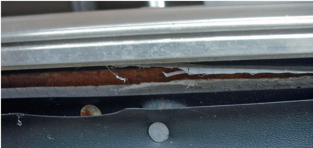
Gap in flashing under door threshold.
