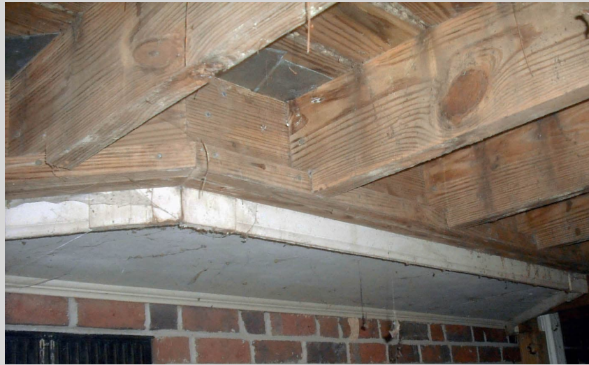
Deck ledger may not be attached to cantilevered framing.
