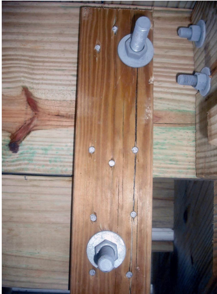
Example of bolted drop header. Vertical 2 \times 4 is split and should be replaced. Bolts should be located near the center of the 2 \times 4 and should be located at least 2" from the bottom of the deck rim joist.
