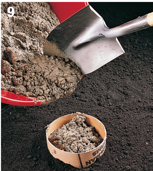
Pour concrete slowly into the tube form , guiding concrete from the wheelbarrow with a shovel. Fill about half of the form, using a long stick to tamp the concrete, filling any air gaps in the footing. Then finish pouring and tamping concrete into the form.
