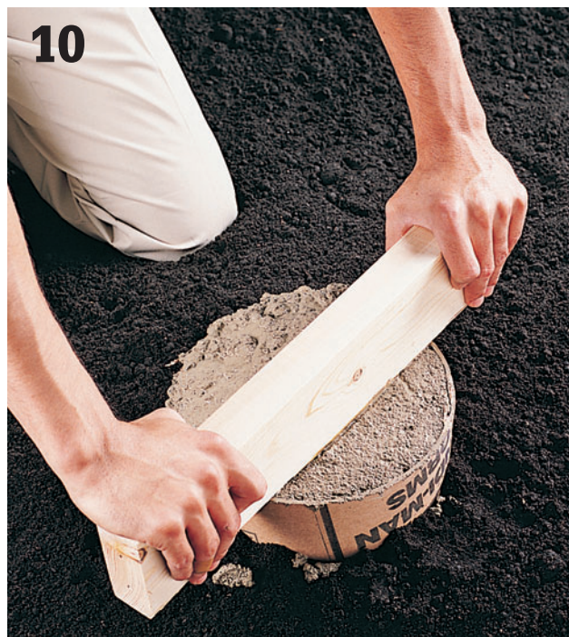
Level the concrete by pulling a 2 × 4 across the top of the tube form, using a sawing motion. Add concrete to any low spots. Retie the mason's strings on the batterboards, and recheck measurements.
