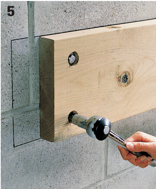
Attach ledger to wall with 3/8 x 4" lag screws and washers, using a ratchet wrench or impact driver. Tighten screws firmly, but do not overtighten.
