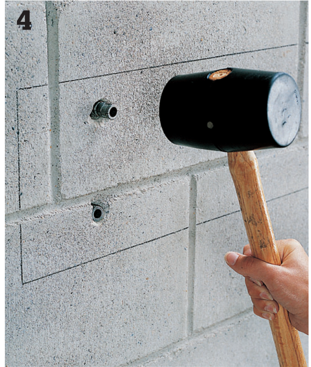
Drive lead masonry anchors for 3/8" lag screws into drilled holes, using a rubber mallet.
