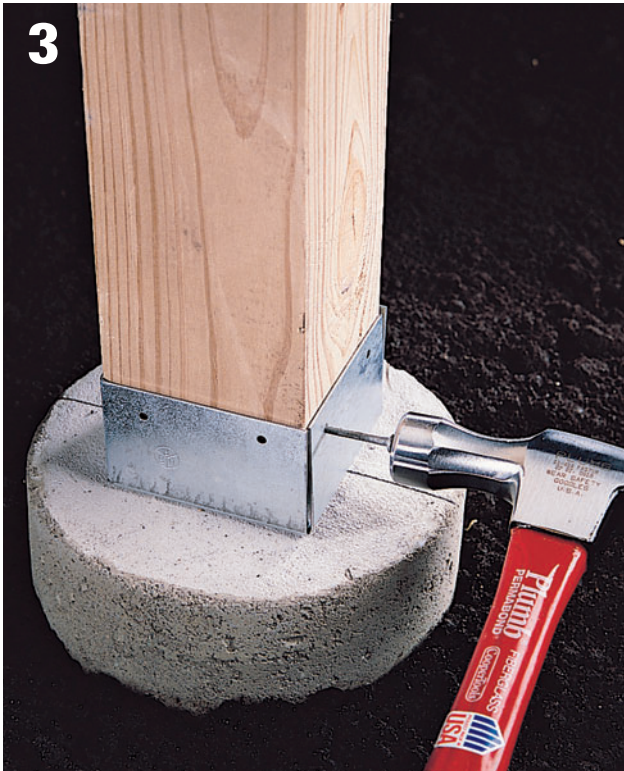
3 Place post in anchor, and tack into place with a single 6d galvanized common nail.
