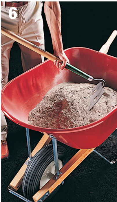
Mix dry ingredients for concrete in a wheelbarrow, using a hoe.
