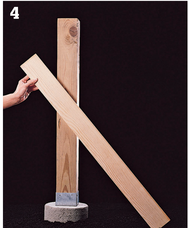
4 Brace post with a 1 × 4. Place the 1 × 4 flat across post so that it crosses the post at a 45° angle about halfway up.
