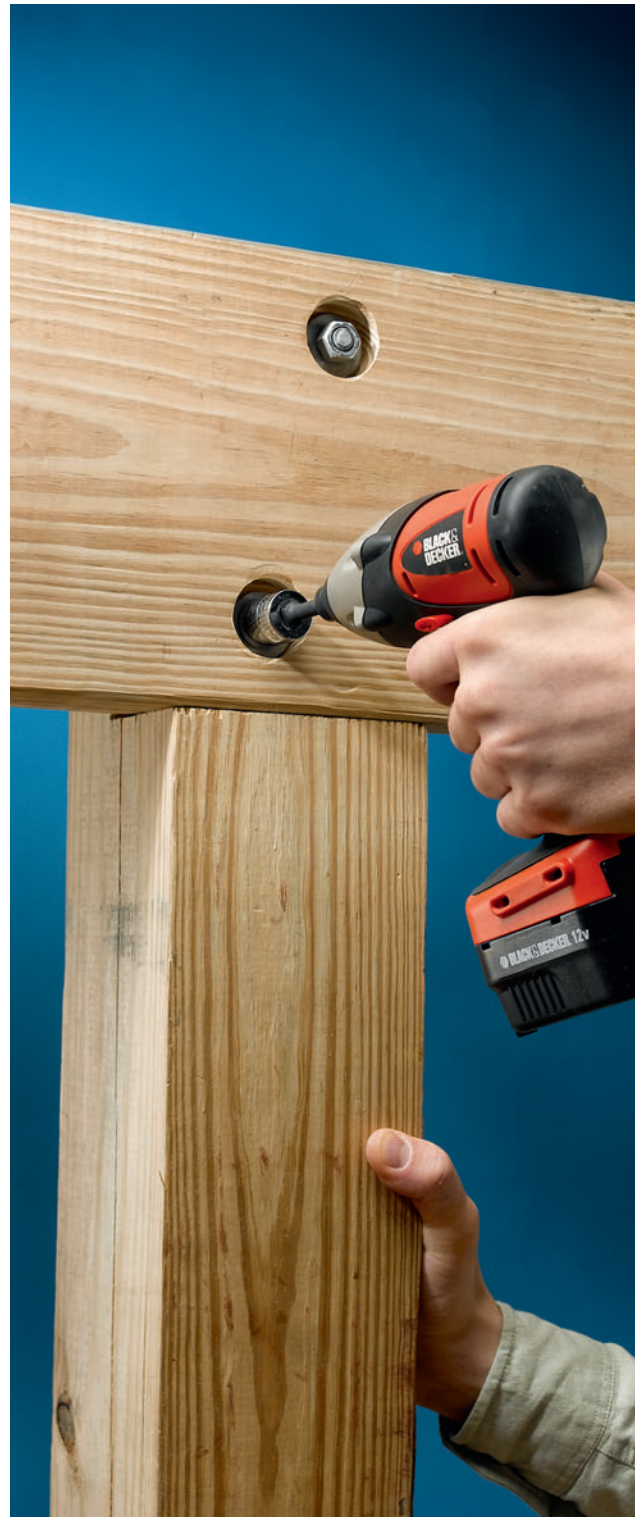
Deck beams , resting in a notch on the tops of the posts and secured with through bolts and nuts, guarantee strong connections that will bear the weight of your deck.
