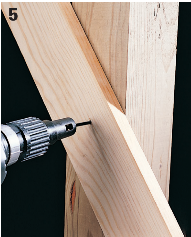
5 Attach the brace to the post temporarily with a single 2" wallboard screw.
