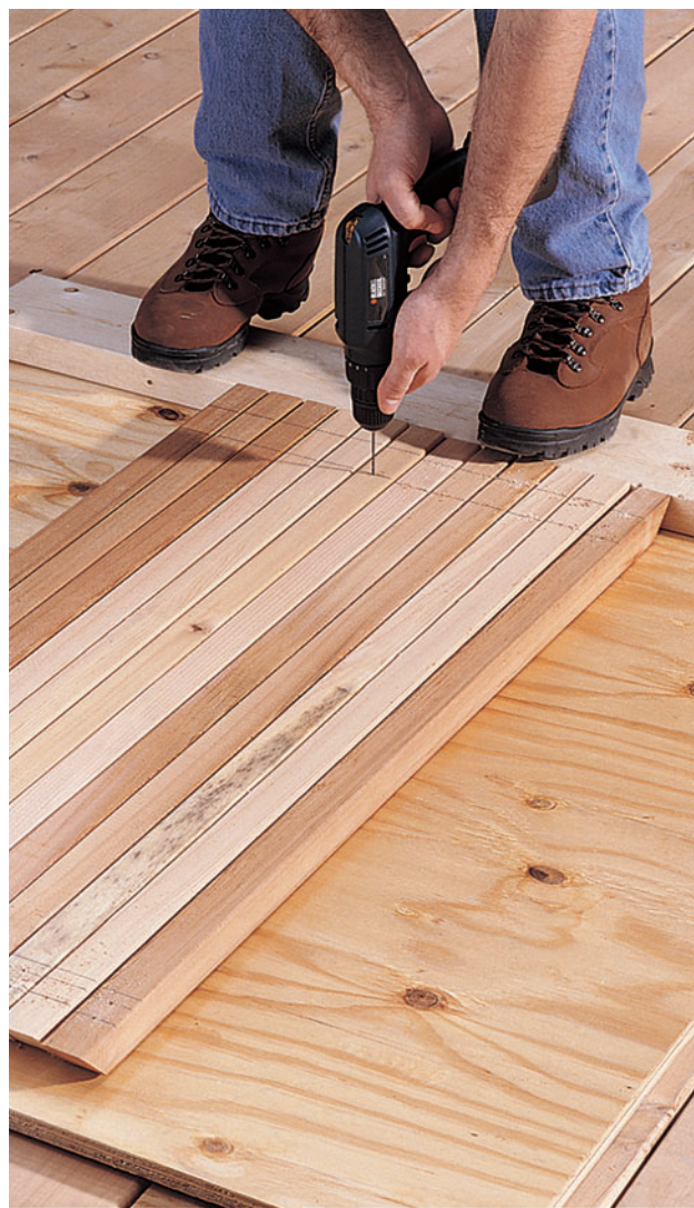
After cutting balusters to length , gang them up and drill ¼" pilot holes through the top and bottom.
