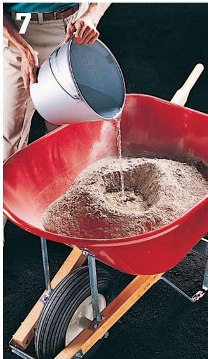
Form a hollow in center of dry concrete mixture. Slowly pour a small amount of water into hollow, and blend in dry mixture with a hoe.
