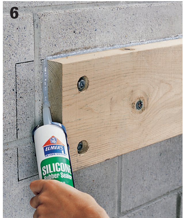
Seal the cracks between the wall and ledger with silicone caulk. Also seal the lag screw heads.
