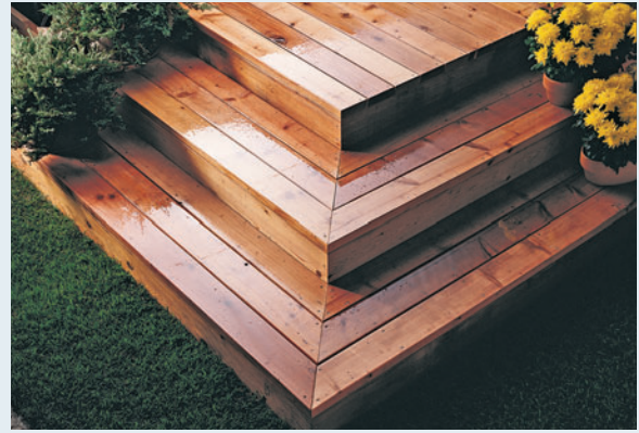
Platform steps feature wide treads. Each step is built on a framework of posts and joists.
