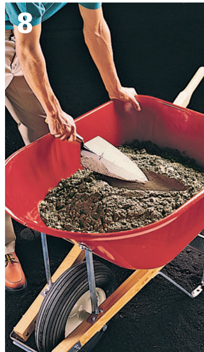
Add more water gradually , mixing thoroughly until concrete is firm enough to hold its shape when sliced with a trowel.
