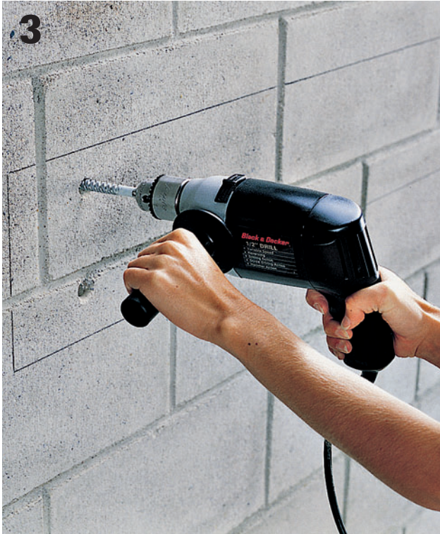
Drill anchor holes 3" deep into masonry, using a 5/8" masonry bit.
