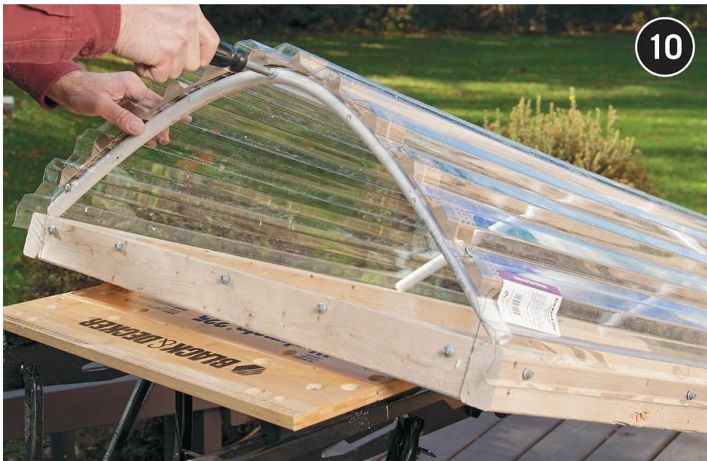
**Set the clear acrylic end panels in place,** butting them against the filler at the top. Mark screw locations. Place the panel on a piece of plywood and predrill with a  $\frac{1}{4}$ " diameter bit to avoid cracking the clear acrylic, which isn't as soft or flexible as the polycarbonate. Screw the panels in place with roofing screws, hand-tightening with a screwdriver to avoid cracking the clear acrylic. Don't overtighten.
