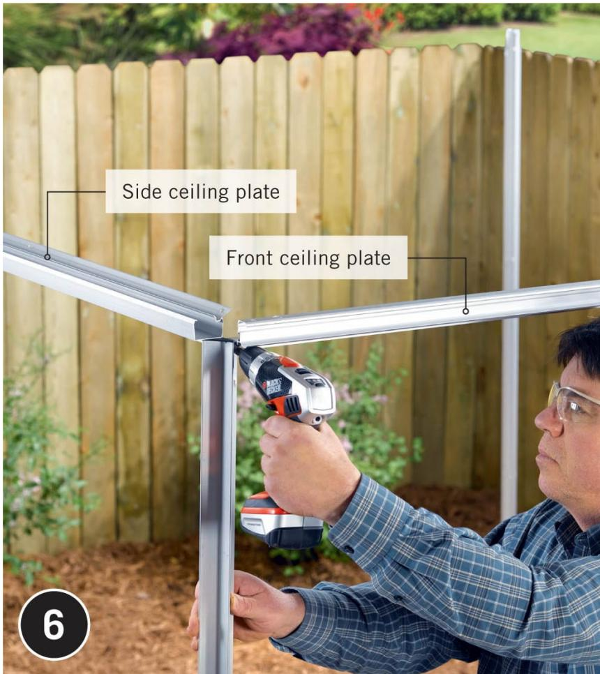
**Install the ceiling plates:** Assemble the pieces for each side ceiling plate. Attach each side plate against the inside of the two corner studs along each side of the greenhouse, making sure the gutter is positioned correctly. Attach the front ceiling plate to the outsides of the corner studs at the front of the building.
