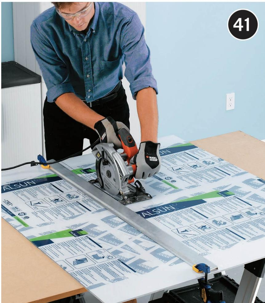
**Make the greenhouse windows.** First, cut the window glazing panels ( $\frac{1}{4}$ " clear polycarbonate is used here) using a circular saw and a straightedge guide. The glazing should equal the full height and width of the window. For convenience, this greenhouse was designed with all six windows exactly the same size.
