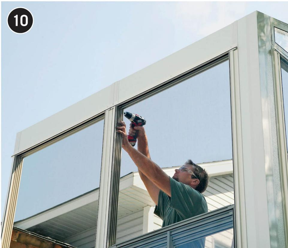
**Install the remaining wall panels,** creating corners and adding upper wall tracks as you go. Frequently check for plumb and level, and make sure all panels are seated firmly in the tracks.
