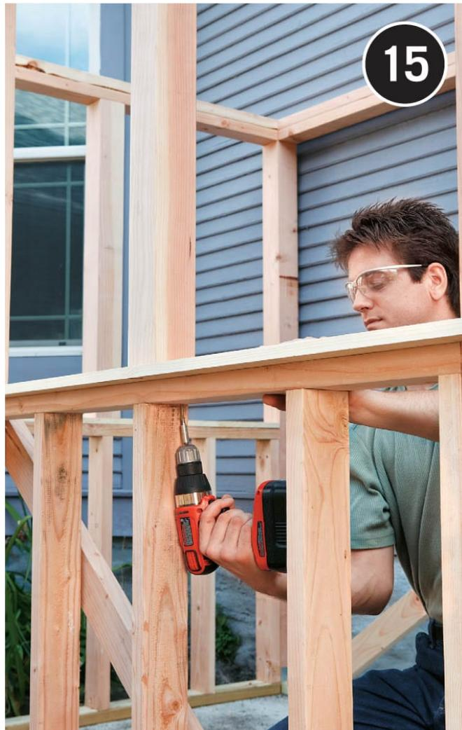
**Add intermediate  $4 \times 4$  posts** between the sills and the undersides of the doubled cap plates. These posts should be situated directly above kneewall studs. The posts are spaced so the distances between posts will create uniform-width bays for the windows.
