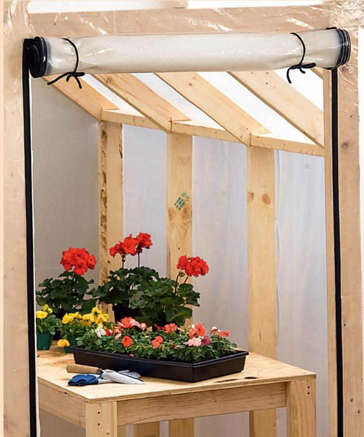
**Plastic door kits**, available from greenhouse suppliers, include self-adhesive zipper strips and are easy to roll up and tie for access or ventilation. You can also create your own roll-up door with zipper strips and plastic sheeting purchased from a building center.
