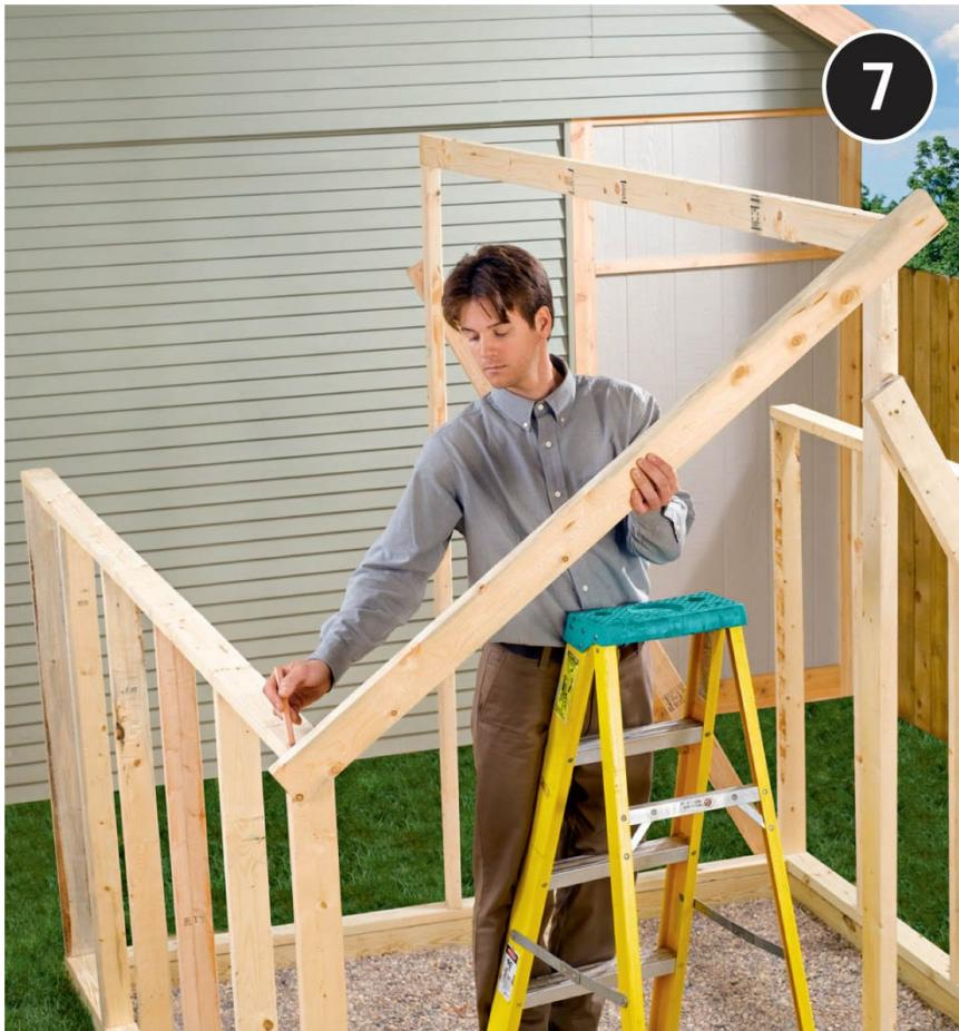
**Create a template rafter** by cutting a  $2 \times 4$  at about 66". Hold the board against the end of the ridge and the top outside corner of a wall cap. Trace along the face of the ridge and the cap to mark the cutting lines for the rafter. Cut along the lines, then test-fit the rafter and make any necessary adjustments for a good fit.
