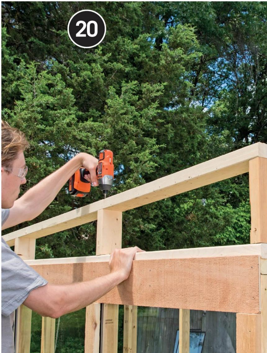
**Measure and cut the other cripple studs** in each top wall and toe-screw them in place with 2½" deck screws. Check that each is plumb and square to the top plate. Miter each end of the top plates and screw them to the cripple studs on each wall.
