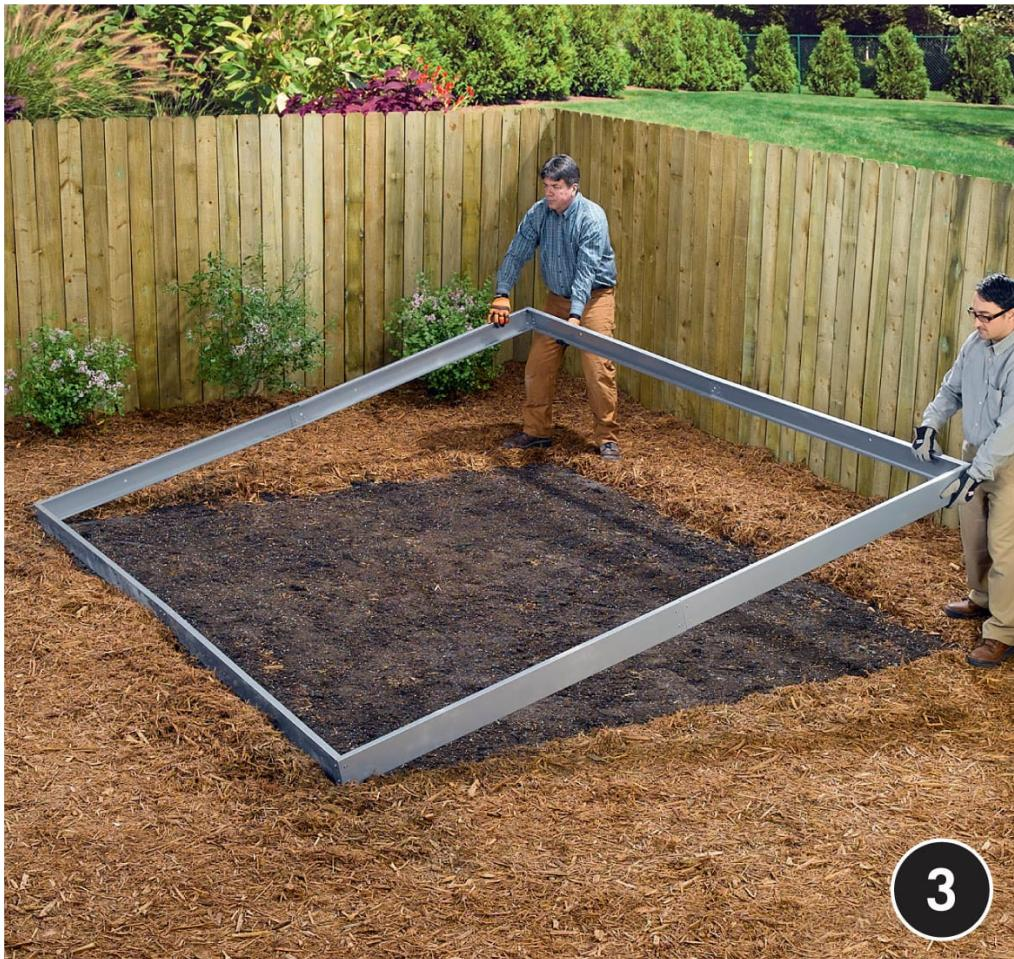
**Assemble the greenhouse base,** using the provided corner and end connectors. Set the base onto the subbase and make sure the base is level. Measure the diagonals to check for square, as before. Add a top dressing of gravel or other fill material inside the base, up to about 1" below the base's top lip. Smooth and level the gravel as before.
