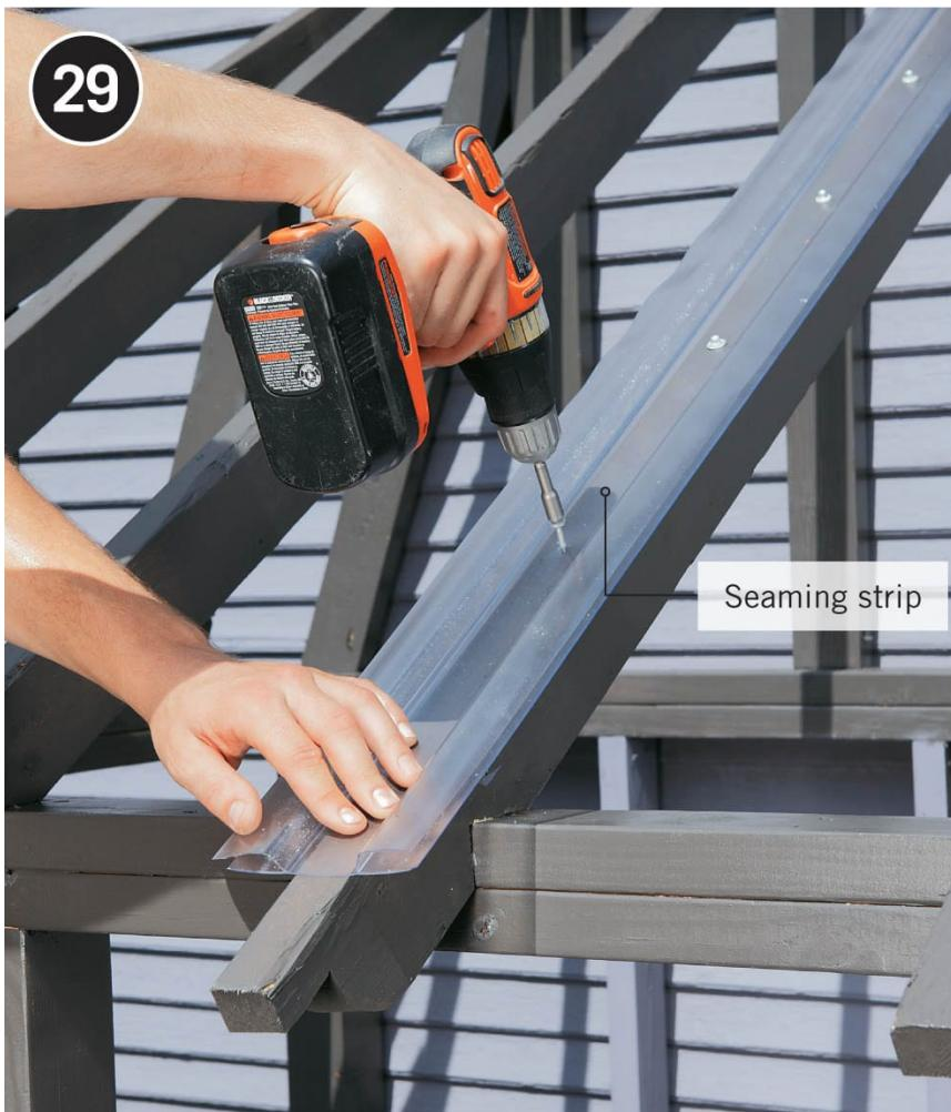
**Begin to fasten the roof panels.** The twin-wall corrugated polycarbonate panels seen here are fastened directly to the rafters. A panel seaming strip with channels on each edge is fastened to the center rafter to create a transition between the two abutting panels. Install the strip first so you can take more accurate width measurements for cutting the panels.
