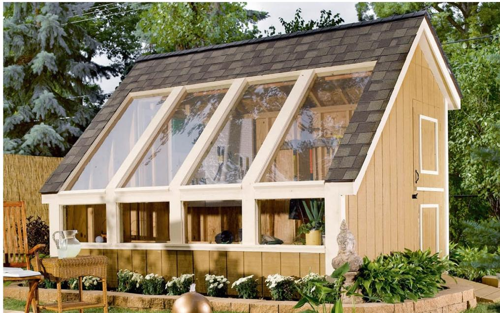
**With slight modifications**, many ordinary sheds can be redesigned as greenhouses. The addition of glass roof panels turns this shed design into an effective greenhouse.
