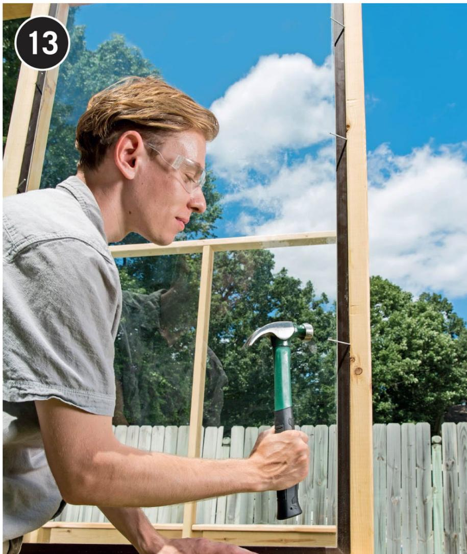
**Pin the window in place** with small brads to allow the silicone to set. Repeat the installation process with the rest of the windows for the three walls.
