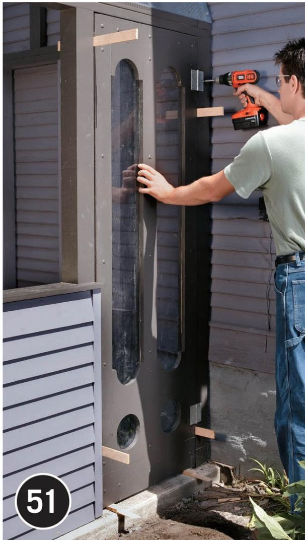
**Hang the door.** Door stop moldings should be installed so the door is flush with the outside greenhouse wall when closed. Add a latch and a handle. If you want to be able to lock the greenhouse, add a hasp and padlock.
