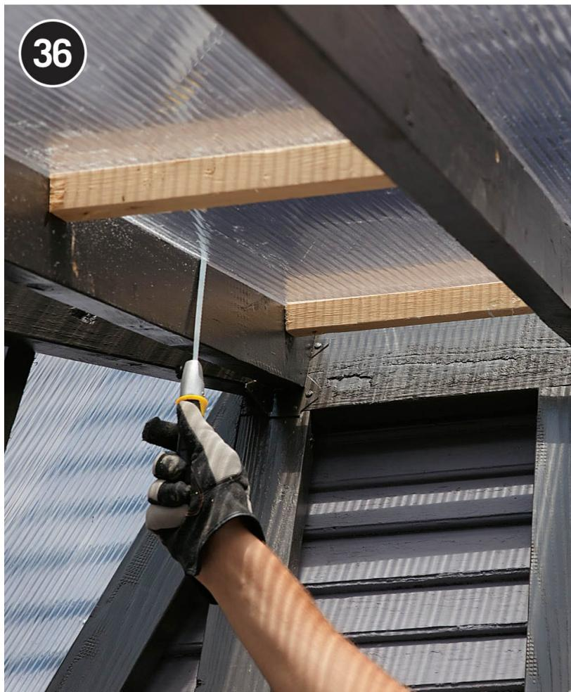
**Cut out the openings in the roof panels.** Drill a starter hole at each corner and then use a drywall saw to make the cuts. Clean up the cut edges with sandpaper.
