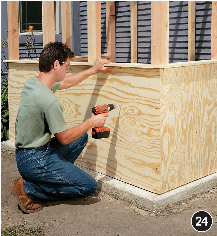
**Cut kneewall sheathing panels** from exterior plywood and attach the panels to the kneewall studs with deck screws.
