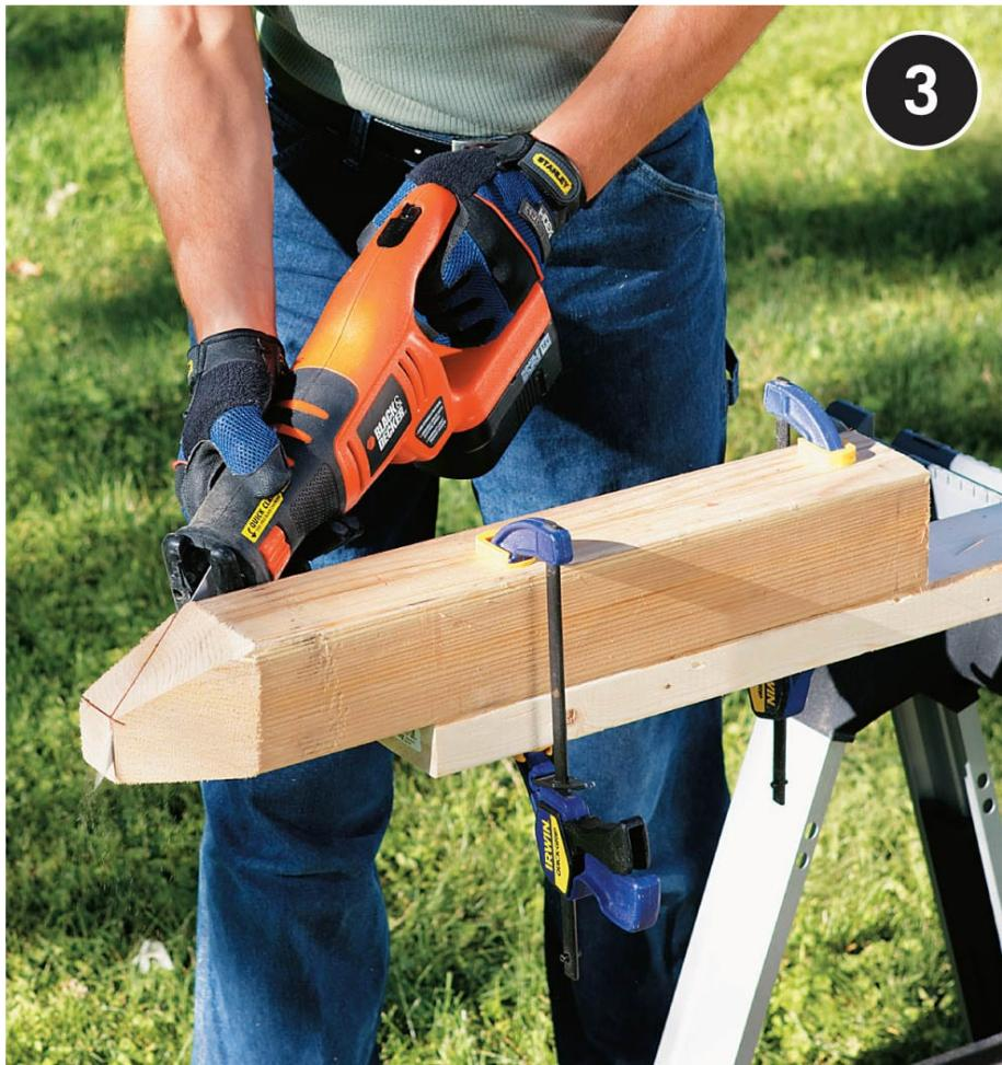
**Create the corner posts** by cutting the 8' 4 × 4 into four pieces roughly 24" each. Trim the ends of each post to a point, using a reciprocating saw or handsaw.
