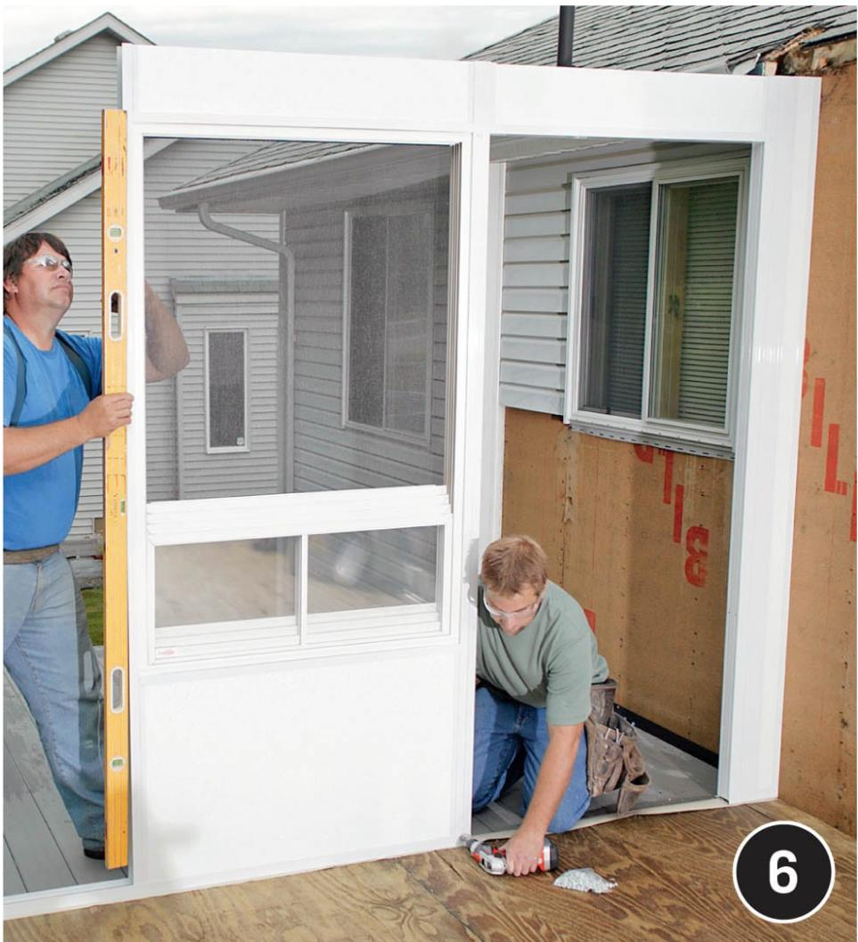
**Add the next panel** according to the installation sequence diagram that comes with your kit. Make sure the panel is plumb and then tack it into position by driving self-tapping screws through the floor flange. The panels lock together at the edges, which will hold them temporarily until the upper wall track can be installed. If you are working in windy conditions, you may need to brace the panels.
