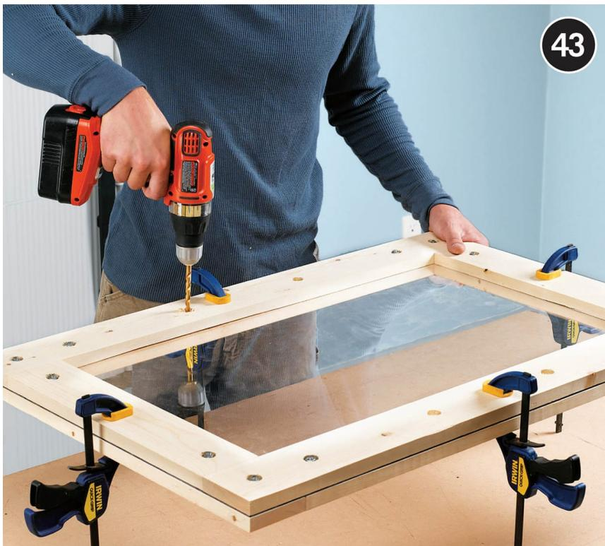
**Drill guide holes** for the bolts that draw the window parts together. Use a bit that's slightly larger than the diameter of the bolt shafts. This allows for slight expansion and contraction of the window parts as the temperature and humidity level change. Counterbore the bolt holes slightly.
