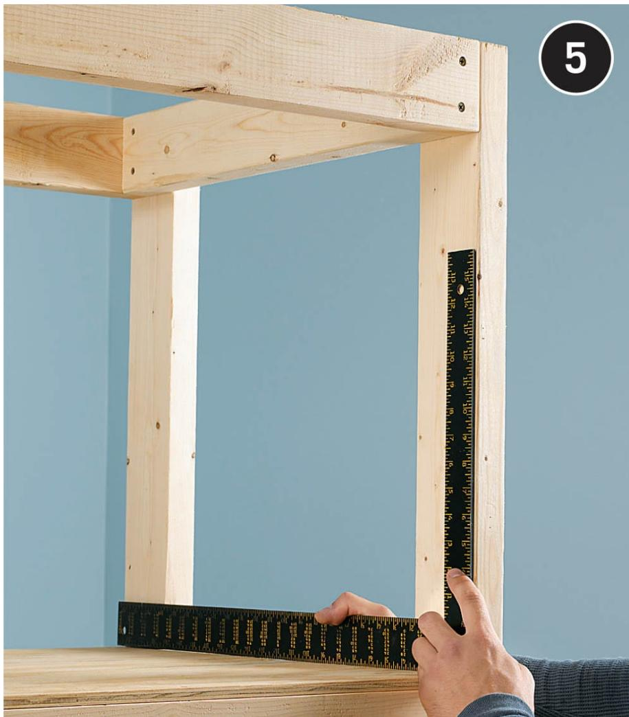
**Fasten the shelves to each leg** with two 2½" deck screws driven through the shelf ends and into the legs. The top edges of each shelf should be on its layout marks (or flush with the ends of the legs), and the front and rear sides should be flush with the outside edges of the legs. Use a square to make sure the shelf and legs are perpendicular before fastening.
