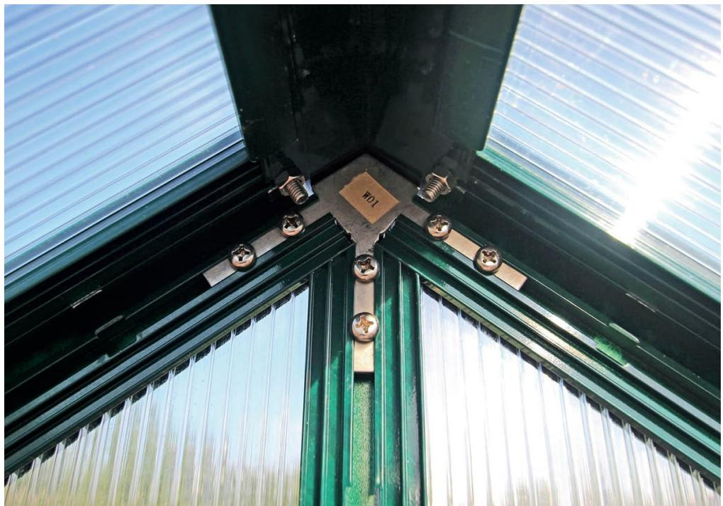
**Determine quality by looking at the fine details.** Inspect any prefab greenhouse for signs of quality construction. This quick-fit fastener makes assembly easier and less stressful, and it will ensure the long-term stability of the greenhouse.
