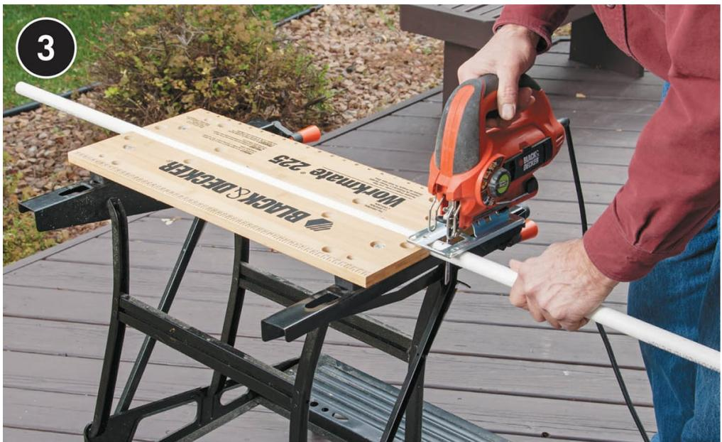
**Assemble the canopy glazing framework** using ½" PVC pipe. Cut all the ribs 37" long. You can cut these easily with a miter saw, hacksaw, or jigsaw.
