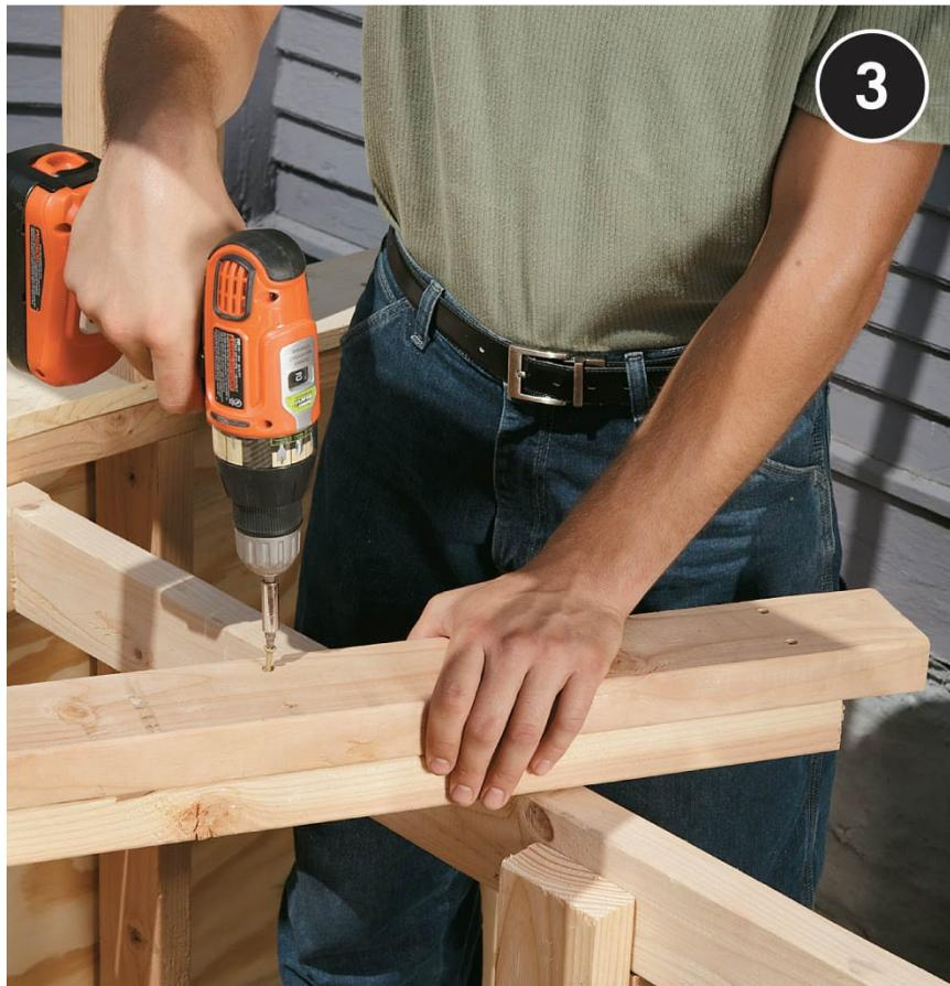
**Install the front legs.** Each leg is created with a pair of  $2 \times 4$ s face-nailed or screwed together. The front  $2 \times 4$  in each pair should fit between the frame and the floor. The back  $2 \times 4$  in each pair is  $2\frac{1}{2}$ " longer to provide a surface for attaching the frame and legs. Join the leg halves with glue and  $2\frac{1}{2}$ " deck screws.
