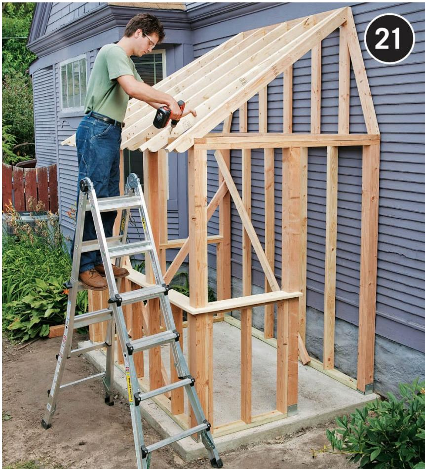
**Fill in the remaining rafters.** If you wish, you can use joist hanger hardware to attach the rafters to the ridge pole. Or, you can nail or screw them. Spacing between rafters should be uniform.
