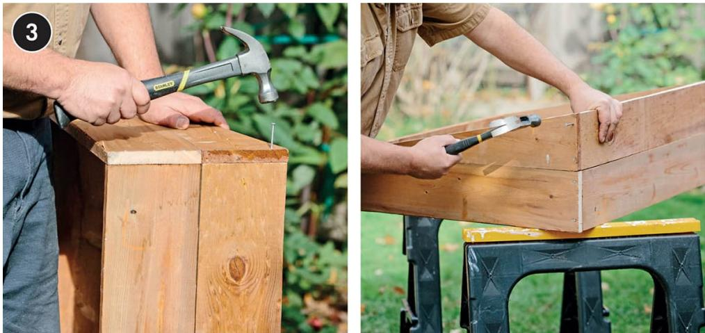
**Use a table saw adjusted to the correct angle, or a jigsaw set to the miter, to bevel-cut the top edges of the front and back frame boards. Drill pilot holes in the edges of the framing pieces, two for each board, at each joint. Tack the frame together with 6d common nails. Check to make sure that the window you've reclaimed fits the frame perfectly and make any adjustments if it does not.**
