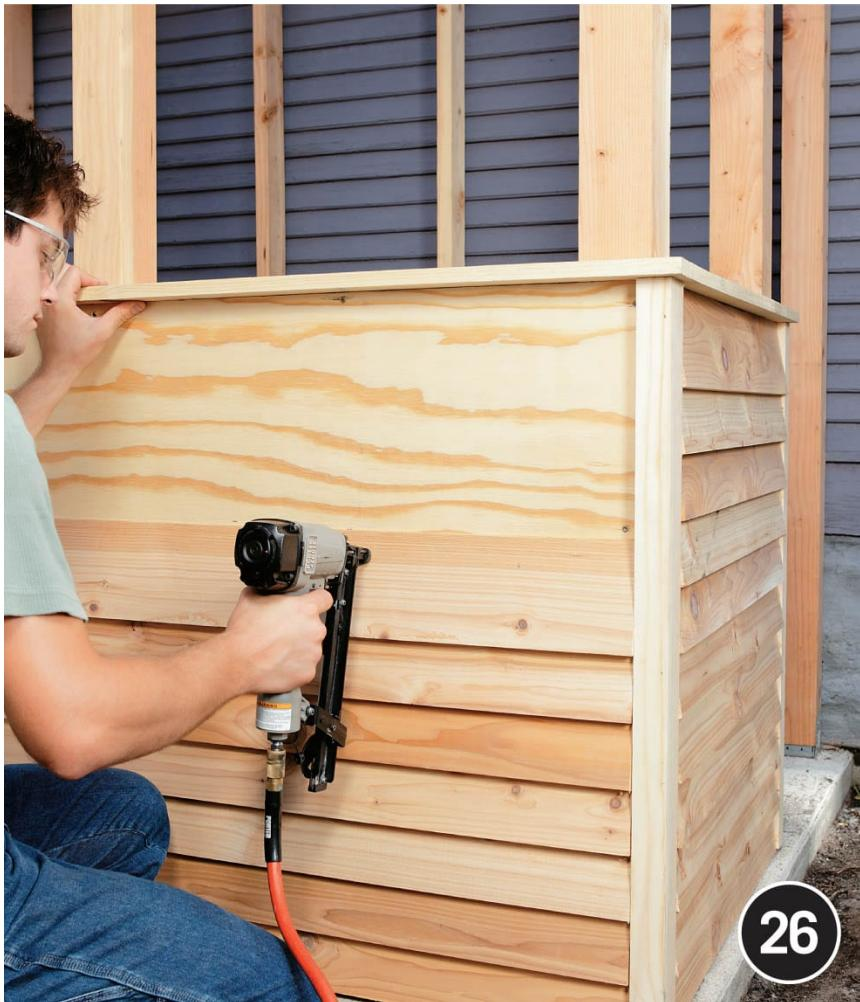
**Install the siding on the kneewall.** Generally, it is a good idea to install siding that matches the house siding. However, a well-chosen contrasting material also can have a pleasing design impact.
