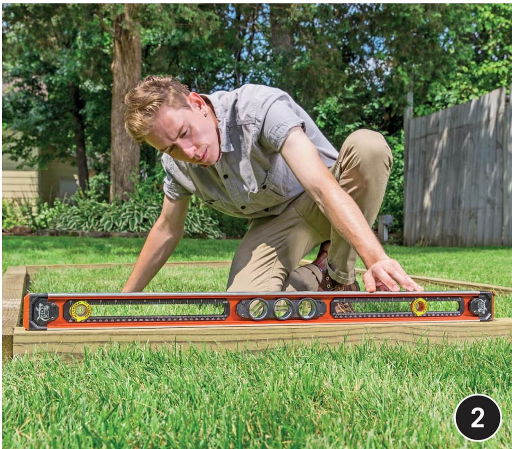
**Fasten the 4 × 4 frame together** by joining the timbers at the corner with 12" spikes, countersunk. Check the frame for level on all sides, side by side, and diagonally. Add or remove gravel under the foundation to level any one side.
