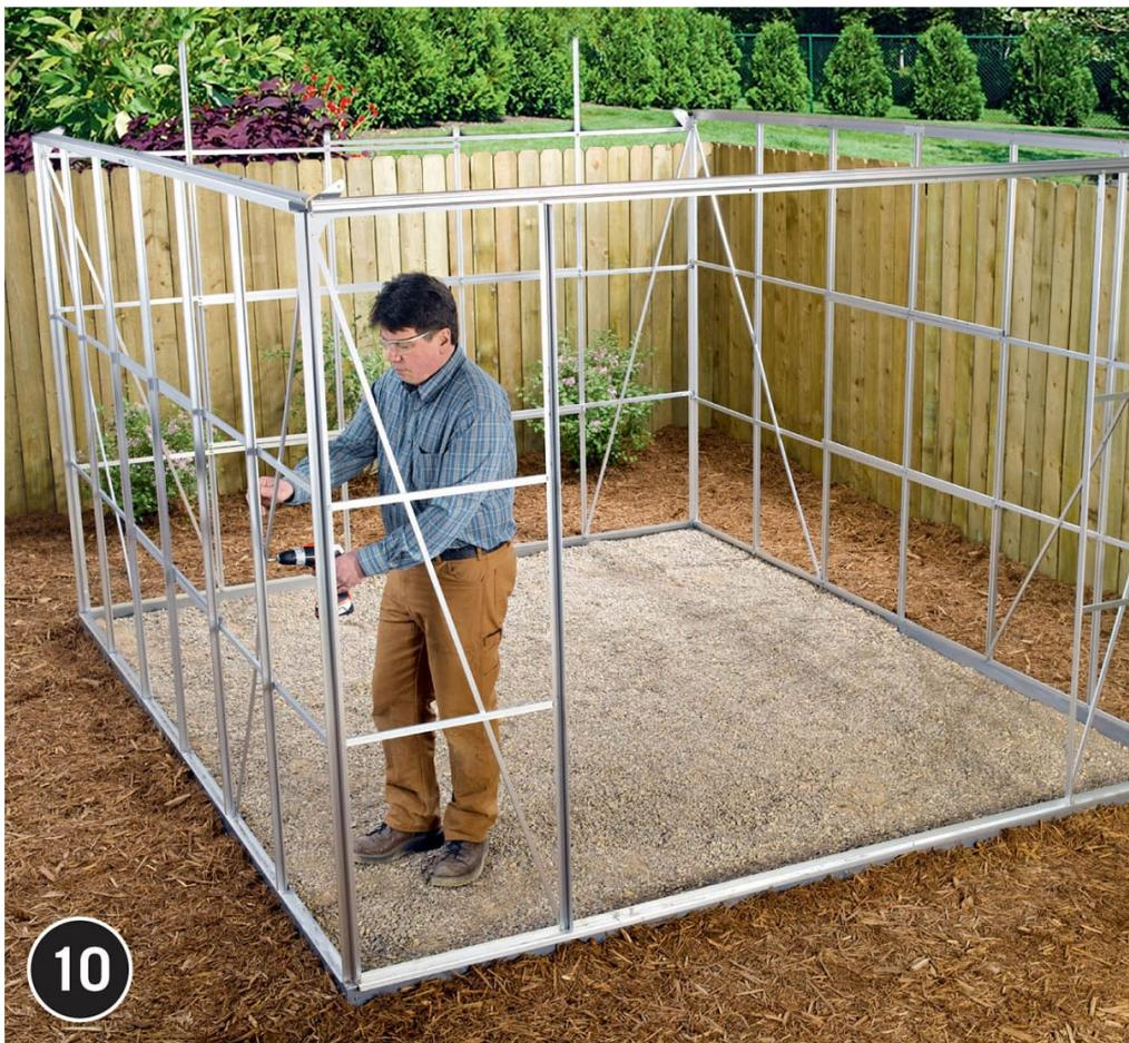
**Add diagonal struts**, as directed by the manufacturer. The struts help to stiffen and square up the walls. As you work, take diagonal measurements between opposing corners at the tops of the walls, to make sure the structure remains square.
