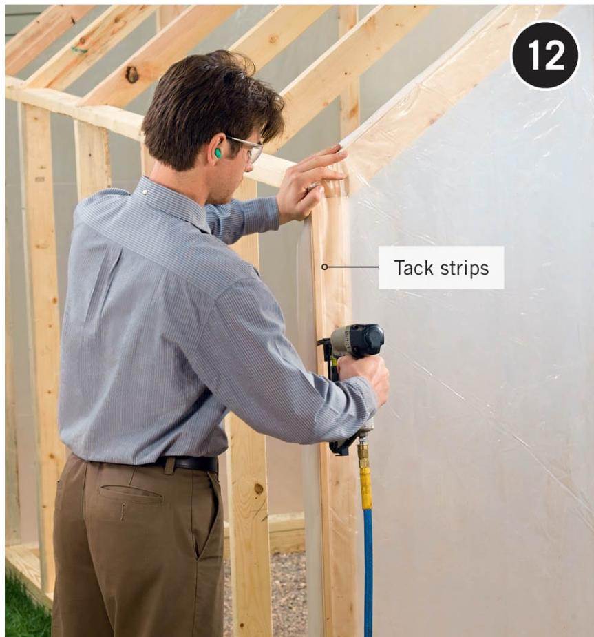
**Begin covering the greenhouse** with the desired cover material (6-mil poly sheeting shown here), starting at the endwalls. Cut the sheeting roughly to size and secure it to the framing with wood tack strips fastened with wire brads. Secure the sheeting at the top first, the sides next, and the bottom last. Trim the excess material along the edges of the strips with a utility knife.
