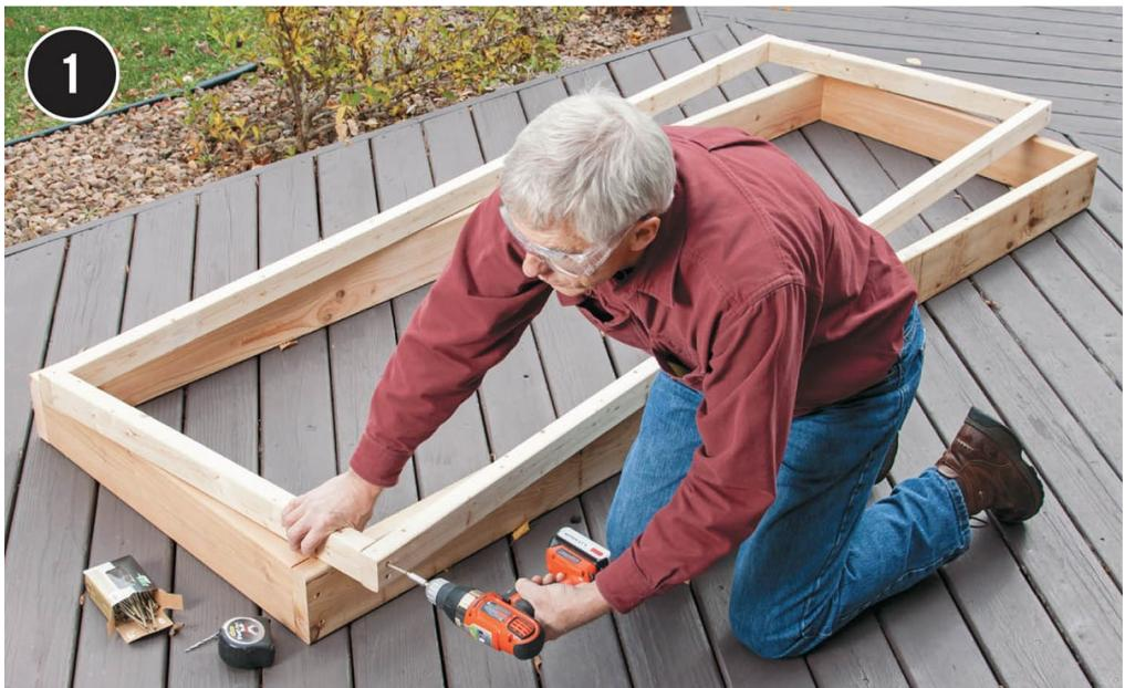
**Drill pilot holes** and fasten the frame end pieces between the frame side pieces with 3" deck screws to create the rectangular frame. Do the same with the base pieces to create the base. Use two screws for each joint.
