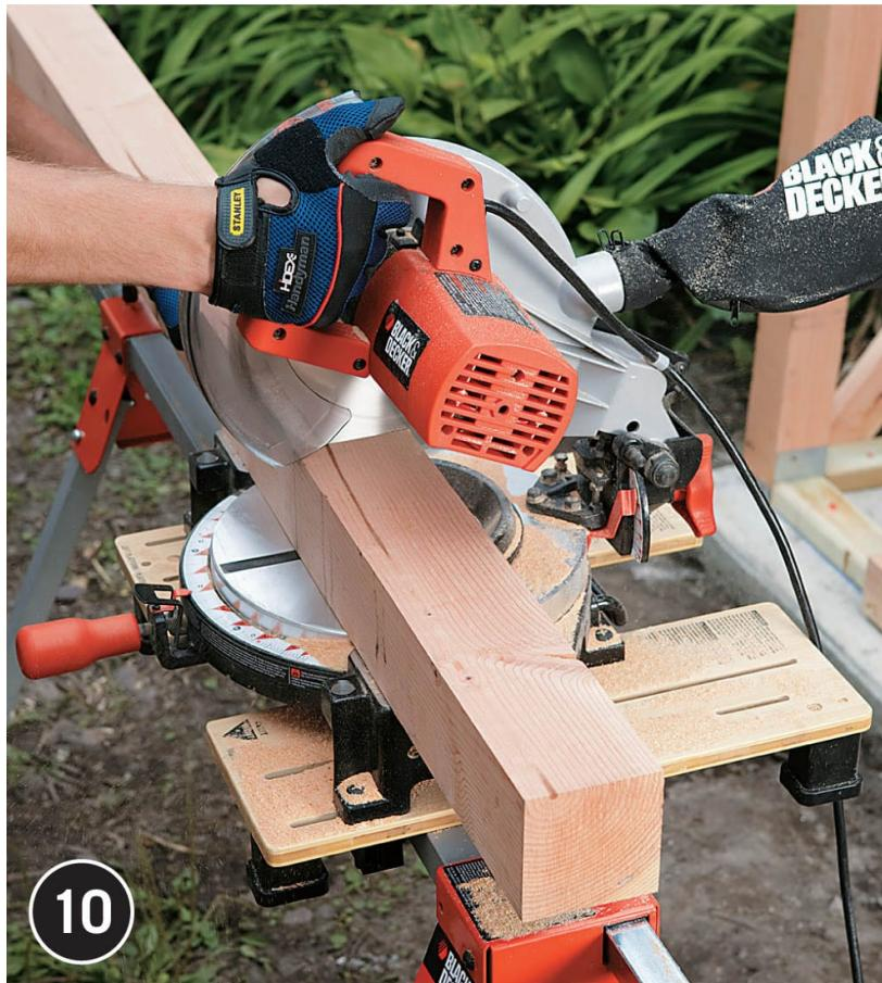
**Remove the posts** for trimming to final height, making sure to note which post belongs in which base. Marking and cutting in this manner ensures that the tops of all posts will be level even though the slab slopes away from the house. Precutting posts to the same length will result in a roof structure that is not flat. Reinstall the posts in the anchors and fasten with joist hanger nails or 16d galvanized nails.
