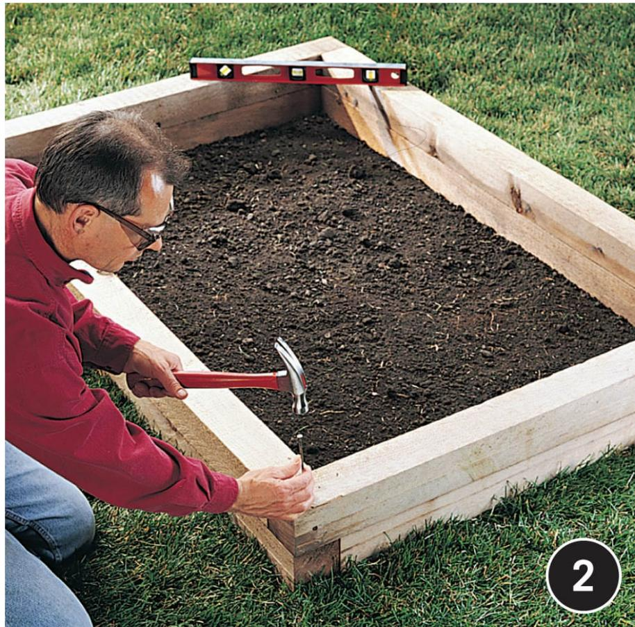
**Set the first course of timbers in the trench.** Check the timbers for level along their lengths and at the corners, adding or removing soil to adjust, as needed. Position the second course on top of the first, staggering the corner joints with those in the first course. Fasten the courses together at each corner with pairs of 6" nails driven through  $3/16$ " pilot holes.
