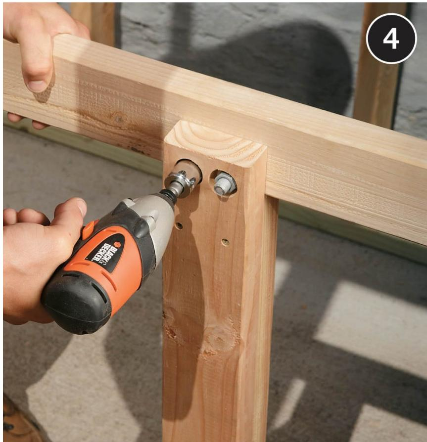
**Attach each leg to the frame** with a pair of  $\frac{1}{2} \times 3\frac{1}{2}$ " carriage bolts. Drill guide holes for the bolt and counterbores for the nuts and washers in the back face of the frame. Do not use washers behind carriage bolt heads.
