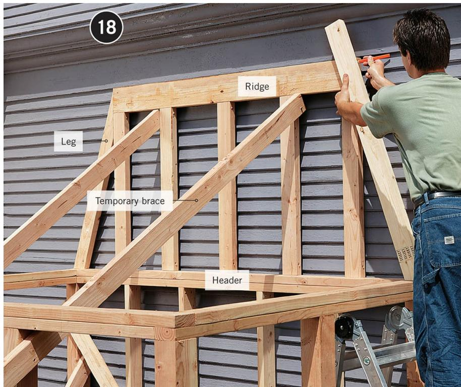
**Position a 2 x 4** so it spans from the ridge pole and past the header. Transfer cutting lines onto the workpiece and then cut the outer support legs to length at the marked angle. Attach the legs with deck screws.
