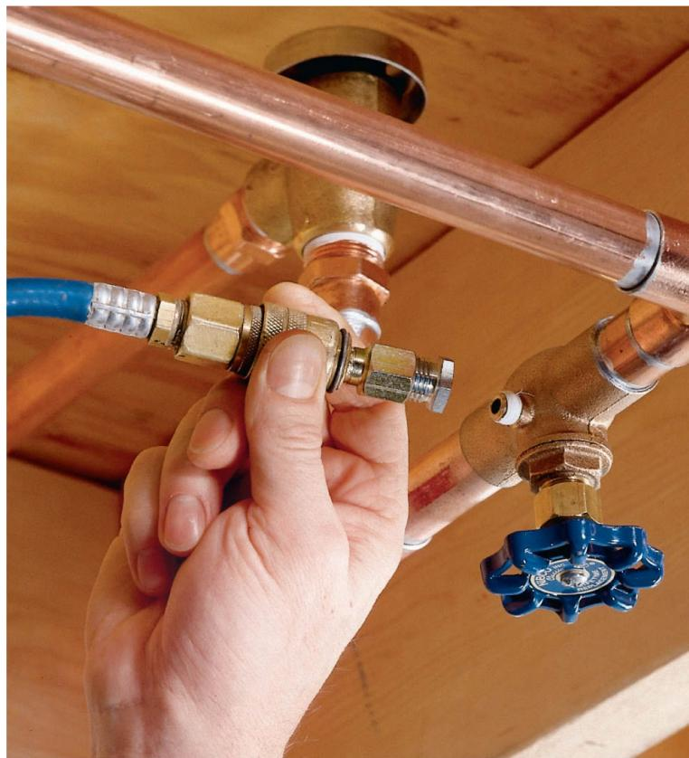
**Winterize a seasonal supply line** using a shutoff valve with an air nipple. With the valve closed and the greenhouse spigot open, blow compressed air (50 psi max.) into the line to remove any water in the tubing. Then, remove the plug from the T-fitting inside the valve box (photo top right) and store it for the winter.
