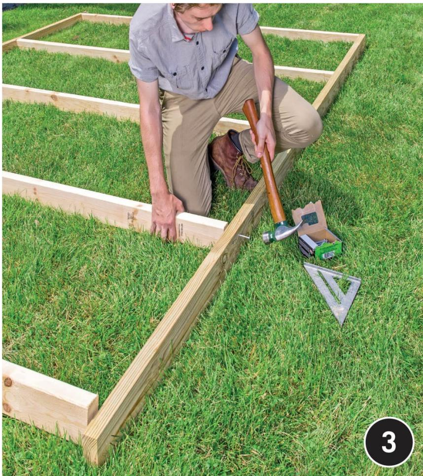
**Working on a clean, flat surface** such as the lawn here, lay out and build one side wall. Nail the sole and top plates to the studs after ensuring that each stud is at a 45° angle to the plate with a speed square.
