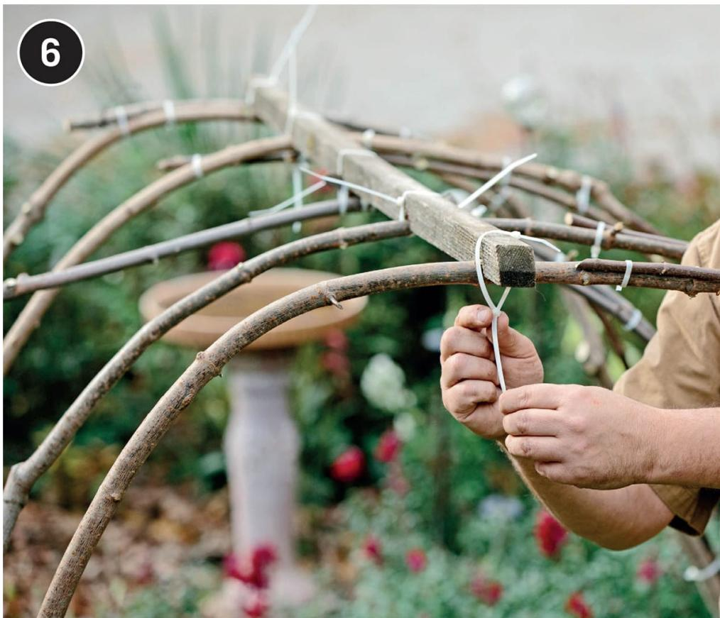
**Lay the ridge pole along the top edge** of the frame base side and mark the positions of the PVC pipe stakes on the branch. Cut slight notches at the marks with a jigsaw. Lay the ridge branch across the hoops so they fit into the notches and zip tie the hoops to the ridge pole.
