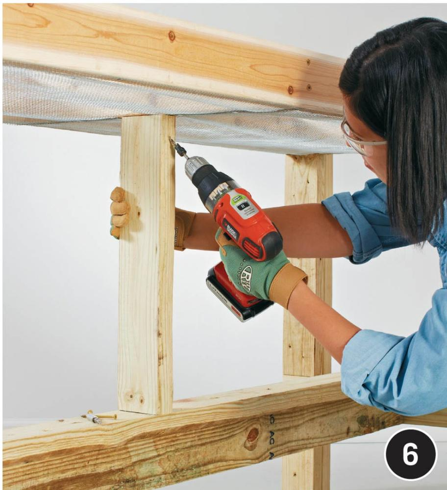
**Place the tray on the ground**, right-side up. Screw the top stretcher to the rails and lower stretcher. Measure the distance from the stretchers to the center divider and cut and fasten the support. Add  $1/16$ " to your measurement just to make sure you have a snug fit.
