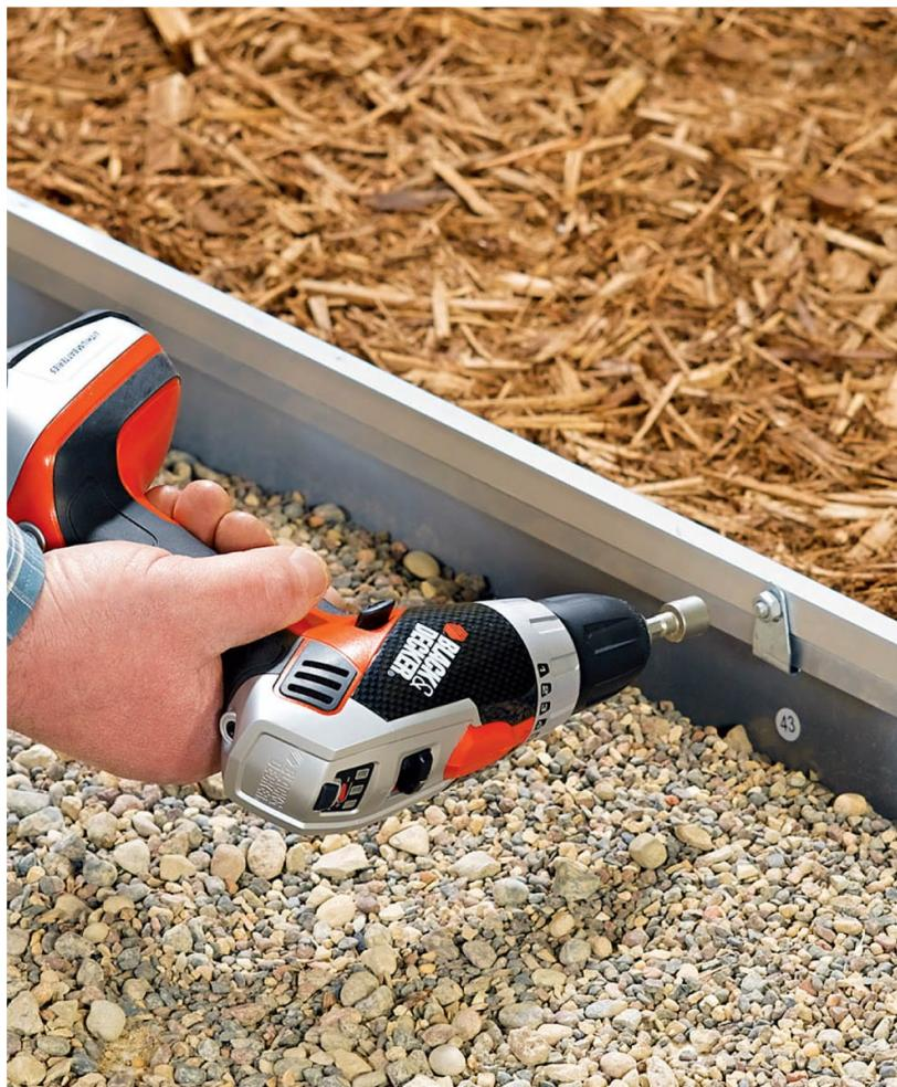
**A cordless drill/driver** with a nut-driver accessory will trim hours off of your assembly time compared with using only hand tools.
