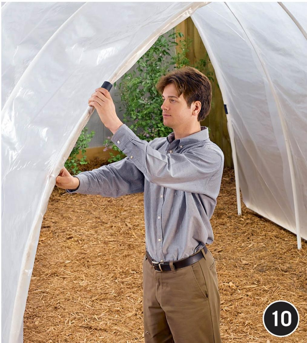
**Secure the cover at the ends** with 6" lengths of 1" PE tubing. Cut the tubing pieces to length, then slit them lengthwise to create simple clips. Use at least six clips at each end of the house. Do not use clips on the intermediate hoops.
