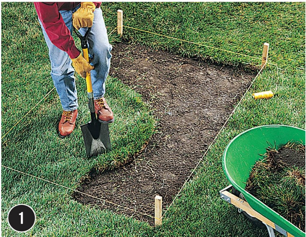
**Outline a 3 × 5' area** with stakes and mason's string. Remove all grass inside the area, then dig a 2"-deep × 6"-wide trench along the inside perimeter of the outline. Cut each of the four timbers into one 54" piece and one 30" piece, using a reciprocating saw or circular saw.
