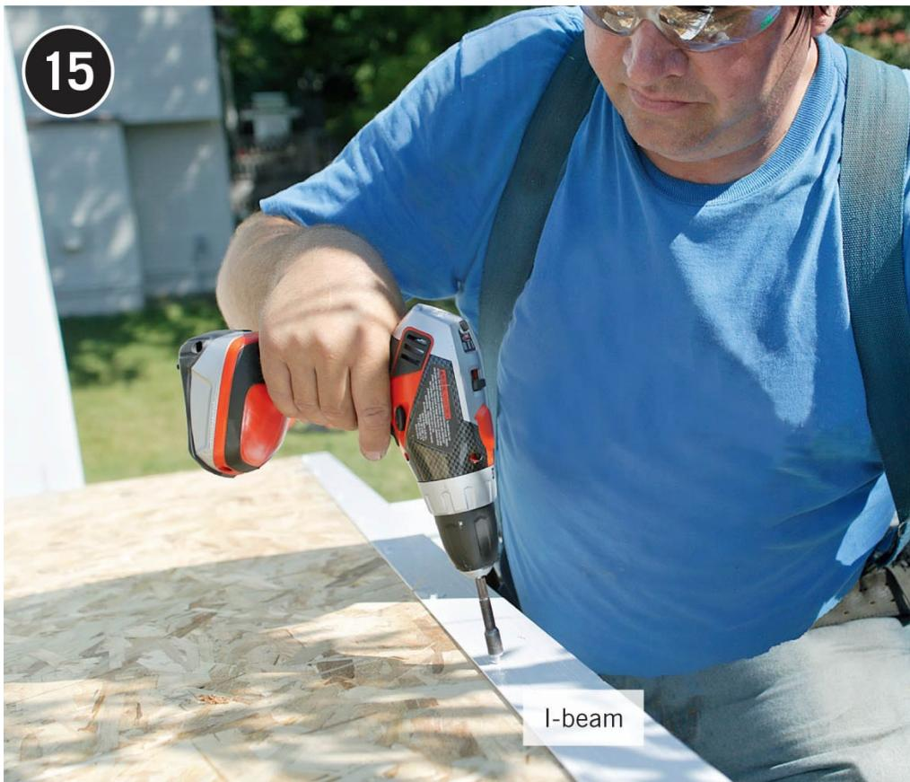
**Install I-beams** on the roof next to the first roof panel. The track on one side of the I-beam should capture the leading edge of the first roof panel. Attach the I-beam to the roof panel with self-tapping screws driven through the I-beam flange and down into the OSB panel surface.
