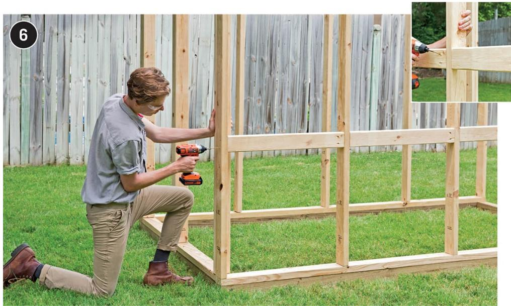
**Screw  $2 \times 4 \times 28\frac{1}{4}$ " spreaders** in the stud cavities of the side and back walls. Toe-screw the spreaders on the inside edges and face-screw through the corners (inset). The tops of spreaders should be 32" above the  $4 \times 4$  base, faces flush with the outside edges of the wall studs.
