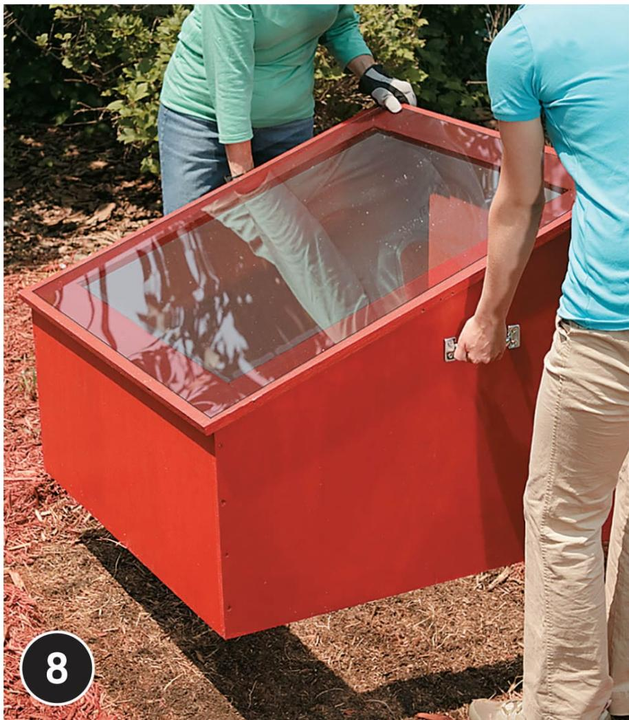
**Move the cold frame to the site.** Clear and level the ground where it will set if possible. Some gardeners like to excavate the site slightly.
