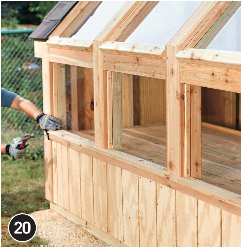
**Complete the trim details** with 1 × 4 vertical corner boards, 1 × 4 horizontal trim above the front wall windows, and ripped 1 × 4 trim and 1 × 2 trim at the bottom of the front wall windows (see the TABLE + LOWER WINDOW DETAIL). Paint the siding and trim, or coat with exterior wood finish.
