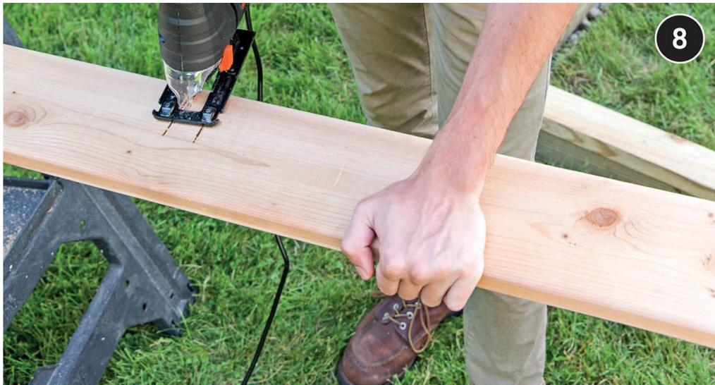
**Use a jigsaw** to cut notches in 5/4 cedar decking to use as window sills on top of the spreaders.
