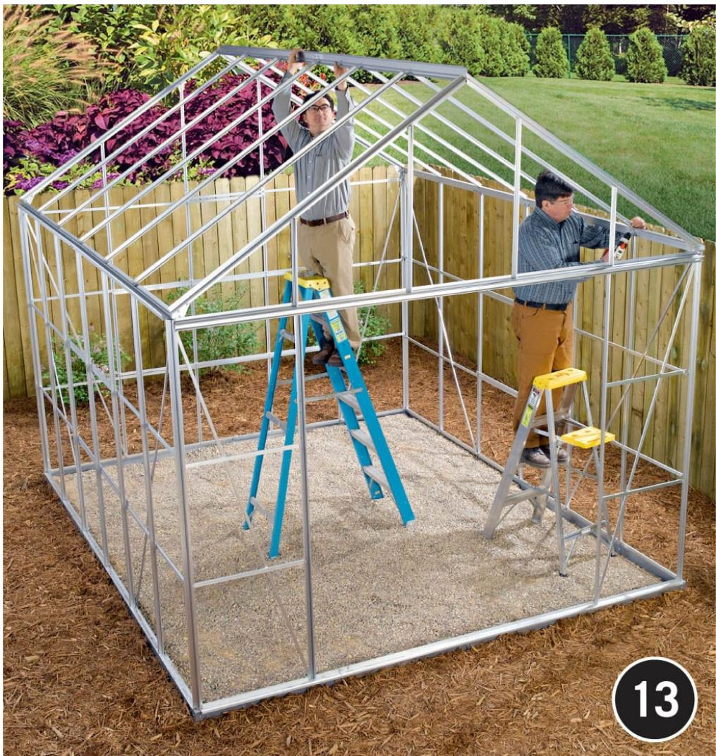
**With at least one helper,** lift the roof into place onto the wall frames. The gable end studs should meet the outside edges of the crown beams, and the ends of the crown beams rest on the outer edge of the corner bracket. Fasten in place with the provided nuts and bolts.
