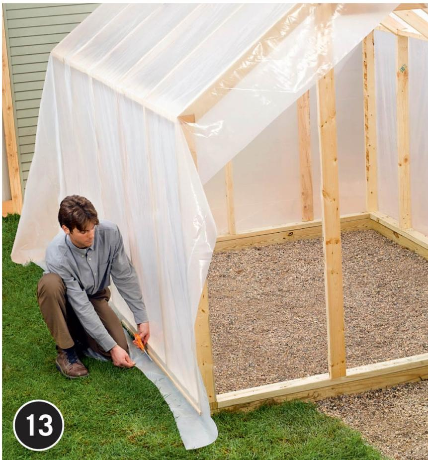
**Attach sheeting to the edges of the sole plate** on one side of the greenhouse, then roll the sheeting over the top and down the other side. Draw it taut, and cut it a little long with scissors. Secure the sheeting to the other sole plate (using tack strips), then attach it to the outside edges of the corner studs.
