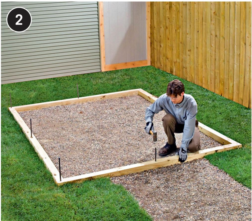
**Cut 12 pieces of #3 rebar** to length at 24" (if necessary), using a reciprocating saw or hacksaw. Drill a  $\frac{3}{8}$ "-diameter pilot hole through each timber, near both ends and in the middle. Confirm that the timber frame is square by measuring diagonally between opposing corners (the measurements must be equal). Drive a rebar spike through each hole, using a hand maul, until the bar is flush with the timber.
