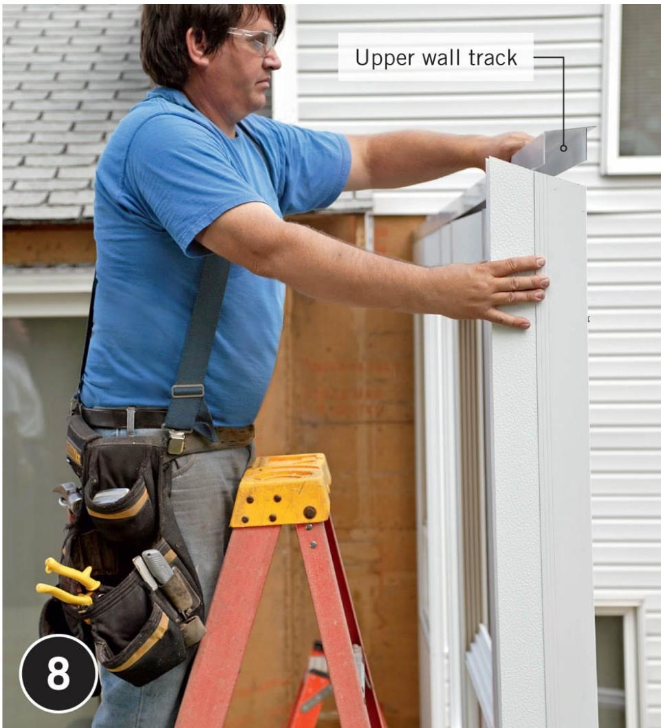
**Fit the upper wall track** over the entire first wall after cutting it to length. The end of the track that joins with the track on the next wall should be mitered to make a neat joint. If the adjoining wall is gabled, this will mean making a relatively tricky compound miter cut. Refer to your plan for the exact angle and don't be shy about asking for help.
