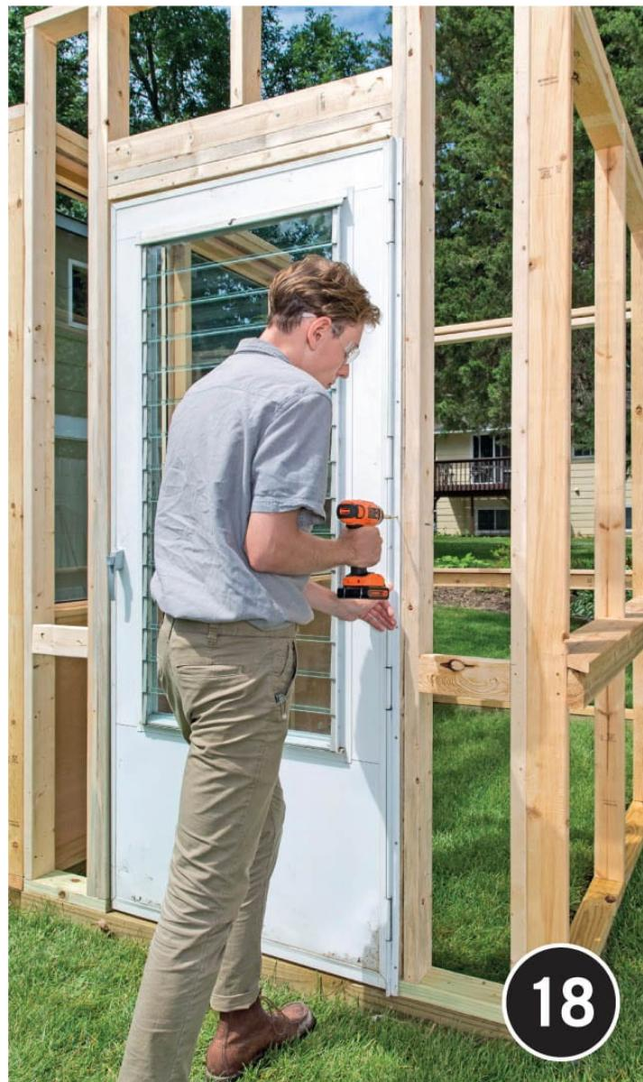
**Frame the front wall** (12" higher than the side walls) in place by measuring and marking stud and doorjamb positions and toe-nailing the members in place. Nail the top cap to the top of the studs and install the door header. Install the door so that it opens outward.
