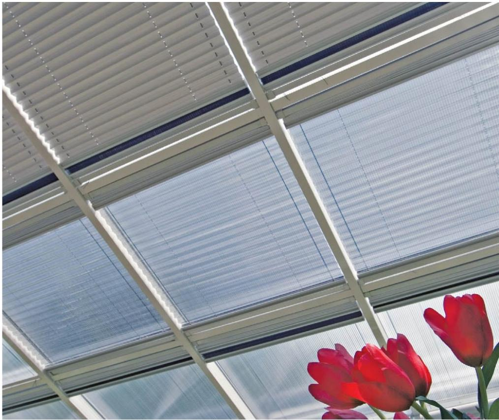
**Skylight shades** give you control over light and heat coming through the roof panels. These 2-in-1 shades have a solid reflective panel that blocks most of the sun's light and heat and a translucent panel that blocks only half of the sunlight to reduce glare and heat gain while letting light filter through.
