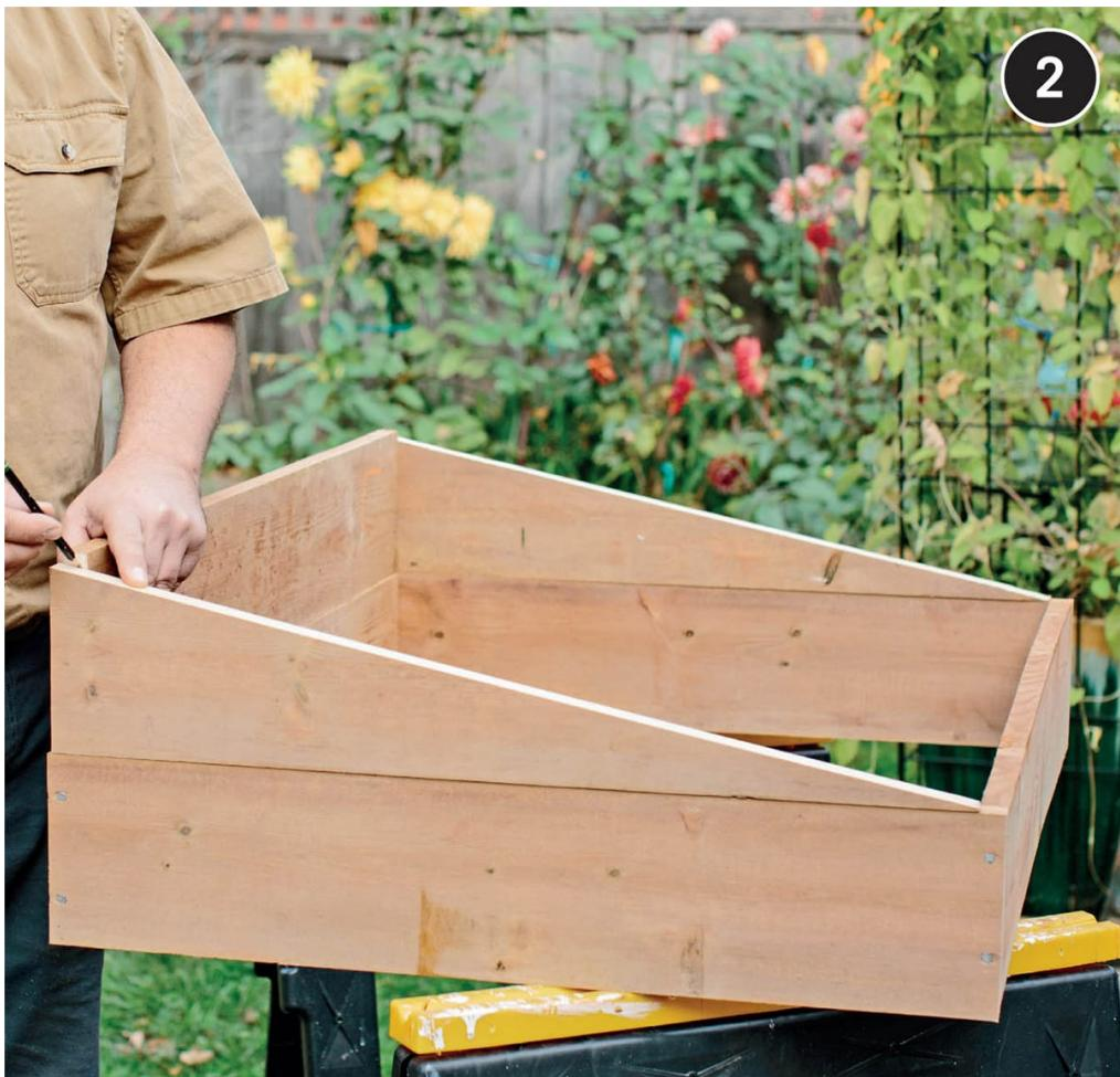
**Cut the board along the marked lines** to make the sloped tops of the side frames. Stand a rear frame board with the face flush to the back edge of the sloped side frame piece. Mark the angled bevel cut on the edge of the rear frame board. Repeat the process with the front frame board.
