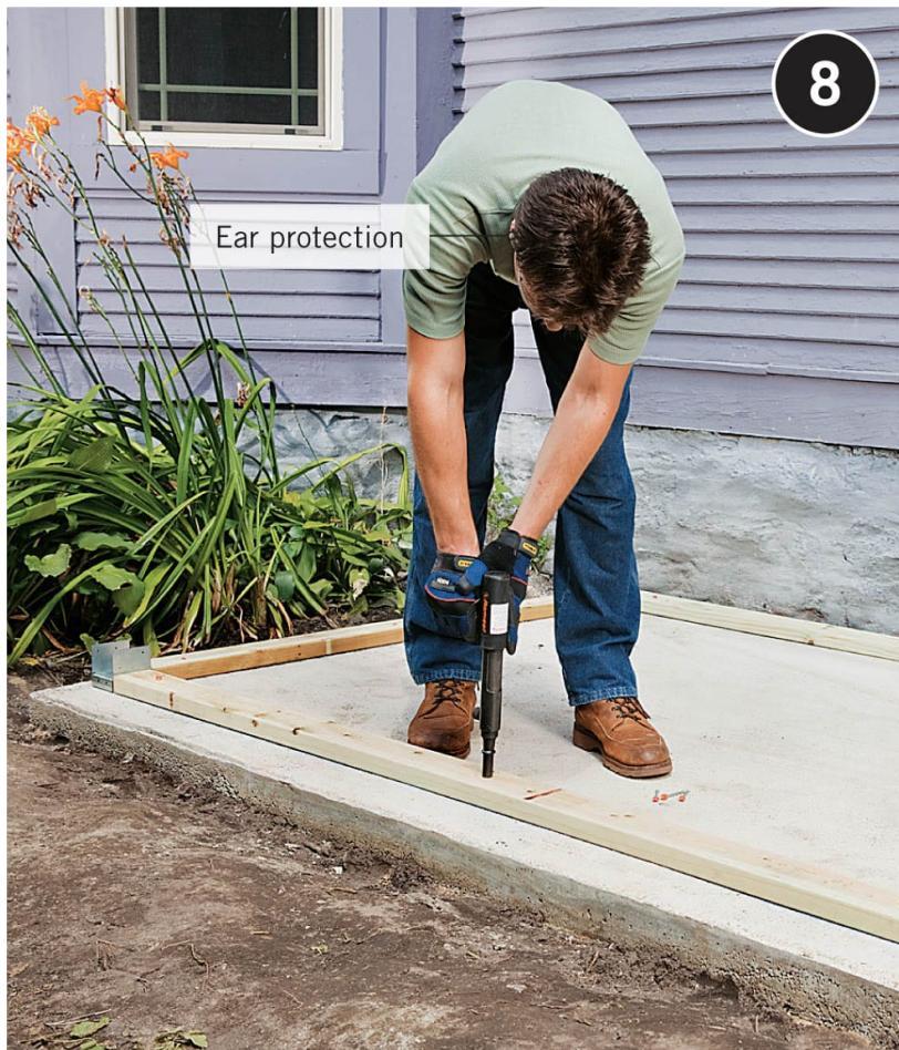
**Cut the 2 × 4 sill plates** to fit between the posts, using pressure-treated lumber. Install the sill plates by fastening with a powder-actuated tool and concrete nails. Or, you can drill guide holes and install masonry anchor sleeves or simply drive concrete screws into the concrete.
