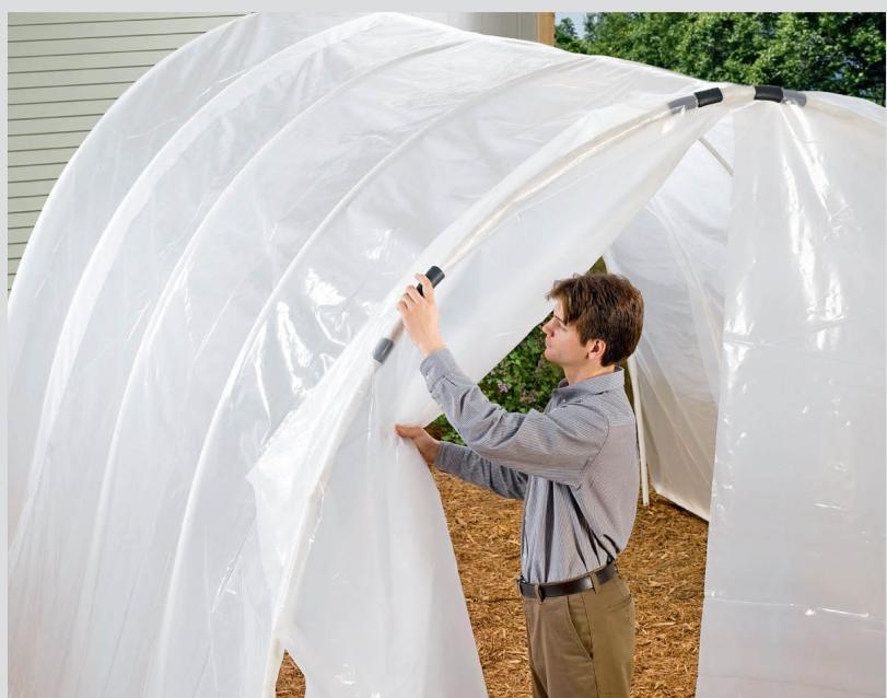
**OPTION:** Make doors by clipping a piece of cover material to each end. (It's best to do this before attaching the main cover.) Then cut a slit down the center of the end material. You can tie or tape the door material to the sides when you want it open and weigh down the pieces with a board or brick to keep the door shut. This solution is low-tech but effective.
