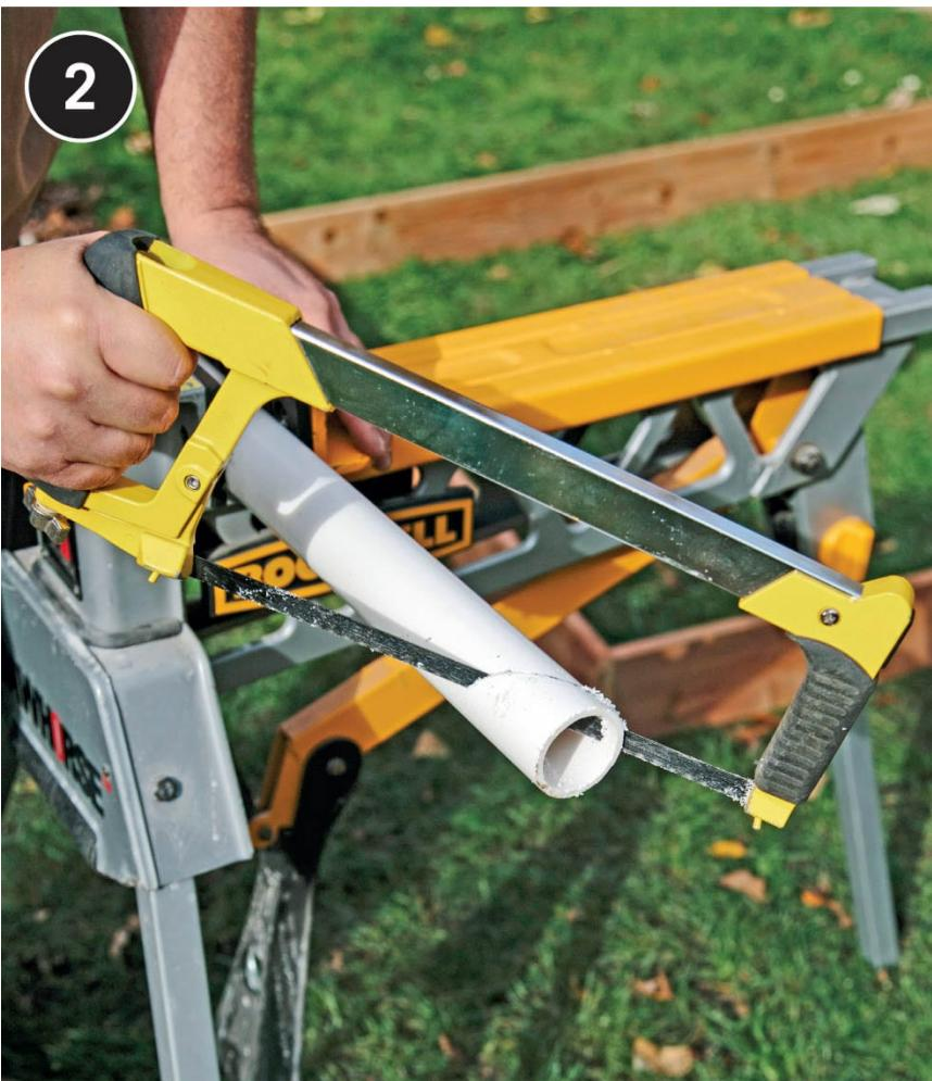
**Use a hacksaw** to cut the PVC pipe scraps to 8" long (they can be longer, but not shorter). Cut one end of each pipe scrap on the diagonal at a severe angle to create a stake point.
