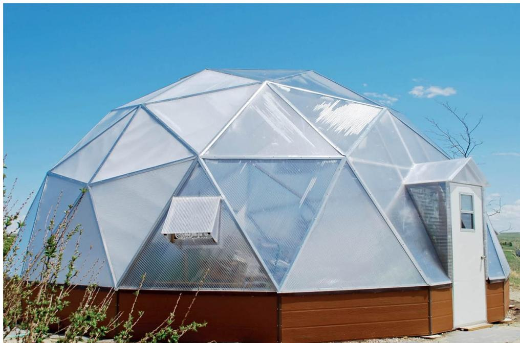
**Do domes in style.** A geodesic dome doesn't need to look simple. This one features a wood knee wall, solid door, and bump-out vent panels. The opaque UV glazing serve the purpose and add to the stylish vibe.
