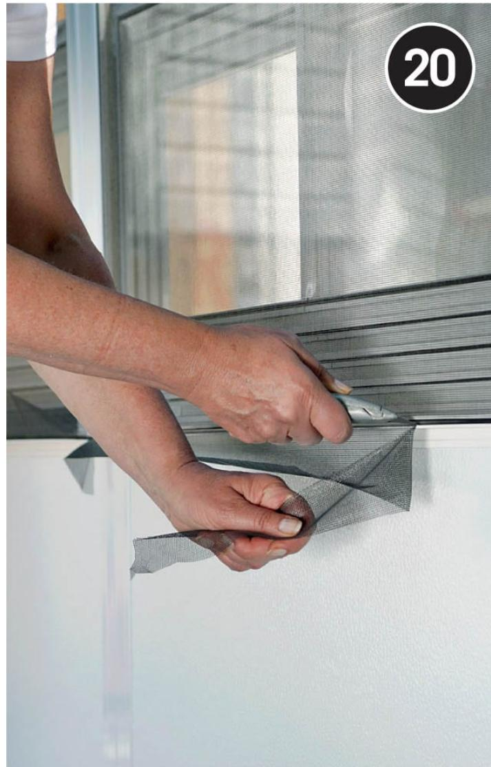
**Make finishing touches**, such as trimming off excess insect screening and painting or cladding the ridge pole. If your sunroom does not have a finished ceiling, add one (tongue-and-groove cedar carsiding is a good choice). Install floorcoverings.
