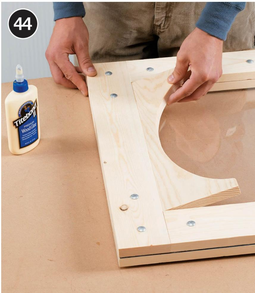
**Cut the arched inserts** to fit at the top of the window frame opening. Install the inserts in the frame with glue and a couple of brads or pin nails. Install an insert on both the interior and the exterior sides of the window. Paint the window frames before installing and touch up after.
