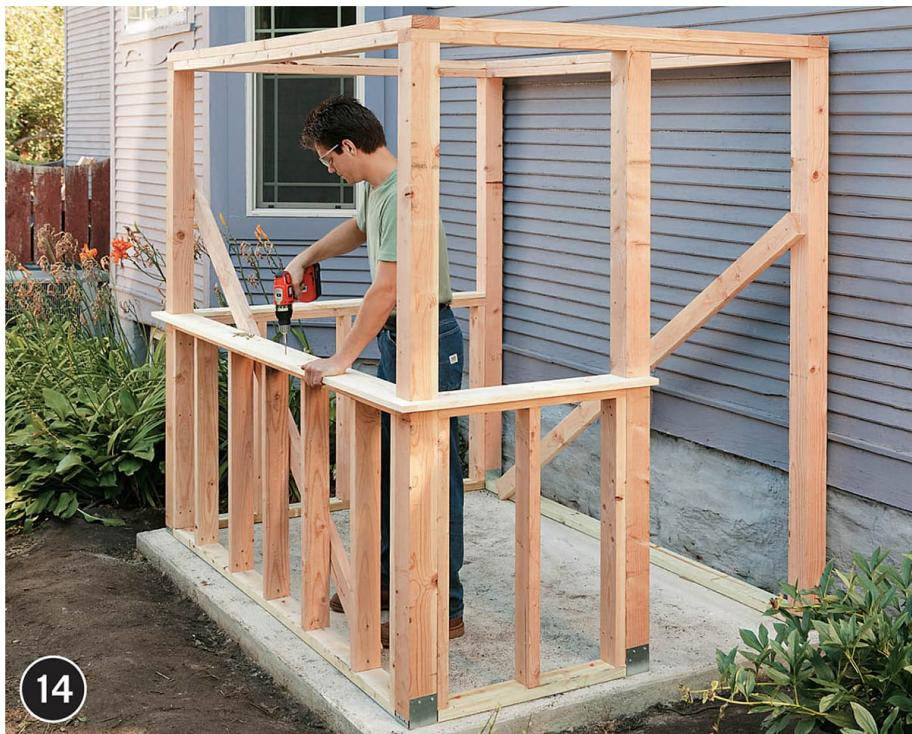
**Add 1 × 6 sills** to the tops of the 2 × 4 kneewalls. The sills will cover the edges of the exterior siding, so make the interior edges flush with interior wall studs and cap plate.
