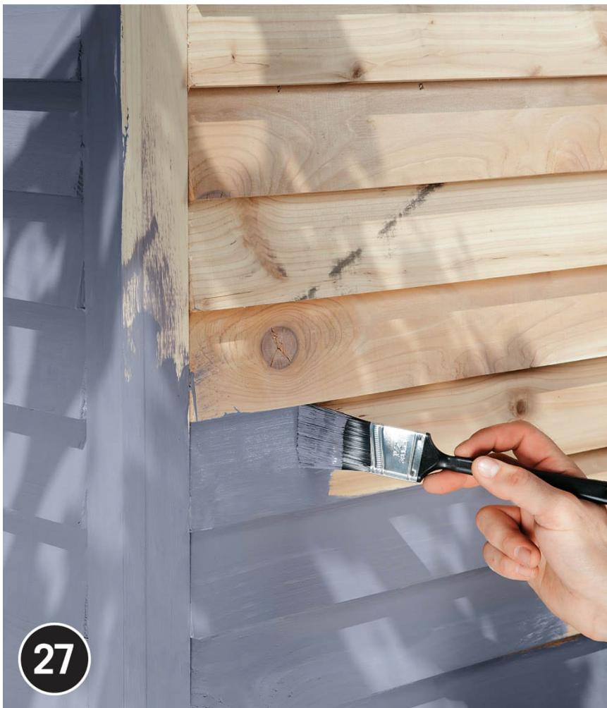
**Paint the structure** prior to adding roof panels and windows with glazing. Two coats of exterior paint is an adequate finish for an exterior lumber product, such as this cedar siding. A base coat of primer is always a good idea.
