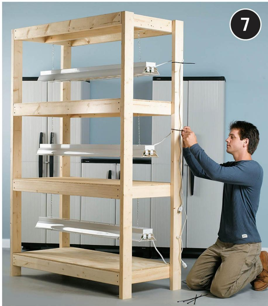
**Route the fixture cords** to the nearest leg of the rack and secure them with zip ties or insulated cable staples. Be sure to leave enough slack in the cord to allow for moving the fixture up and down. If necessary, use an approved extension cord to extend a fixture cord to the power strip location.
