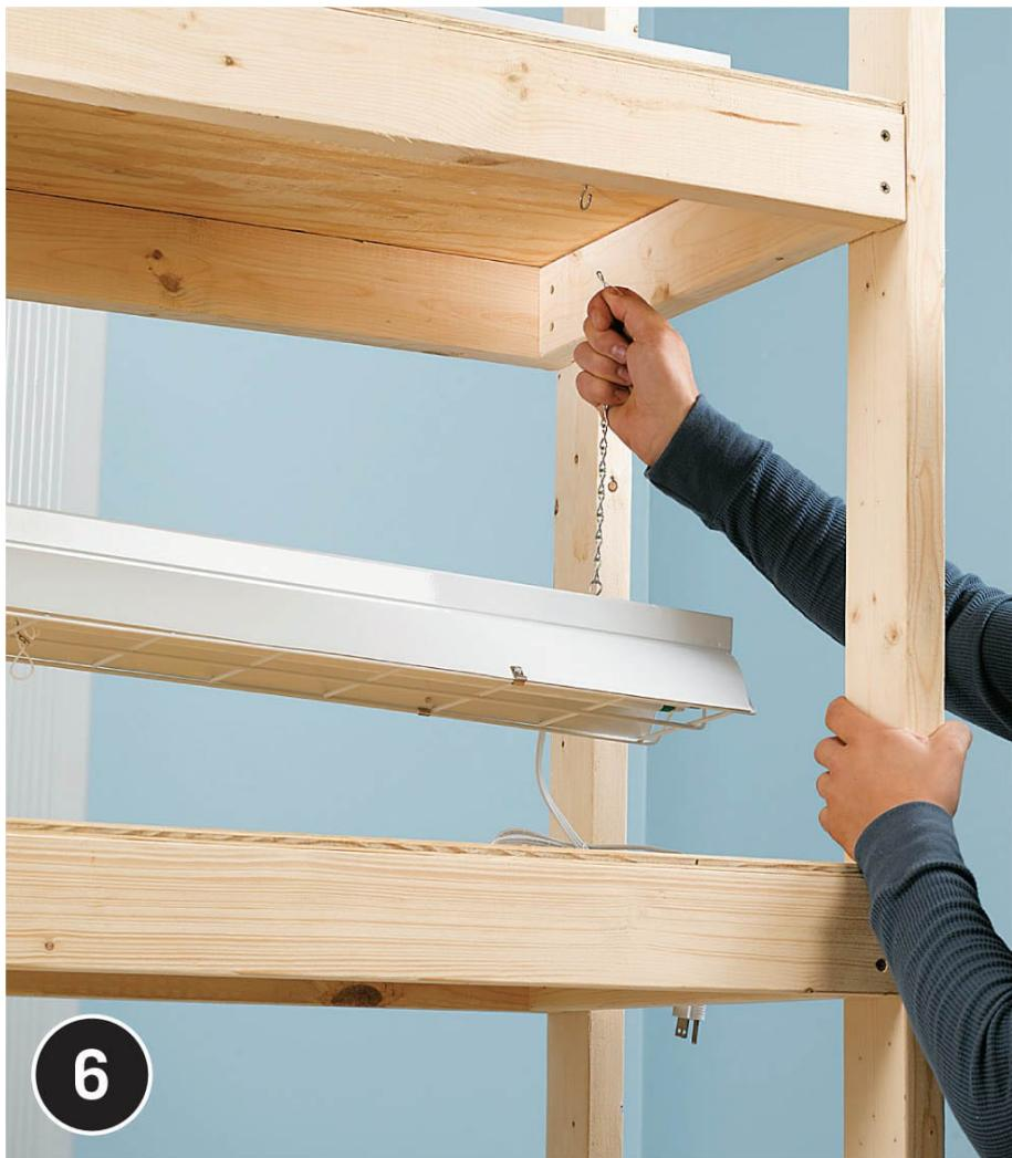
**Hang the light fixtures**, using chain and S-hooks. Cut the chain into 18" lengths, using wire cutters, and attach each to one end of each fixture, using S-hooks or wire, as applicable. Attach the other end of the chains to the plywood shelf above, using S-hooks.
