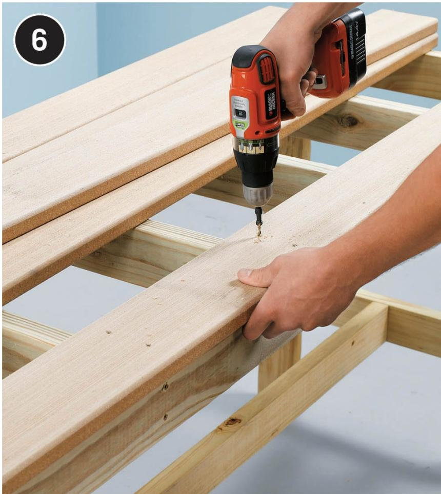
**Cut the top decking boards to length.** Clamp the first board in place so it overhangs the front and ends of the top frame by  $\frac{3}{4}$ ". If the deck boards are crowned (slightly curved across the face), make sure the convex side faces up. Drill two pilot holes at the center of each top frame end and top support location, countersinking the holes slightly. Fasten the board with  $2\frac{1}{2}$ " deck screws.
