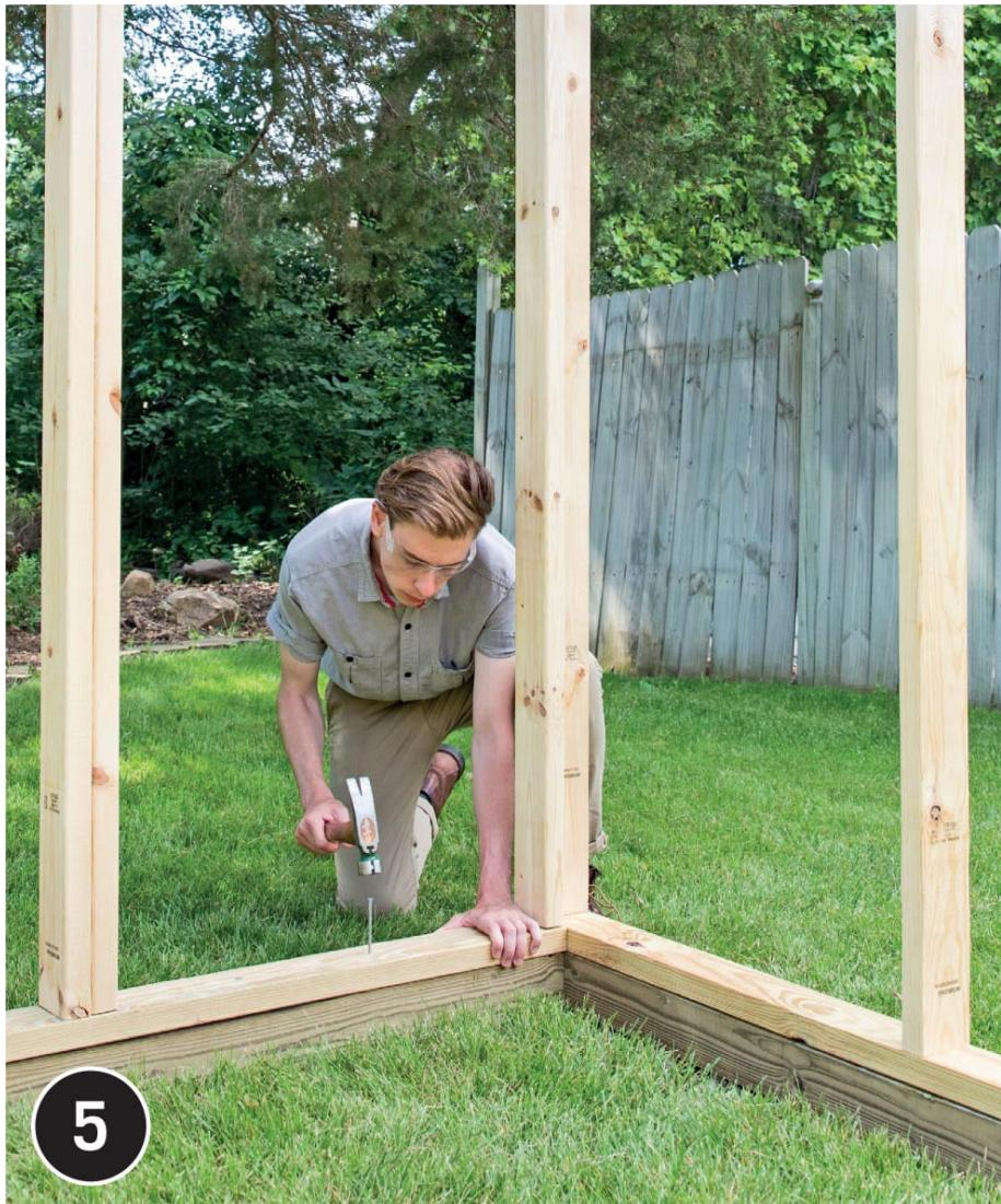
**Once the two side walls** are constructed and nailed in position, build and raise the rear (nondoor) wall into place and nail it to the foundation 4×4. Screw the walls together at the corners with 3" wood screws.
