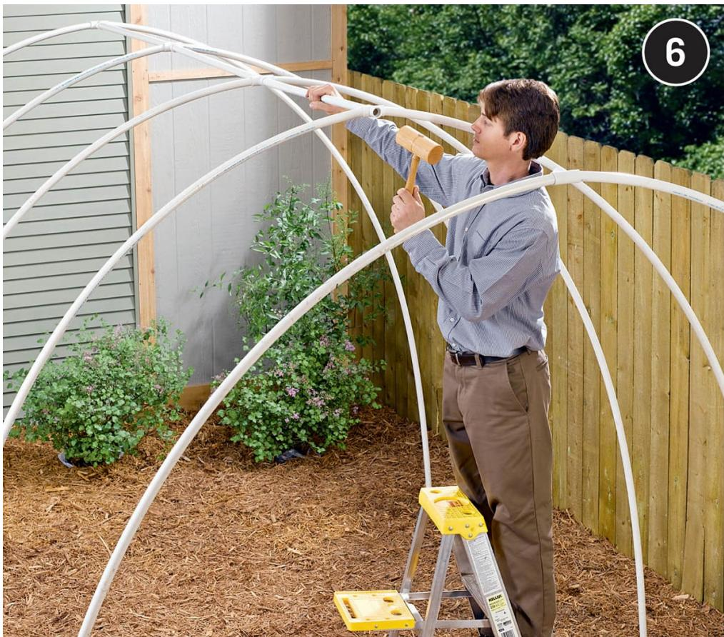
**Add the ridge pole sections** to tie together the hoop frames. The correct length for the ridge poles depends on the socket depth of the fitting you use, so you'll have to measure the fittings and calculate length of the ridge pieces. If necessary, tap the end of each ridge piece with a wood or rubber mallet to seat it fully in the fitting socket.
