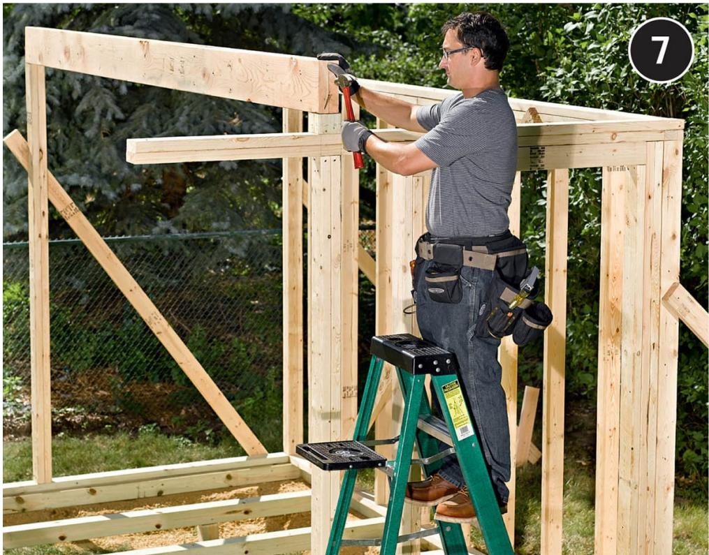
**Construct the rafter header** from two 2 × 8s cut to  $142\frac{3}{4}$ ". Join the pieces with construction adhesive and pairs of 10d common nails driven every 24" on both sides. Set the header on top of the side wall posts, and toenail it to the posts with four 16d common nails at each end.
