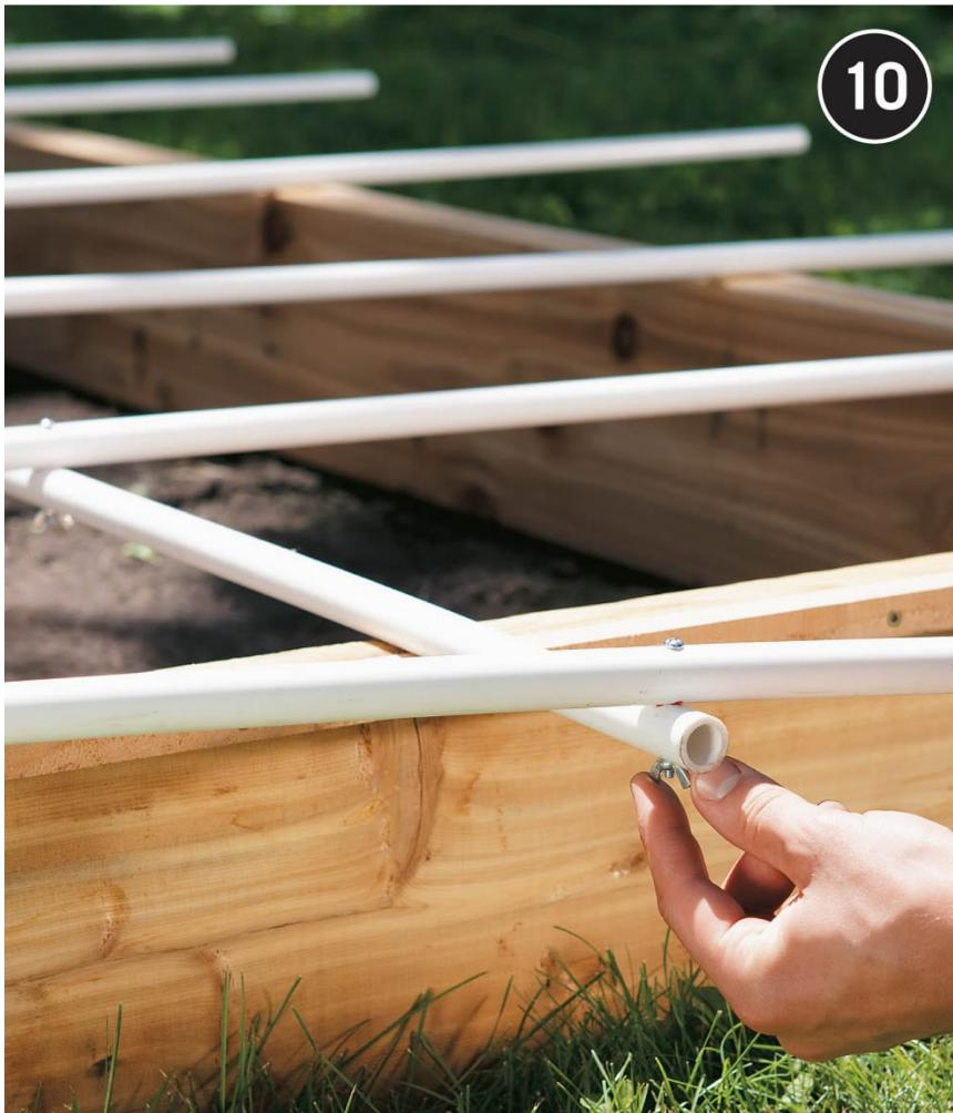
**Assemble the cover frame,** using  $1\frac{1}{2}$ " machine bolts and wing nuts. Fit a rib over the top of the ridge pole at each hole location. Insert the bolt through the rib and ridge and secure with a wing nut. The wing nuts allow for quick disassembly of the frame.
