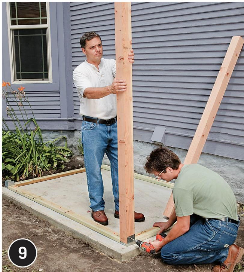
**Tack the posts** in the standoff post bases with a couple of deck screws, making sure they are resting cleanly on the standoff pads. Also brace the posts with  $2 \times 4$  braces so they are plumb. Tack all the posts in position and plumb them and then mark level cutting heights using a laser level or level for reference.
