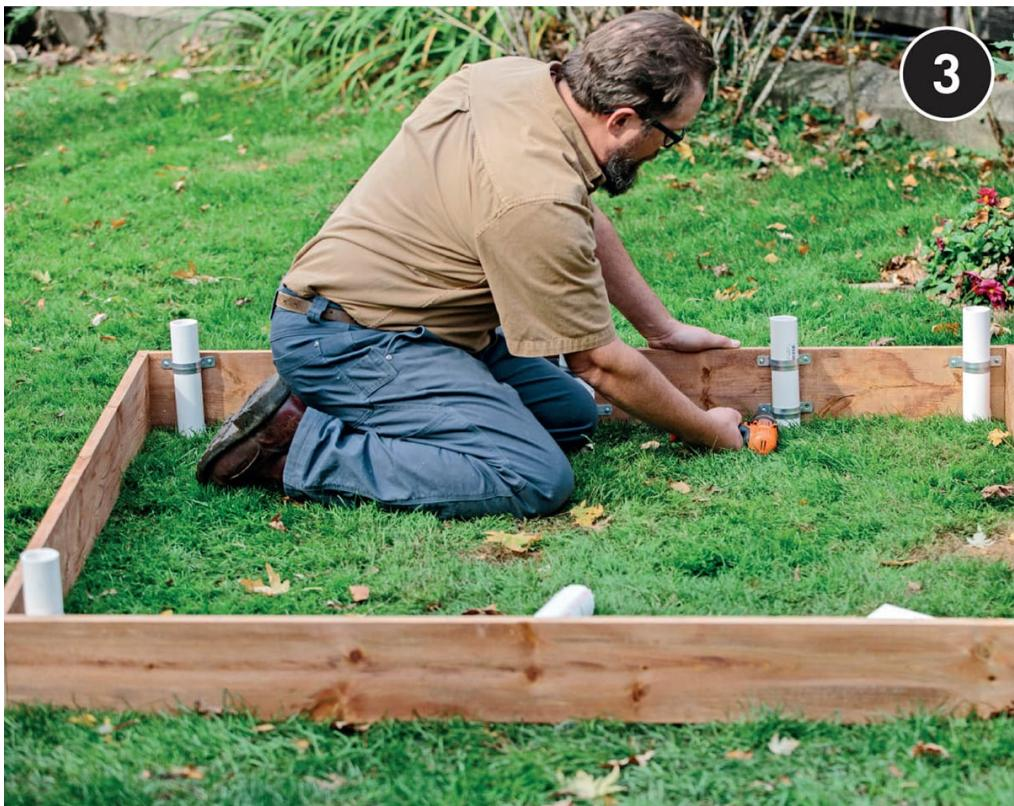
**Attach the PVC pipes** to the inside frame faces, spacing them 1' apart. Use two pipe strap clamp brackets per pipe. The pipes should project about 1" above the top edge of the frame side.
