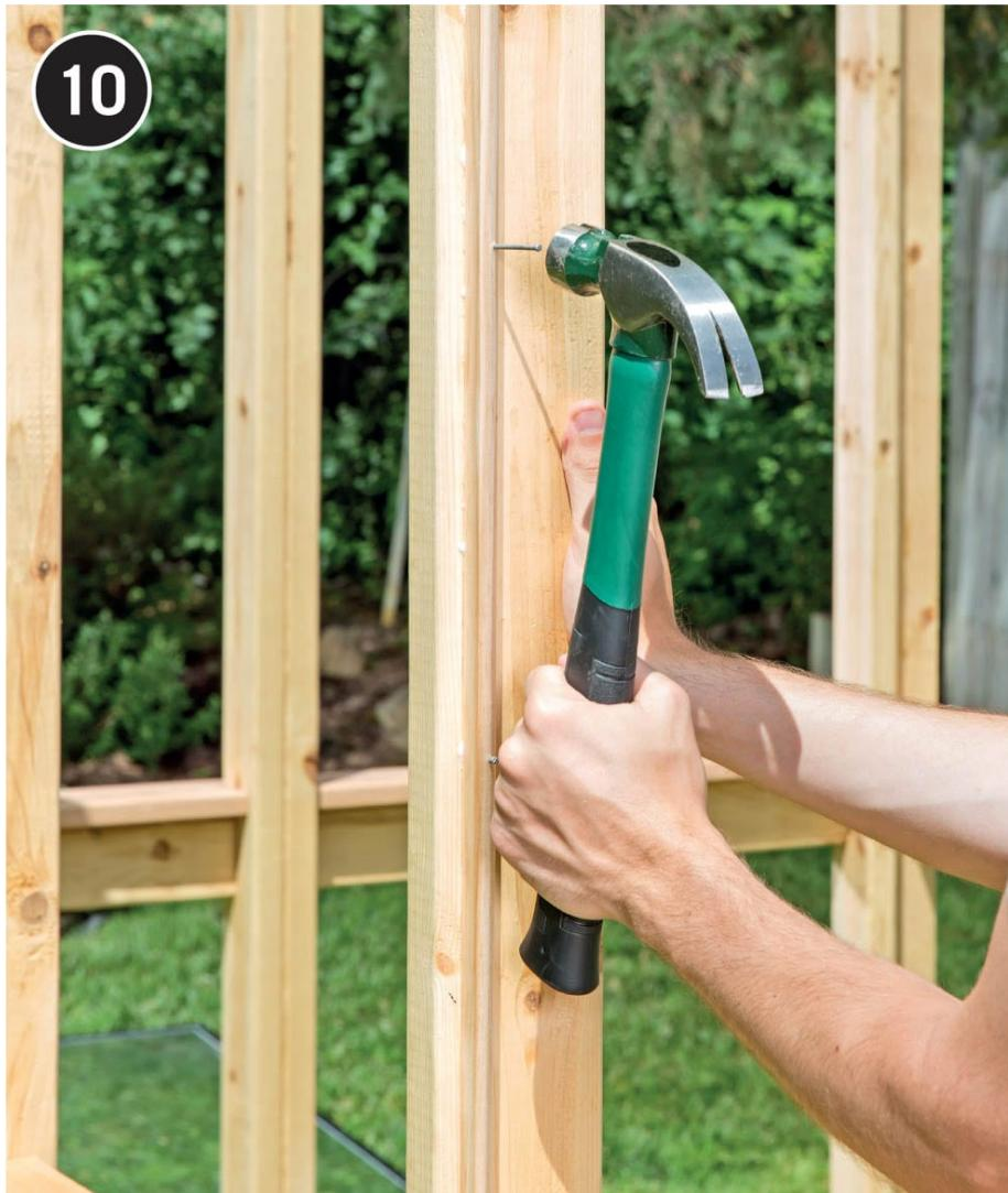
**Miter-cut retainer strips** from  $\frac{3}{4}$ " quarter-round stock for the window openings. Drill pilot holes for nailing, then coat the bottom faces of the strips with construction adhesive and nail them in place with exterior finish nails. You may have to adjust for the windows you reclaim. The windows here varied in height by up to  $\frac{1}{2}$ ".
