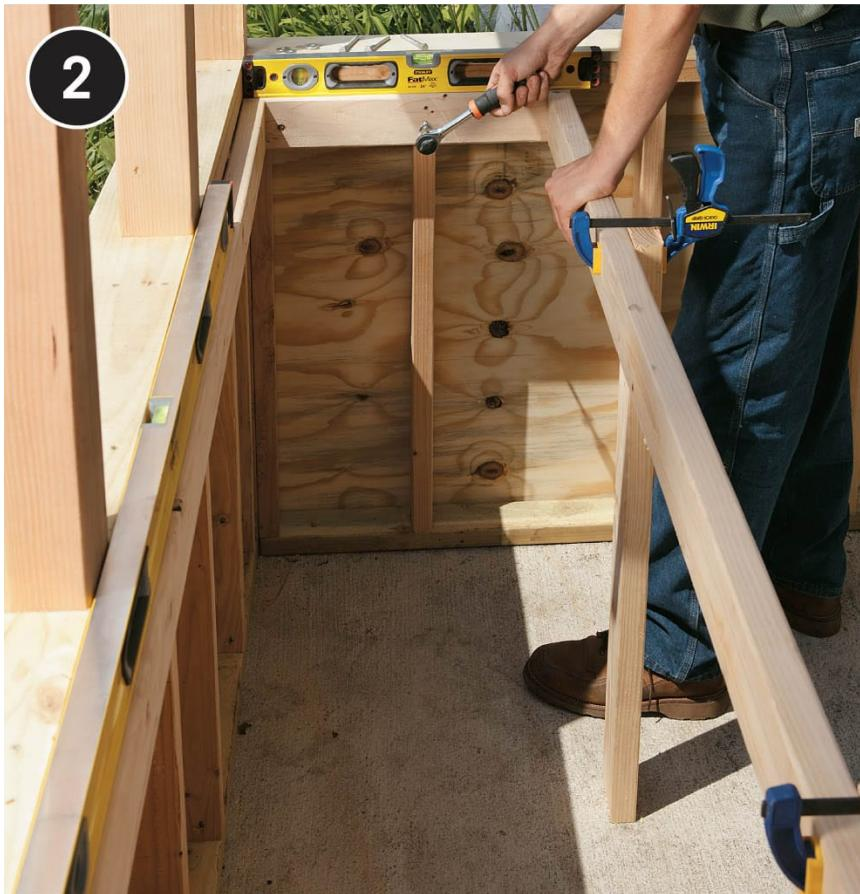
**Attach the benchtop frame** to the greenhouse wall studs using  $\frac{3}{8} \times 3$ " lag screws. Before driving the lag screws, tack the back of the frame to the long wall with deck screws. The tops should be 36" above the floor. Then, clamp a  $2 \times 4$  brace to the front rail of the frame and adjust it until level. Drill guide holes and drive one lag screw per wall stud at the back rail and on the ends.
