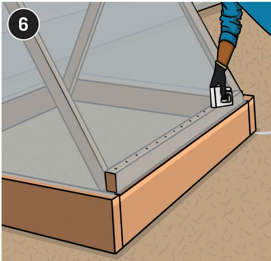
**Cut the 1 x 2 to length** for the door flap, if necessary. Wrap the free end of the plastic sheet around the board, until the board sits flush against the base brace with the door closed (the plastic will overlap the leg edges on both sides). When you're sure the length is correct, staple the plastic to the weight board.
