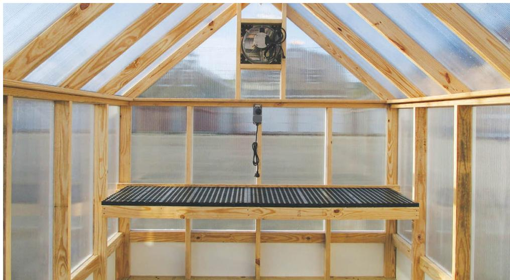
**A built-in gable-end workbench** provides abundant work surface that takes up as little space as possible (notice that the lack of legs leaves a wealth of storage space underneath). A rubber top surface is low maintenance, easy to clean, and the ideal durable material for the greenhouse. It won't rot, collect mold, or degrade under prolonged sunlight exposure.
