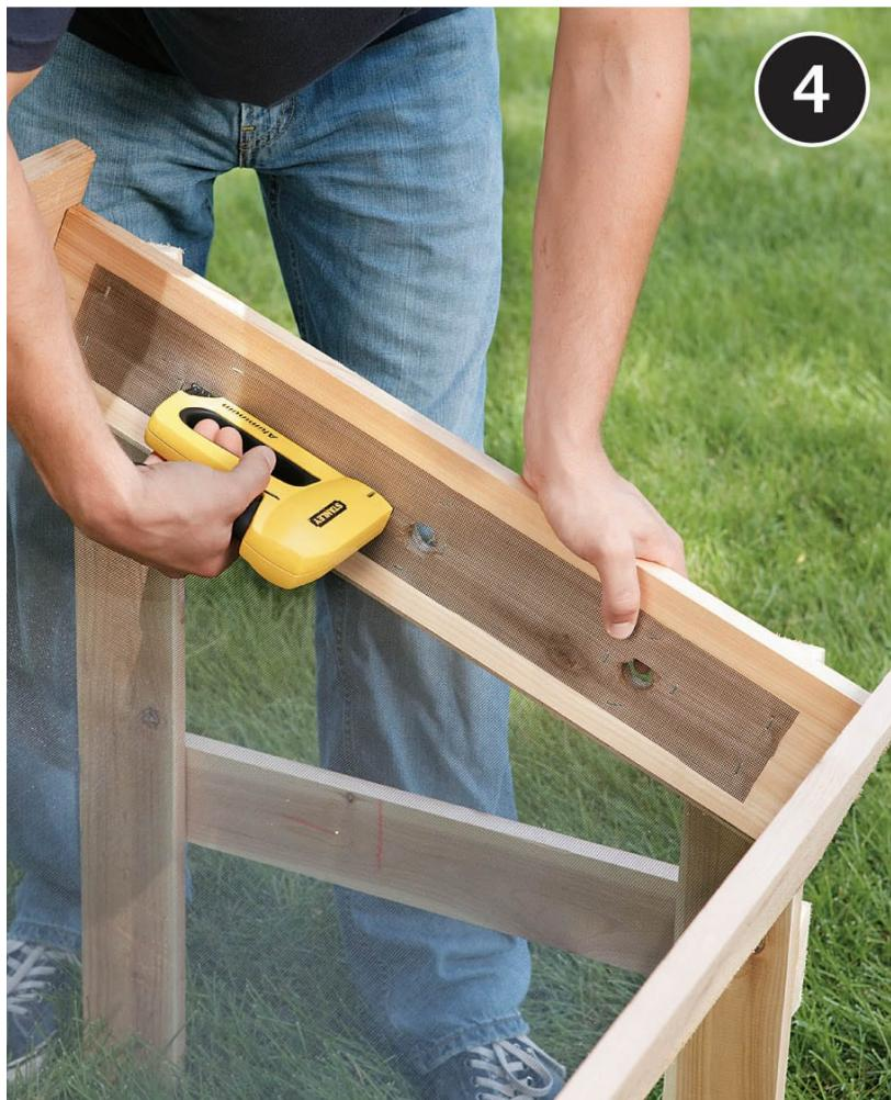
**Drill three 1" holes** for ventilation in each 1 × 6" board equally spaced along the length of the board, leaving 5" of room on each end for the posts. Staple leftover insect mesh behind the ventilation holes on the inside of the frame.
