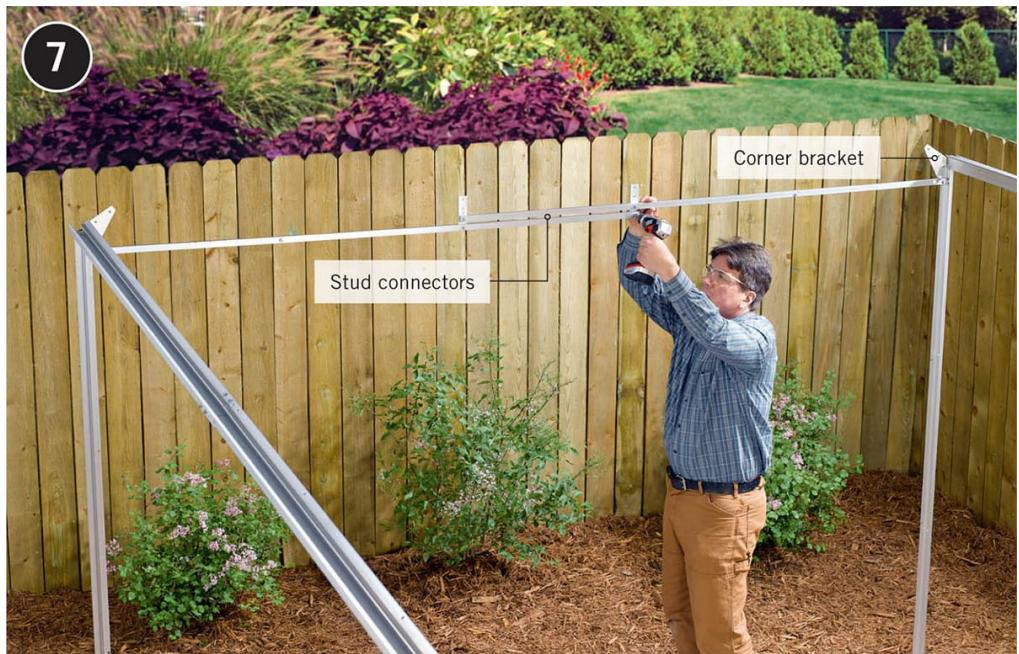
**Attach the other side ceiling plate** along the other side, flat against the inside of the corner studs. Then attach corner brackets to the rear studs, and construct the back top plate by attaching the rear braces to the corners and joining the braces together with stud connectors.
