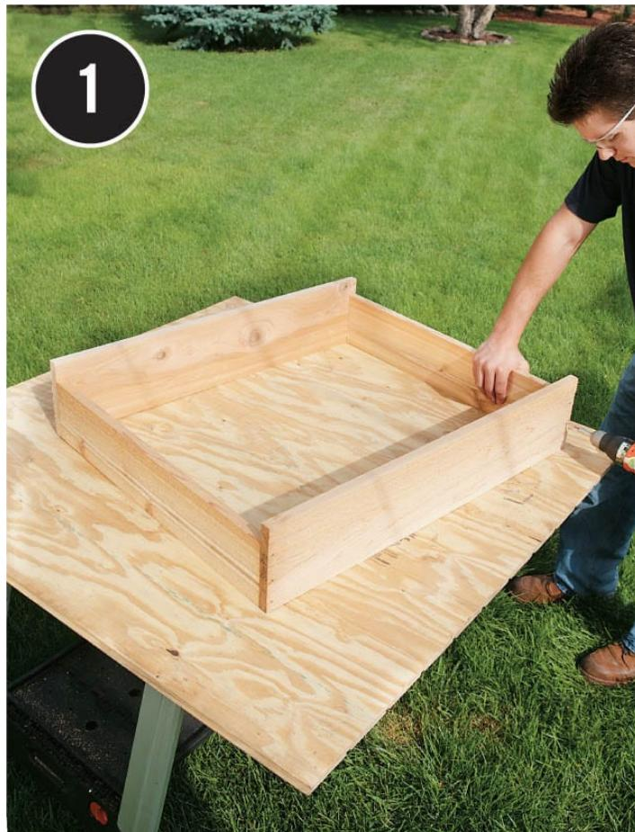
**Assemble the box.** Attach the wider boards for the frame by driving 2" screws through the faces of the 1 x 8" boards into the ends of the 1 x 6" boards. There will be a difference in height between these pairs of boards so that the window sash can sit flush in the recess created.
