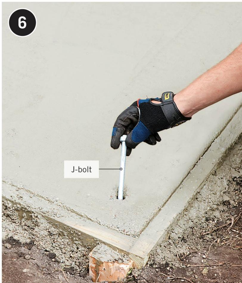
**Set J-bolts into the concrete** after it sets up and after you have rounded the edges with an edger tool. Make sure to follow your plan closely for the J-bolt positions. Cover the concrete with sheet plastic and allow it to dry overnight before removing the forms.
