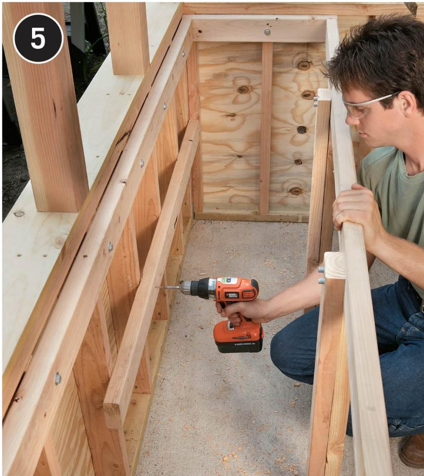
**Attach a 2 × 4 ledger** to the front wall studs to support the 2 × 4 shelf supports that run from the front of the bench to the wall. Use 3" deck screws driven at kneewall stud locations.
