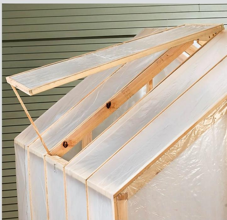
**OPTION:** Make a vent window. First, cut a hole in the roof in one rafter bay and tack the cut edges of the plastic to the faces (not the edges) of the rafters, ridge pole, and wall cap. Then build a frame from 1 x 2 stock that will span from the ridge to the top of the kneewall and extend a couple of inches past the rafters at the side of the opening. Clad the frame with plastic sheeting and attach it to the ridge pole with butt hinges. Install a screw-eye latch to secure it at the bottom.
