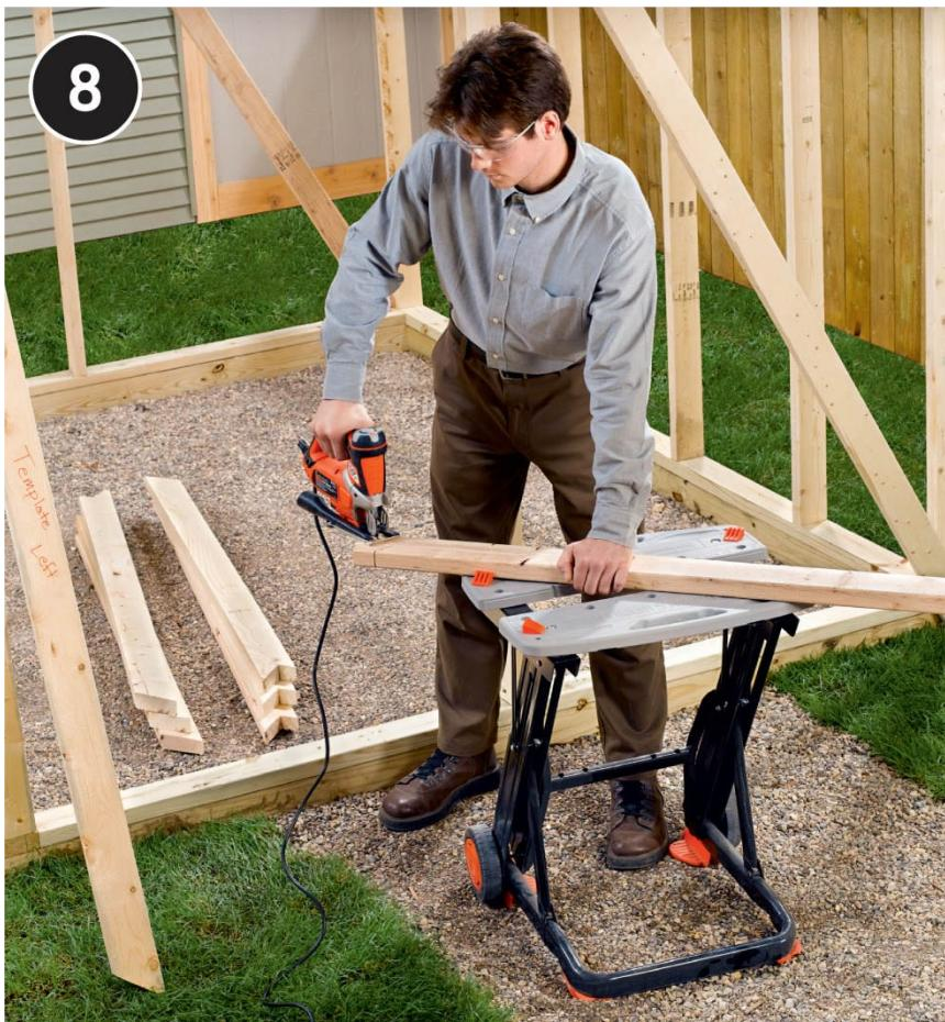
**Mark and cut the remaining rafters**, using the template to trace the cutting lines onto each piece of stock.
