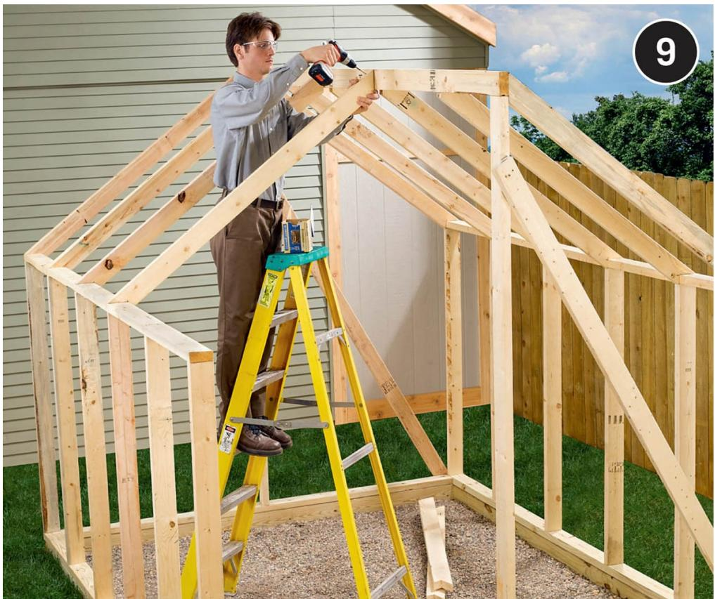
**Install the rafters,** using the deck screws driven at an angle into the kneewall caps and the ridge. The rafters should be aligned with the studs and perpendicular to the ridge.
