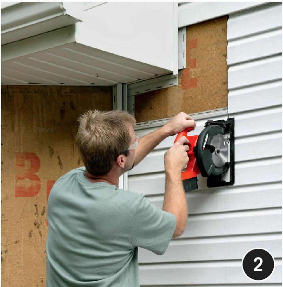
**Prepare the house walls** for installation of the vertical wall tracks. Mark a cutting line on the siding at the track location and remove siding so you can fasten the tracks to the wall sheathing.
