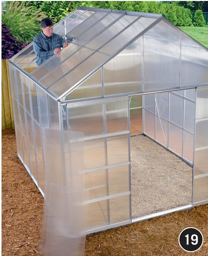
**Install the roof panels and roof-window panels** so that the top edges fit up under the edge of the crown or window support and the bottom edges align over the gutters.
