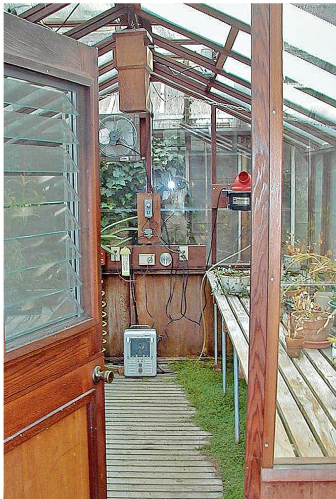
**A portable space heater** may be all the supplemental heat your greenhouse requires. Use it with caution, and make sure yours shuts off automatically if it overheats or is knocked over.
