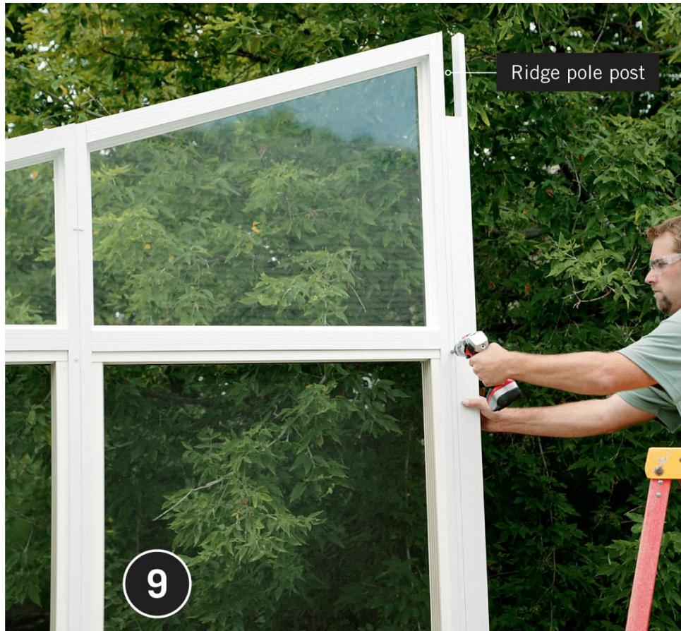
**Continue installing panels on the second wall.** If it is a gabled wall, install panels up to the midpoint; then cut the three-part, ridge pole support post to fit, and install it by driving screws through the post and into the wall panel. Make sure the saddle formed at the top of the post is sized to accept the ridge pole.
