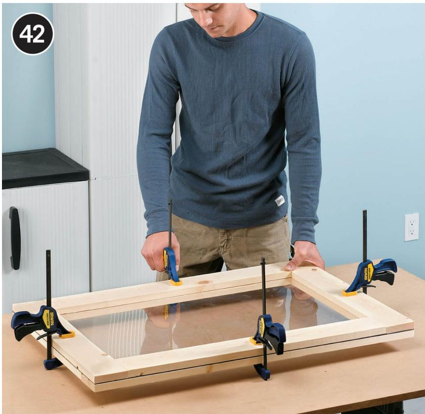
**Cut the rails and stiles** for the window frame to length from 1 × 4 pine stock. Assemble the frame parts around the glazing panel, clamping them together temporarily. Use the glazing panel as an alignment reference: if the panel is square and the frame edges are flush with the glazing all around, your window is square.
