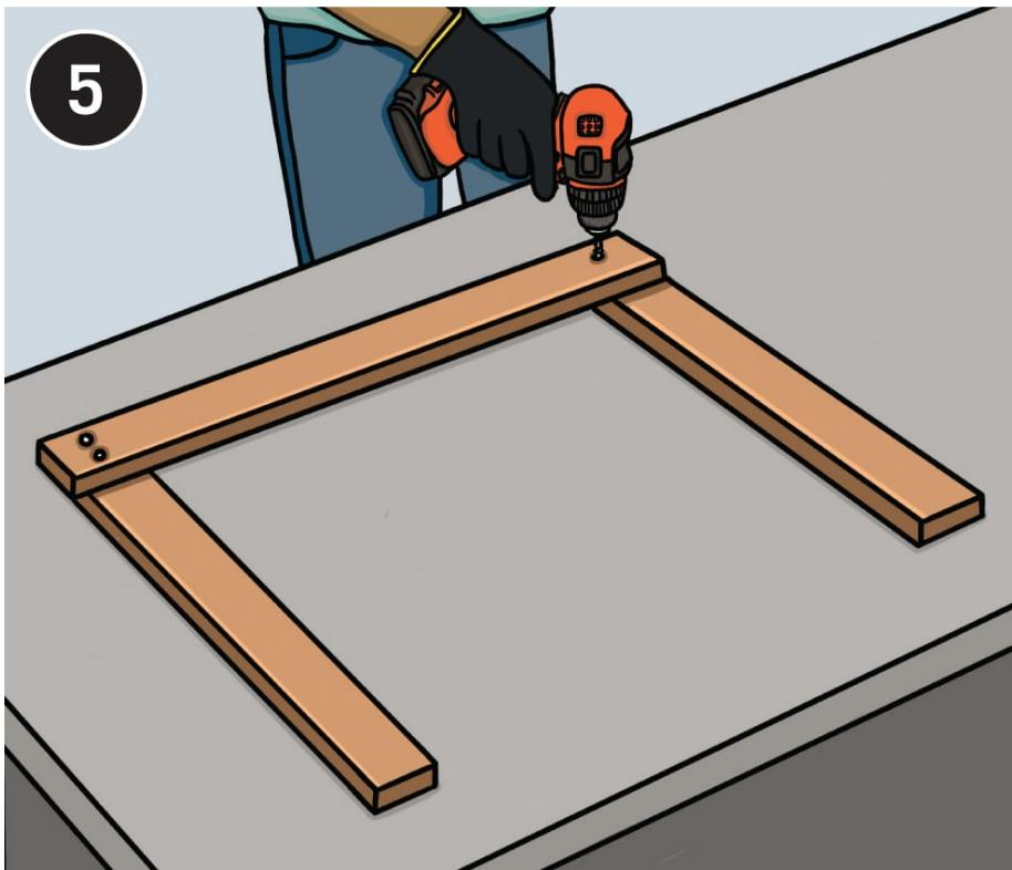
**Set two 4 x 4 legs** on a flat, level work surface, parallel to each other. Place a side skirt board across the legs. Align it flush to the end and the outside edge of each leg. Drill a two pilot holes on each end of the board, and screw the skirt board to the legs with 2" deck screws.
