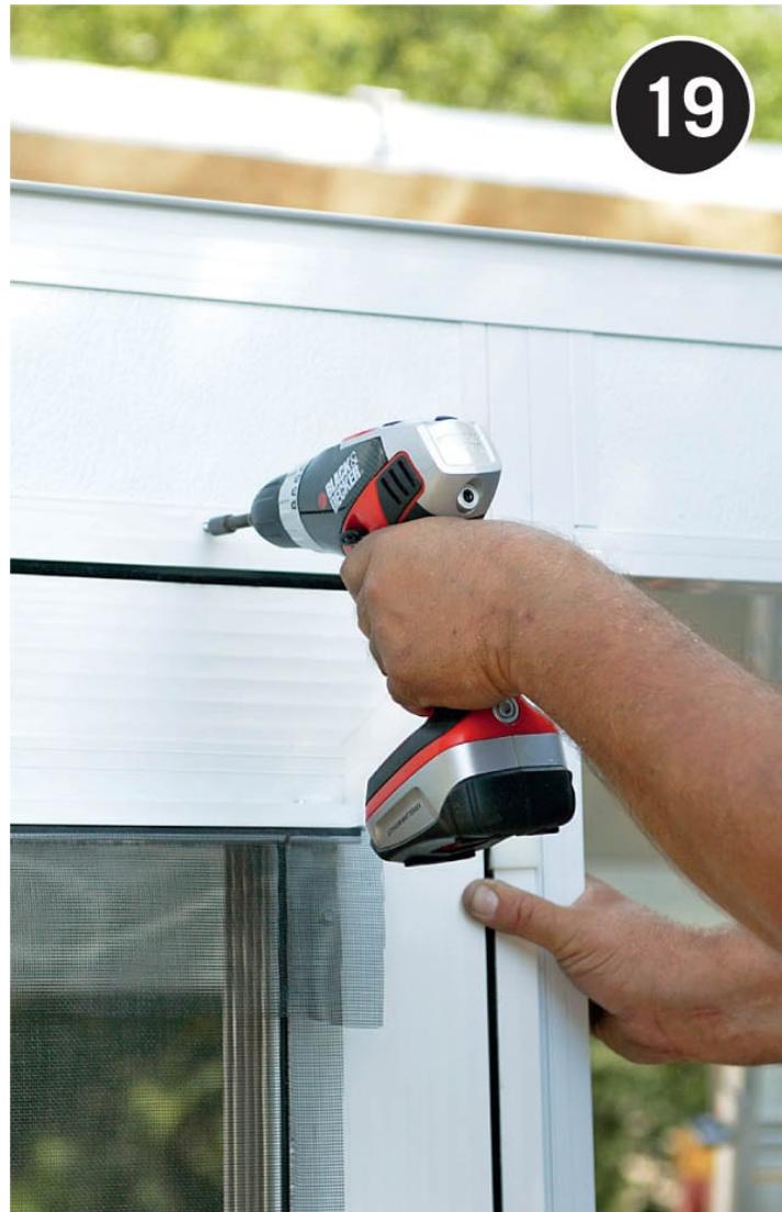
**Install the prehung doors** by fastening the door nailing flanges to the frames that create the door opening. Make sure the door is level and plumb before driving fasteners. Attach the door handle and latch.
