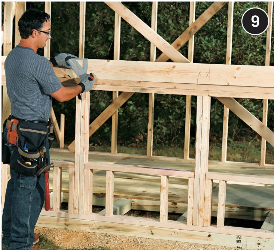
**Cut the 2 × 6 ridge board** (154 $\frac{3}{4}$ "). Mark the rafter layout onto the ridge and front and rear wall plates following the FRONT FRAMING and REAR FRAMING. Install the A and B rafters and ridge. Make sure the B rafters are spaced accurately so the windows will fit properly into their frames; see the WINDOW SECTION ([here](#)).
