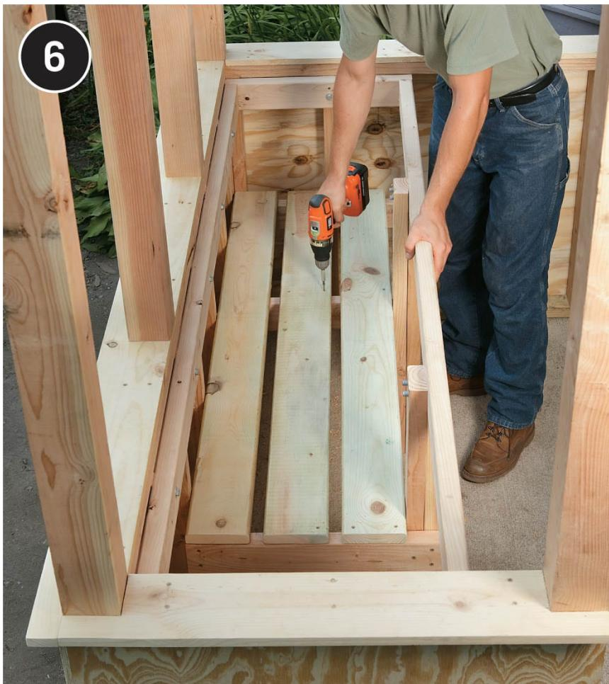
**Attach 2 × 4 shelf supports** to the legs and attach a 2 × 4 shelf support to the endwall. Then, fasten the shelving material to the tops of the supports. The best height for the shelf depends on the height of the containers you plan to set on the shelves beneath the removable section of the top.
