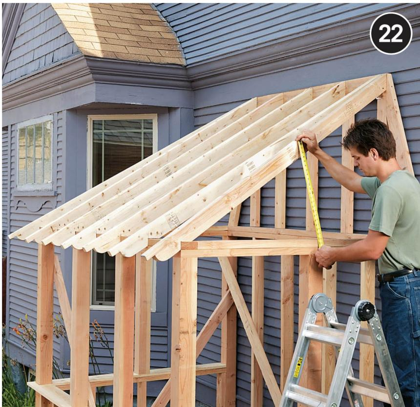
**Measure from the corner rafters** to the endwall headers to find the lengths for the side rafters in the hip wall configuration. Cut 2 × 4 workpieces to length for each rafter.
