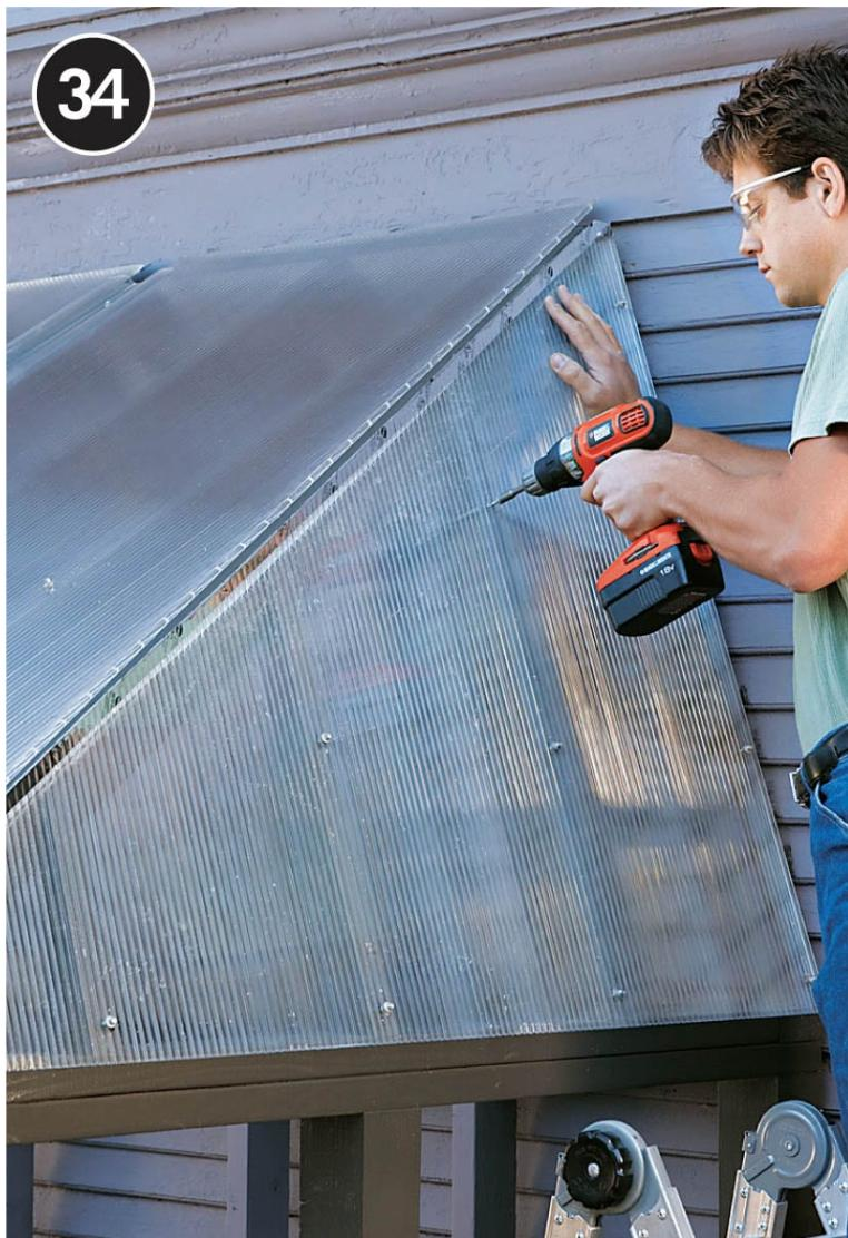
**Cut the side roof panels to fit** and attach them with rubber gasket screws. The hip seams will be covered with flashing (see [here](#)).
