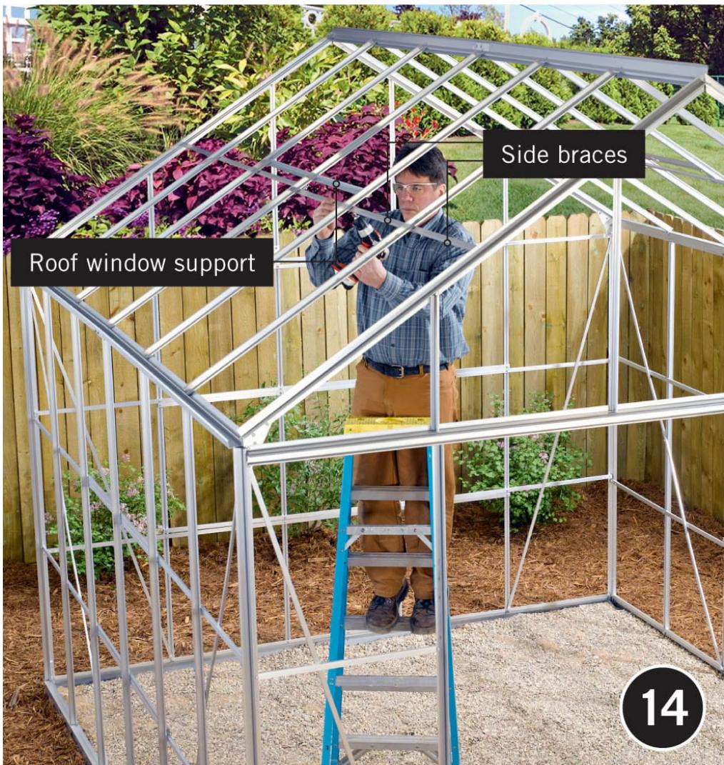
**Attach the side braces** and the roof-window support beams to the underside of the roof rafters, as specified by the manufacturer's instructions.
