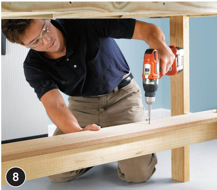
**Complete the pot shelf** by cutting the remaining half-piece of deck board to length. Position the board so it is centered side-to-side over the stretcher and overhangs both leg supports by  $\frac{3}{4}$ ". Fasten the board to the stretcher and leg supports with  $2\frac{1}{2}$ " deck screws driven through pilot holes.
