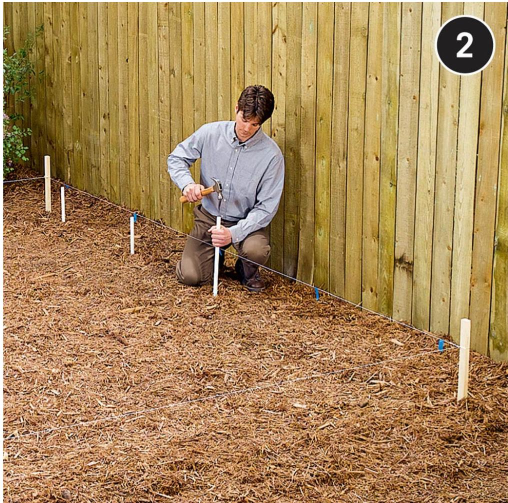
**Cut a 24"-long stake** from  $\frac{1}{2}$ " CPVC pipe for each leg of each frame hoop. Plastic pipe is easy to cut with a plastic tubing cutter or a hacksaw. Mark the layout strings at 36" intervals, using tape or a marker. Drive a stake at each marked location, using a hand sledge or hammer. Keep the stakes plumb and drive them in 14" deep, so only 10" is above ground.
