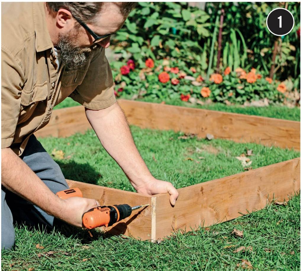
**Clear the hoophouse site** of large rocks and yard debris. On a clean, flat surface, assemble the base frame by drilling pilot holes through the frame edges and screwing the frame together with 2" galvanized screws. Cut individual branches with loppers to length as necessary. Cut off or sand down any protrusions that might puncture the plastic.
