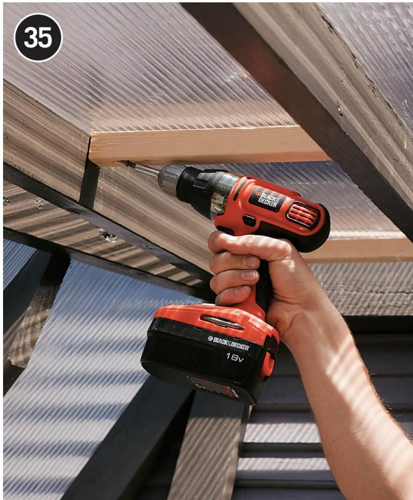
**Frame openings for the roof vent cutouts.** Install a pair of parallel framing members at the top and bottom of each opening. The tops of the frames should be flush against the roof panel.
