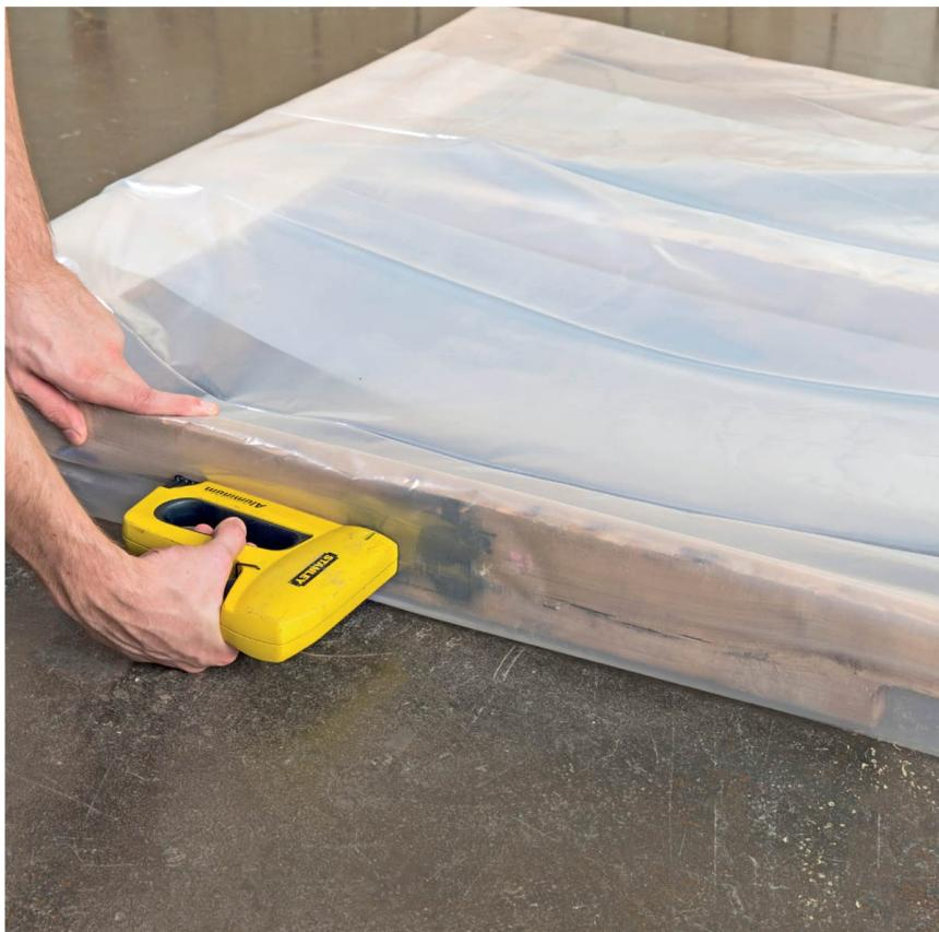
**Modifying a pallet like this**—removing the center rails and replacing them with 6-mil polyethylene sheeting—is one of the many ways you can upcycle these handy throwaways. This crude “window” can be used as a building block to form walls and a roof for a greenhouse.
