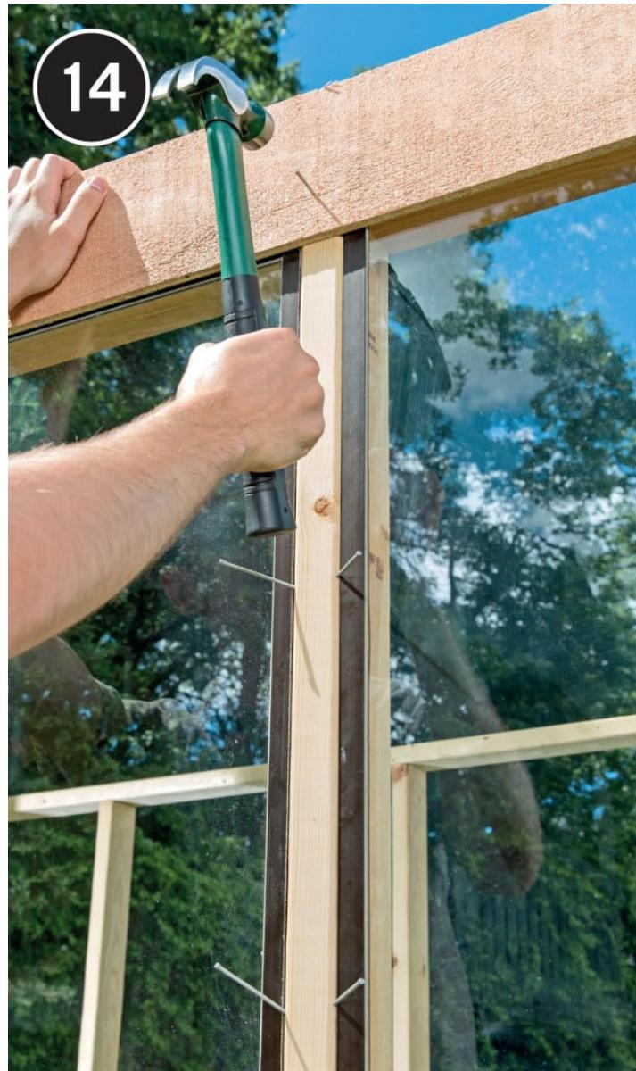
**Measure and cut 2 x 6 fascia boards** for the top of each wall. Use 3" 6d galvanized nails to tack the board to the top plates of the wall all the way around. The fascia should cover any gaps at the tops of the windows.
