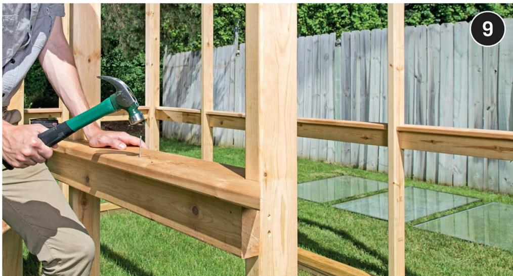
**Dry-fit the cedar sills** and then miter the corners if the fit is correct. Coat the tops of the spreaders with construction adhesive and nail the cedar sills in place with exterior finish nails.
