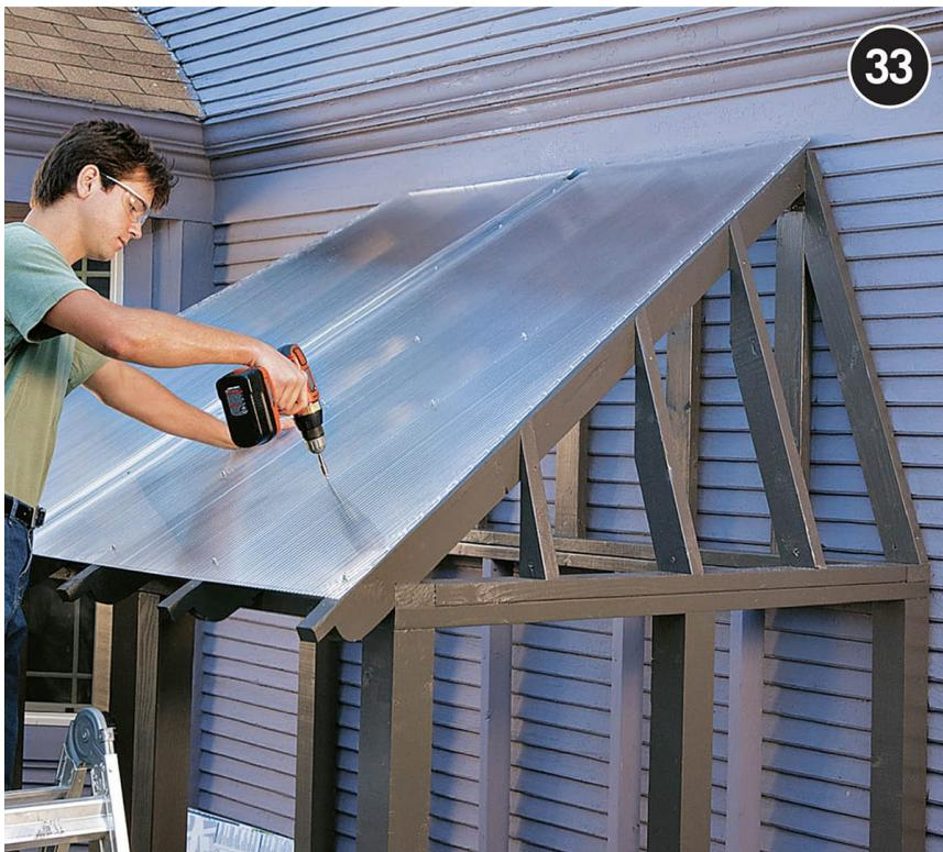
**Fasten the roof panels** with rubber-gasket equipped pole barn screws driven every 12" at each rafter or purlin. Take care not to overdrive the screws, but be sure they penetrate far enough to create a tight seal.
