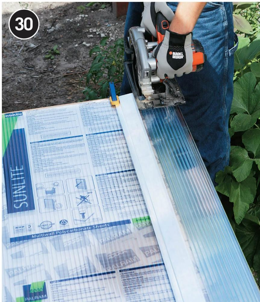
**Cut the first roof panel to rough size** using a circular saw fitted with a fine-tooth panel-cutting blade. Use a straightedge cutting guide. Or, use a tablesaw if you have access to one.
