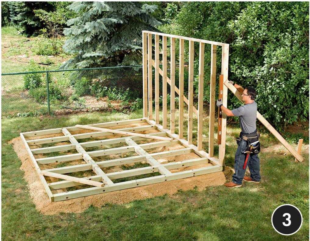
**To frame the rear wall,** cut one top plate and one pressure-treated bottom plate (142 $\frac{3}{4}$ "). Cut twelve studs (81"). Assemble the wall following the layout in the REAR FRAMING ([here](#)). Raise the wall and fasten it to the rear rim joist and the intermediate joists, using 16d galvanized common nails. Brace the wall in position with 2 x 4 braces staked to the ground.
