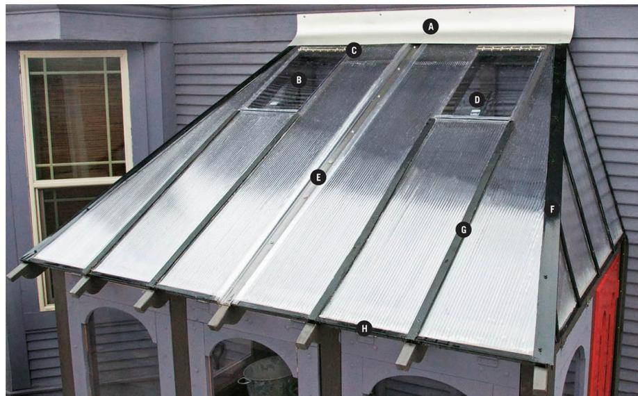
**Add trim elements to complete the roof.** Parts of the roof trim system include: flashing over ridge (A); clear vent panel (B) attached with piano hinge (C) and automatic closer (D); seaming strip (E); metal drip cap for edges (F);  $\frac{1}{4} \times 1\frac{1}{2}$ " wood battens at rafter locations (G); vinyl cap molding at eave edges (H).
