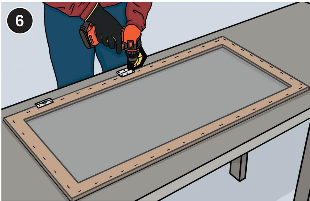
**Screw the butt hinges** to the frame. Set the frame in place on the cold frame, and screw the hinges to the back wall.
