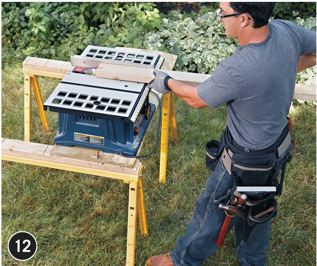
**Create the inner and outer window stops** from 10'-long 2 × 4s. For stops at the sides and tops of the roof windows and all sides of the front wall windows, rip the inner stops to 2¼" wide and the outer stops to 1" wide; see the WINDOW SECTION and WINDOW DETAIL ([here](#)). For the bottom of each roof window, rip the inner stop to 1½"; bevel the edge of the outer stop at 45°.
