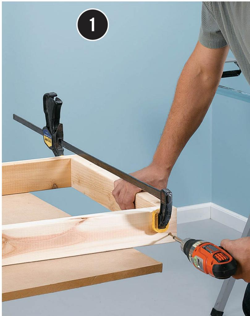
**Assemble the top frame** by clamping the side pieces over the ends of the end pieces so they're flush along the top edges. Fasten each corner with two  $3\frac{1}{2}$ " deck screws.
