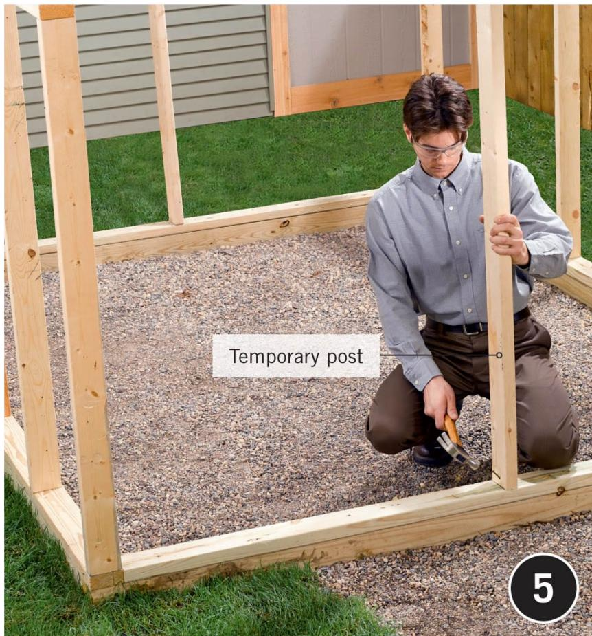
**Begin the endwalls** by cutting and installing the end sole plates to fit between the side plates, using 3" deck screws. Cut the ridge support posts to length. Toenail one post at the center of each end sole plate. Check the posts with a level to make sure they're plumb before fastening.
