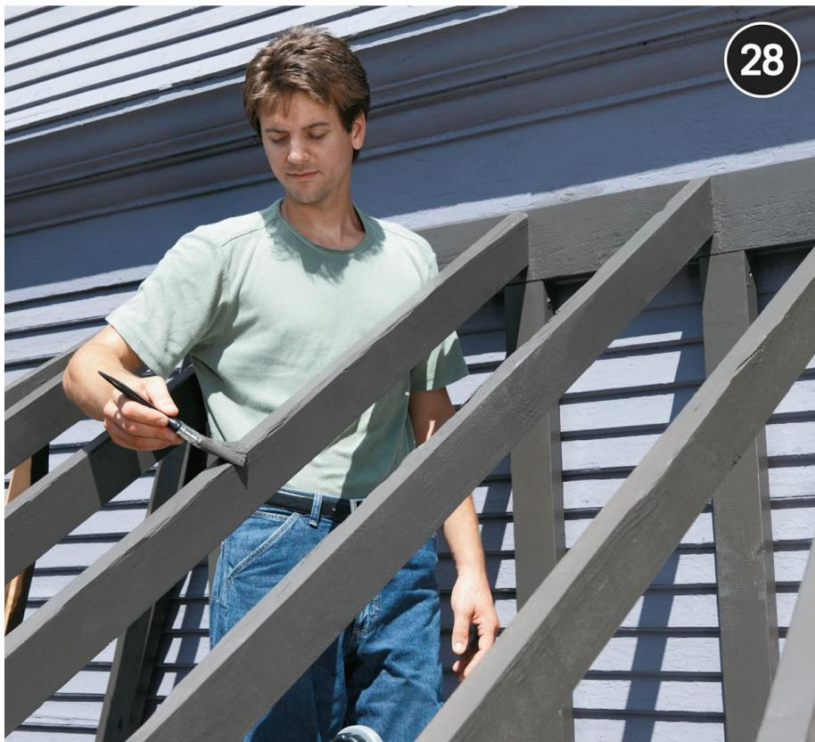
**Also seal the roof structure with paint** before installing the roof panels. The charcoal colored paint seen here recalls the color of wrought iron, which was used frequently to construct greenhouses and related Victorian structures, such as orangeries.
