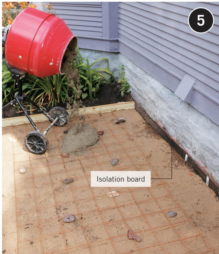
**Pour concrete into the form.** For a slab of the dimensions shown (4" thick by 68 × 84") approximately 15 cu. ft. (1/2 yard) of concrete is required (thirty 60-pound bags of dry mix). Settle the concrete by rapping the forms lightly with a mallet, and then strike off the material before floating.
