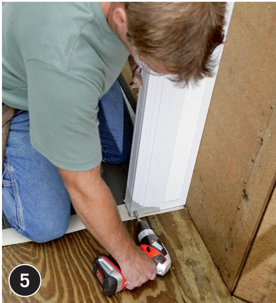
**Install the first wall panel.** In many cases, the first panel will be a narrow filler strip that is simply a solid wall panel and does not contain windows. Install the panel by driving 1" self-tapping screws through the floor track flanges and into the bottom frame of the panel. Make sure the panel is plumb and firmly seated against the track.
