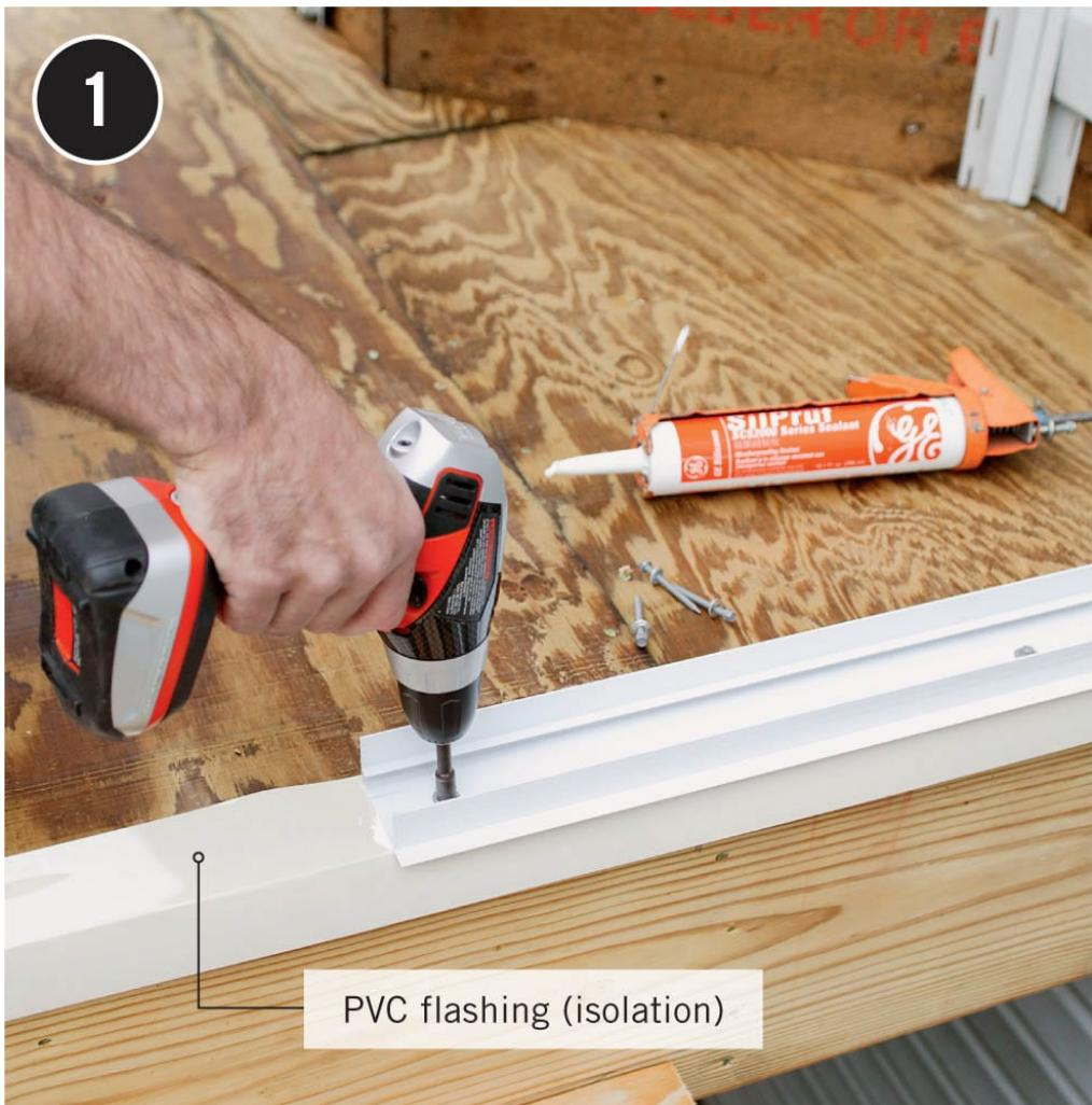
**Install the aluminum floor track channels** at the perimeter of the installation area. Use a bead of weatherproof silicone sealant and self-tapping, 2" hex-head screws with EPDM rubber washers to secure the track. Square layout lines should be marked prior to installation. If your plywood substrate layer is treated with ACQ or copper azole wood treatment, protect the aluminum tracks from corrosion by installing an isolation layer of PVC flashing (sold in rolls).
