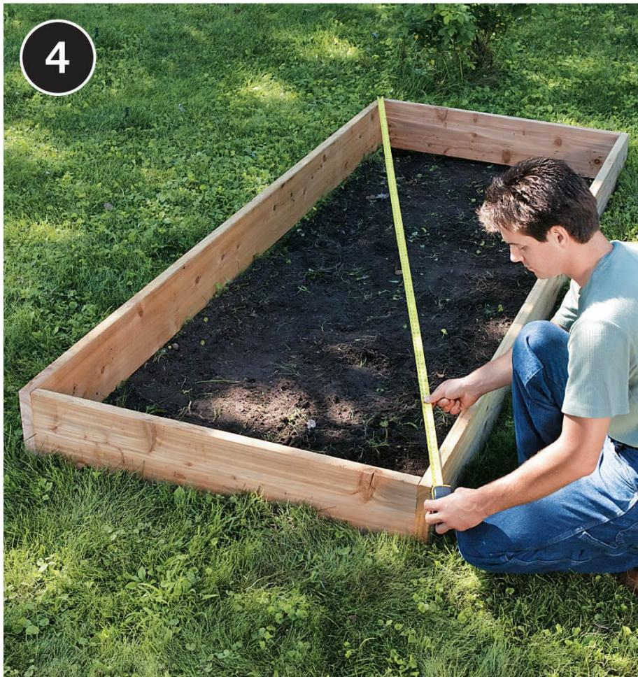
**Set the bed frame into place**, then measure diagonally between opposing corners to check for square: the frame is square when the measurements are equal.
