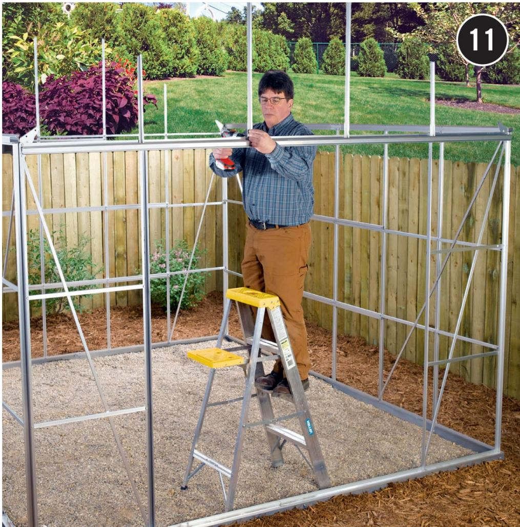
**Fasten the gable-end stud extensions** to the front and back walls of the greenhouse. The top ends of the studs should angle upward, toward the peak of the greenhouse.
