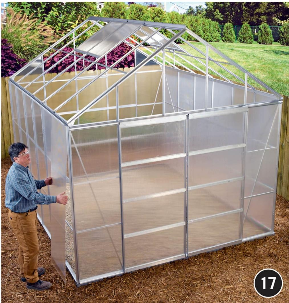
**Install the panels one by one**, using panel clips. Begin with the large wall panels. Position each panel and secure it by snapping a clip into the frame, at the intervals specified by the manufacturer's instructions.
