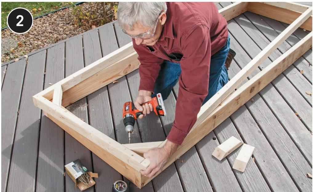
**Stabilize the corners** of the canopy frame with braces cut to 45° angles at both ends. Install the braces on-the-flat, so their top faces are flush with the tops of the canopy frame. Drill pilot holes and fasten through the braces and into the frame with one 2½" screw at each end. Then, drive one more screw through the outside of the frame and into each end of the brace. Check the frame for square as you work.
