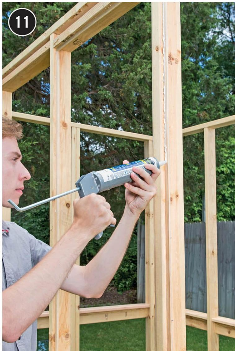
**Lay a thin bead** of clear silicone caulk into the retainer strip channel for the first window.
