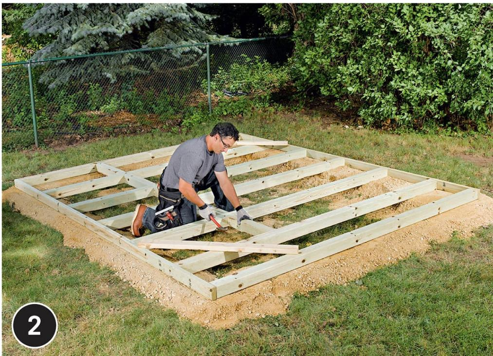
**Cut ten 4 × 4 blocks** to fit between the joists. Install six blocks  $34\frac{1}{2}$ " from the front rim joist, and install four blocks  $31\frac{1}{2}$ " from the rear. Toenail the blocks to the joists. All blocks, joists, and sills must be flush at the top.
