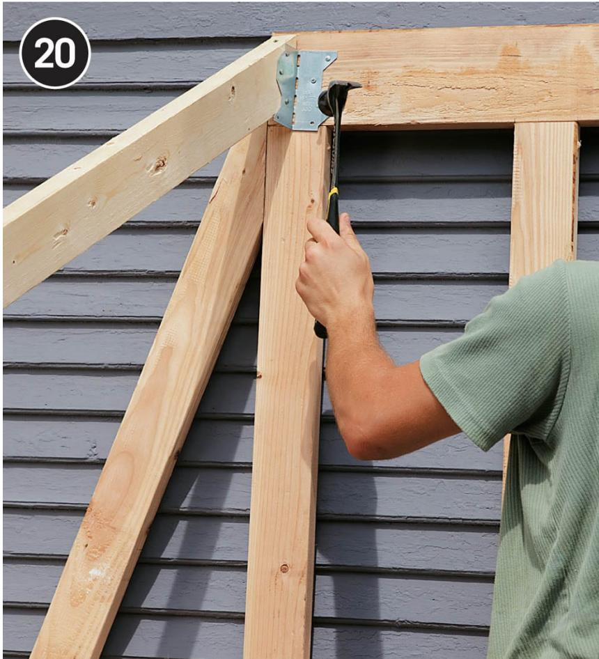
**Install the corner rafters.** First, attach skew joist hangers to the ends of the ridge pole for the skewed rafters that extend out to the front corners. Nail the rafters into the hangers with joist hanger nails. Toenail them (or drive screws toenail style) to the header.
