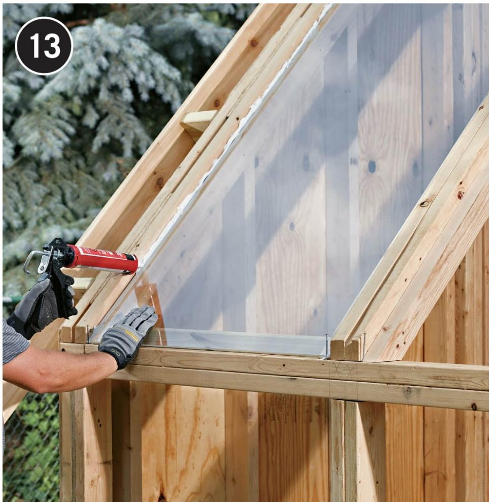
**Install each window as follows.** Attach inner stops as shown in the drawings, using galvanized finish nails. Paint or varnish the rafters and stops for moisture protection. Apply a heavy bead of caulk at each location shown on the drawings (HEADER + WINDOW DETAIL, WINDOW SECTION/DETAIL, TABLE + LOWER WINDOW DETAIL). Set the glazing in place, add another bead of caulk, and attach the outer stops. Cover the rafters and stop edges with 1 x 4 trim.
