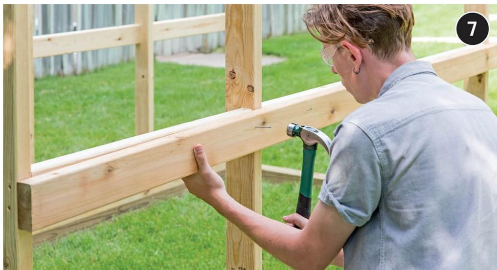
**Face-nail** a  $2 \times 4$  cedar ledger around the perimeter of the greenhouse so that the top of the ledger is flush with the tops of the  $2 \times 4$  spreaders.
