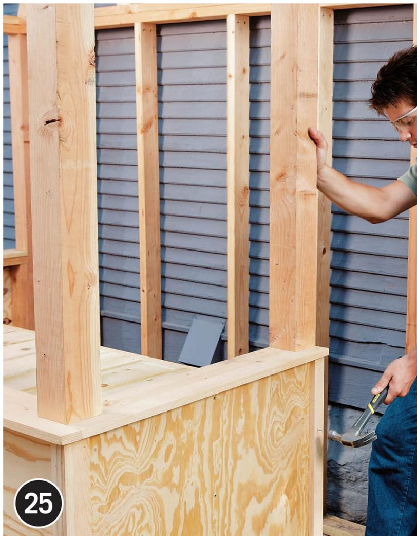
**Cut and install trim boards and corner boards** according to your plan for siding the kneewall. The tops of the trim boards should butt against the undersides of the sills.
