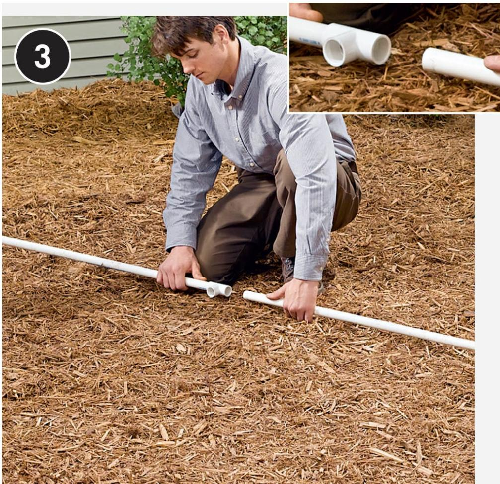
**Join the two legs** for each frame hoop with a fitting. Use a T-fitting for the end hoop frames and a cross fitting for the intermediate hoop frames. No priming or solvent gluing is necessary. (The friction-fit should be sufficient, but it helps if you tap on the end of the fitting with a mallet to seat it.)
