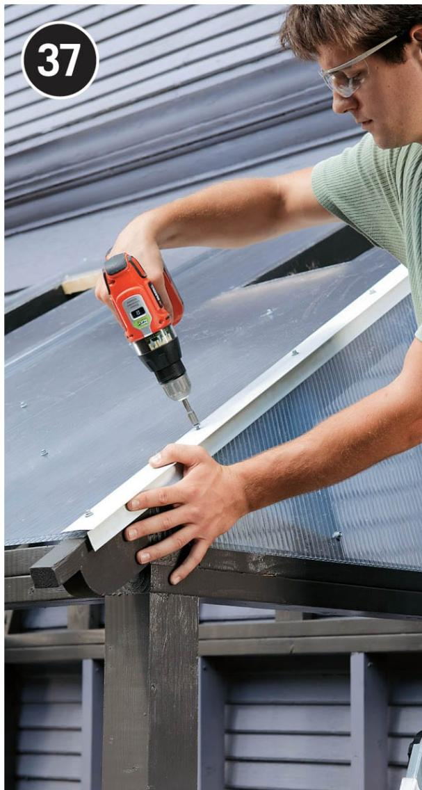
**Install flashing** over the hip roof seams. Here, common drip cap flashing is being fastened with rubber-gasket screws driven into the roof rafters.
