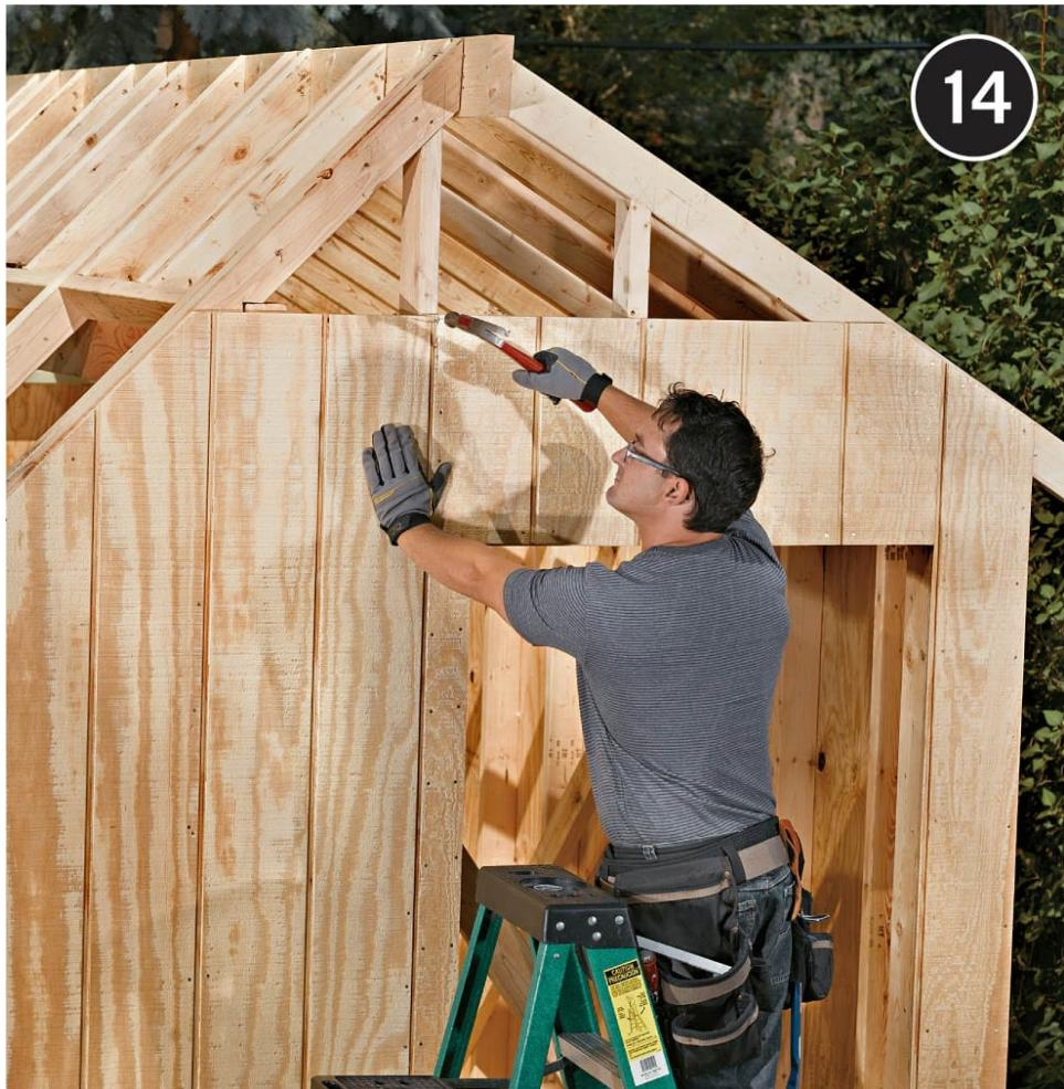
**Cover the walls with T1-11 siding**, starting with the rear wall. Trim the sheets as needed so they extend from the bottom edges of the rafters down to at least 1" below the tops of the foundation timbers. On the side walls, add Z-flashing above the first row and continue the siding up to the rafters.
