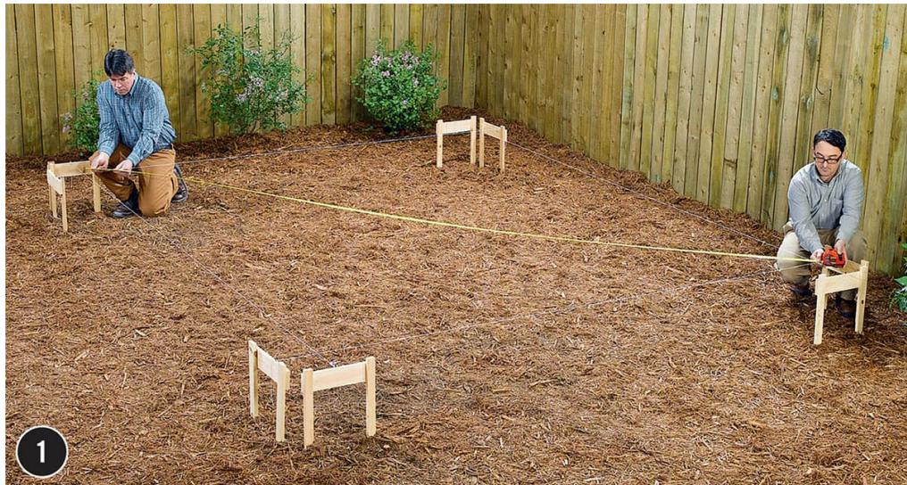
**Establish layout lines for the gravel subbase**, using stakes or batterboards and mason's string. The excavation area for the subbase should be at least 2" wider and longer than the outside dimensions of the greenhouse. Make sure the layout is perfectly square (the lines are perpendicular to one another) by measuring diagonally between opposing corners: the layout is square when the measurements are equal.
