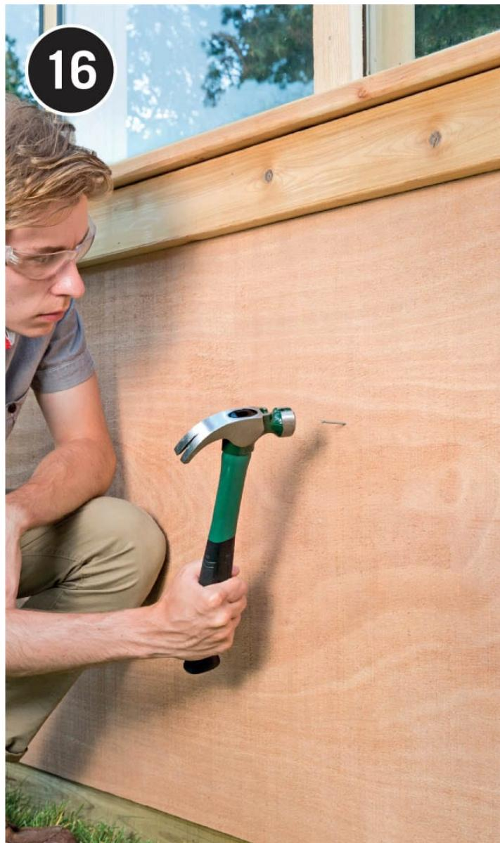
**Measure and cut  $\frac{1}{2}$ " exterior grade plywood** for the half-wall cladding at the bottom of each wall. Nail it in place with 2" 6d nails.
