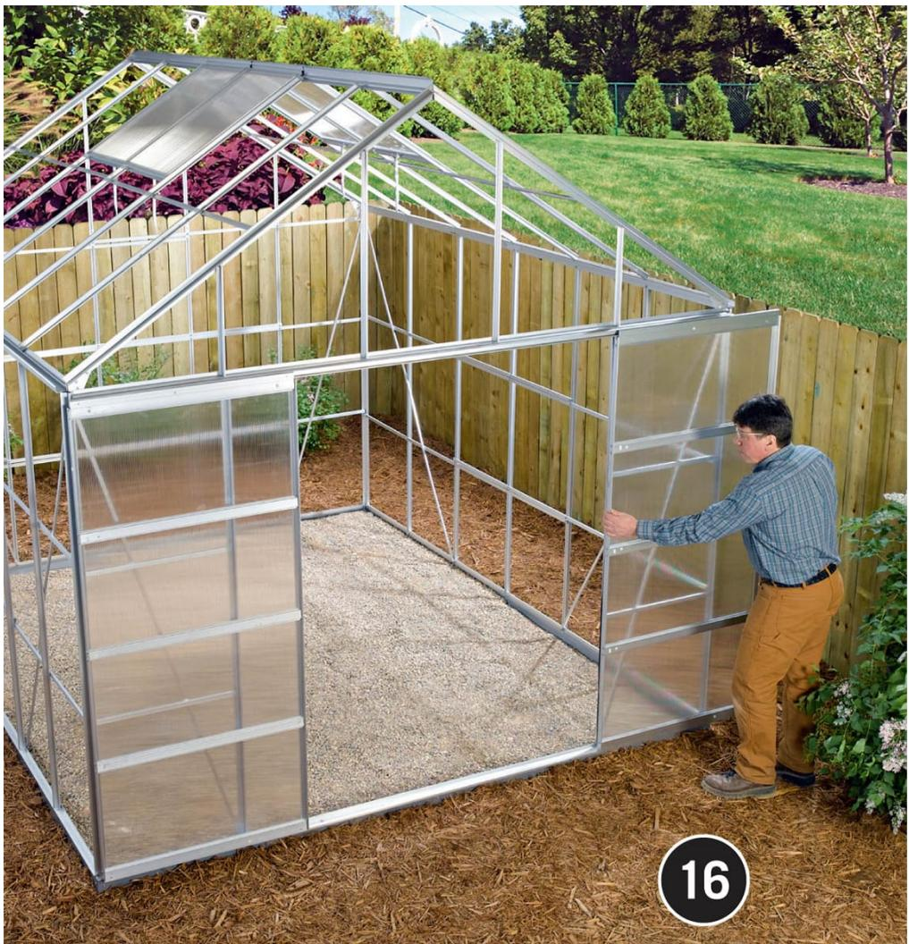
**Assemble the doors,** making sure the top slider/roller bar and the bottom slider bar are correctly positioned. Lift the door panels up into place onto the top and bottom wall plates.
