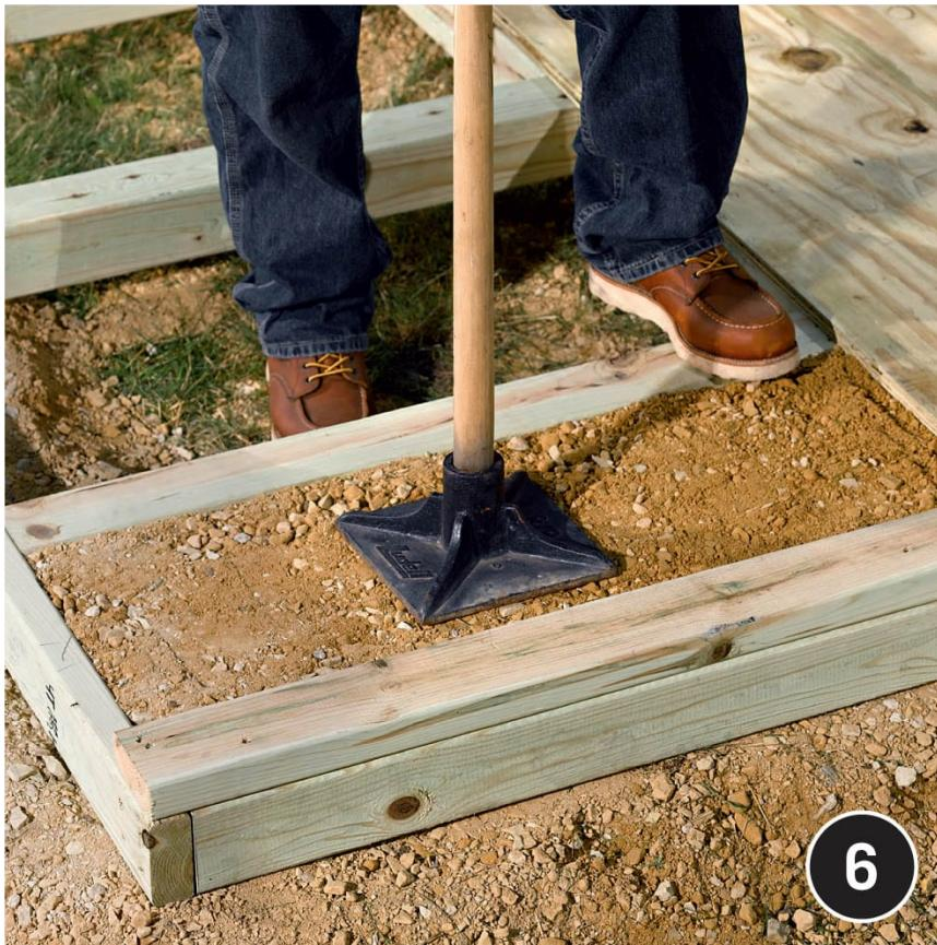
**Trim two sheets of  $\frac{3}{4}$ " plywood** as needed and install them over the joists and blocking as shown in the FLOOR FRAMING PLAN, leaving open cavities along the front of the shed and a portion of the rear. Fasten the sheets with 8d galvanized common nails driven every 6" along the edges and 8" in the field. Fill the exposed foundation cavities with 4" of gravel and compact it thoroughly.
