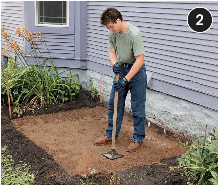
**Install a 4 to 6" thick layer of compactible gravel** to create a stable subbase. Tamp the gravel with a hand tamper or rental compactor. The tamped surface should slope away from the house at a very shallow rate—about  $1/16$ " per foot. Insert an isolation board strip (usually made of asphalt-impregnated fiberboard) between the slab area and the foundation wall to keep the structures separate.
