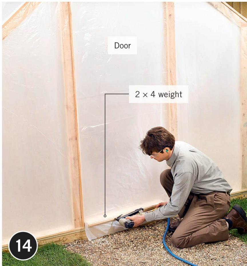
**Create the door**, using a piece of sheeting cut a little larger than the door opening (or purchase a door kit; see photo below). Secure the top of the door to the header with a tack strip. Weight the door's bottom end with a  $2 \times 4$  scrap cut to length.
