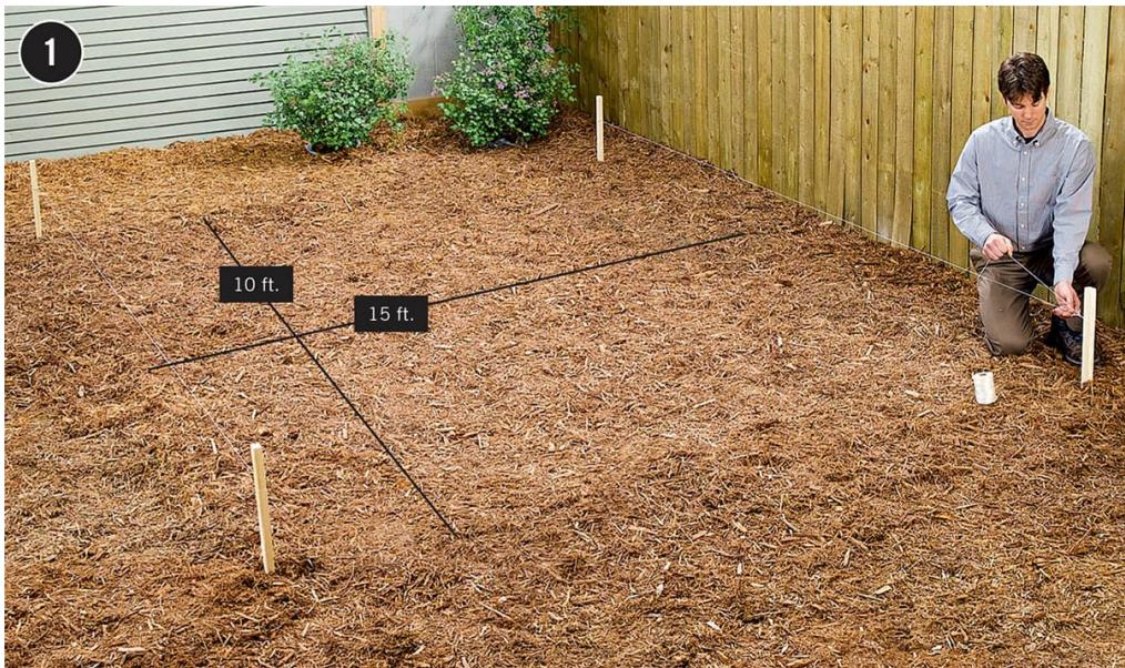
**Lay out the installation area**, using stakes and mason's string. Stake the four corners to create a rectangle that is 10' wide and 15' long. To make sure the layout is square (the strings are perpendicular), measure diagonally between opposing corner stakes: when the measurements are equal, the layout is square.
