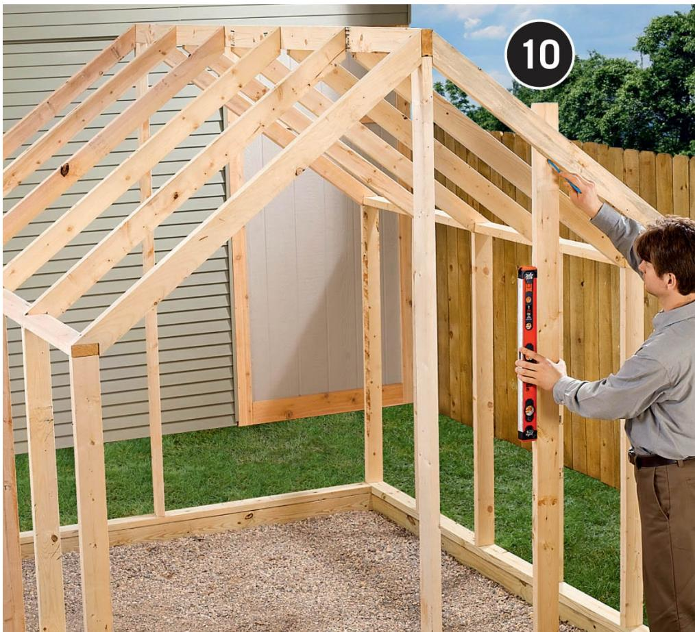
**Mark the two door frame studs** by holding them plumb and tracing along the bottom edge of the rafter above. Position the studs on-the-flat, so the inside edge of each is 16" from the center of the support post (for a 32"-wide door, as shown). Install the studs with angled screws. Cut and install two studs on the rear endwall, spacing them evenly between the kneewalls and support post.
