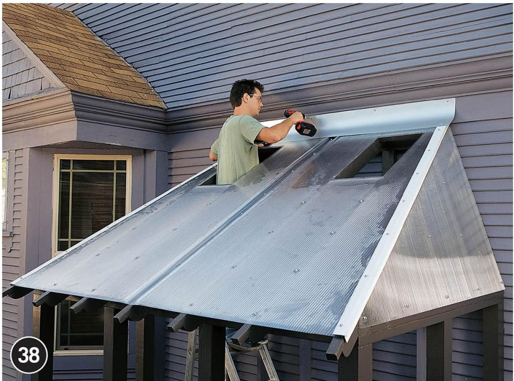
**Cover the gap** between the standalone greenhouse structure and the house with metal flashing. Aluminum handy flashing (12" width) can be fastened to the house and lightly creased so it extends over the gap and forms a seal without any physical connection to the greenhouse.
