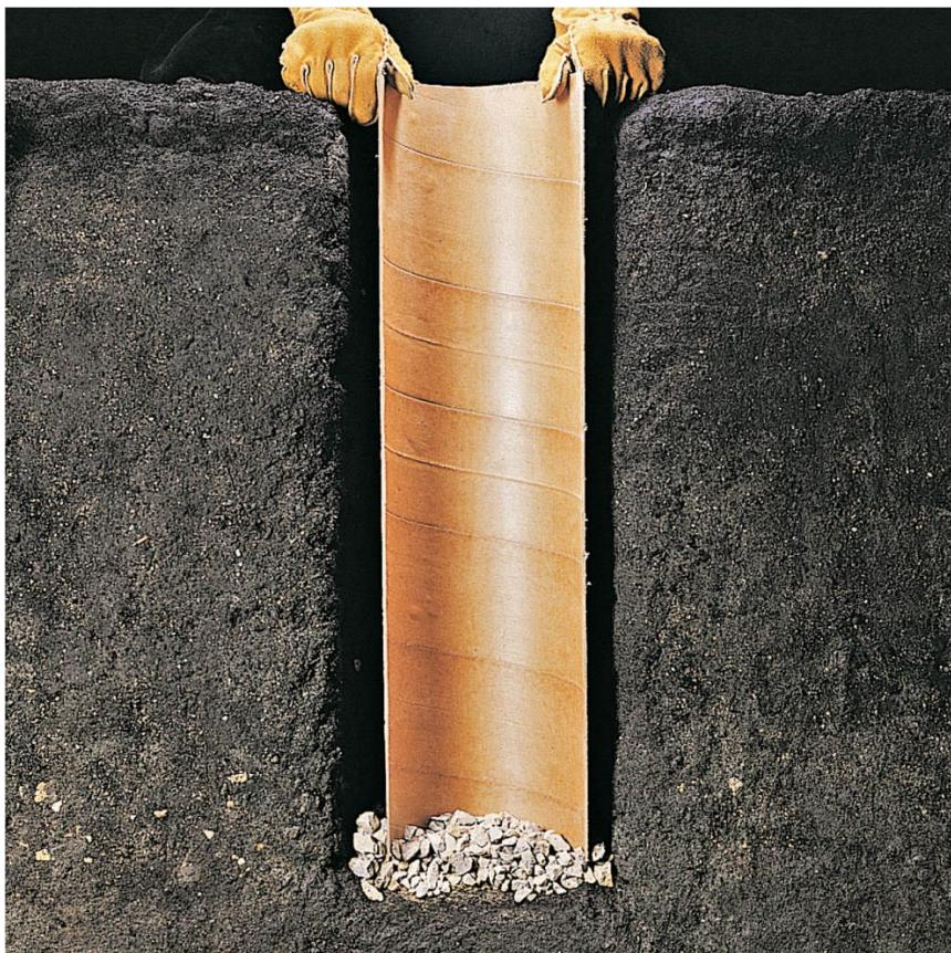
**Pier footings** are structural concrete columns poured in tube forms set below the frost line—the same foundation used to support deck posts. Pier foundations are appropriate for some kit and custom greenhouses and are often used on large commercial hoop-style houses. Anchor bolts embedded in the wet concrete provide fastening points for the greenhouse base or wall members.
