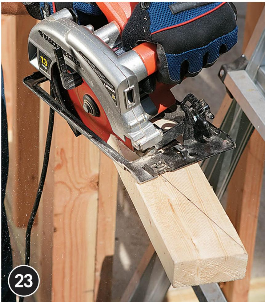
**Clamp the side rafter workpieces** to a sturdy worksurface and cut the top and bottom angles with a circular saw or jigsaw. The side rafters in this design do not overhang the wall headers. Attach the side rafters with screws driven through pilot holes.
