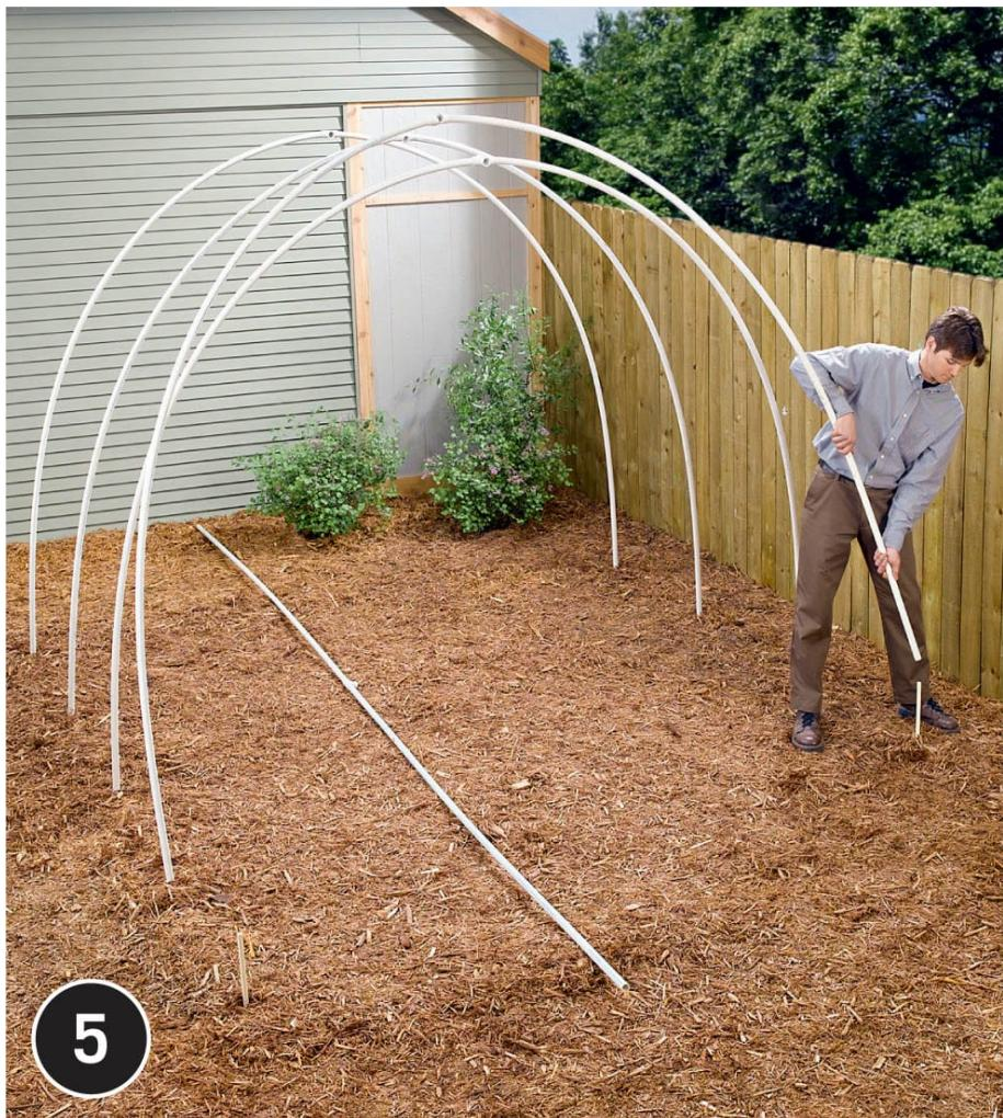
**Continue adding hoop frames** until you reach the other end of the structure. Wait until all the hoop frames are in place before you begin installing the ridge poles. Make sure the cross fittings on the intermediate hoop frames are aligned correctly to accept the ridge poles.
