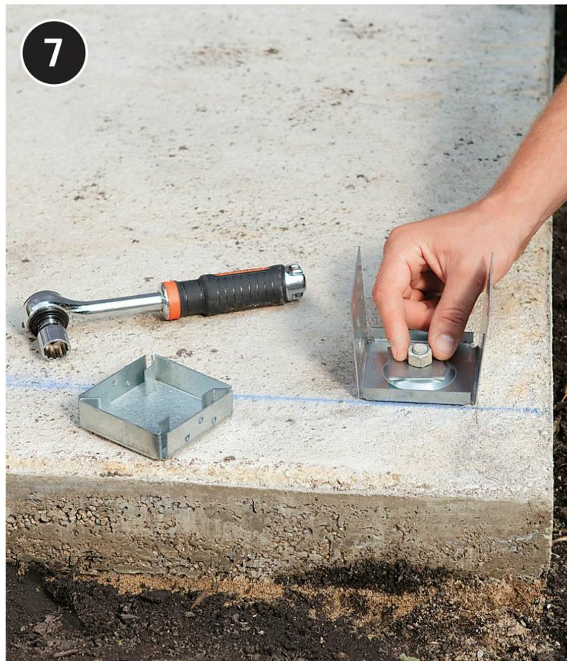
**Install post anchors** at the corners and at the doorjamb location. Standoff posts that elevate the post bottom slightly will greatly reduce the amount of water the post end will wick up from the footing.
