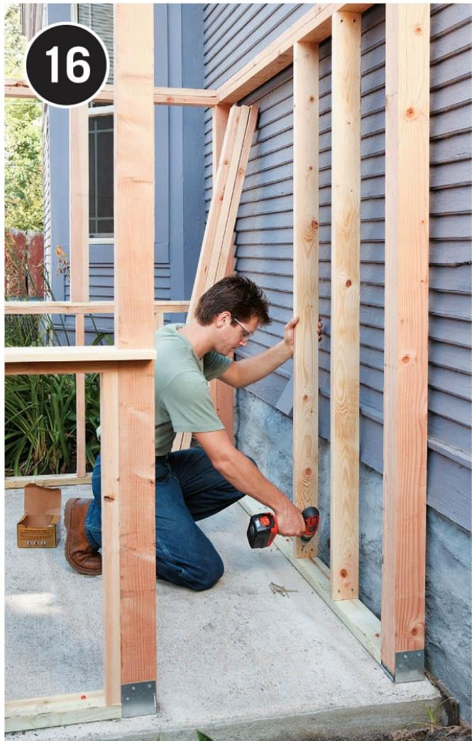
**Install back wall studs** between the back sill plate and the back cap plates, spaced 16" on center. Do not attach these studs to the house—they must remain isolated from it structurally.
