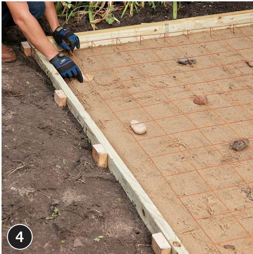
**Add reinforcement in the concrete area.** For most DIYers, metal re-mesh is an easy reinforcement material to work with. It is sold in  $5 \times 50'$  rolls and in  $4 \times 8'$  sheets. Prop the re-mesh on some small stones or bolsters. The edges of the reinforcement should be at least 4 to 6" away from the sides, and no closer than 1" to the concrete surface.
