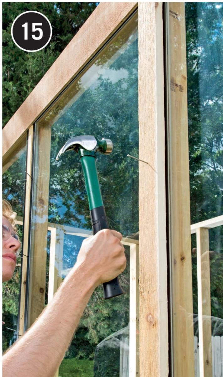
**Measure and cut 1 x 3 cedar strips** to run between the fascia at the top and the sill. Drill pilot holes and nail the strips in place on the studs with 3" 6d nails.
