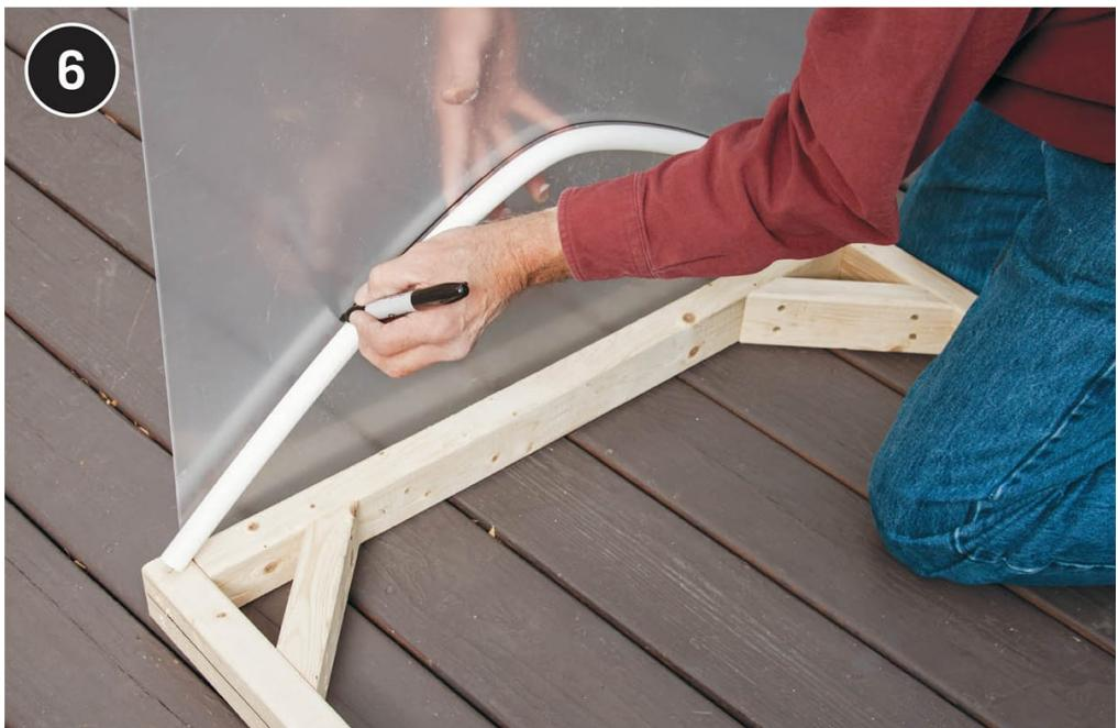
**Hold up and mark** a smooth piece of clear acrylic for the end panels. The clear acrylic should cover the  $2 \times 3$  and follow the curving top of the PVC. Cut the clear acrylic with a plastic-cutting jigsaw blade.
