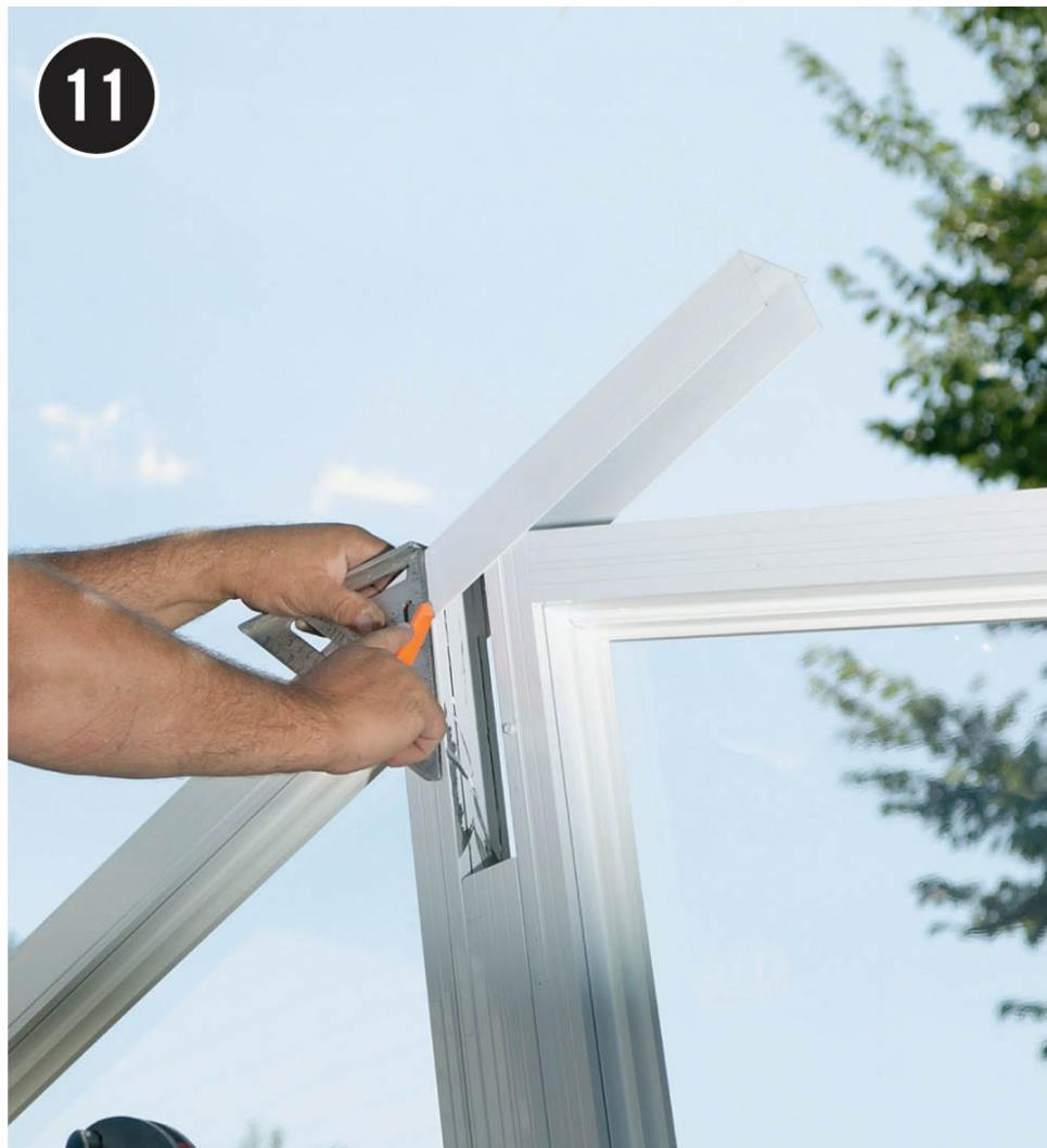
**Mark the upper wall tracks** at the gable for cutting by transferring the edges of the ridge pole saddle onto the ends of tracks. Cut them to length and the correct angle with a power miter saw and metal cutting blade. Or, you can use an old combination blade that you don't mind making dull.
