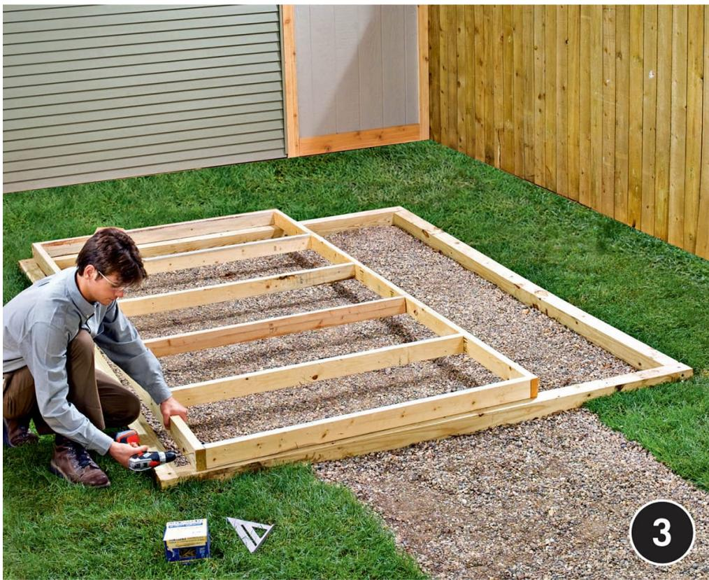
**Cut the sole plates, caps, and studs** for the two kneewalls. Mark the stud layouts onto the plates and caps, spacing the studs at 24" on center. Assemble each kneewall by driving 3" deck screws through the sole plates and caps and into the ends of the studs.
