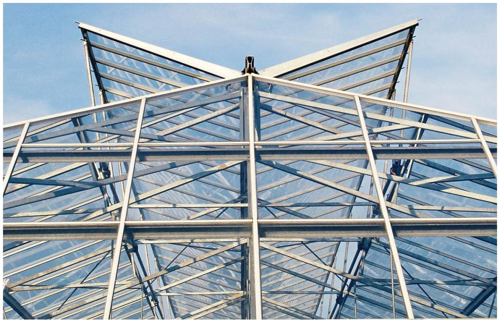
**Roof vents** that are triggered to open automatically by sensor alerts are far and away the most important component of a greenhouse cooling system. But additional cooling devices may be necessary.
