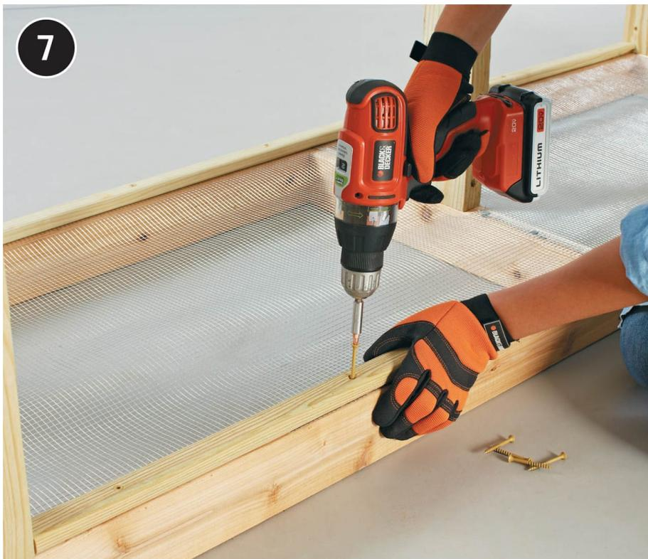
**Predrill the 1 x 2s** every 8 to 10". Flip the tray over then screw the 1 x 2s to the bottom of the tray, flush with the outside edges and covering the hardware cloth.
