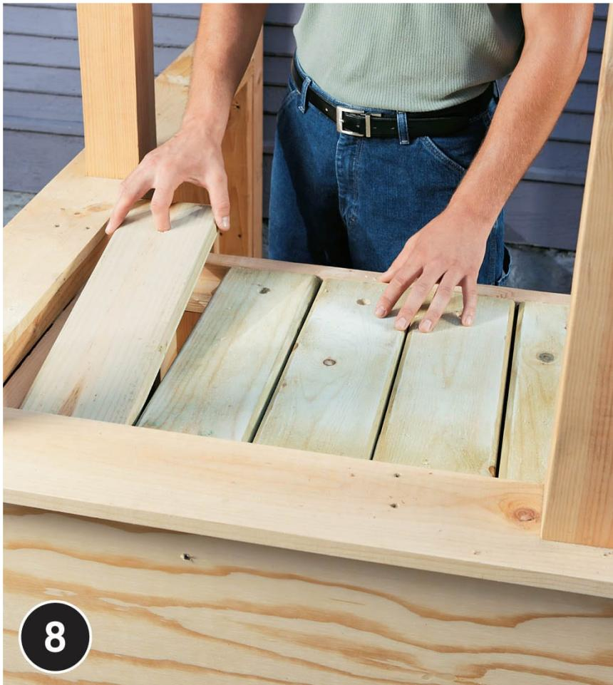
**Cut the benchtop slats** from treated or cedar decking (or composite if you prefer). Attach the slats over the first two bays by driving a pair of deck screws into each slat end and the cleat below. Do not fasten the deckboards over the right end bay. Drill 1" finger holes near the end of each board and simply set them on the cleats so they can be removed to access the shelf below. If you wish, finish the bench with stain, sealant, or paint.
