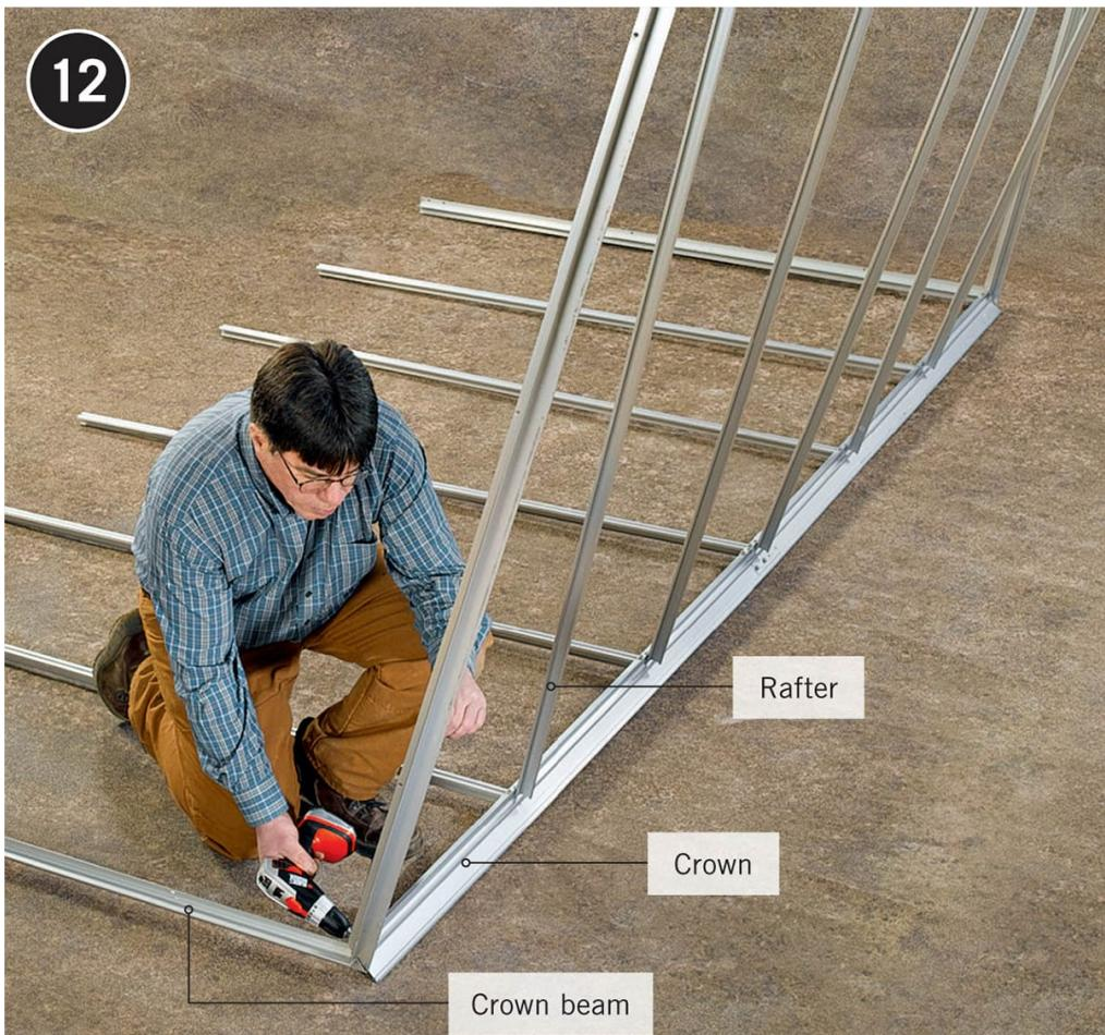
**Assemble the roof frame** on a flat area near the wall assembly. First assemble the crown-beam pieces; then attach the rafters to the crown, one by one. The end rafters, called the crown beams, have a different configuration, so make sure not to confuse them.
