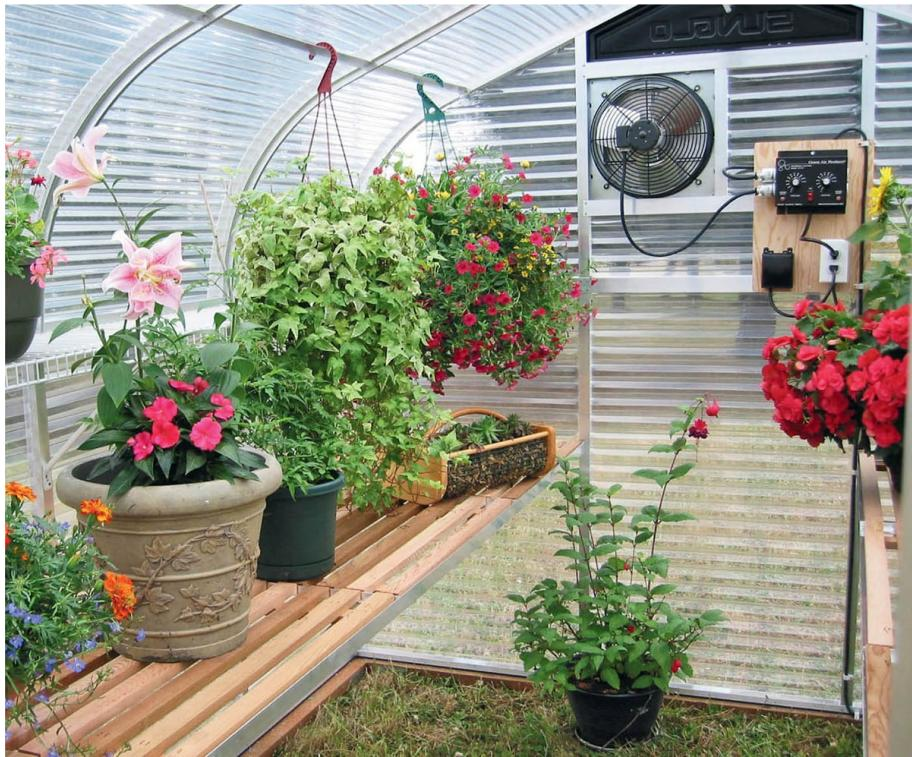
**A vent fan like this one** can be attached to a controller that opens the shutters and turns on the fan at precise levels of humidity or temperature, or on a timer. This actively ventilates the greenhouse, as opposed to the passive ventilation of a roof vent.
