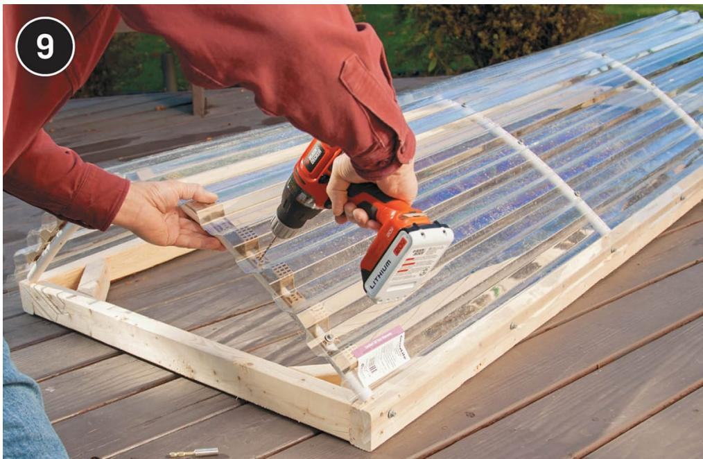
**Lap the second sheet over the first,** leaving roughly the same amount of panel hanging over the  $2 \times 3$ . Fasten the second sheet the same way as the first. Insert filler strips at each end under the polycarbonate, then drill through those into the PVC ribs. Now add additional screws about every  $1/6$ “. You can just predrill the holes with the  $1/8$ “ bit (the polycarbonate panels are soft enough that the screws will drive through them without cracking).
