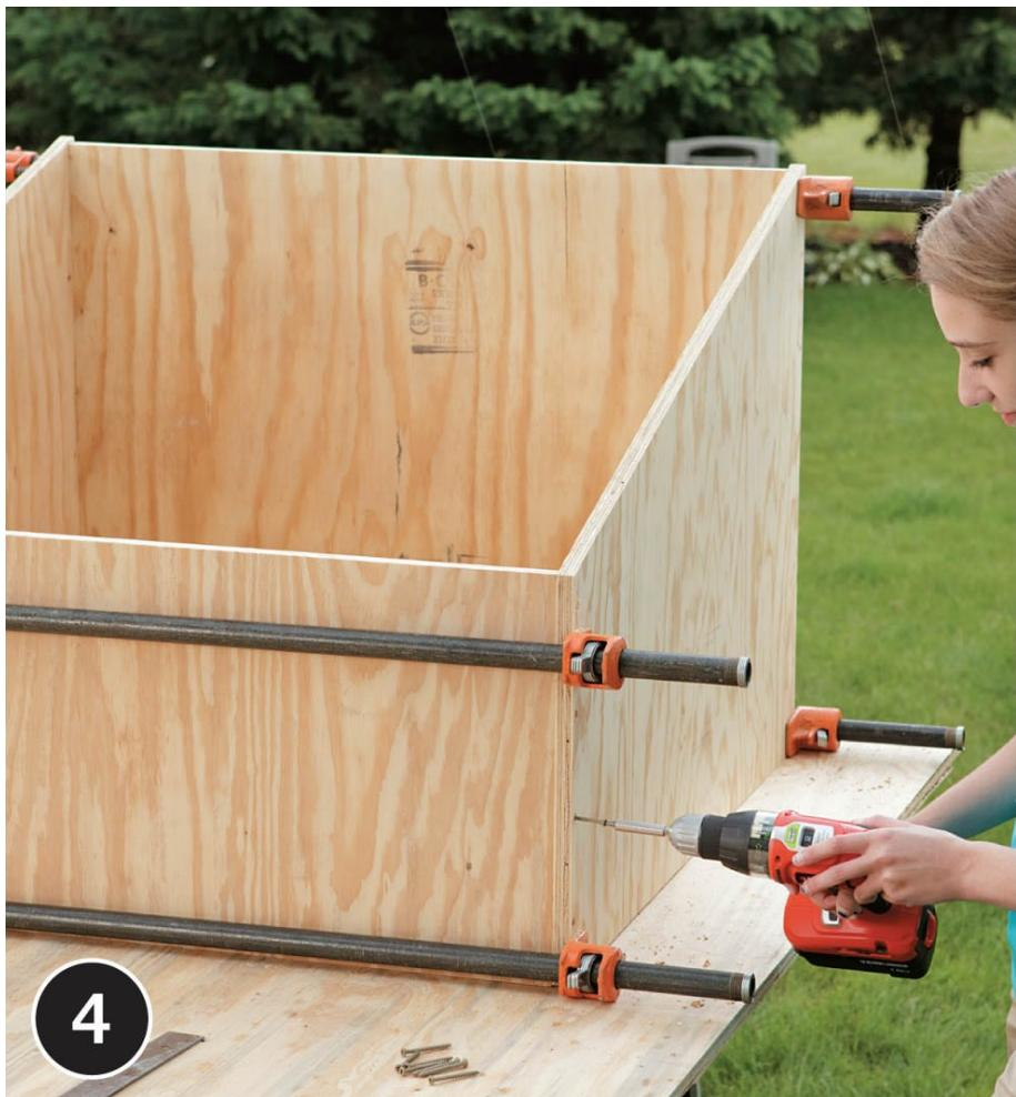
**Reinforce the joints** with 2 or 2½" deck screws driven through countersunk pilot holes. Drive screws every 4 to 6" along each joint.
