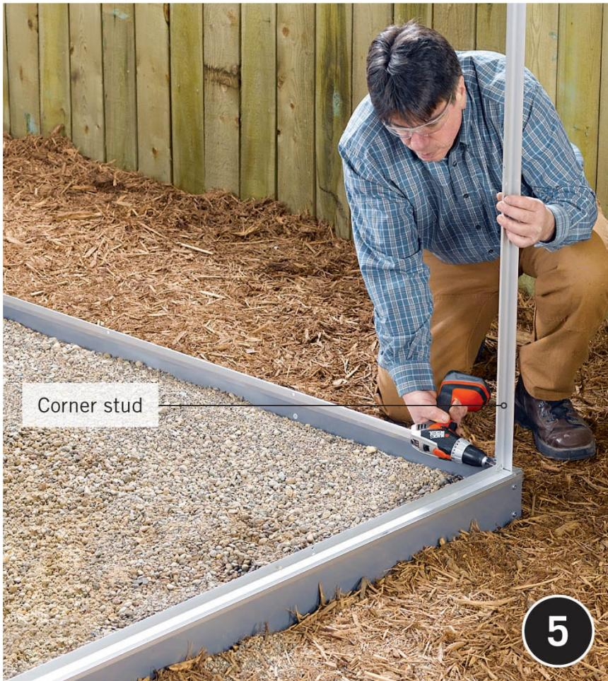
**Fasten the four corner studs** to the bottom wall plates, using hold-down connectors and bolts. In this system, each corner stud is secured with two connectors.
