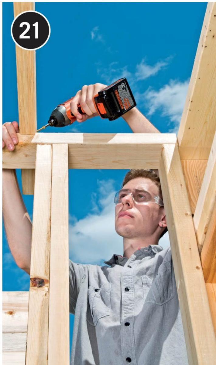
**Measure and cut the 2 x 4 rafters** and toe-screw them running front wall to back wall. There should be a 6" overhang on both ends.
