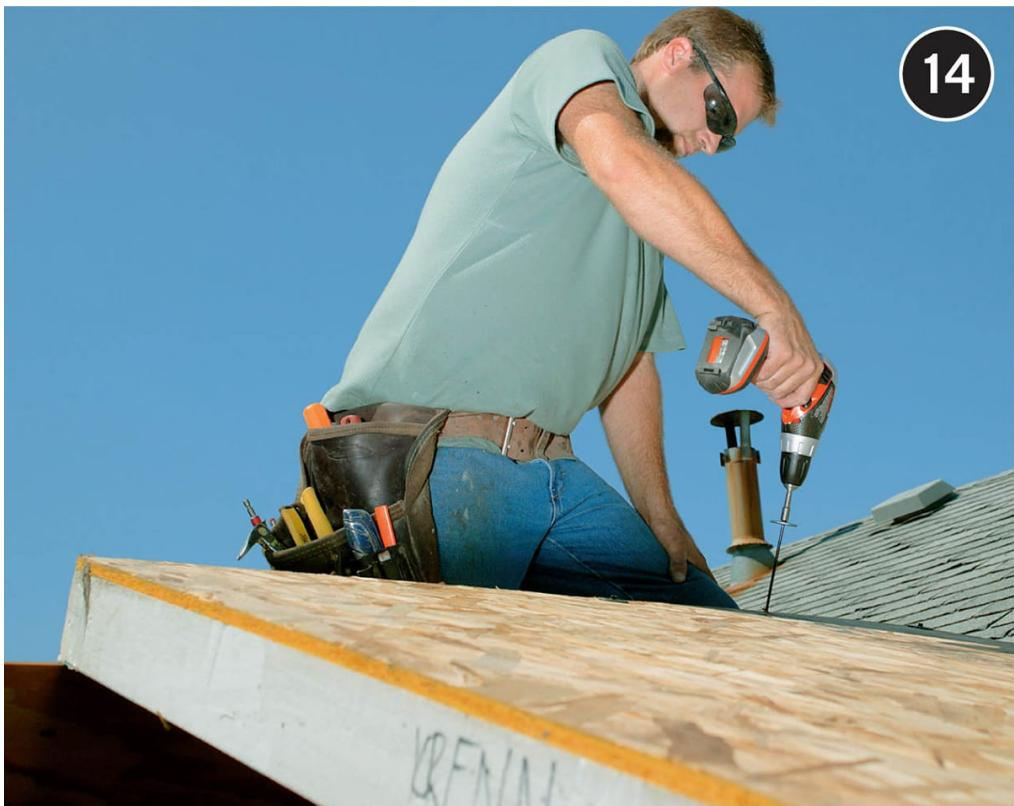
**Begin installing roof panels.** The full-width panels seen here are 4' wide, yet they are strong enough to meet minimum dead load ("snow") requirements even in cold climates. The panels are attached with long insulation screws that are fitted with fender washers and driven into the ridge pole and upper wall track.
