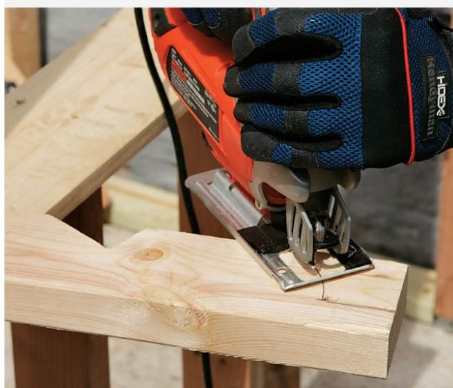
**Cut the rafters.** Set workpieces in position against the  $2 \times 6$  ridge pole and mark the point where they meet the header. Make a birdsmouth cutout in each rafter so it will rest flush on the header (top photo). Cut a decorative profile on each rafter end according to the diagram on [this page](#) (bottom photo).
