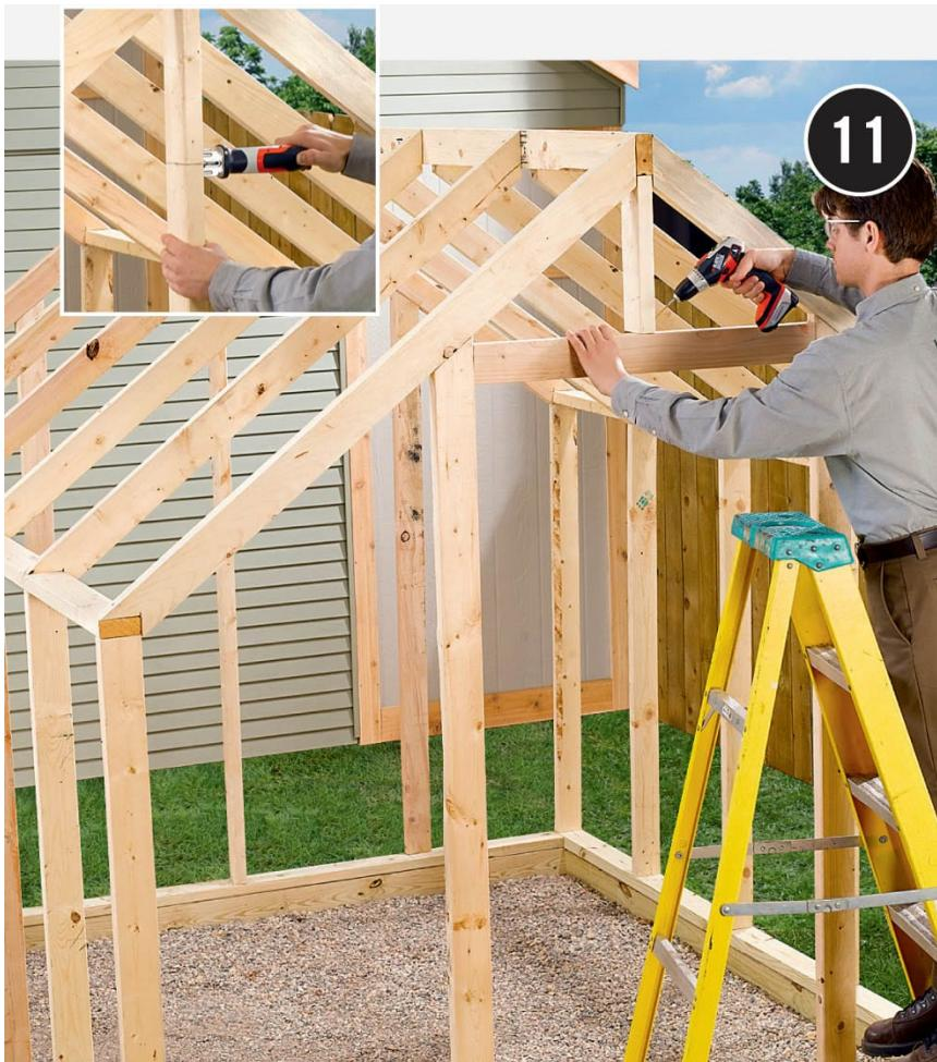
**Complete the door frame:** Mark the front support post 78" (or as desired) up from the sole plate. Make a square cut at the mark, using a circular saw or cordless trim saw (inset), then remove the bottom portion of the post. Cut the door header (from the post waste) to fit between the door studs. Fasten the header to the door studs and remaining post piece with screws.
