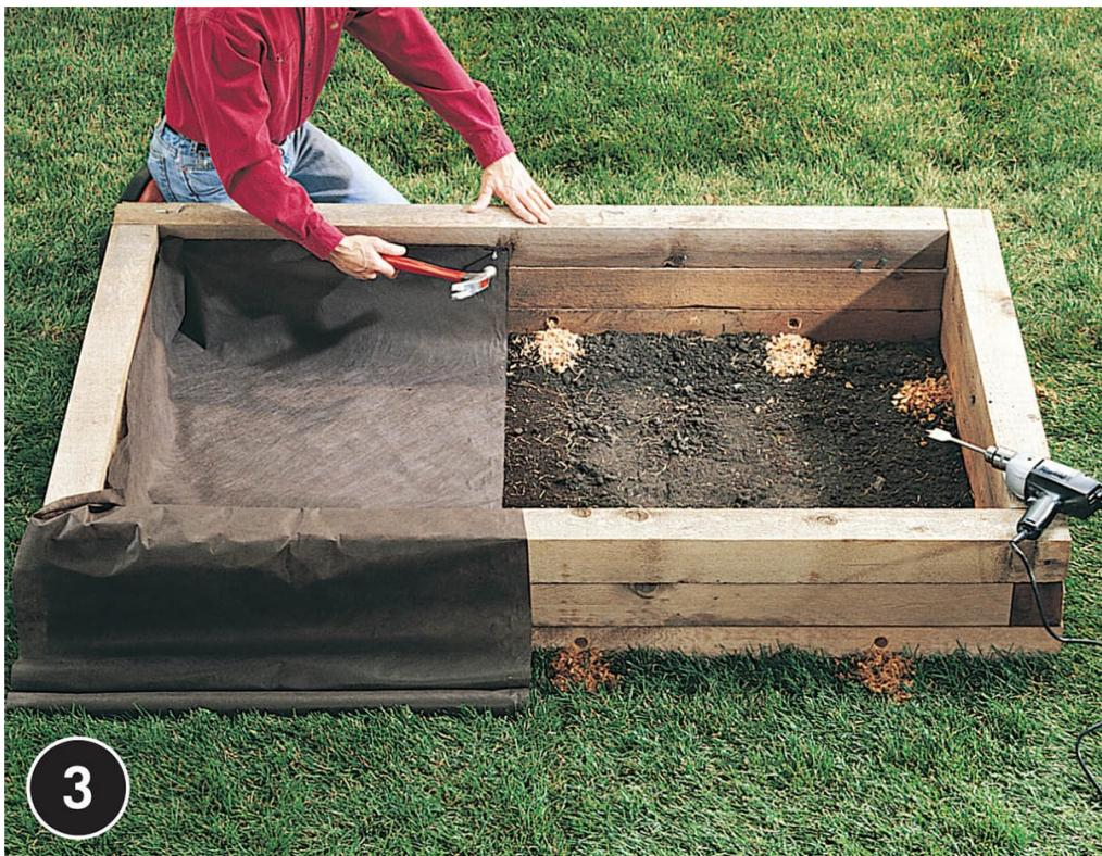
**Line the bed with landscape fabric** to contain the soil and help keep weeds out of the bed. Tack the fabric to the lower part of the top course with roofing nails. Some gardeners recommend drilling 1"-diameter weep holes in the bottom timber course at 2' intervals. Fill with a blend of soil, peat moss and fertilizer (if desired) to within 2 or 3" of the top.
