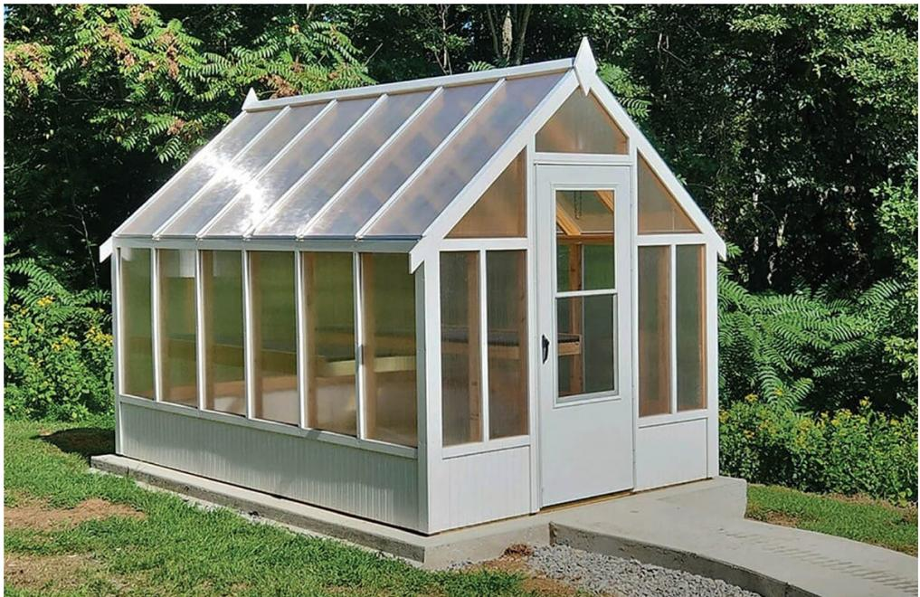
**Commit to concrete.** A concrete slab is perhaps the most stable and permanent of foundations. It creates a grounded look and a stage for a handsome greenhouse like the wood model here. A concrete pathway, poured at the same time as the slab, makes for easy access and a complementary visual. Over time, the gardener can fill in around the slab and walkway with potted plants to soften the look.
