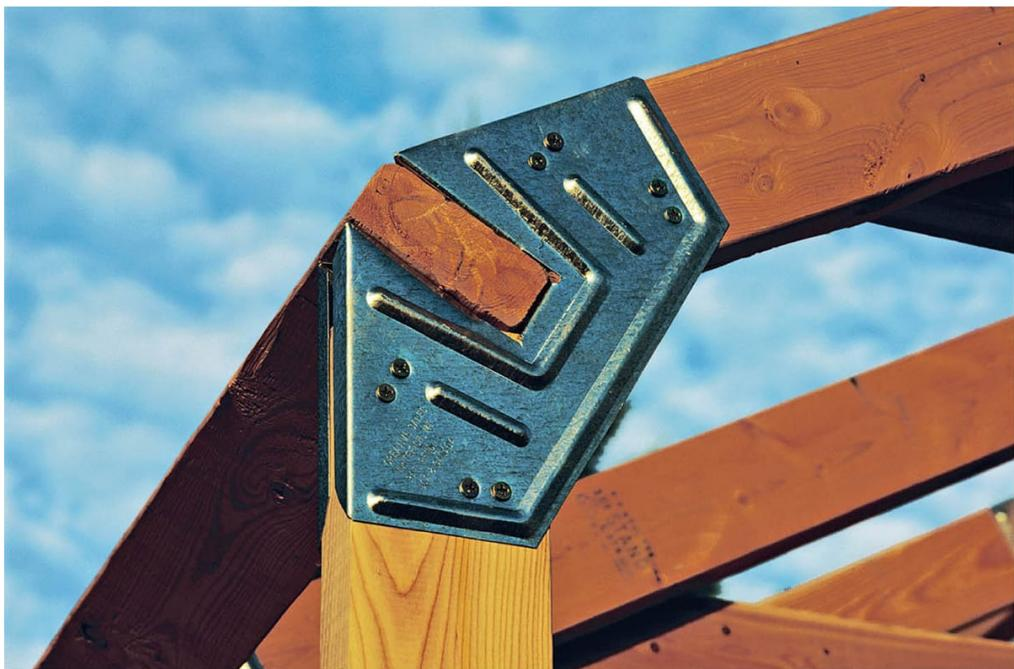
**Seek details** that aid construction—modern greenhouse manufacturers offer many construction shortcuts that make building your greenhouse easier. This framing connector alleviates the need for multiple miter cuts, shaving quite a bit of time off the construction process.
