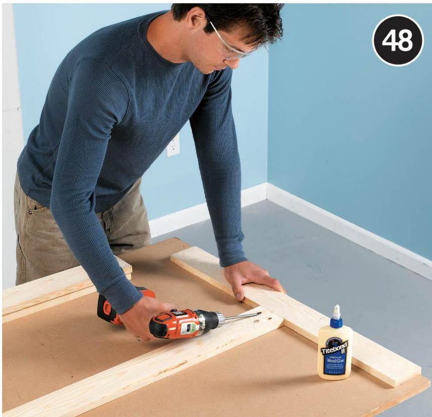
**Assemble the door frame.** The center stiles should be attached to the frame rails with pocket screws or with deck screws driven toenail style. Clamp the parts together, sandwiching a piece of  $\frac{1}{4}$ " polycarbonate between the frames.
