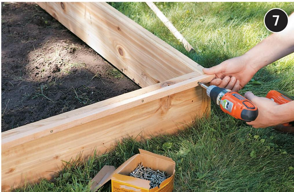
**Install the cleats:** Rip a 1 × 4 into four  $\frac{3}{4}$ "-wide strips, using a circular saw or table saw (it's okay if the last strip isn't exactly  $\frac{3}{4}$ "). Fasten the strips along the perimeter of the bed frame, flush with the top edges, using  $1\frac{1}{4}$ " deck screws driven through pilot holes. Cut the strips to length as needed to complete each run. Fill the bed with soil and compost, as desired.
