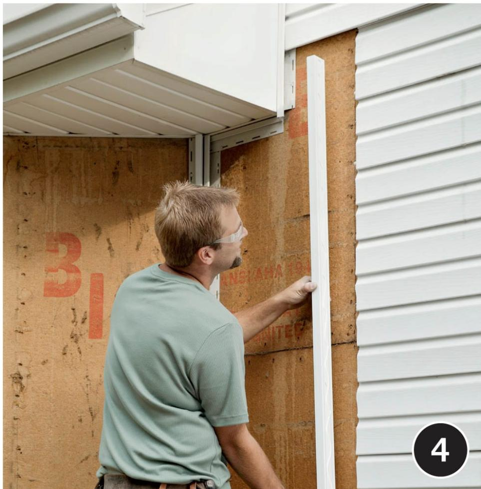
**Install the vertical wall track channels** with silicone sealant and self-sealing screws. If the wall sheathing will not accept screws and is not backed by plywood sheathing, you will need to install sturdy wood or wood sheathing backers to secure the track.
