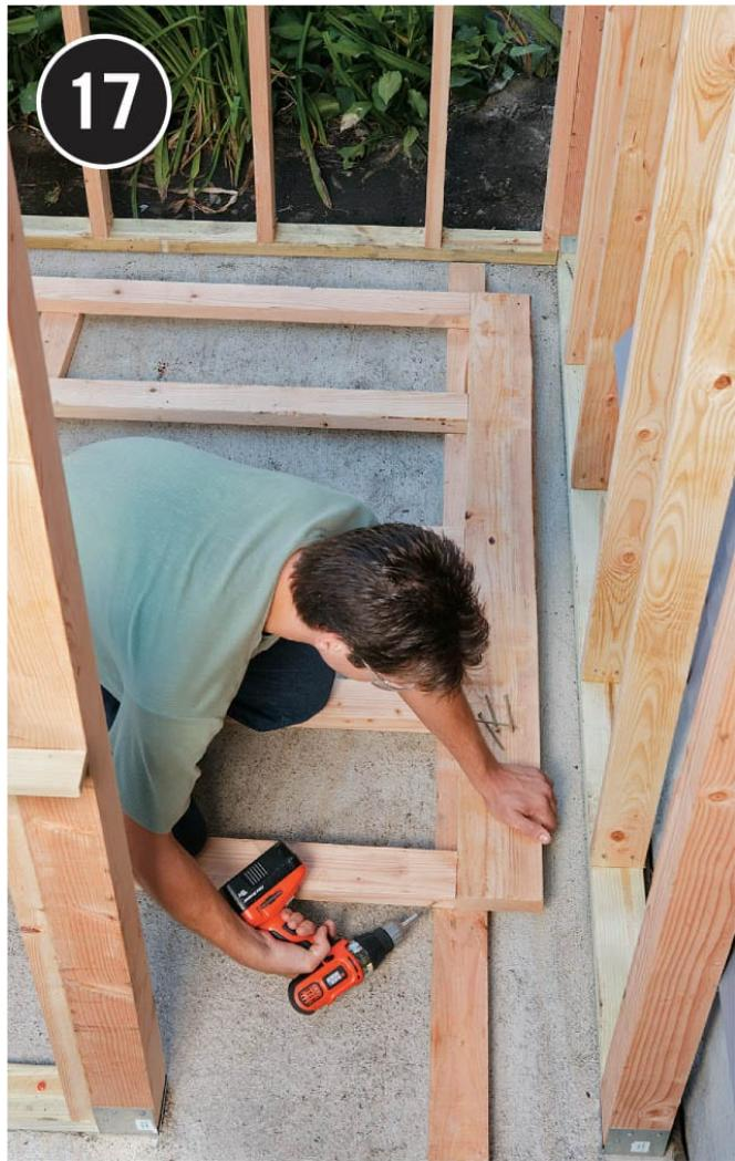
**Construct and attach** the roof ridge support wall, featuring a  $2 \times 6$  on edge at the top of the wall. It is easiest to build this wall on the ground and then erect it as a unit. Use a pair of  $2 \times 4$  braces to keep the support wall stable while you attach the rafters.
