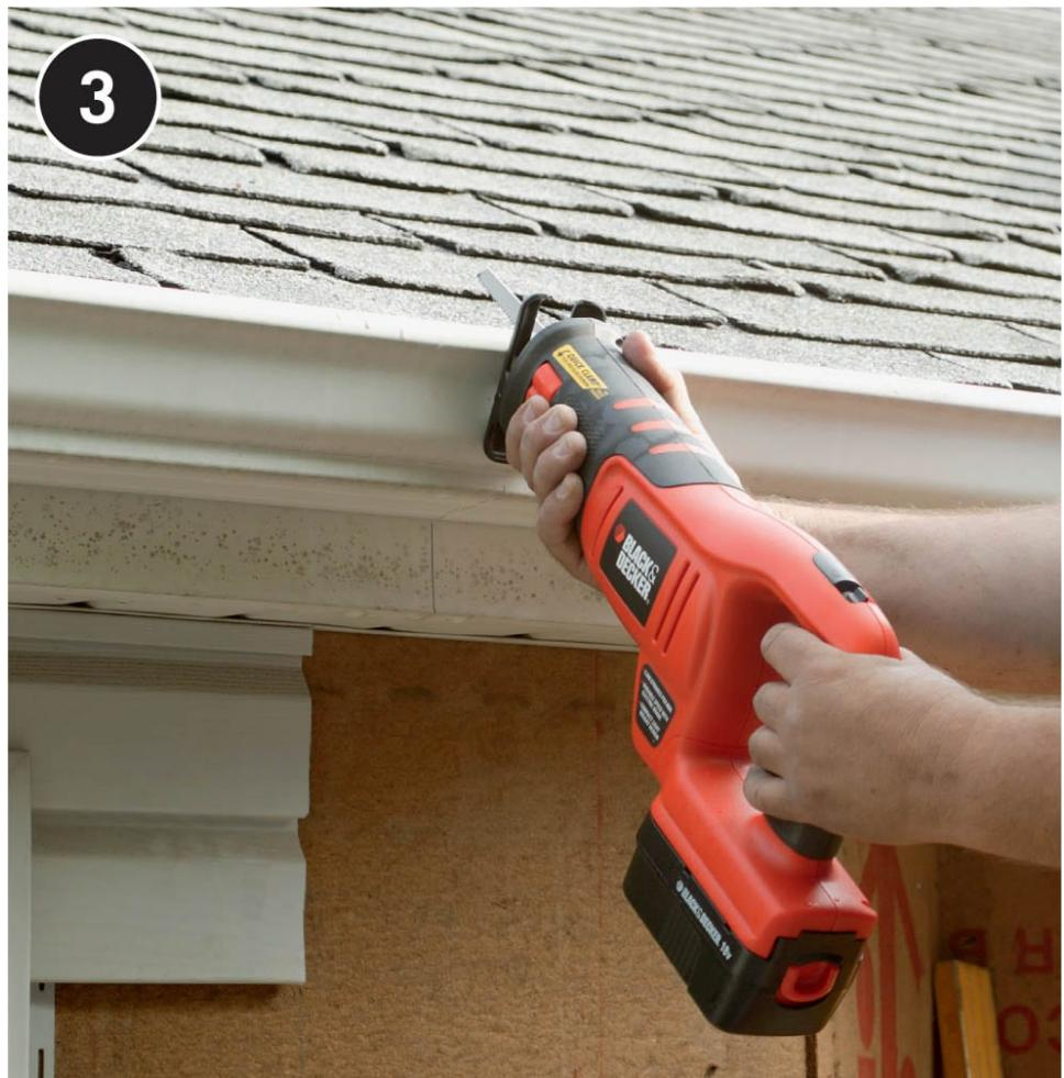
**Remove gutters and other obstructions** from the installation area. The exact requirements for this step depend on the configuration of your roof and how you will be tying into the roofline or wall to make space for the sunroom roof.
