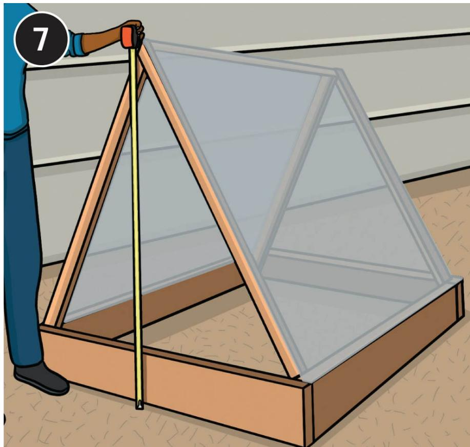
**Set the frame in place.** Measure the triangle opening on one side. Add 2" all around, transfer the measurements to the plastic sheet, and cut the triangle for the tent ends. Repeat with the opposite side.
