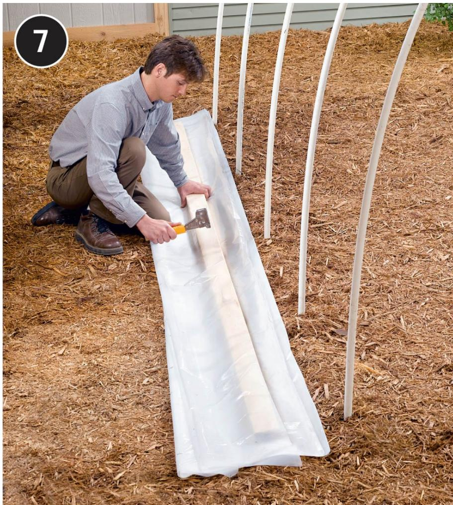
**Cut four 2 × 4s to length** (15' as shown). Cut the cover material to length at 16' (or as needed so it is several inches longer than the house at both ends). Staple one edge of the cover to one of the 2 × 4s, keeping the material taut and flat as you work from one end to the other
