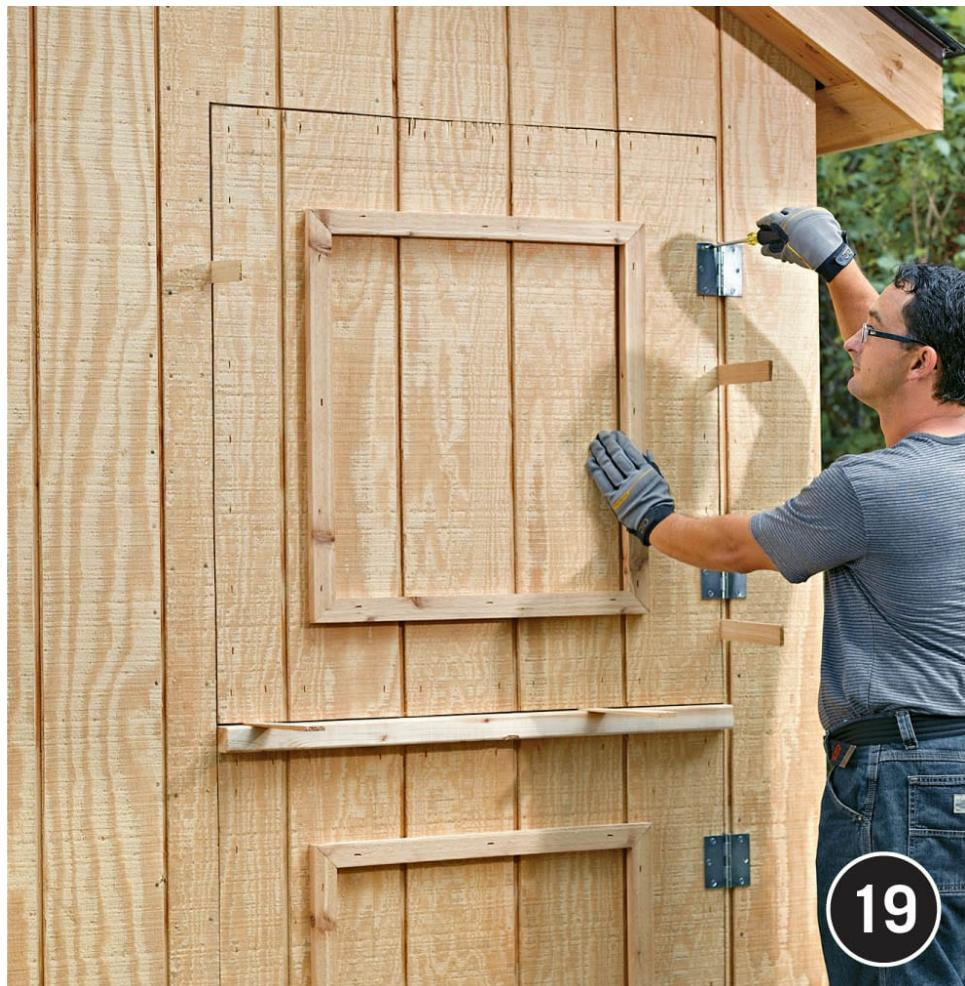
**Build each of the two door panels** using T1-11 siding,  $2 \times 2$  bracing, a  $2 \times 4$  bottom rail, and  $1 \times 2$  trim on the front side; see the DOOR CONSTRUCTION drawings ([here](#)). The panels are identical except for a  $2 \times 4$  sill added to the top of the lower panel. Install  $1 \times 2$  stops at the sides and top of the door opening. Hang the doors with four hinges, leaving even gaps all around. Install a bolt latch for locking the two panels together.
