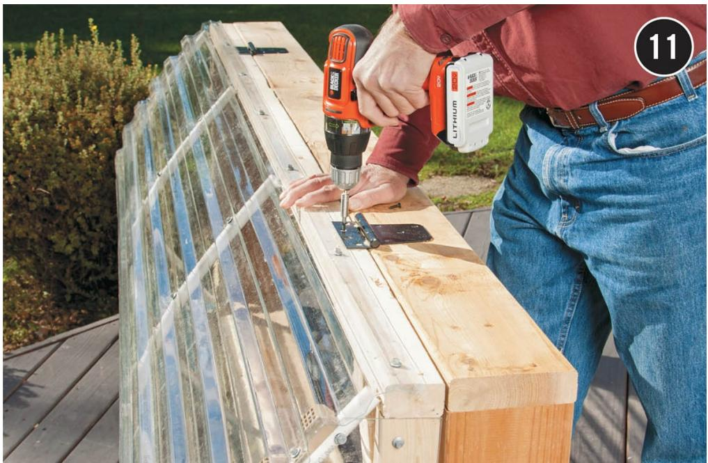
**Mount the canopy to the cold frame base** with two exterior hinges. The canopy frame should fit flush over the base on all sides. Screw in two hook-and-eye latches in front.
