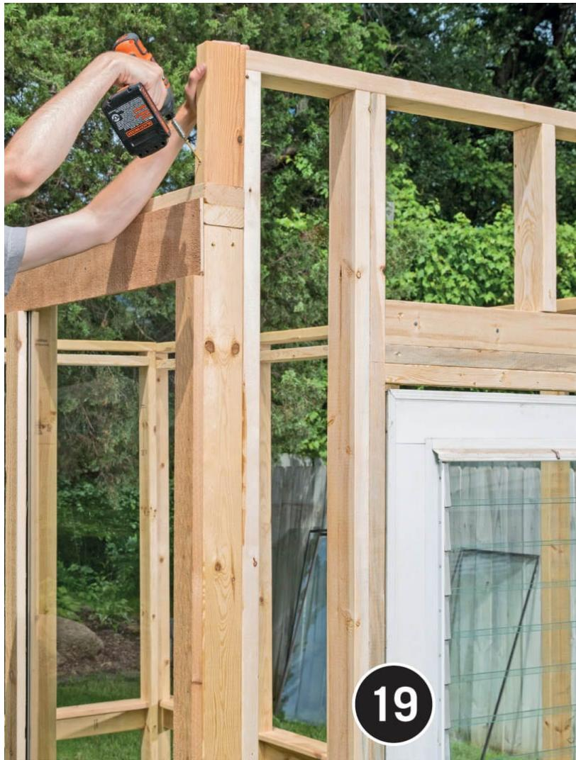
**Use 2½" deck screws** to toe-screw the front cripple studs for the triangular top walls on both sides.
