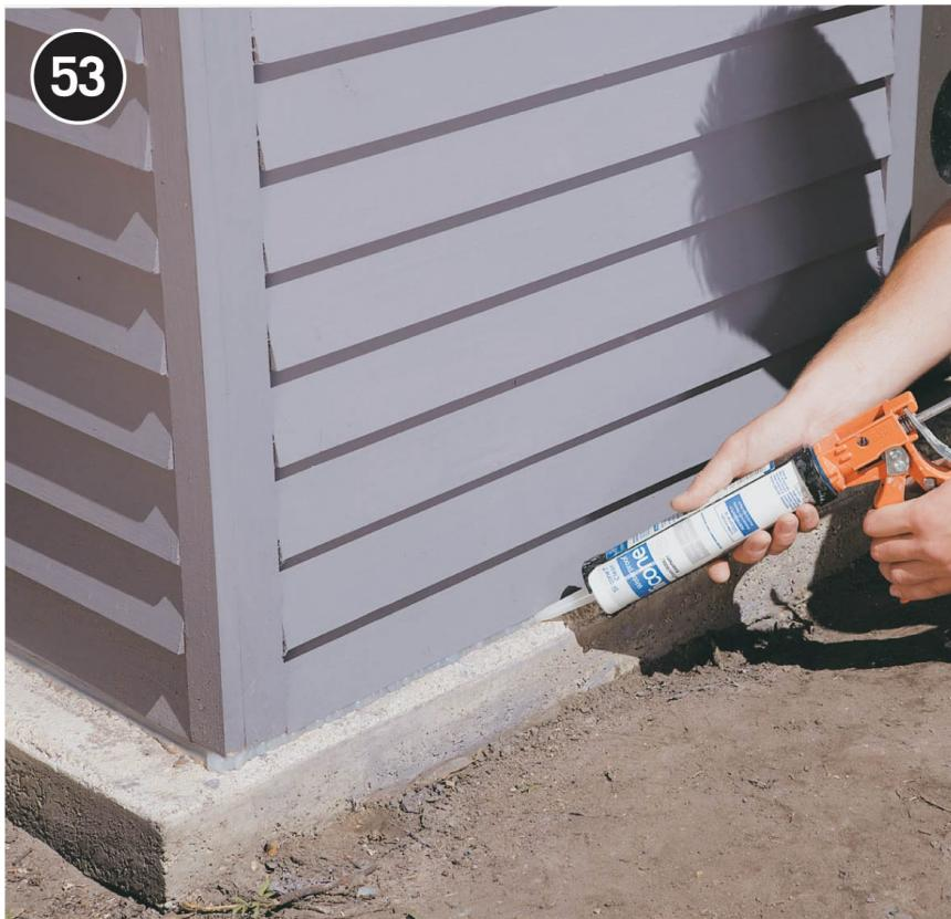
**Make sure the foundation is clean and dry, then fill the gap between the concrete and the siding with clear silicone caulk.**
