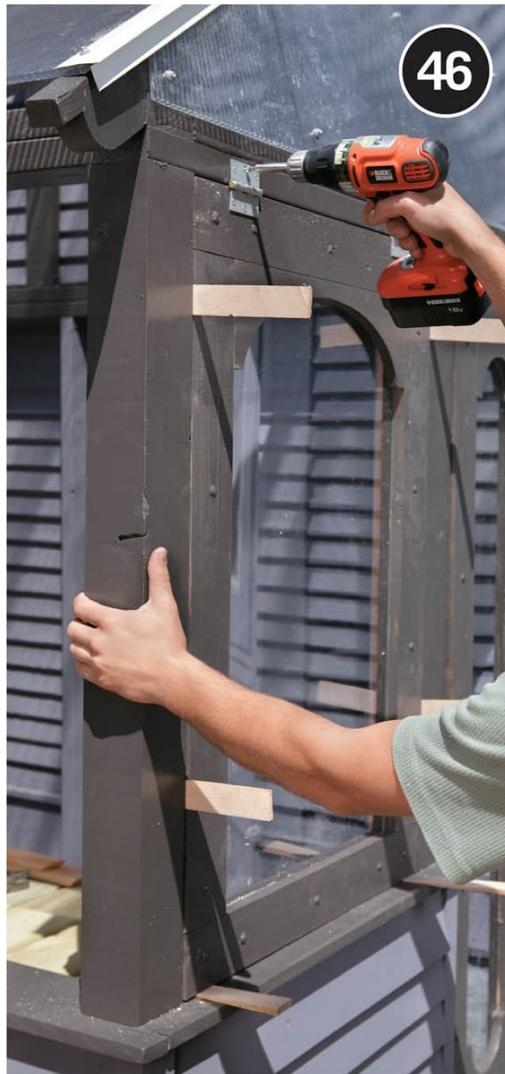
**Install operable windows** by centering the window unit in the opening, using shims to center it side-to-side and top-to-bottom. Hang the windows with exterior-rated pairs of butt hinges.
