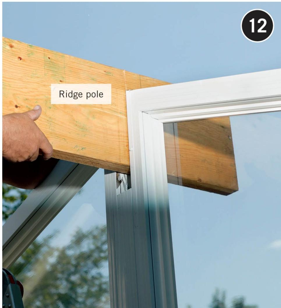
**Set the ridge pole into the saddle** in the ridge pole post, and adjust it until the overhang is correct. Check the length: if the pole does not end at the correct point on the other end, recut it or adjust your overhang amount. Secure the end by driving screws through the ridge pole post and into the ridge pole.
