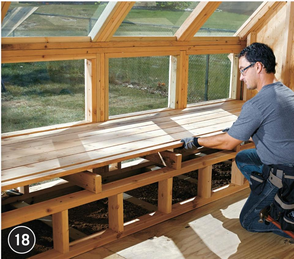
**Construct the planting tables** from  $2 \times 4$  lumber and  $1 \times 6$  boards, as shown in the TABLE + LOWER WINDOW DETAIL and BUILDING SECTION. The bottom plates of the table legs should be flush with the outside edges of the foundation blocking.
