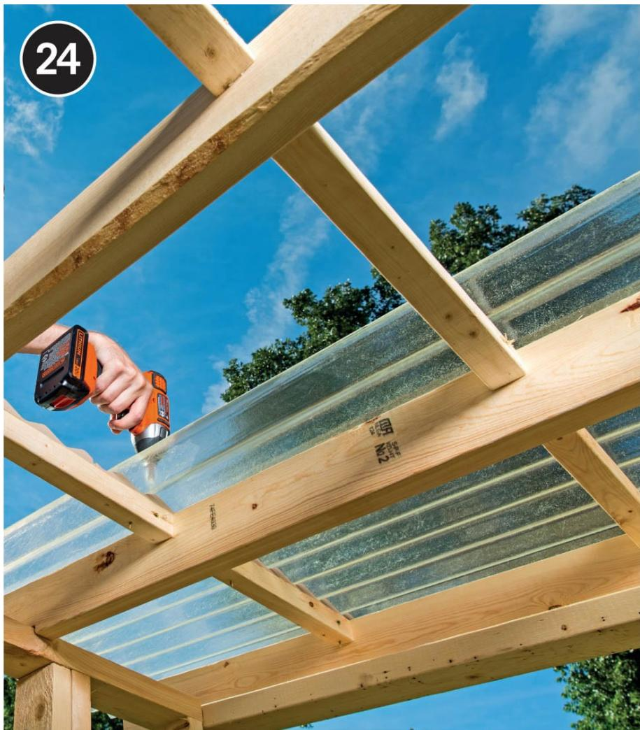
**Drill pilot holes** for the fiberglass panels and screw them in place to the purlins using 1" screws and rubber washers. Paint or stain the exterior of the greenhouse and, if using in a cooler season, cover all the clerestory windows with 6- to 8-mil plastic sheeting stapled in place.
