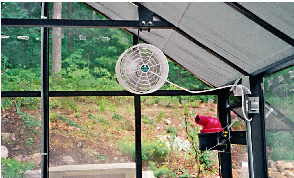
**Roof shades**, along with vents, help prevent a greenhouse from overheating in direct sunlight. Here, a combination of circulating fans and cloth shades mounted on the interior of the south-facing glass helps protect plants.
