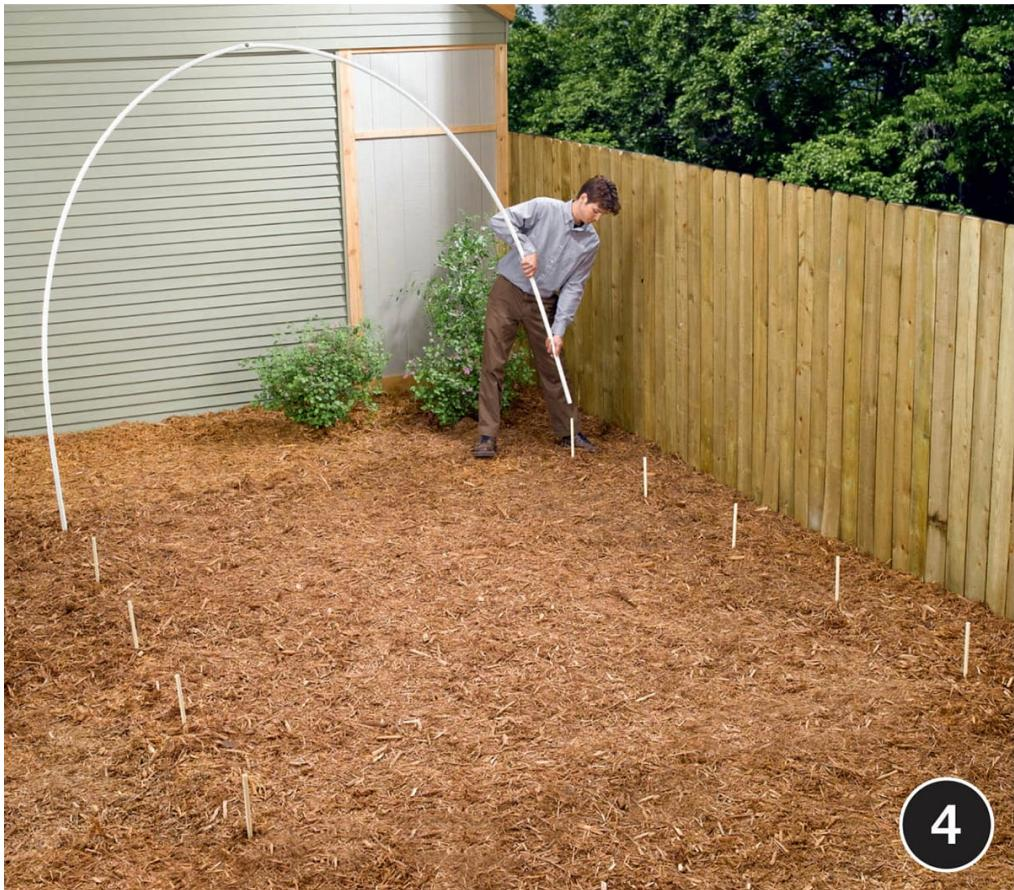
**Slip the open end** of one hoop-frame leg over a corner stake so the pipe is flush against the ground. Then bend the pipes so you can fit the other leg end over the stake at the opposite corner. If you experience problems with the pipes pulling out of the top fitting, simply tape the joints temporarily until the frame is completed.
