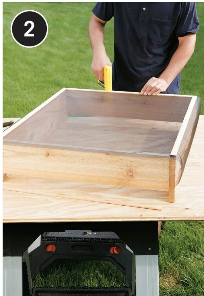
**Install the mesh.** Staple the screen to the frame. Then tack the retainer strips over the screen to the frame with 3 to 4 brad nails per side. Trim off the excess mesh.
