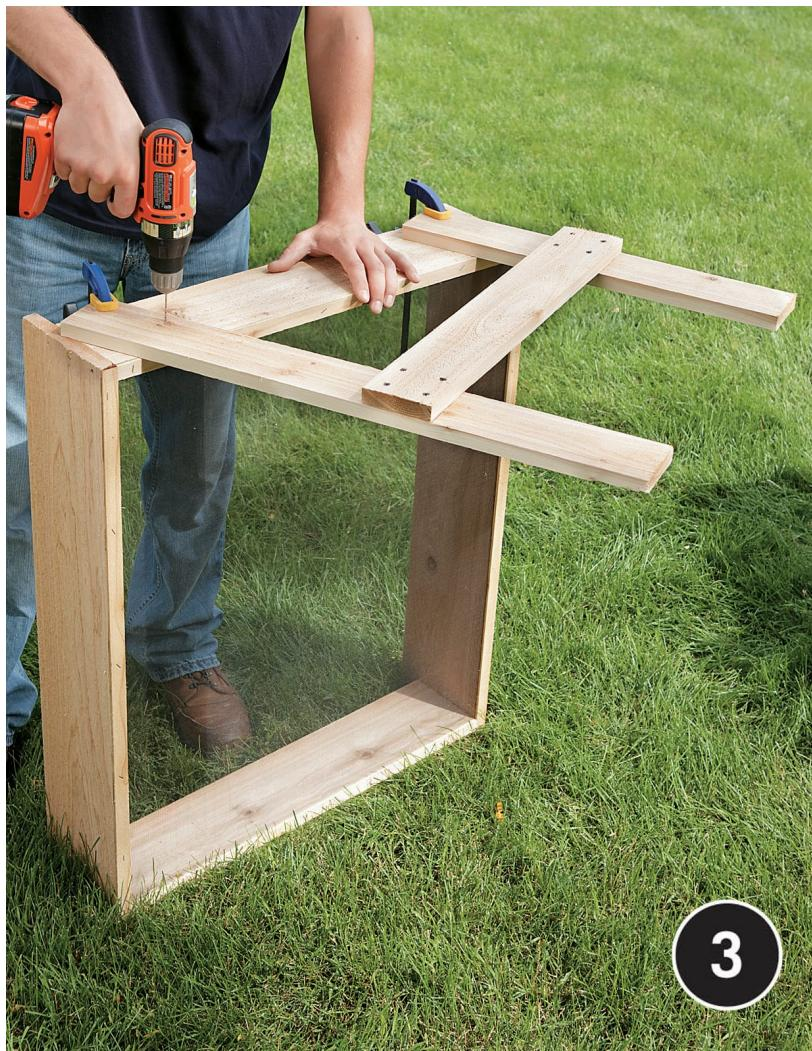
**Build the stand.** Attach each 24" board to a 30" board (in the back) and a 22" board (in the front) with 1½" deck screws. Then attach the finished posts to the frame with three 1½" deck screws in each post.
