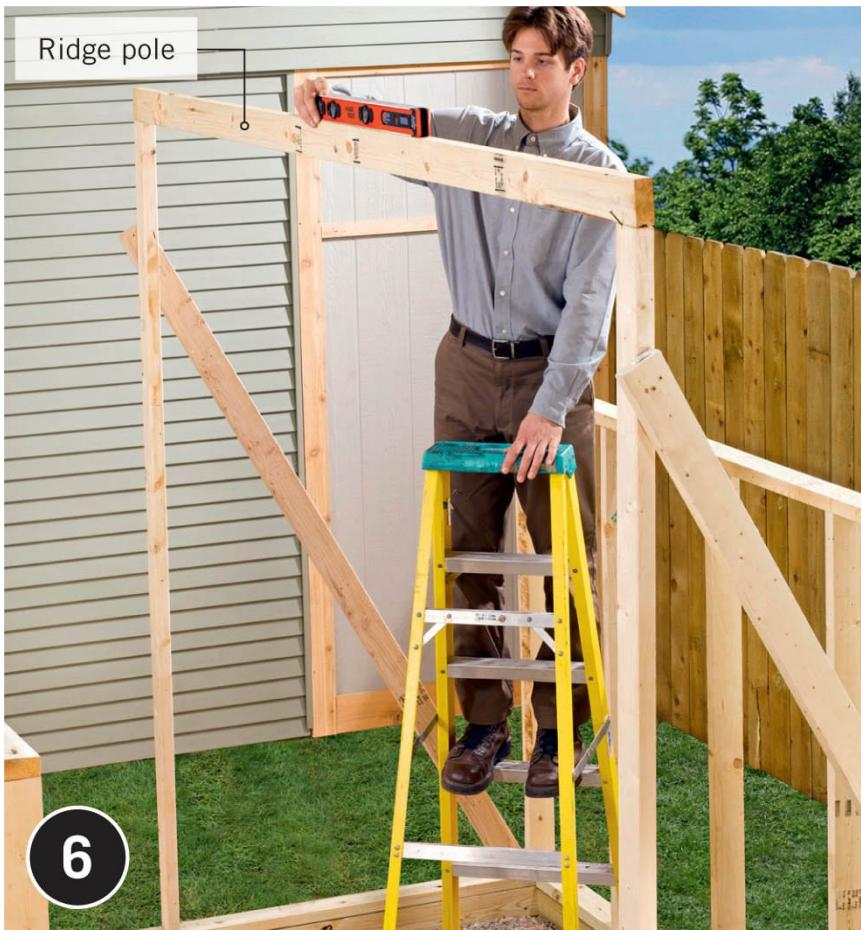
**Set the ridge pole on top of the support posts** and check it for level. Install temporary cross braces between the outer wall studs and each support post, making sure the posts are plumb before fastening the braces. Double-check the posts and ridge for plumb and level, respectively.
