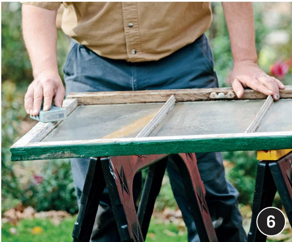
**Clean up the window,** sanding rough spots as necessary, and recaulking the window if needed. Prime and paint the window (paint it a darker color to absorb heat during the day and release it at night).
