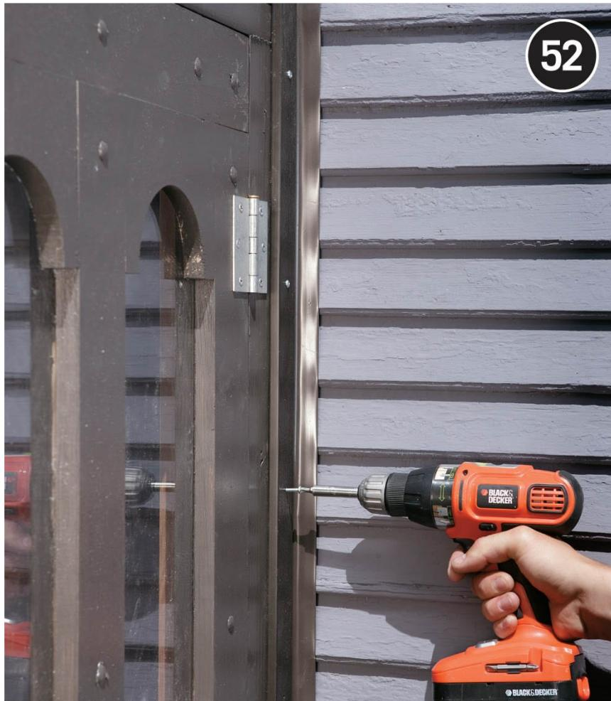
**Attach a garage door sweep** (or comparable weatherstripping product) to cover the gaps between the greenhouse and the house. Flashing, such as drip cap, may be used to cover the gaps on the downsloping sides of the hip roof.
