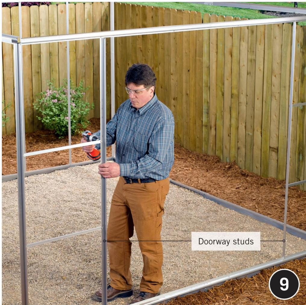
**Install the doorway studs** at either side of the greenhouse door on the front end of the building. Install the side studs along both side walls of the greenhouse.
