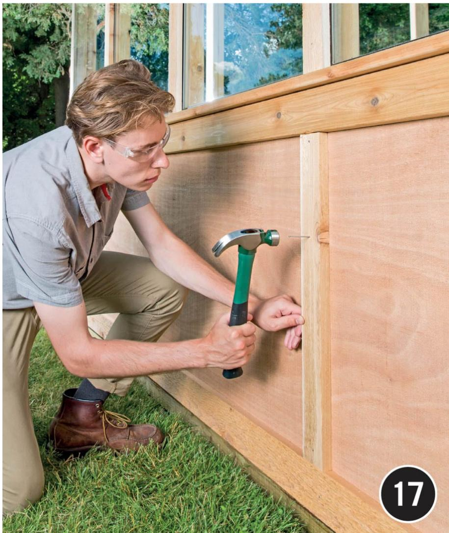
**Measure and cut 2 × 4 cedar base trim, 1 × 3 cedar corner boards, and 1 × 3 cedar battens. Nail them in place with exterior finish nails, positioning the battens between the base trim and the underside of the sill, continuing the vertical line of the stile trim.**
