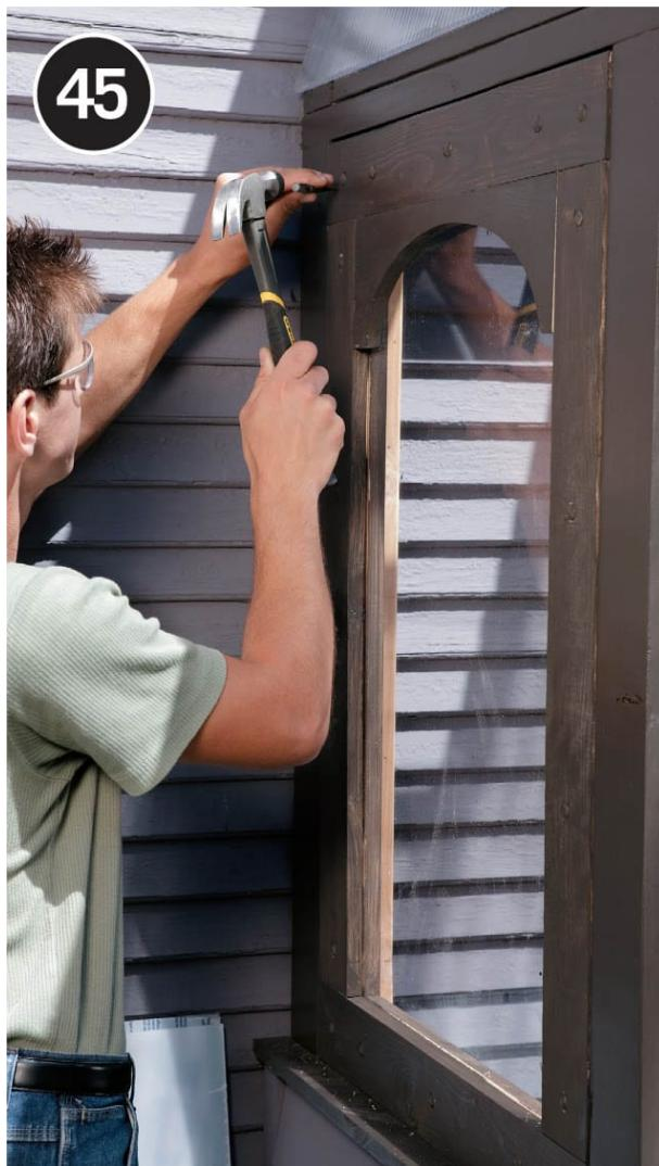
**Attach door stop molding** on the perimeter of each window opening, set so the window will be flush with the framed openings. Install fixed windows (if any) by centering the window unit in the opening side to side and driving a few 8d finish nails through pilot holes in the window and into the posts. Angle the pilot holes so the nail will not contact the glazing.
