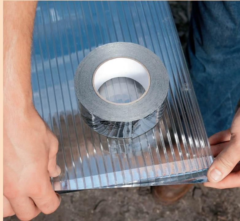
**Use foil tape** to cover the top edges of corrugated panels, protecting the edges from moisture and insects (spiders love to lay eggs in channels like these). The edge on the bottom of the panel can be covered with foil tape also, but you'll need to poke a small weep hole at the end of each channel so condensation can drain out. Or, you can use an alternate method such as L-shaped trim to protect the open panel ends (see Step 54).
