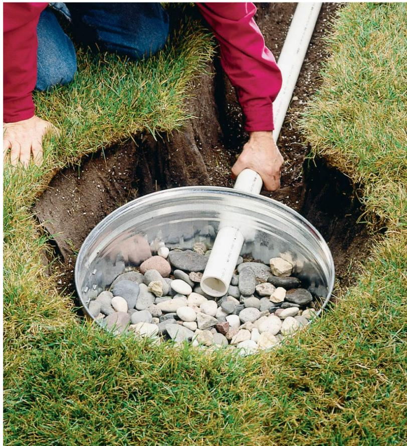
**A greenhouse with a water supply of any sort** should also have a drain. A dry well can be made with an old trash can or other container perforated with holes and filled with coarse rock. The well sits in a pit about 2' in diameter by about 3' deep and is covered with landscape fabric and soil. Dry wells are for draining graywater only—no animal waste, food scraps, or hazardous materials.
