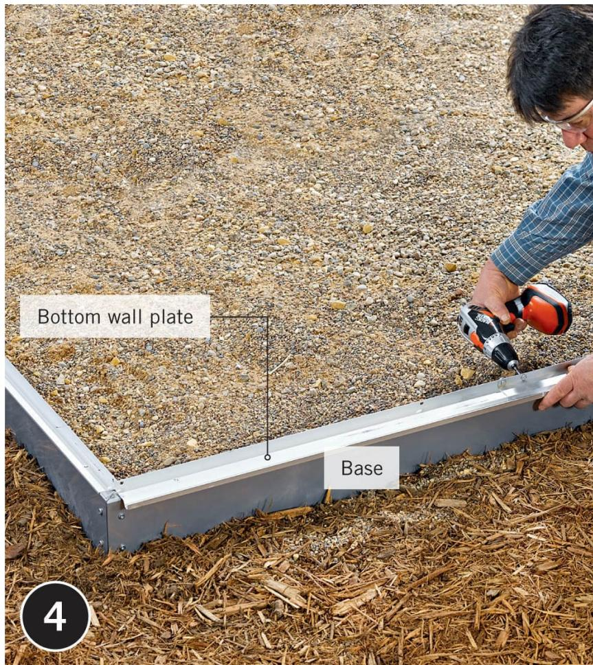
**Attach the bottom wall plates** to the base pieces so that the flanged edges face outside the greenhouse. In most systems, the floor plates will interlock with one another, end to end, with built-in brackets.
