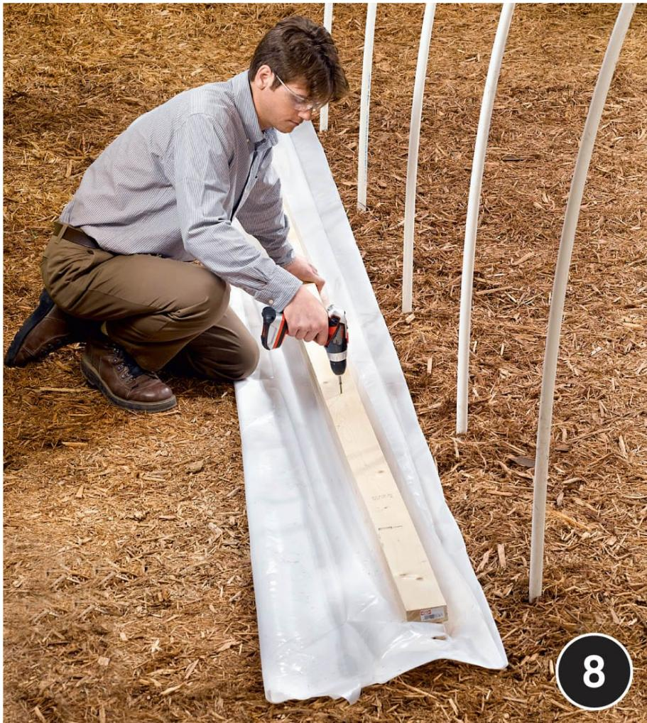
**Lay another 2 × 4 over the first** so their ends and edges are flush and the cover material is sandwiched in between. Fasten the two boards together with 2½" deck screws driven every 24" or so. Position the board assembly along the base of the hoops and pull the free end of the material over the tops of the hoops to the other side.
