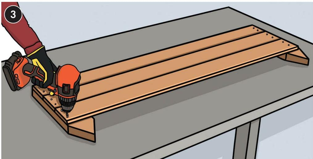
**Lay out three deck boards** stacked in a column. Align the longer post stakes with the column's top and outside edges, on both sides of the column. Screw them to the boards with 2" wood screws. Repeat the process with the shorter stakes and two deck boards (the top front deck board must be a wider 6" board) to construct the front wall.
