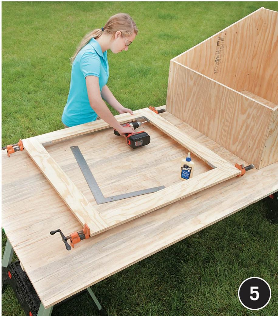
**Make the lid frame.** Cut the 4"-wide strips of  $\frac{3}{4}$ " plywood reserved from step 1 into frame parts (2 @ 31" and 2 @ 38"). Assemble the frame parts into a square  $38 \times 39$ " frame. There are many ways to join the parts so they create a flat frame. Because the Plexiglas cover will give the lid some rigidity, simply gluing the joints and reinforcing with an L-bracket at each inside corner should be more than adequate structurally.
