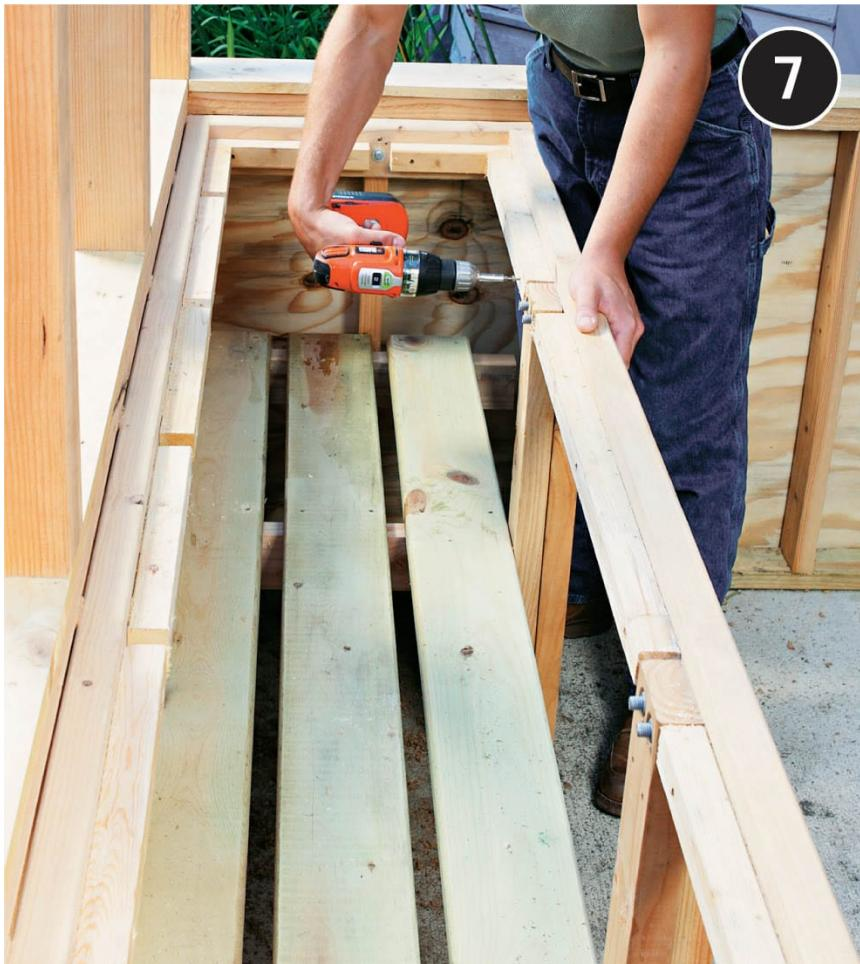
**Glue and screw 2 x 2 cleats** around the inside perimeter of the benchtop frame. The cleats should be positioned so they are level and the top faces of the deckboard slats will be about  $\frac{1}{8}$ " above the frame tops when they rest on the cleats. Install a full-length cleat along the back wall and fill in between the legs at the front.
