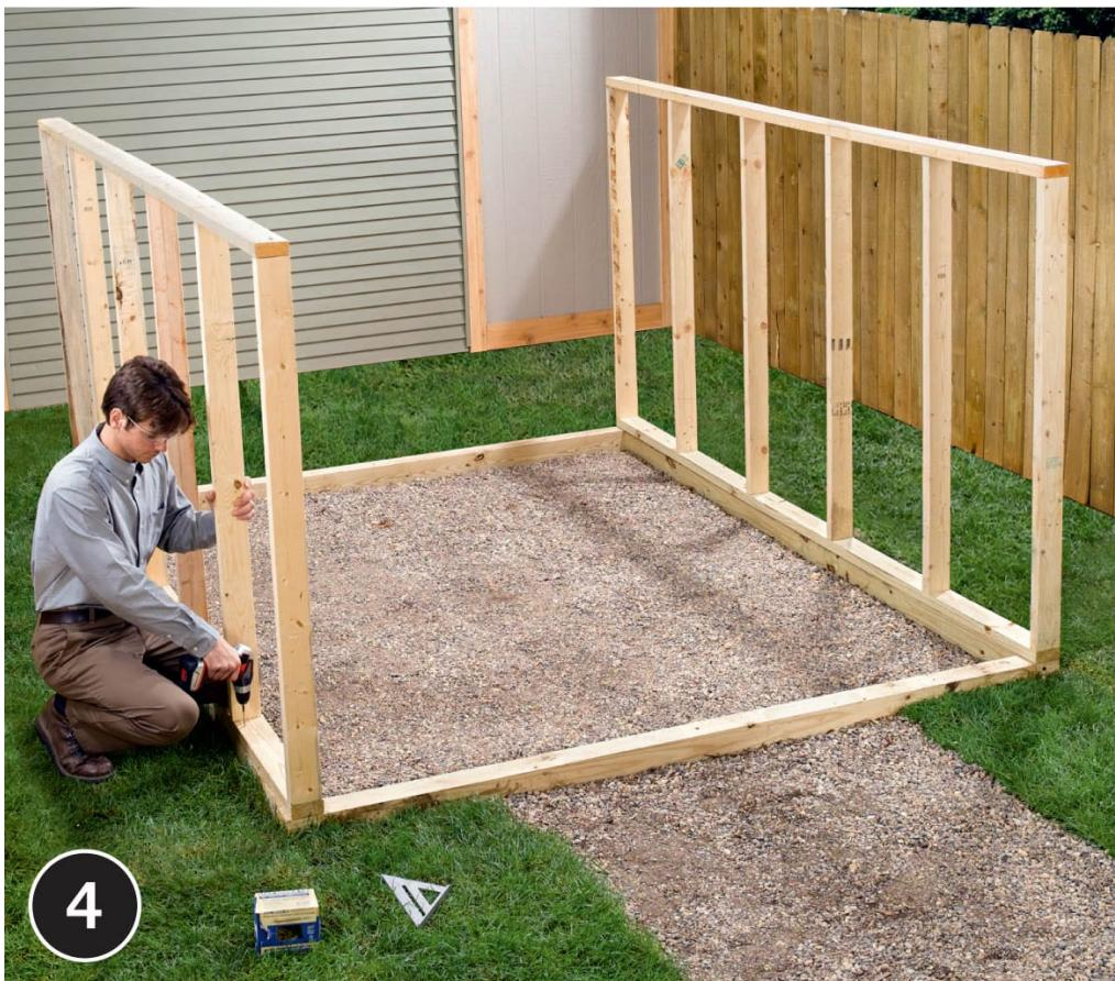
**Install the kneewalls** onto the timber base. Set each wall onto a side timber so the sole plate is flush with the ends and side edges of the timber frame. Fasten the sole plate to the timber with 3" deck screws.
