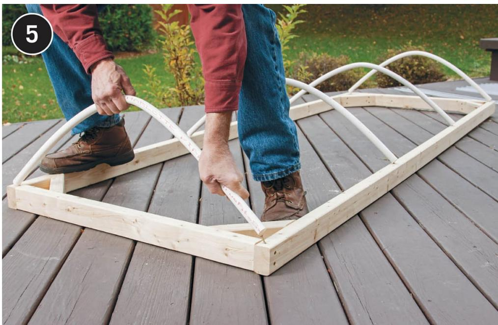
**Install the PVC ribs** by putting one end over the 2" screw, then curving the PVC until the other end fits over the opposite screw. Take your time with this, and use a helper if you need.
