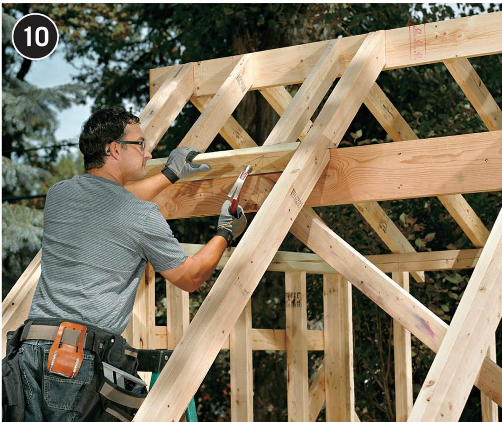
**Cut a pattern “C” rafter**, test-fit, and adjust as needed. Cut the remaining seven C rafters and install them. Measure and cut four  $2 \times 4$  nailers ( $311\frac{1}{16}$ “) to fit between the sets of B rafters (as shown). Position the nailers as shown in the HEADER + WINDOW DETAIL ([here](#)) and toenail them to the rafters.
