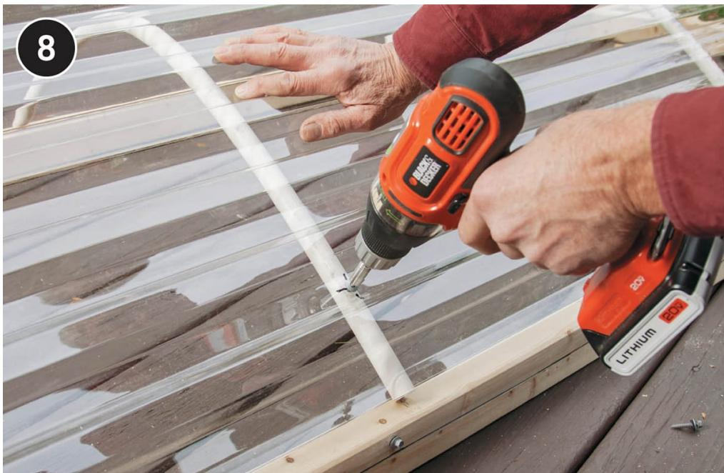
**Adjust the PVC ribs** until the predrilled holes in the roof panels are centered on them, then predrill the PVC with a  $\frac{1}{8}$ " bit. Fasten the panels to the two center ribs.
