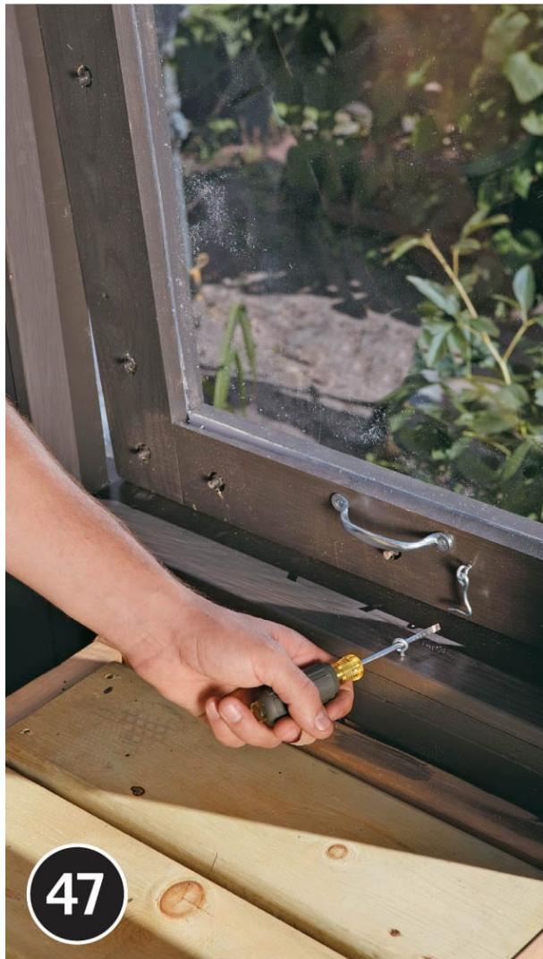
**Install door pulls and eyehooks** on the interior side of the window. Locate the pulls so they are centered and near the tops of the bottom window frame rails. Locate the eyehooks so there will be slight tension when the hook is in the screw eye—this will limit any rattling of the window.
