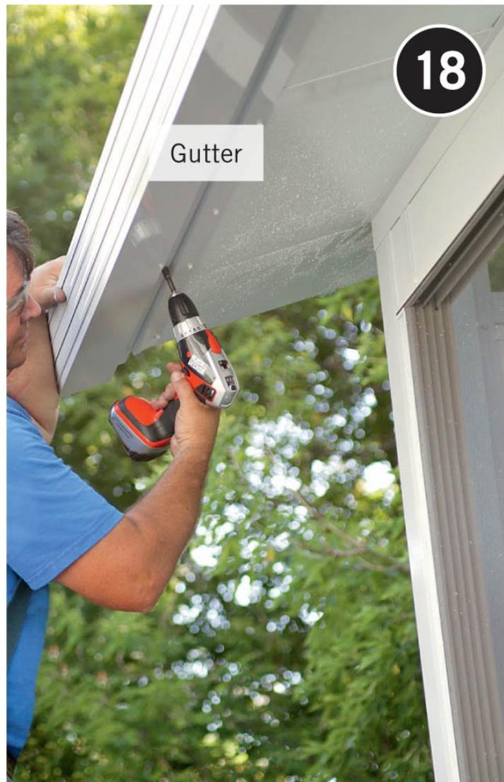
**Install fascia and gutters.** The materials seen here are designed specifically to work with the roof panel system of this kit. The fascia snaps over the ends of the roof panels and is secured with screws. The gutters fit into tracks on the fascia and are secured with screws.
