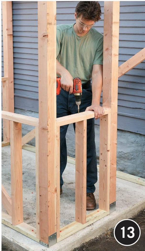
**Build stud walls** for the kneewalls between posts. Space the kneewall studs so they will be positioned beneath the intermediate posts. Attach the cap plate to the tops of the studs.
