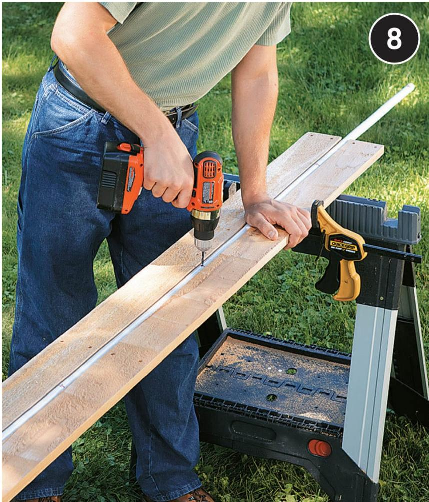
**Mark and drill the ridge pole** for the cover frame, using one of the 10' PVC pipes. Make a mark 1" from each end, then mark every 24" in between. The marks should form a straight line down the length of the pipe. At each mark, drill a  $3/16$ "-diameter hole straight down through the pipe.
