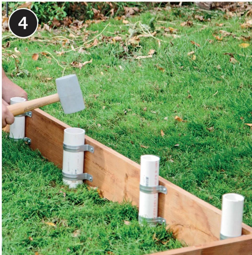
**Move the base frame** to the final site. Check that the frame is level and square by measuring diagonals and adjust as necessary. Use a wood mallet to hammer the PVC stakes into the ground, alternating sides, until the frame is secure.
