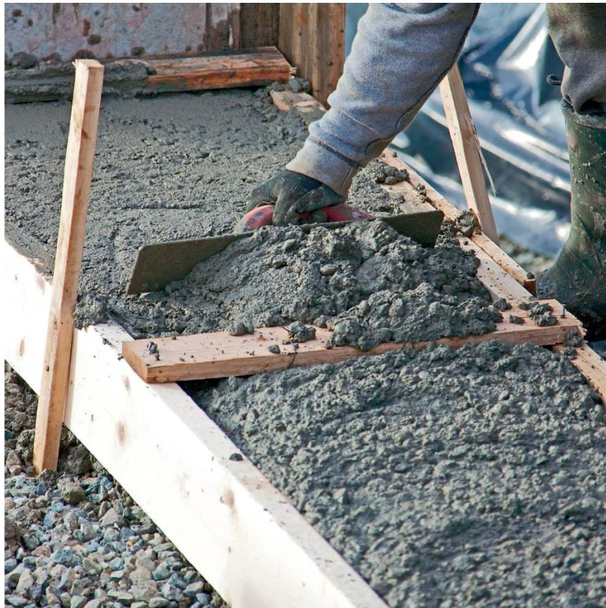
**A concrete footing** provides a structural base for a large greenhouse or a masonry kneewall. Standard footings are continuous and run along the perimeter of the structure. They must extend below the frost line (the depth to which the ground can freeze in winter; varies by climate) to prevent frost heave and should be at least twice as wide as the greenhouse walls they support.
