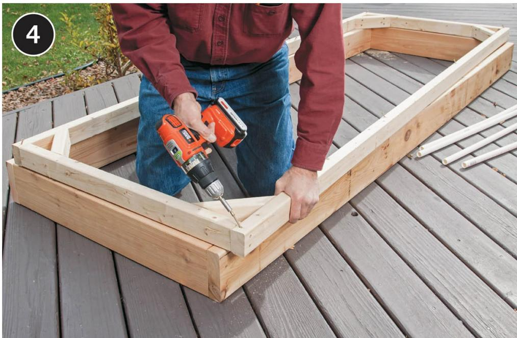
**Use 2" deck screws** as receptors for the PVC pipes. Drive the screws in 1" from edge and  $\frac{3}{4}$ " from the ends, angling the screws at about 35 to 45° toward the center. Leave about  $\frac{3}{4}$ " of the screw exposed. Drive two additional screws in at  $32\frac{1}{4}$ " from each end.
