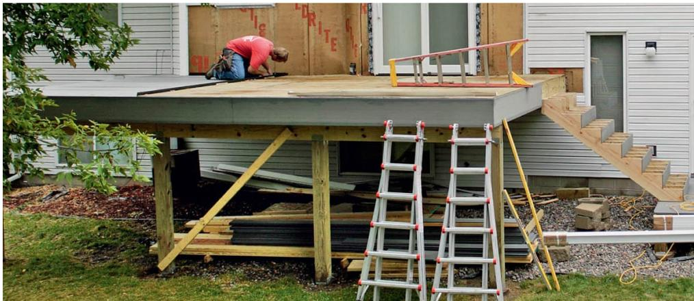
**To prepare for this new sunroom addition,** an old deck was replaced with a new, beefier model. It features a sturdy staircase with enough room on the left side of the addition for an open-air grilling area that is accessed through a door in the sunroom. Instead of decking, the deck area in the sunroom installation area is covered with  $\frac{3}{4}$ " tongue-in-groove plywood sheathing.
