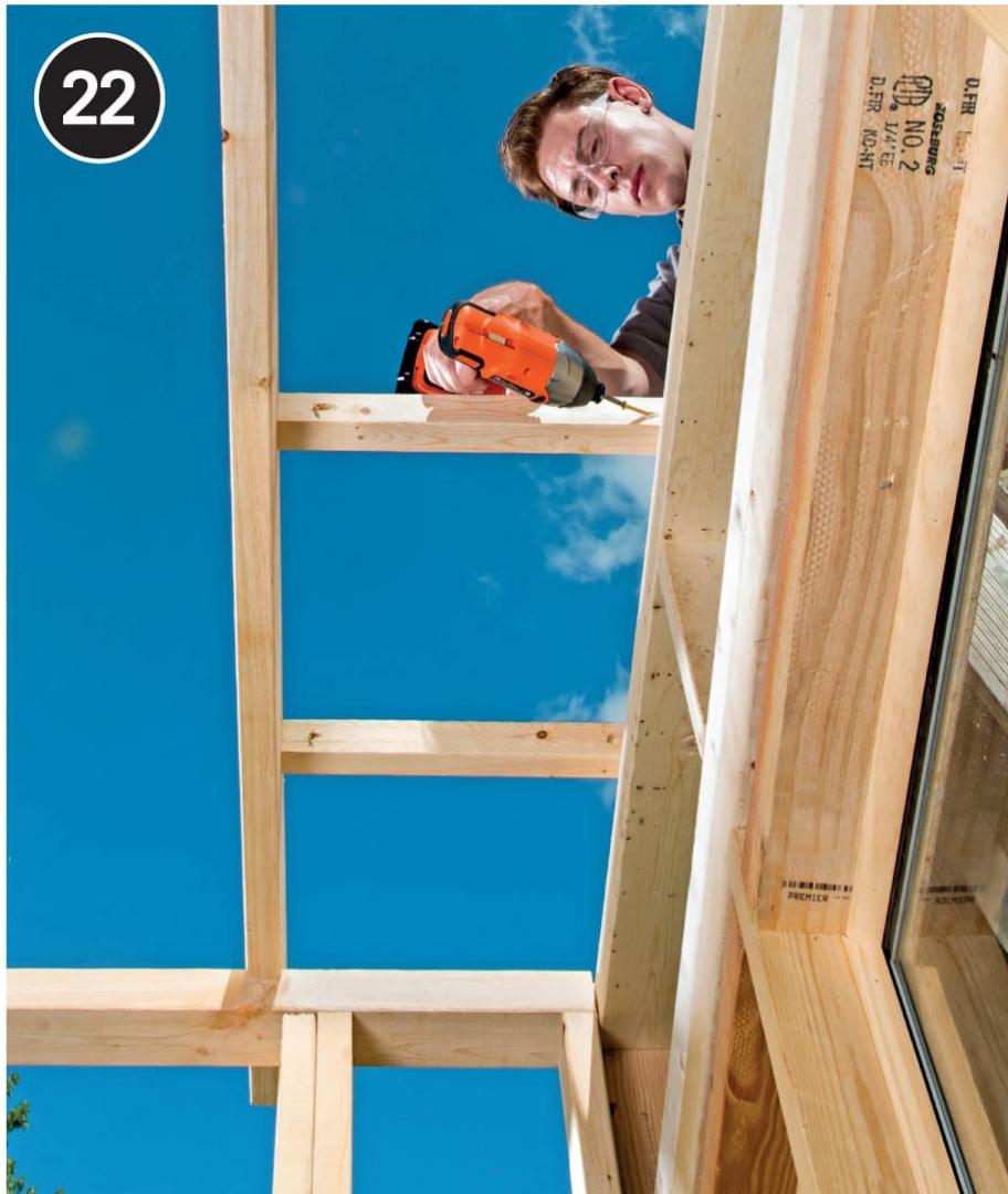
**Measure and cut the 2 × 2 purlins** for the gaps between the rafters. Toe-screw them in place, spaced 11½" on center.
