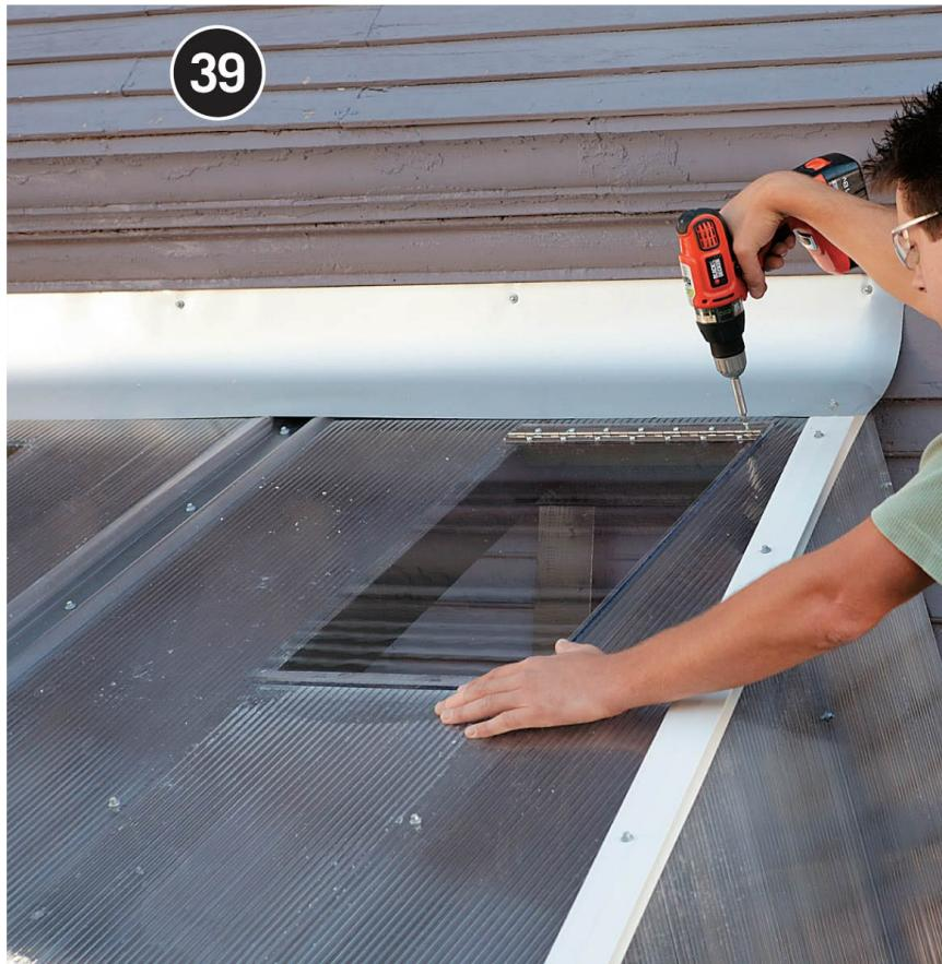
**Install roof vent covers.** (Here, the installation of the covers was postponed to allow access through the vent holes for installing flashing.) Use a piano hinge to attach each roof vent cover to the roof.
