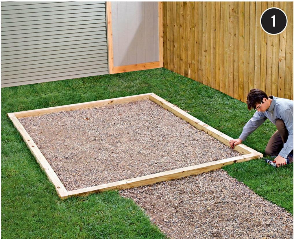
**Prepare the installation area** so it is flat and well drained; then cut the base timbers to length. Arrange the timbers so they are flat and level and create a rectangle with square corners. Drive a pair of 8" timber screws at each corner, using a drill/driver with a nut-driver bit.
