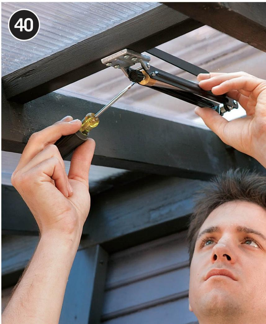
**Attach an automatic window vent opener** to each roof vent cover, according to the hardware manufacturer's instructions. These devices have internal sensors that lift the vent cover when the greenhouse overheats.
