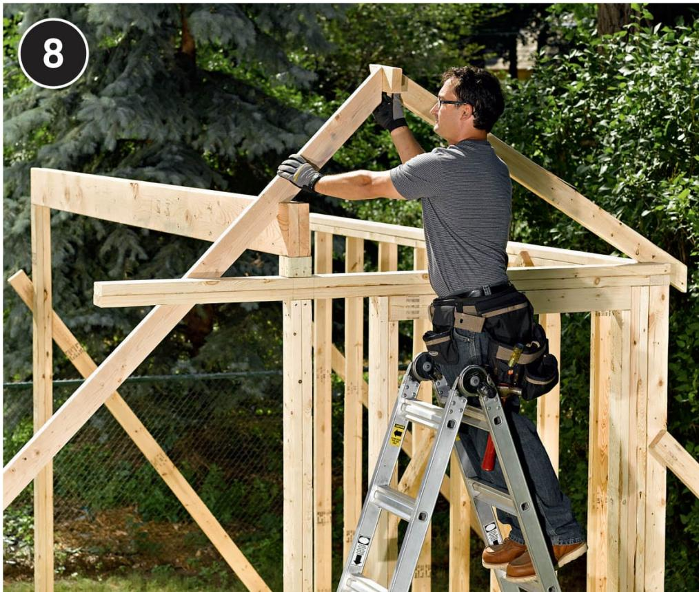
**Cut one of each** “A” and “B” pattern rafters using the RAFTER TEMPLATES ([here](#)). Test-fit the rafters. The B rafter should rest squarely on the rafter header, and its bottom end should sit flush with outside of the front wall. Adjust the rafter cuts as needed, then use the pattern rafters to mark and cut the remaining A and B rafters.
