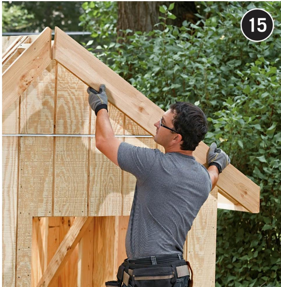
**Install 1 × 6 fascia** over the ends of the A rafters. Keep all fascia  $\frac{1}{2}$ " above the rafters so it will be flush with the roof sheathing. Using scrap rafter material, cut the 2 × 4 lookouts ( $5\frac{1}{4}$ "). On each outer B rafter, install one lookout at the bottom end and four more spaced 24" on center going up. On the A rafters, add a lookout at both ends and two spaced evenly in between. Install the 1 × 6 rake boards (fascia) as shown in the RAKE BOARD DETAIL ([here](#)).
