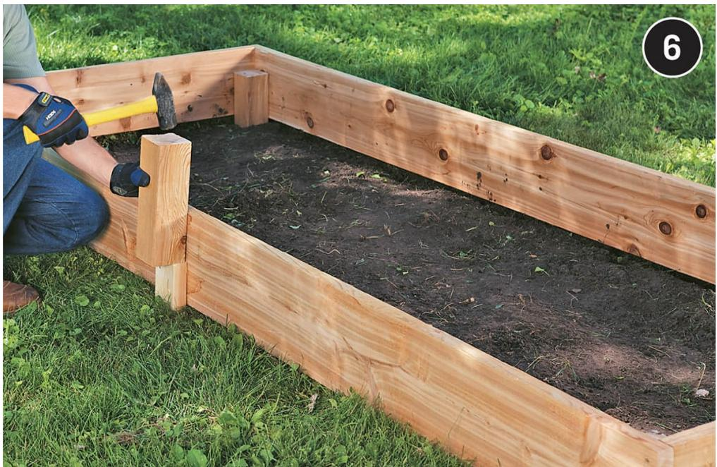
**Add a 2 x 4 stake** at the midpoint of each frame side, to help keep the lumber from bowing out over time. Cut the stake to a point and drive it down below the top edge of the frame. Tack the stake to the frame with a couple of screws.
