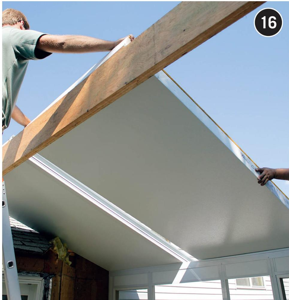
**Add the next roof panel to the roof**, sliding it into the open side of the I-beam. Square the panel with the roof, and then drive insulation screws down through the panel and into the ridge pole and the upper wall track. Add the next I-beam and fasten it with self-tapping screws.
