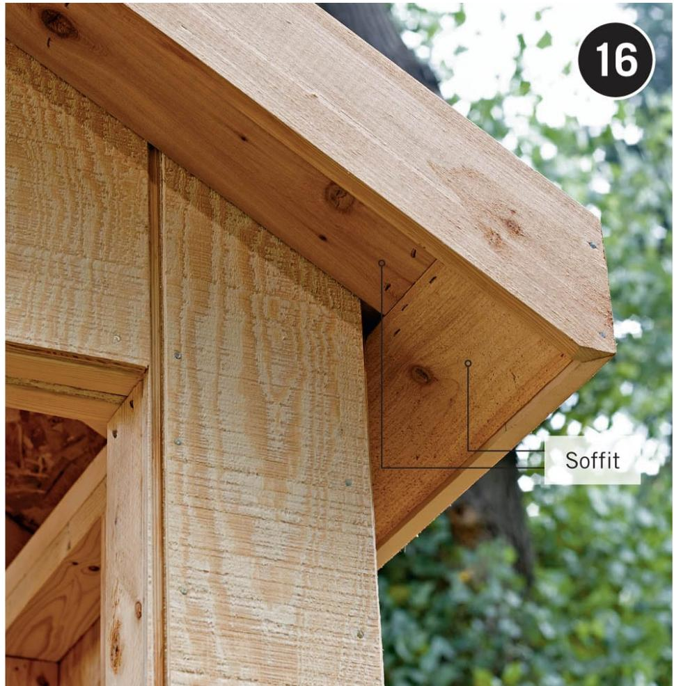
**Rip 1 × 6 boards** to  $5\frac{1}{4}$ " width (some may come milled to  $5\frac{1}{4}$ " already) for the gable soffits. Fasten the soffits to the lookouts with siding nails. Rip a 1 × 8 board for the soffit along the rear eave, beveling the edges at  $30^\circ$  to match the A rafter ends. Install the soffit.
