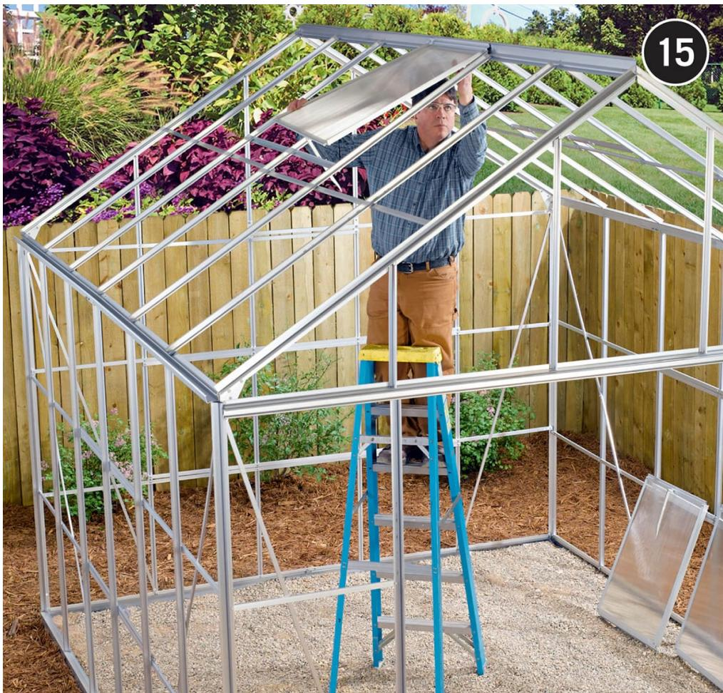
**Build the roof windows** by first connecting the two side window frames to the top window frame. Slide the window panel into the frame; then secure it by attaching the bottom window frame. Slide the window into the slot at the top of the roof crown; then gradually lower it in place. Attach the window stop to the window support beam.
