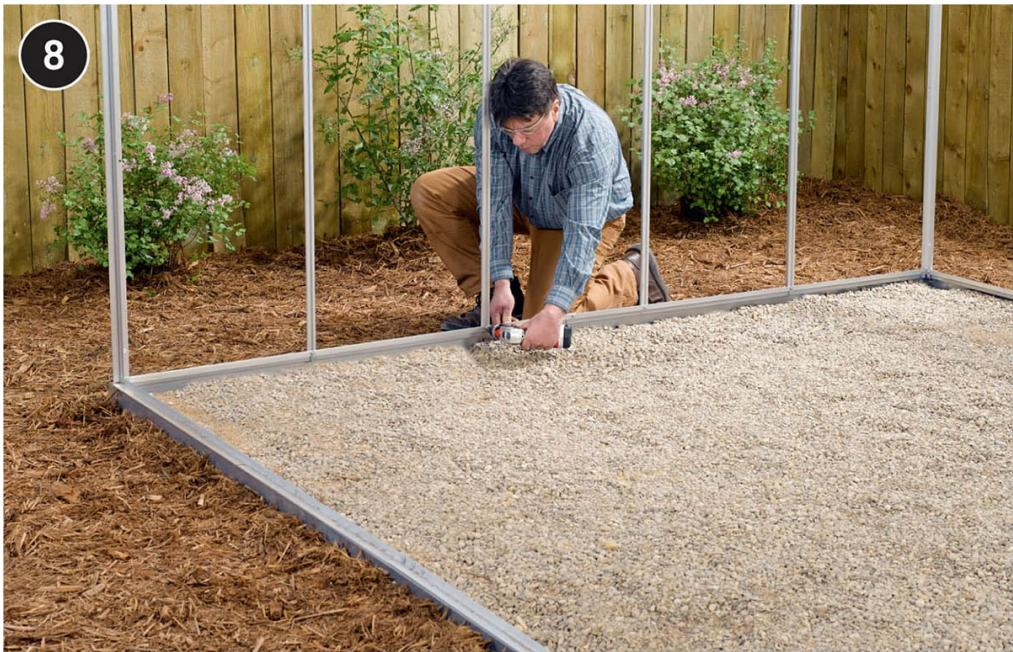
**Fasten the left and right rear studs** to the outside of the rear floor plate, making sure the top ends are sloping upward, toward the peak of the greenhouse. Attach the center rear studs to the rear floor plate, fastening them to the stud connectors used to join the rear braces.
