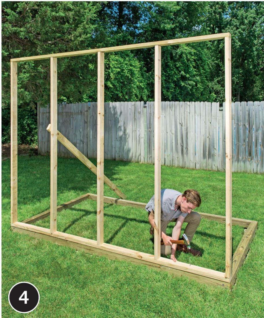
**Raise the wall**, check for plumb, and brace it into position. Nail the sole plate to the foundation timber with 8d nails.
