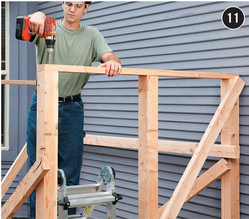
**Cut the 2 × 4 endwall cap plates to length** and screw them to the tops of the corner posts with 3" deck screws. Test frequently to make sure the corners are square and the edges are flush with the post edges.
