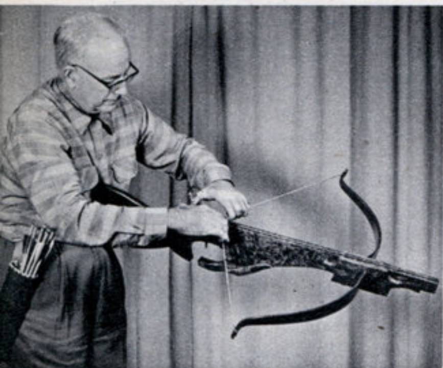
The proper method of cocking the crossbow with a bolt in firing position. As shown here, practice cocking without a bolt until you acquire skill.
