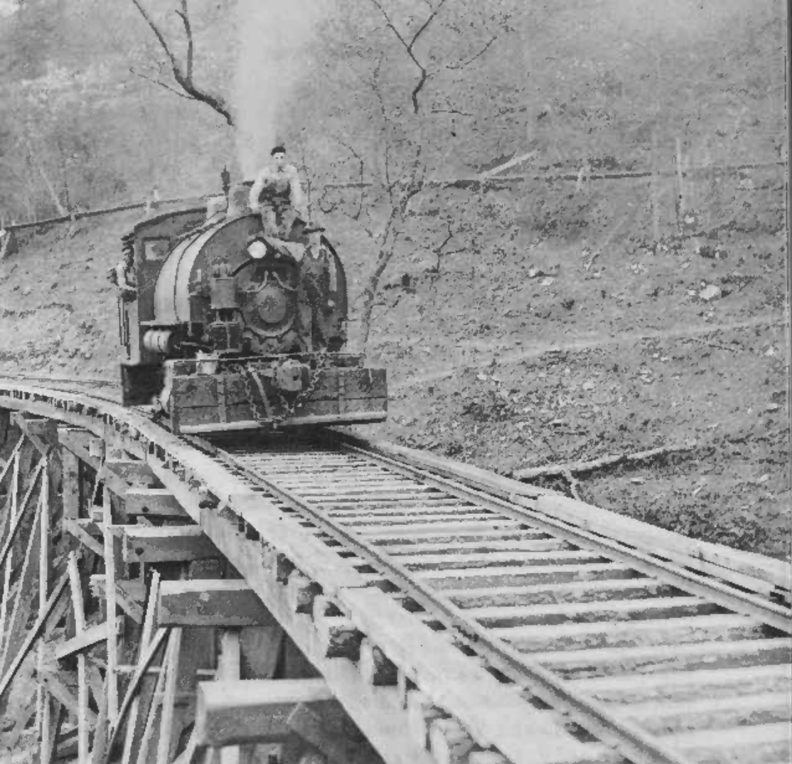
This spur was built off the Tallulah Falls track to facilitate the building of Burton Dam (which created Lake Burton) by the Georgia Power Company. (Photograph courtesy of Tom Moss)
