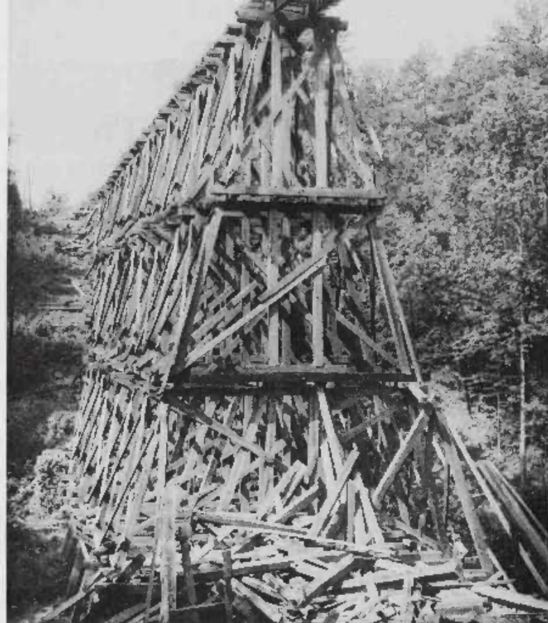
This picture of the Panther Creek trestle being taken down in 1962 shows the possible devastation of a collapsing trestle.
