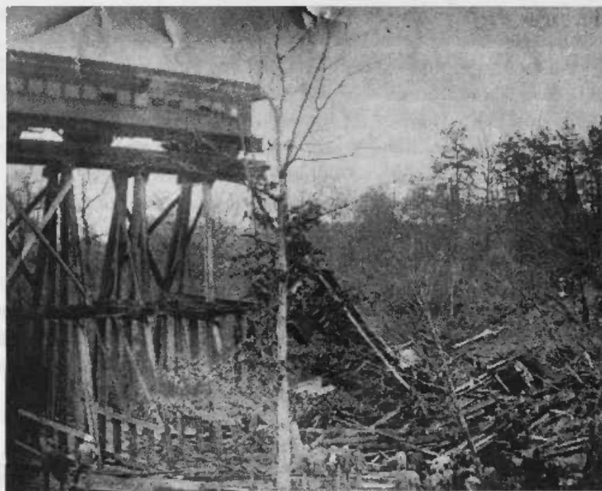
The Hazel Creek trestle collapsed under the weight of a passenger train. This photograph shows how many of the supporting beams are gone from under the passenger car that remained on the tracks.
