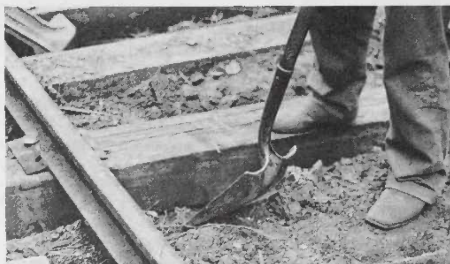
A section crewman tamps dirt around a tie.
