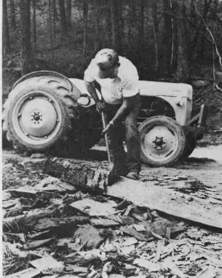
Dan Crane, Sr., demonstrates part of the process of hewing a cross tie.
