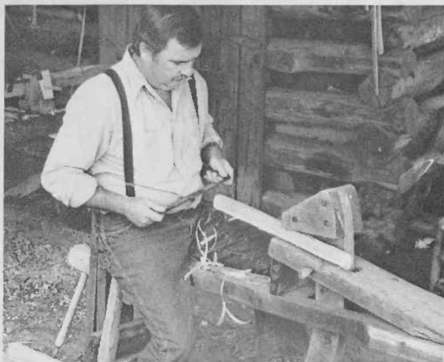
Jimmy uses a drawknife to shave the wood down to the desired size. He then drills a small hole in the center of each end to accommodate the pointed screw on the head and tailstock of the lathe.
