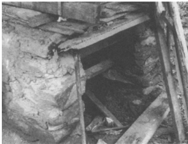
PLATE 13 The furnace is a simple stone and cement structure with pieces of angle iron used as a supporting frame
