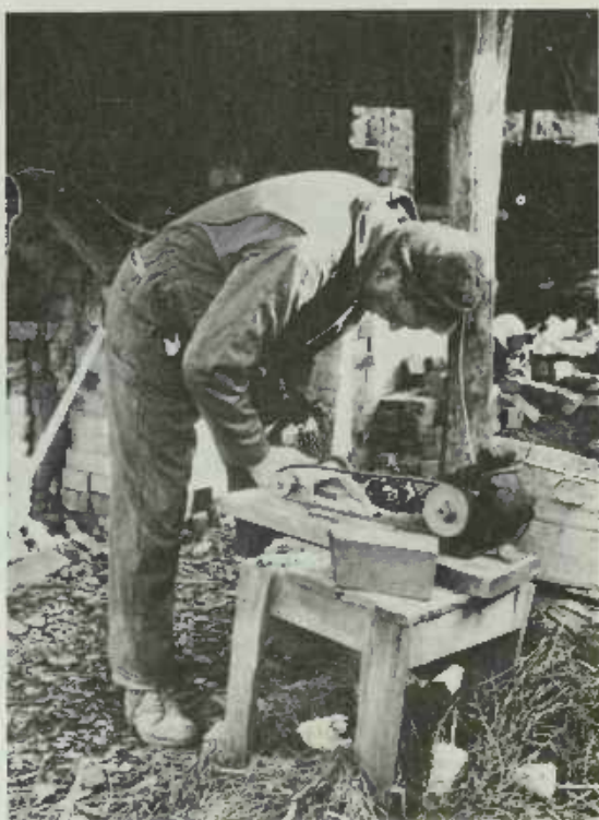
PLATE 131 If there are beads of glaze left around the bottom edge of any of the pieces, Lanier grinds them off before selling the piece.
