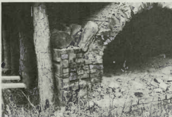
PLATE 122 Between the vertical log posts and the kiln's sidewall, and behind the brick column visible here, is a long trough filled with dirt for insulation against the sidewall.
