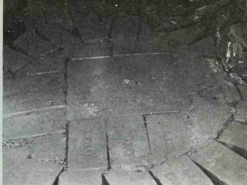
PLATE 395 A view of the center of the kiln floor. This is the only area of the floor that is solid, and is the coolest part of the kiln. Note how the bricks have spaces between them as they go out from the center. The lattice floor of the kiln is eighteen to twenty-four inches above the actual dirt bottom of the kiln. There are channels running under the lattice floor to a tunnel at the rear of the kiln which goes into the chimney, creating a draft for the kiln fires.
