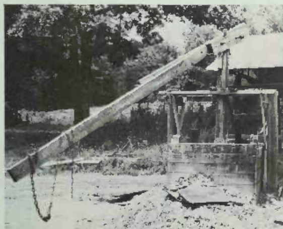
PLATE 303 When preparing clay, Norman puts as much raw clay as he needs into the mill from the pile beside it, wets it down, and makes about 150 revolutions with the tractor.
