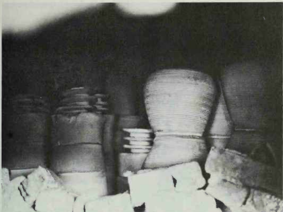
PLATE 327 Norman loads the ware and fires the kiln through the same door, because "that's the way I learned." He has seen kilns with a door in the side of the firebox so that longer wood can be pitched in, but he likes his way best. Unglazed ware, since it won't stick together, is stacked as high as five pieces high in tight rows that run lengthwise in the kiln. The flash wall is visible in the foreground of the above photograph.
