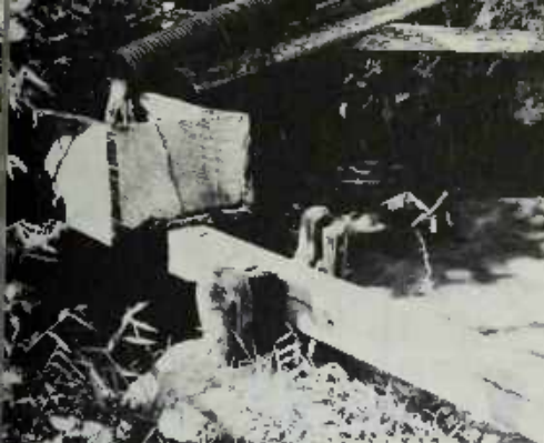
PLATE 277 On a subsequent visit, Burlon had built a new mill, and it was in operation. Water was directed into a box at one end of the horizontal shaft.
