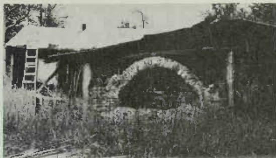
PLATE 120 When the chimney on Lanier's kiln partially collapsed in April of 1983, he removed it. Without the chimney, the construction of the end of the arch was easily visible . . .
