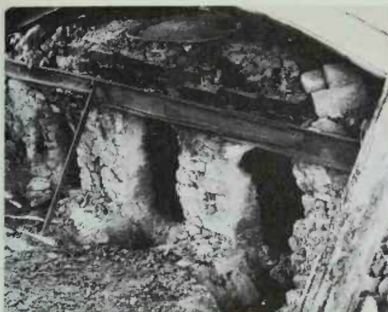
PLATE 287 Burlon's kiln from the breast end, showing the holes through which he fires it and the three corresponding flue holes.
