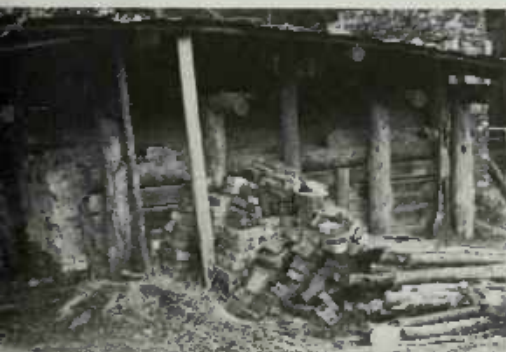
PLATE 117 The kiln Ianier used until the spring of 1983. This kiln's dome was arched higher than those of previous ones, and it was loaded through the fire pit end instead of the chimney end.
