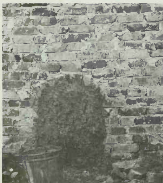
PLATE 107 One brick in the chimney door was left loose so that it could be removed during firing in order to observe the cones.
