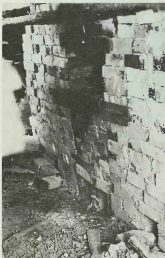
PLATE 128 The door was bricked partway up, and then a steel beam was fitted into place on top of the last row of bricks. The remaining hole is the one through which Lanier shoved pine slabs during the firing.
