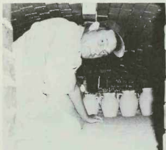
PLATE 101 Lanier setting the ware in preparation for firing. Then, as now, no ware was stacked. "There's just one layer of glazed ware."
