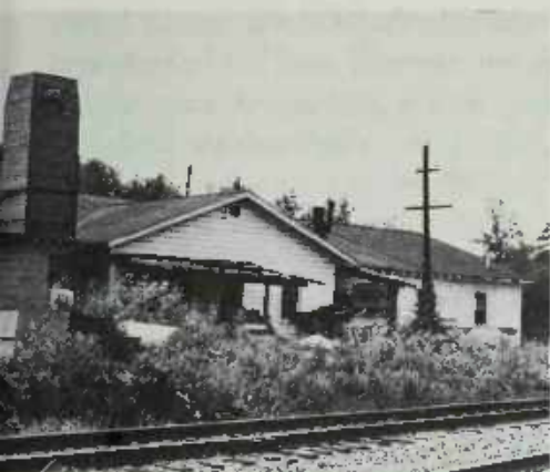
PLATE 401 A rear view of Brown's Pottery showing the large kiln chimney at left. The vibrations from fast-moving trains occasionally cause pottery in the kiln to fall.
