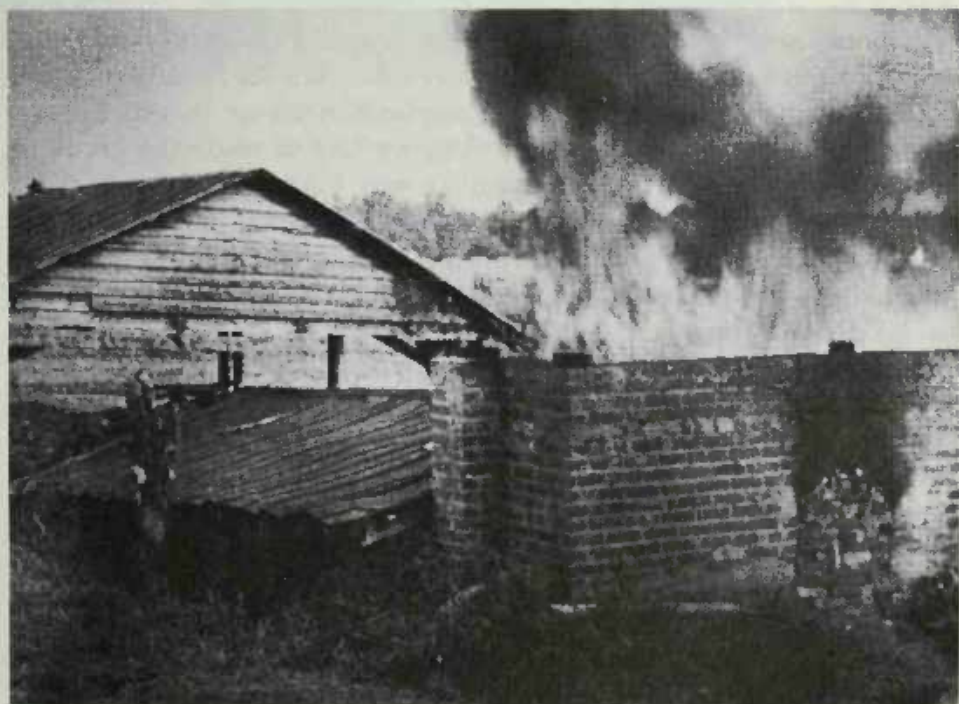
PLATE 293 An old photograph in Burlon's collection shows the kiln being fired. Note how the door in the chimney end is bricked up.
