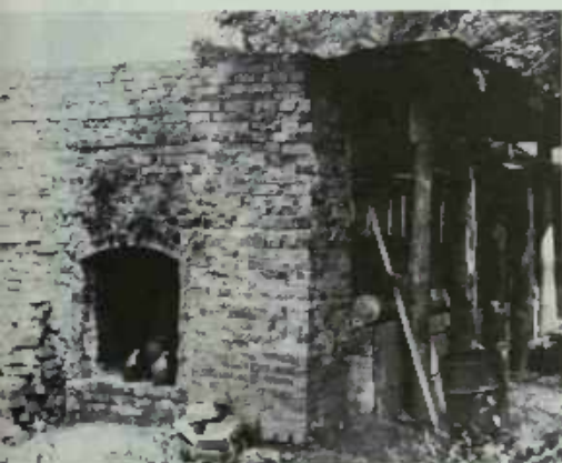
PLATE 116 A day or so later, after the kiln has cooled off, the bricks are removed from the door and the finished ware unloaded. In this photograph, taken in the mid seventies, Lanier had rebuilt the kiln and had left a larger door in the chimney than in his previous one.
