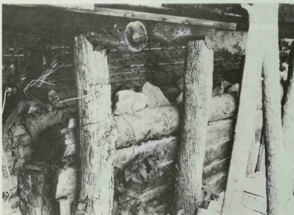
PLATE 119 Nevertheless, as in previous kilns, Lanier had the base of the dome securely braced. In this case, mortar was used between the bricks in the dome instead of red clay mud. It burned through and dropped out in many places. When the kiln was being fired, Lanier said, "You can see through every crack in it. It just takes a little bit more wood, and it really don't matter. The fire is still confined in it, and that's what you want."
