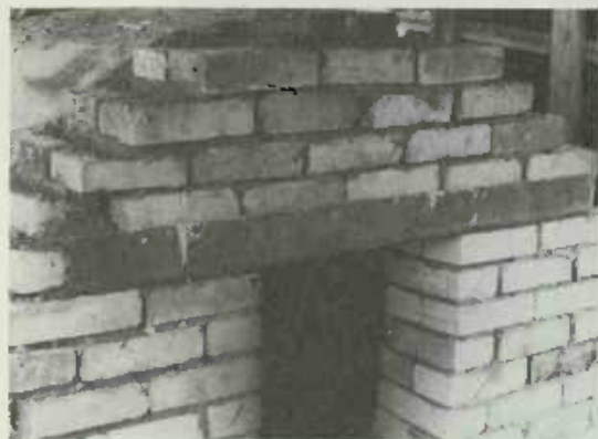
PLATE 94 With a piece of heavy angle iron placed across the top of the doorway, Cleater was able to finish the end. The two blackened bricks whose ends are visible at the top of this photograph are two of four bricks that Cleater salvaged from his father's kiln and set into his own for good luck.
