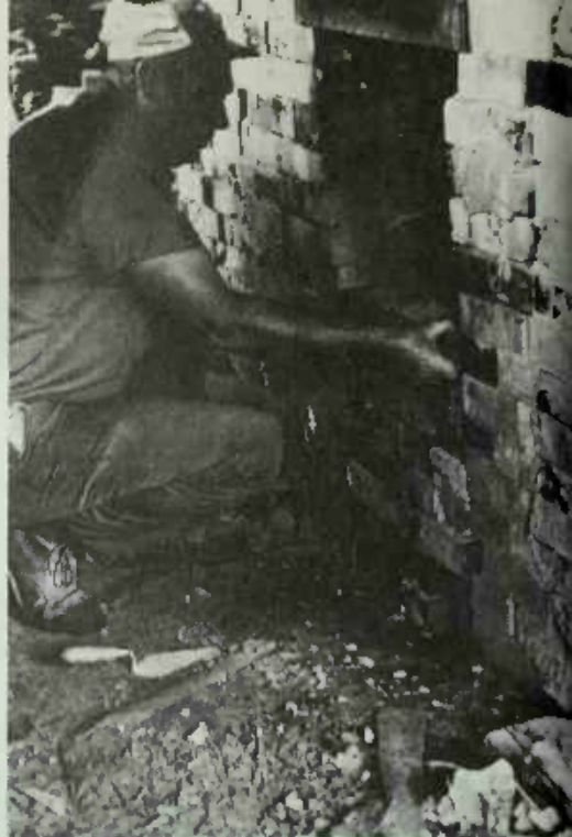
PLATE 127 To fire the kiln, Lanier bricked up part of the fire pit door after loading the ware in, making sure to leave two small draft holes in the bottom.
