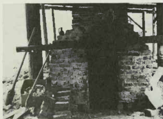
PLATE 142 On either side of the door, at the base, a draft hole is visible. Lanier has found that they are too small and plans to enlarge them before he fires the kiln again.
