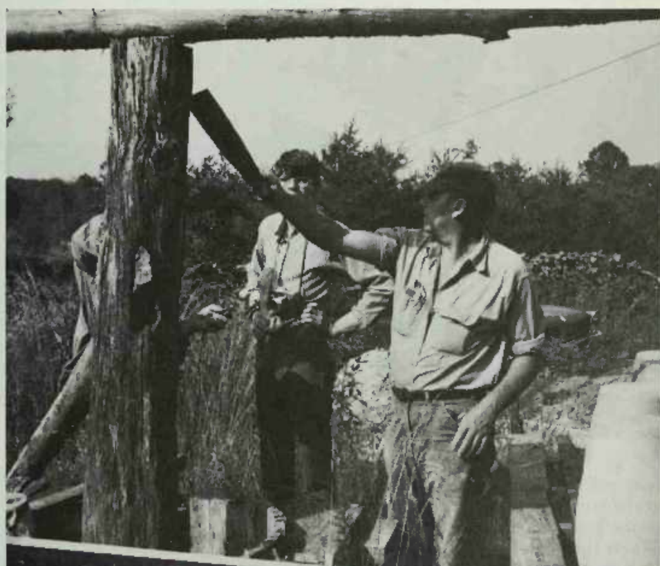
PLATE 49 When the mill is constructed, a hole is drilled into either end of the vertical pole or "staff" Lanier is pointing at. Into each hole, a white-oak pin or dowel at least an inch and three-quarters in diameter and six inches long is inserted. The end of one pin goes through the flooring of the mill, which is made of two-by-sixes and two-by-eights resting flat on the ground. The end of the other pin goes into the horizontal pole overhead. In this way the staff is held in place, but it can still rotate.
