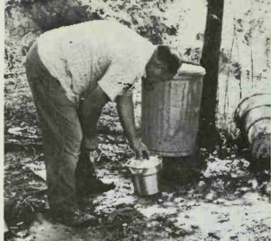
PLATE 274 Burlon inspecting a bucketful of pulverized glass from the mill. It will be sifted and the larger pieces returned to the mill for further processing.
