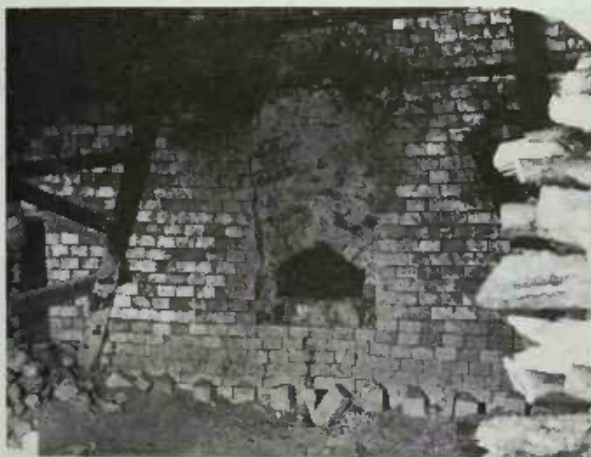
PLATE 328 To fire, the loading door in front is bricked up, leaving an opening through which the four cords of pine slabs needed for the 2400° F. burn will be loaded.
