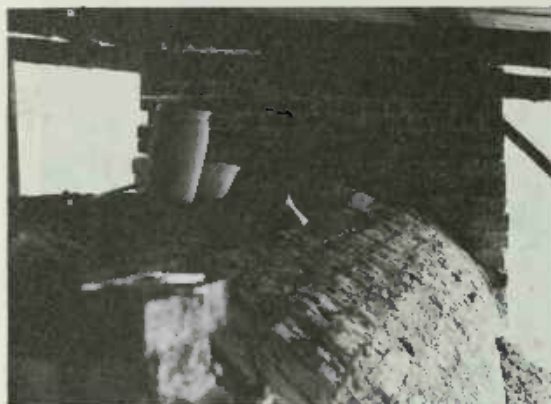
PLATE 139 The arch of the new kiln is a perfect half circle.
