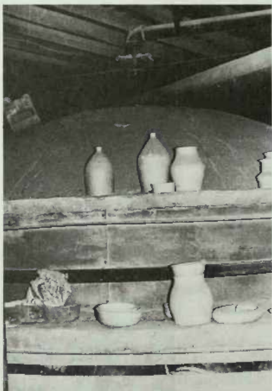
PLATE 398 A view of the kiln showing the domelike top. Note the expansion bands and cable.
