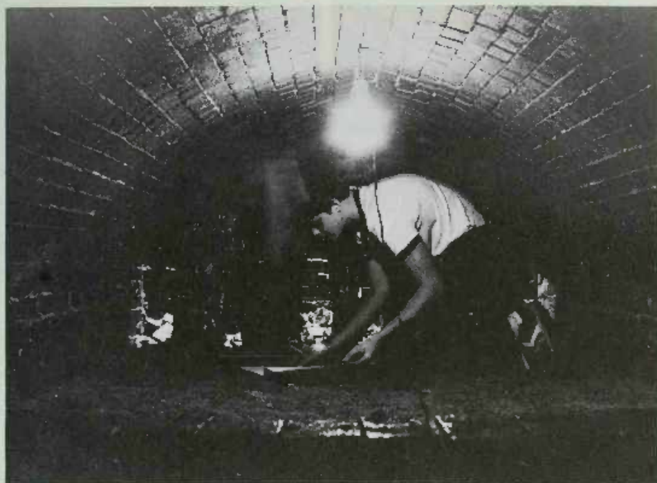
PLATE 124 Curtis Weaver measuring the inside of the kiln Lanier stopped using in 1983. Beyond him, the flues in the base of the chimney are barely visible. In this case, instead of three large flues as in the previous kilns, Lanier had a row of smaller ones across the entire end [see Plate 125].
