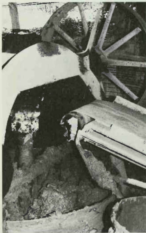
PLATE 382 The conveyer belt bringing dry clay into the clay mill to be mixed with water and packaged Ohio clays.
