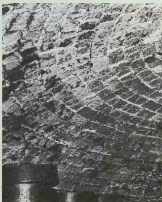
PLATE 396 The firebrick-lined ceiling of the kiln.
