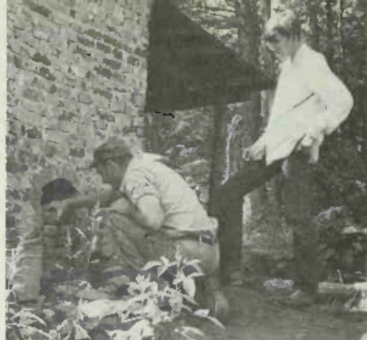
PLATE 105 Before firing the old kiln, Lanier would brick up the door in the chimney end through which he had loaded the ware.
