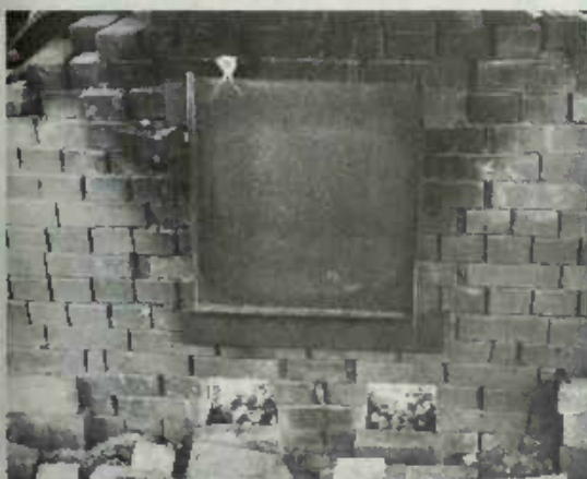
PLATE 219 Two of the draft holes in front of the kiln are left open during firing.
