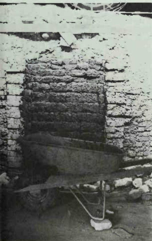
PLATE 390 The kiln sealed and ready to be fired.
