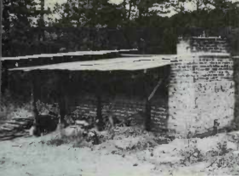
PLATE 136 The new chimney is stepped in in two places. At its base, the three removable bricks are visible. When these are slipped out, the holes afford Lanier a view of the ware and cones inside the kiln when it is being fired.
