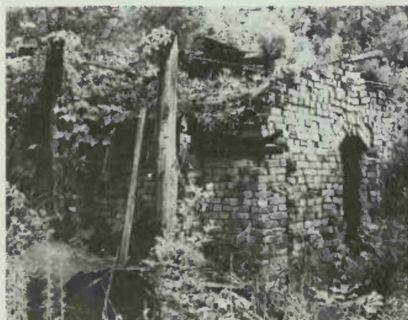
PLATE 323 A second abandoned kiln, its walls supported by brick columns braced by wooden poles foreshadowing the design of the kiln Norman uses today.
