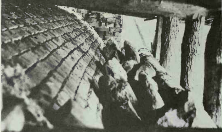
PLATE 118 Looking down the outside of the dome toward the chimney, the increased curve of the dome is visible; in this case, in Lanier's words, a "half circle. And it don't need all them braces on the side of it to hold it up. If it's a perfect half circle, that thing will hold itself up."
