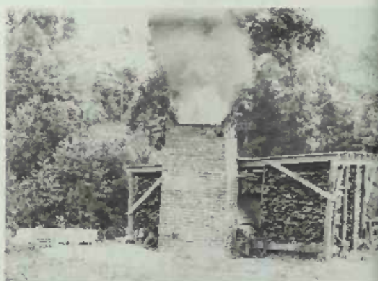
PLATE 97 That done, Cleater finished the chimney, keeping the walls two bricks thick until the chimney was nearly to the roof line of the kiln shed. Then he stepped the thickness down to one brick and tapered the walls in to close the opening slightly. Several weeks later he burned a kiln of ware, and we were there to get this photograph.
