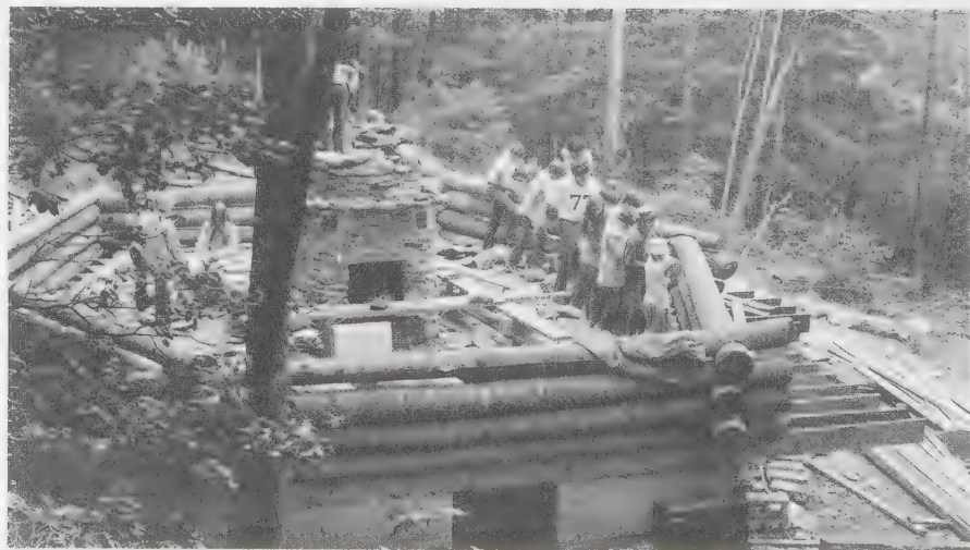
As one group of students raised wall logs into place, another worked on the central chimney.
