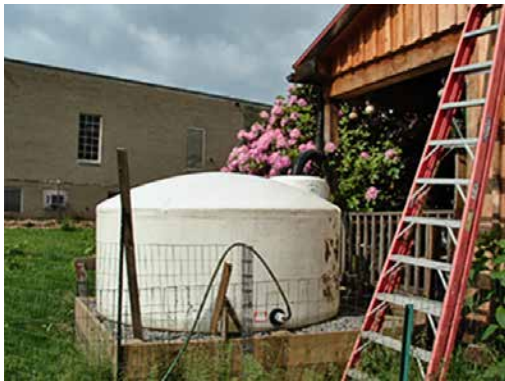
The cistern set up on stone foundation.
