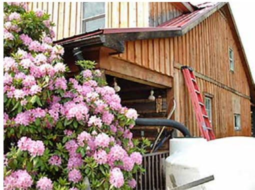
Cistern for rain garden connected to house.
