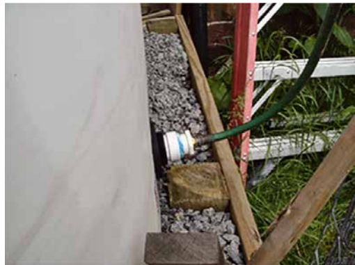
Cistern outflow connection for rain garden.
