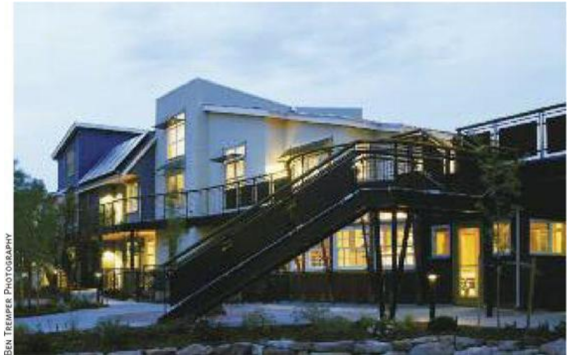
View of courtyard at dusk.
