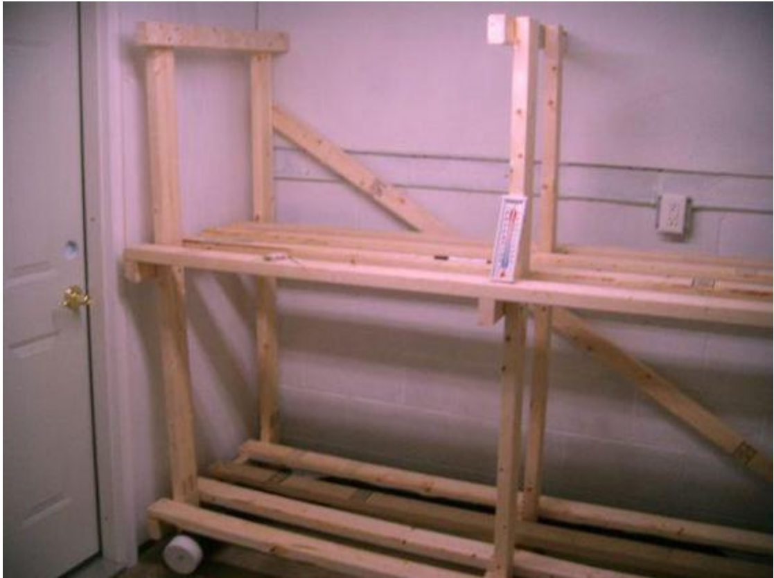
Homemade shelves built from 2X4s allowed for plenty of ventilation. Emily propped them up on bricks to keep their feet out of the water that sometimes flows over the floor.
