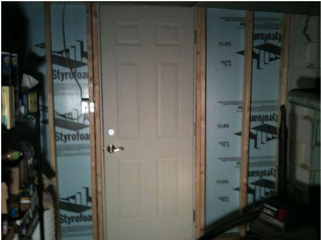
The majority of the foam insulation was used to insulate the walls.
