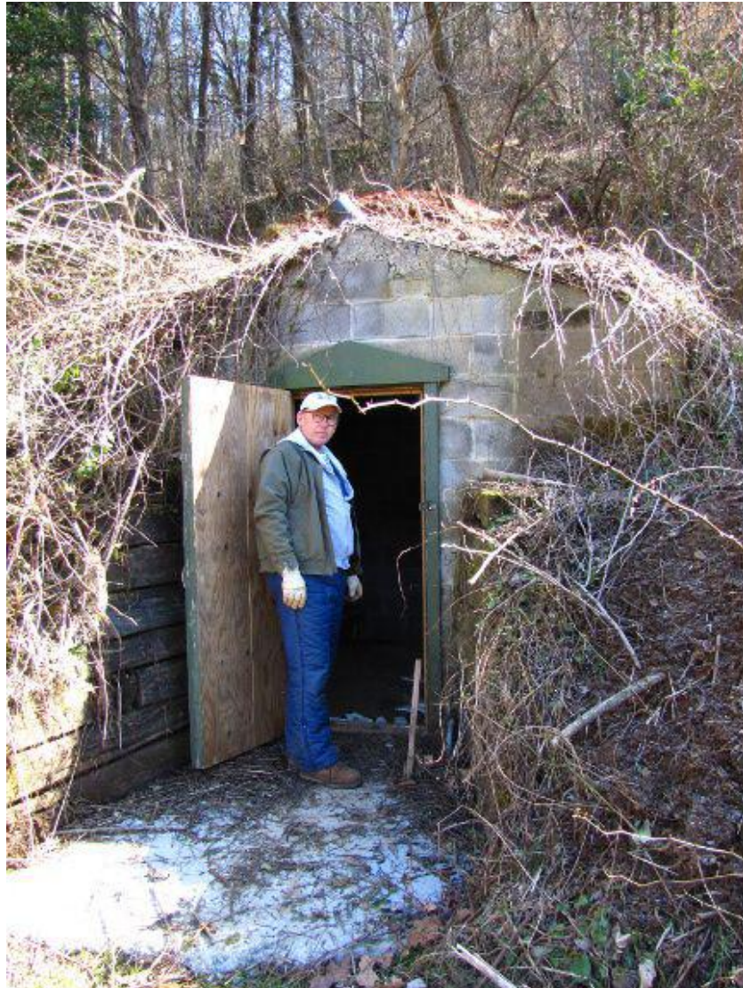
Frank's root cellar is built into a north-facing hillside.
