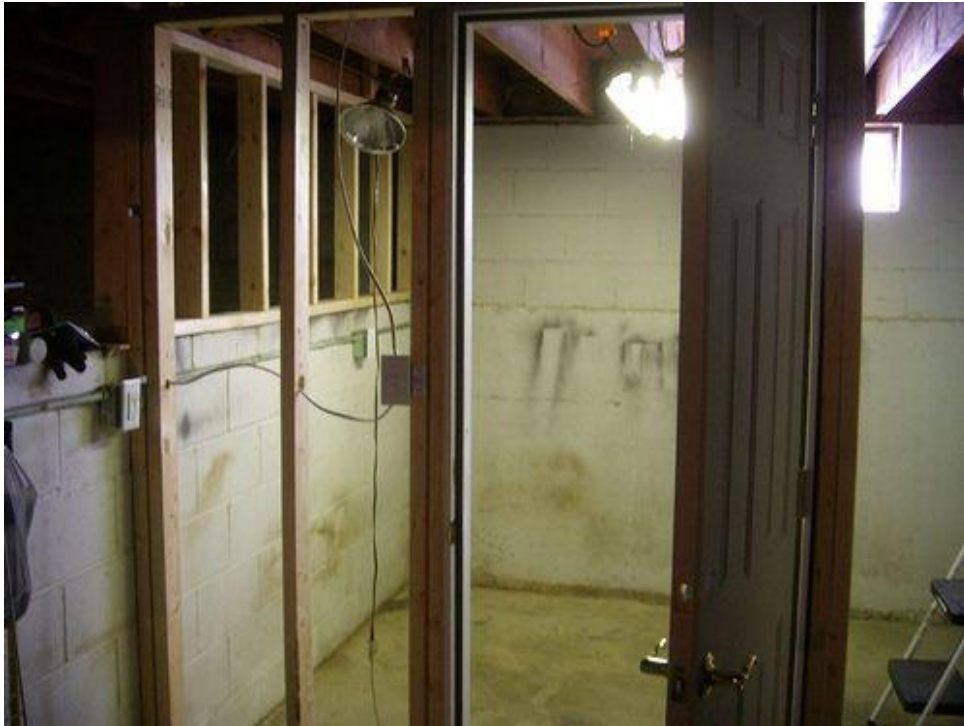
Separating the root cellar area from the rest of the basement required Emily to build one large wall and one small wall.
