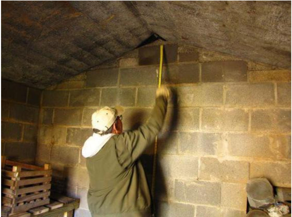
The ceiling consists of between-three-and-four inches of concrete reinforced with rebar and remesh.
