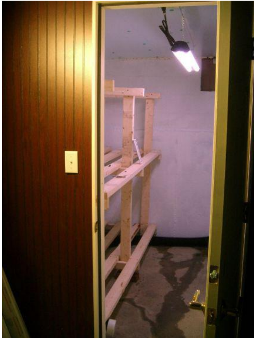
This paneling was later taken down to prevent the growth of mold.
