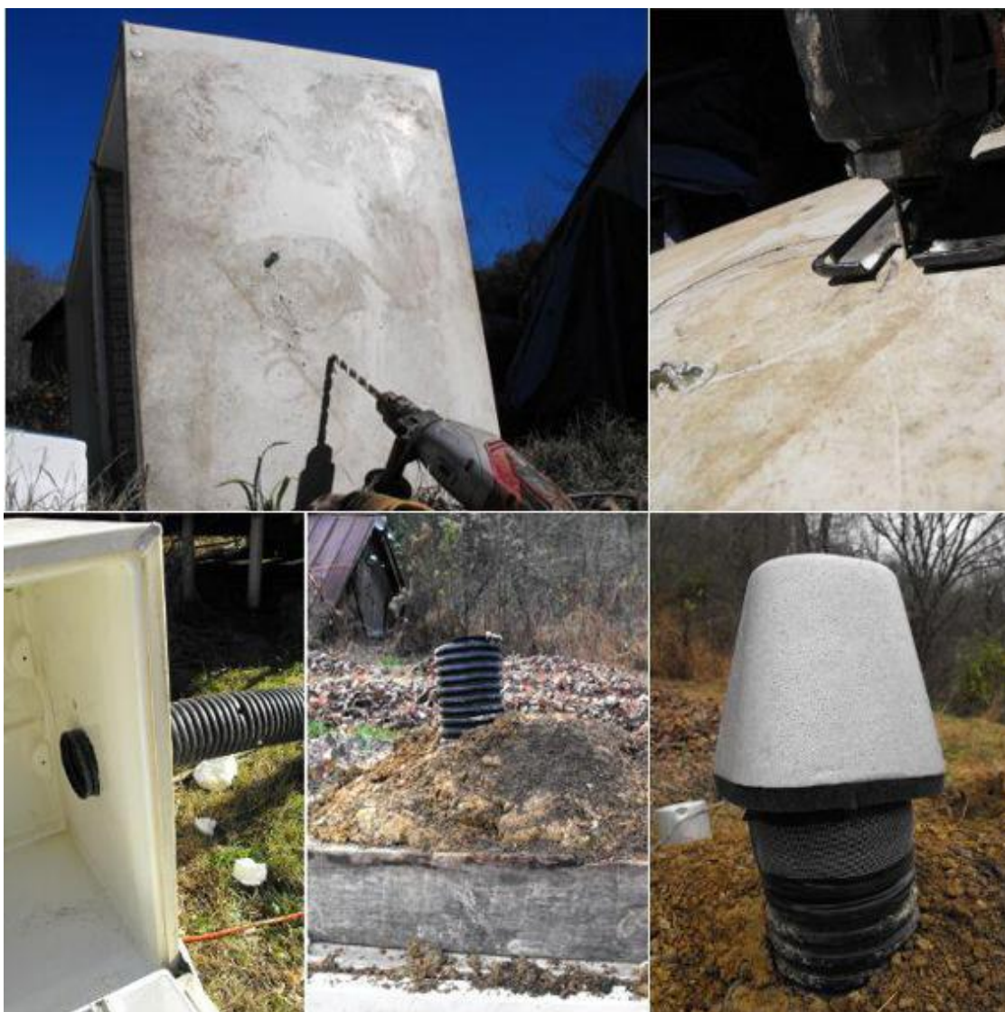
Be sure to provide a capped ventilation pipe.
