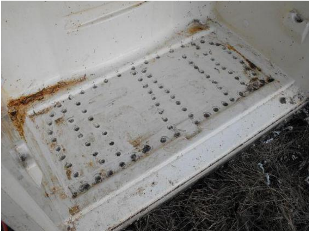
Holes in the bottom of the fridge allow air to come up from underground.
