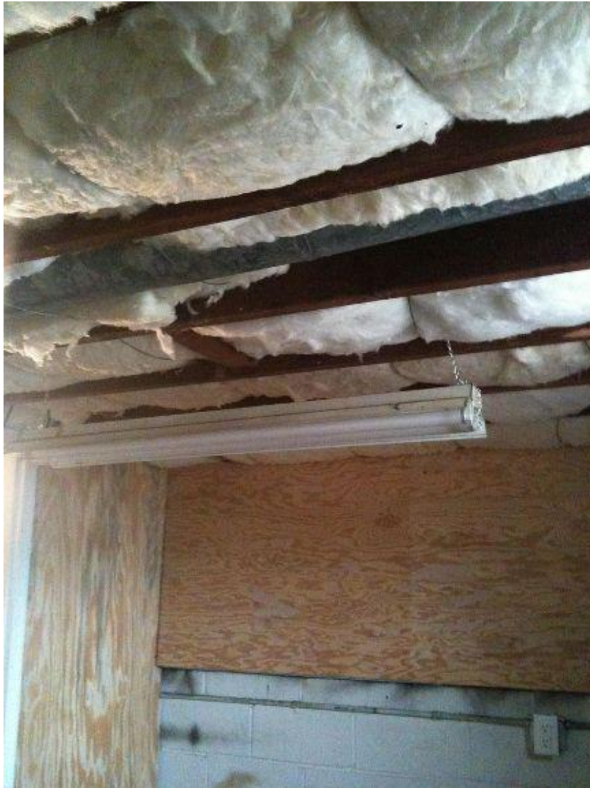
Fiberglass insulation in the ceiling prevented house warmth from seeping down into the root cellar.
