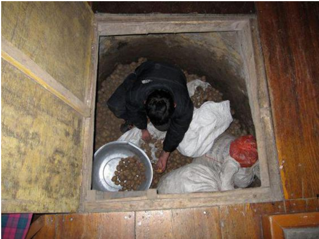
This simple root storage pit is under the dining-room floor.
