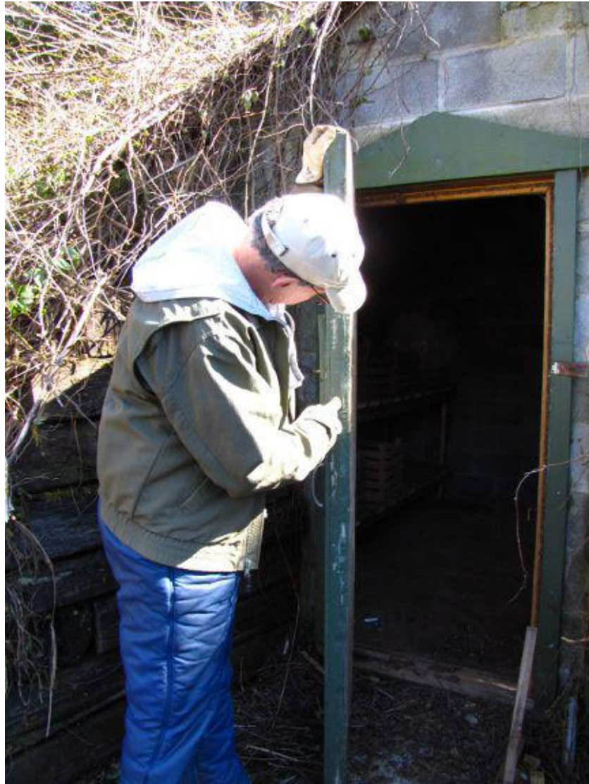
This homemade door is made from plywood sandwiching a 2.25-inch-thick piece of foamboard insulation.
