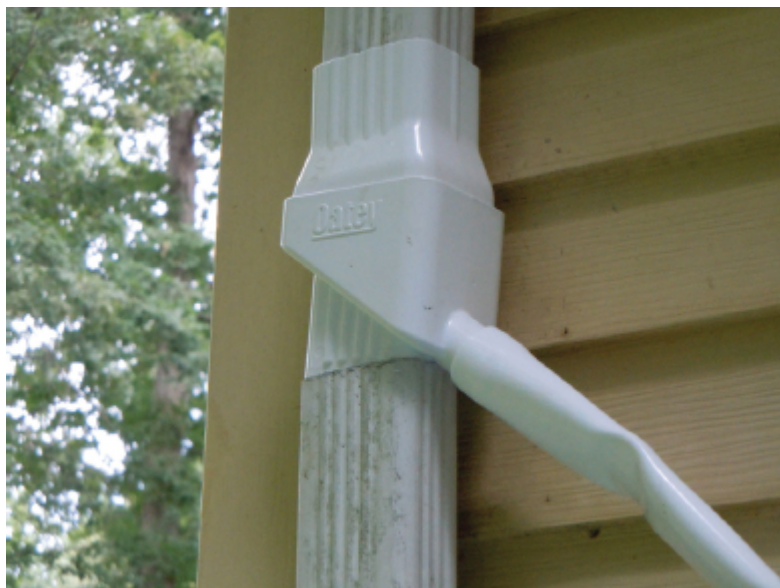
Diverter installed on gutter
