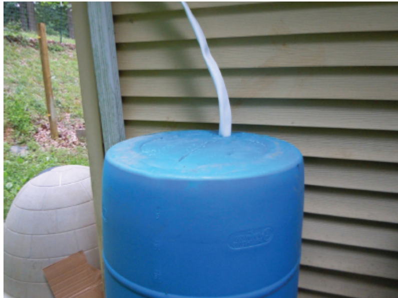
Hose from diverter into barrel
