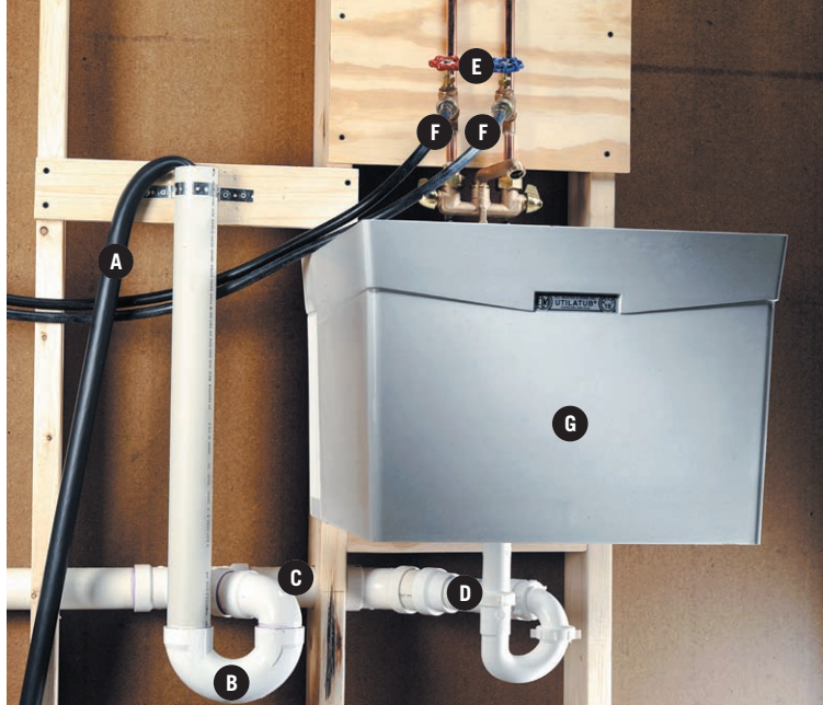
A washing machine with standpipe drain: washing machine drain hose (A), 2" standpipe drain with trap (B), waste line (C), utility sink drain pipe (D), hot and cold supply lines with hose bibs (E), rubber supply hoses to washing machine (F), and utility sink (G).
