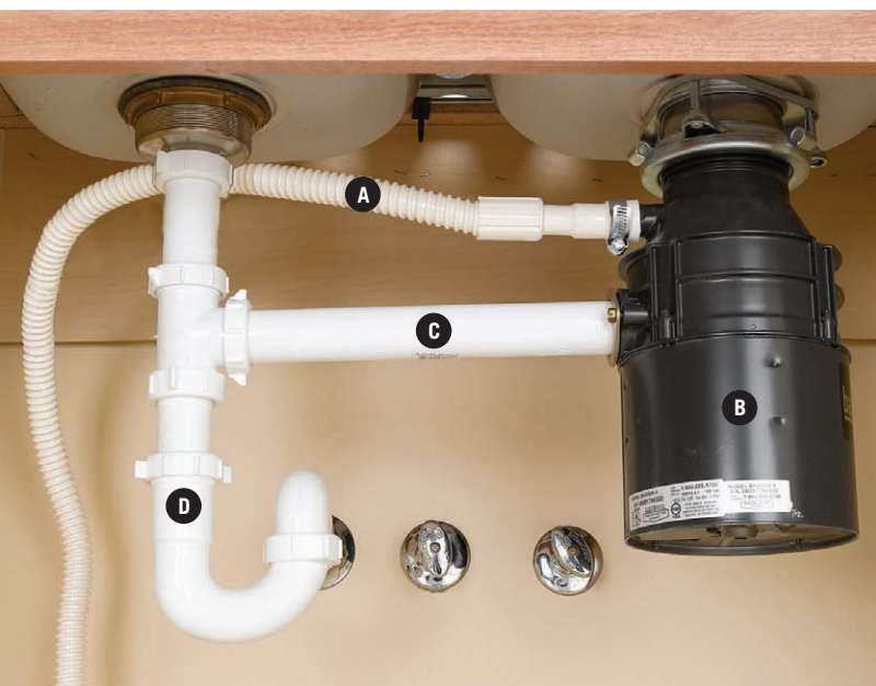
In this arrangement, the dishwasher drain hose (A) attaches to the garbage disposal (B), and a trap arm (C) leads from the disposal to the P-trap (D).
