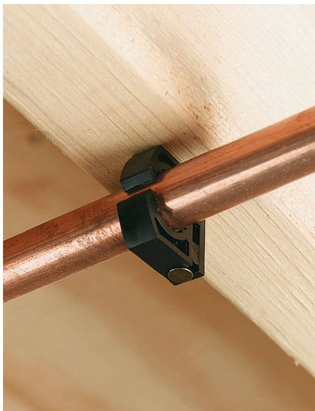
A tube strap holds pipe away from a framing member. Just snap the strap on and drive in a nail.
