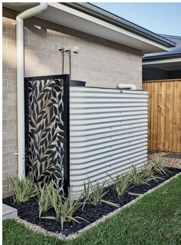
This large gray water reservoir is connected to multiple appliances through the back wall of the home, creating a simple method for irrigating the yard during the dry months.
