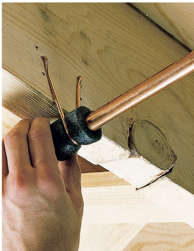
Loose pipes may bang or rub against joist hangers, creating noise. Use pieces of foam rubber pipe insulation to cushion pipes.
