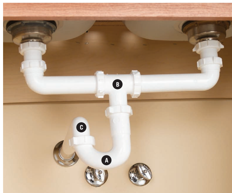
A “center tee” arrangement has a single P-trap (A) that is connected to a waste tee (B) and the trap arm (C).
