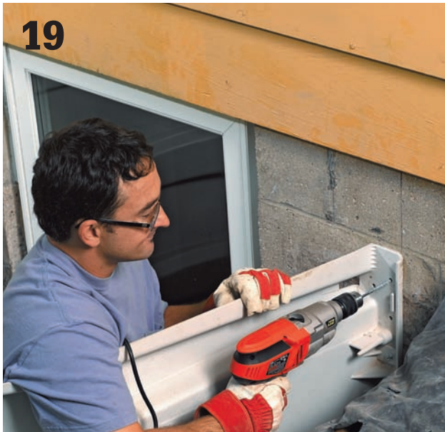
19 Fasten the window well sections to the foundation wall with concrete sleeve anchors driven into pre-bored pilot holes. You could also use masonry nails driven with a powder actuated nailer.
