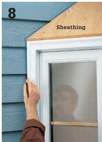
8 Set the roof frame on top of the window, with the sheathing loosely tacked in place. Trace the outline of the window and roof unit onto the siding. Leave a gap of about 1/2" around the roof unit to allow room for flashing and shingles.
