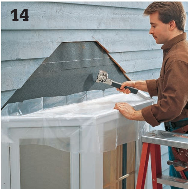
14 Staple sheet plastic over the top of the window unit to serve as a vapor barrier. Trim the edges of the plastic around the top of the window using a utility knife.
