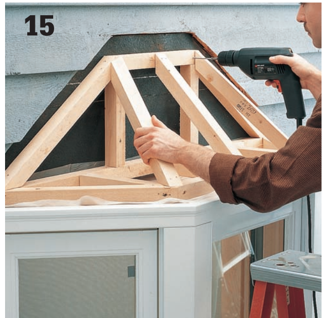
15 Remove the sheathing pieces from the roof frame, then position the frame on top of the window unit. Attach the roof frame to the window and to the wall at stud locations using 3" utility screws.
