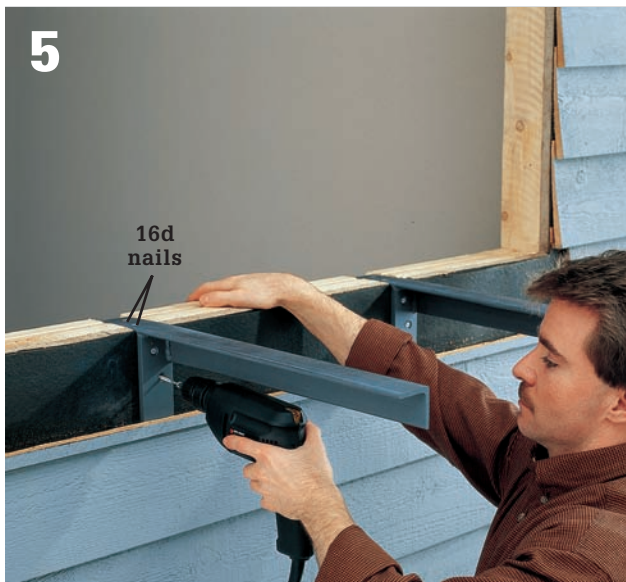
5 Attach the braces to the rough sill with galvanized 16d common nails. Drive 3" utility screws through the front of the braces and into the rough sill to prevent twisting.
