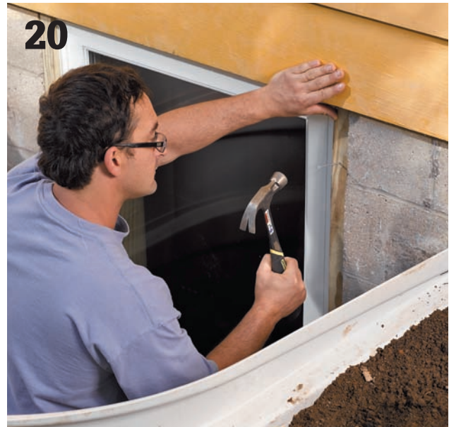
20 When all the well sections are assembled and secured, nail pieces of treated lumber trim around the window frame to hide the nailing flange. Complete the well installation by using excavated dirt to backfill around the outside of the well. Pack the soil with a tamper, creating a slope for good drainage. If you are installing a window well cover, set it in place and fasten it according to the manufacturer's instructions. The cover must be removable.
