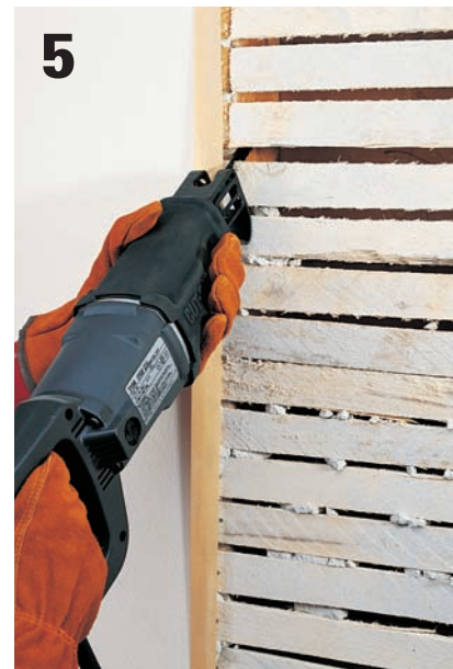
5 Cut through the lath along the edges of the plaster using a reciprocating saw or jigsaw.
