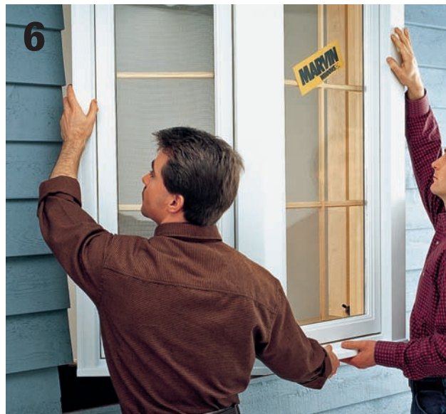
6 Lift the bay window onto the support braces and slide it into the rough opening. Center the unit within the opening.
