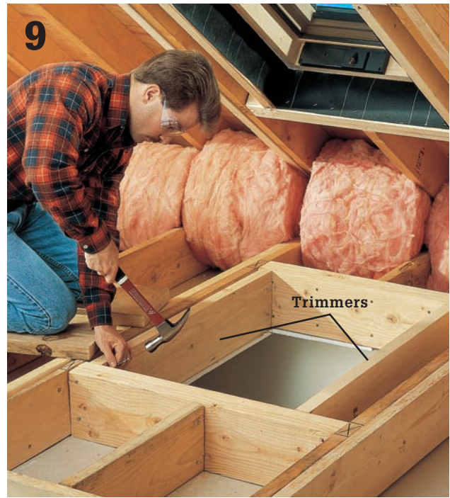
9 Complete the ceiling opening by cutting and attaching trimmers, if required, along the sides of the ceiling cutout between the header and sill. Toenail the trimmers to the header and sill with 10d nails.
