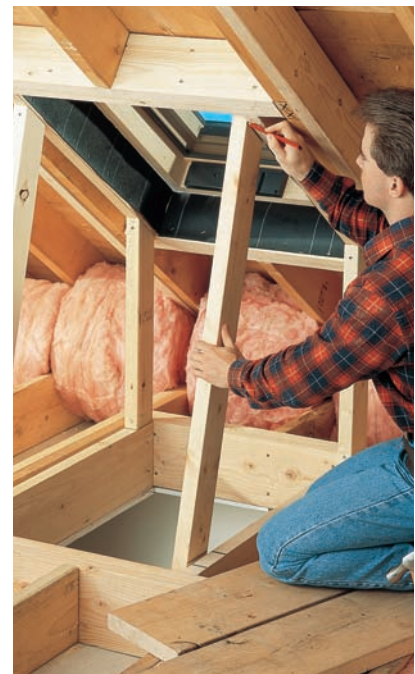
10 Install 2 × 4 corner posts for the skylight shaft. To measure for the posts, begin with a 2 × 4 that is long enough to reach from the top to the bottom of the shaft. Hold the 2 × 4 against the inside of the framed openings, so it is flush with the top of the rafter header and the bottom of the joist header (left photo). Mark cutting lines where the 2 × 4 meets the top of the joist or trimmer and the bottom of the rafter or trimmer (right photo). Cut along the lines, then toenail the posts to the top and bottom of the frame with 10d nails.
