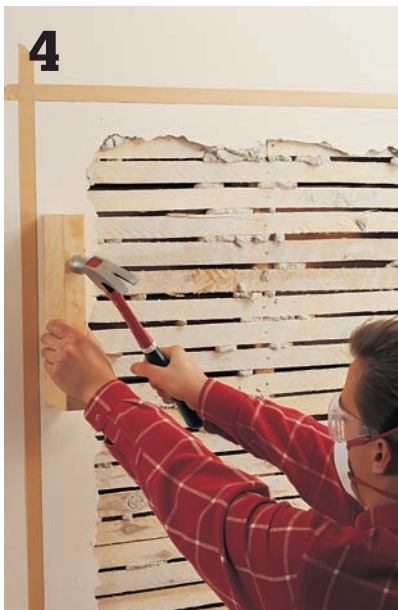
4 Break the plaster along the edges by holding a scrap piece of 2 × 4 on edge just inside the scored line and rapping it with a hammer. Use a pry bar to remove the remaining plaster.
