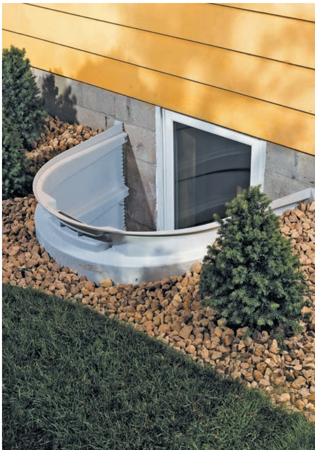
Replacing a small basement window with an egress window is a big job, but it is required if you want to convert part of a basement into livable space, especially a bedroom.
