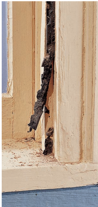
Weather stripping and insulation may begin to deteriorate. Telltale signs include crumbling foam or rubber.
