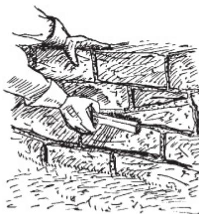
*A wire brush and water will eventually remove mortar stains from stone.*
